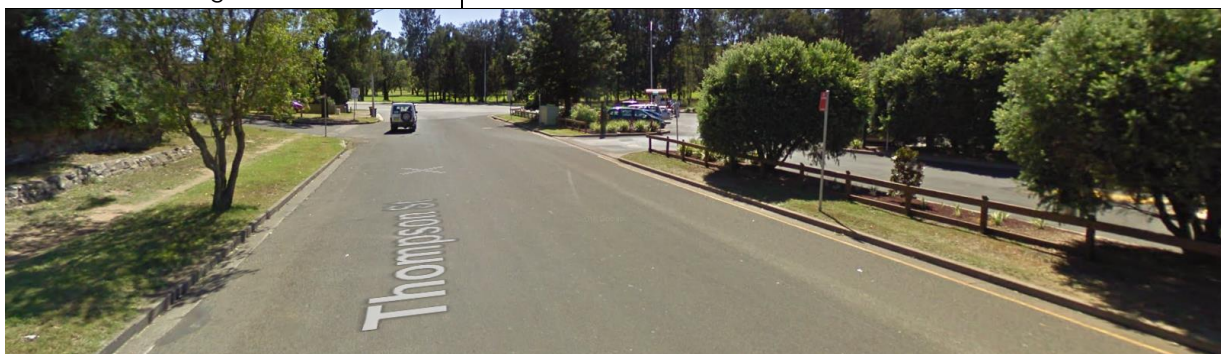
Figure 9 – Thompson Street – Northbound towards Maitland Street
