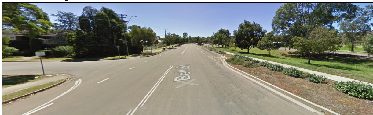
Figure 10 – Bell Street – Northbound towards Clifford Street
