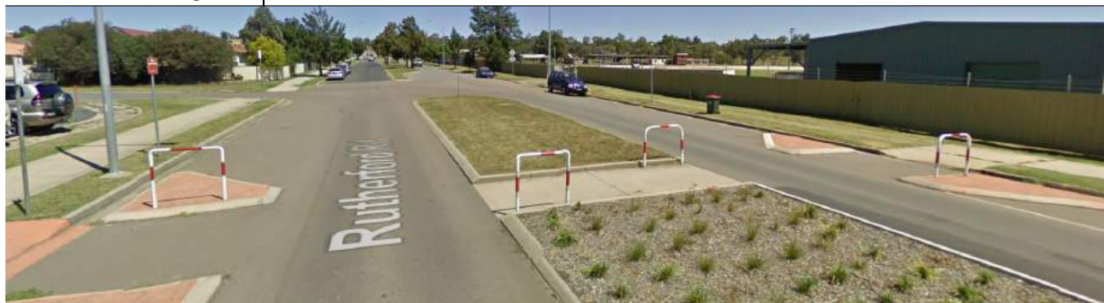
Figure 26 – Rutherford Road – Southwestbound towards Arcacia Drive
