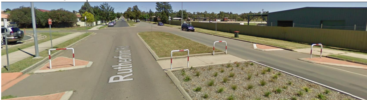
Figure 26 – Rutherford Road – Southwestbound towards Arcacia Drive
