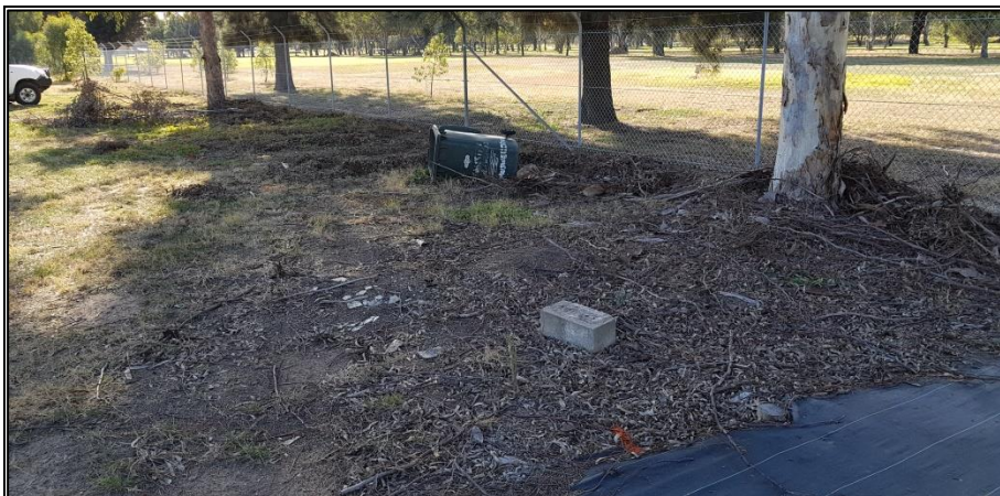
Figure 8: Fibrous cement fragments encountered adjacent to the northern boundary in the south eastern portion of the site, looking north
