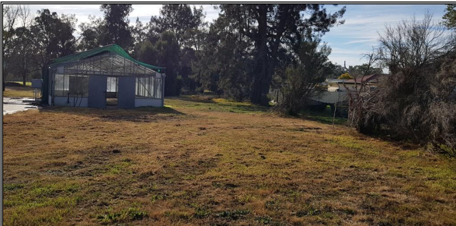
Figure 2: Glasshouse in the south eastern portion of the site, looking north
