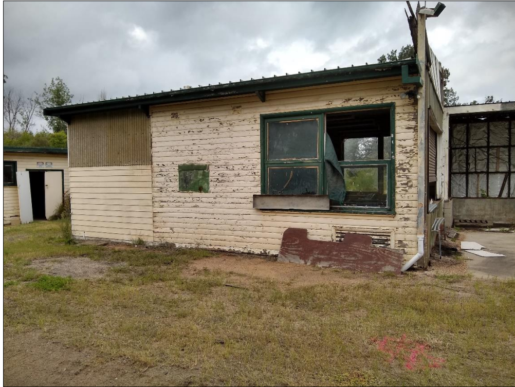
Figure 17: Typical surface area along the north eastern side of Building 5.
