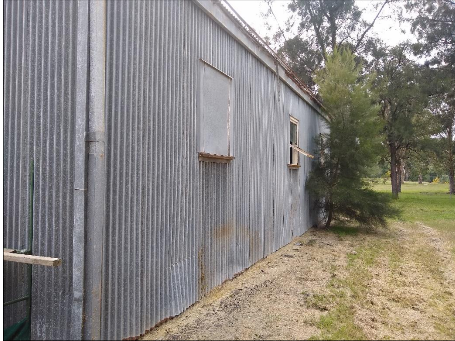
Figure 25: Typical surface area around Building 9.
