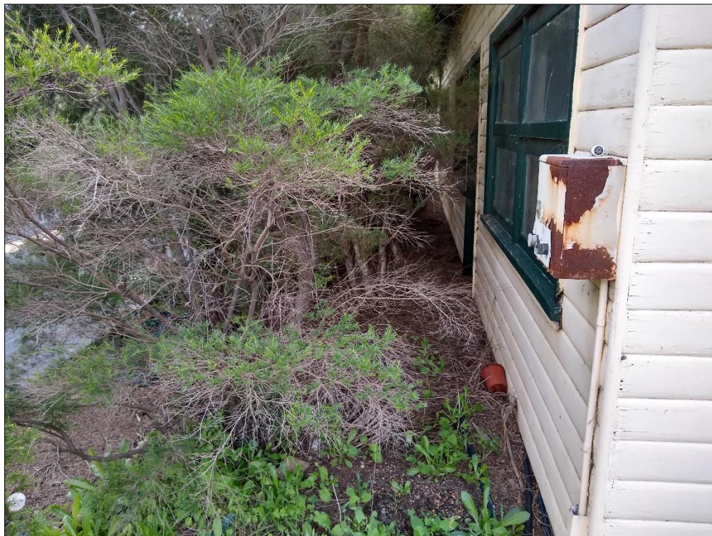
Figure 22: Garden bed running along the south western face of Building 8.
