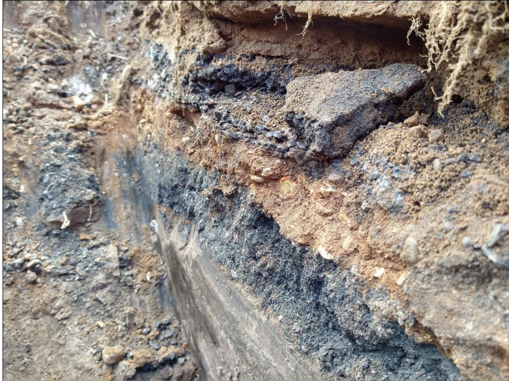
Figure 37: Photo of buried asphalt from test pit 106A (upper dark grey materials and ash filling (lower dark grey materials)).
