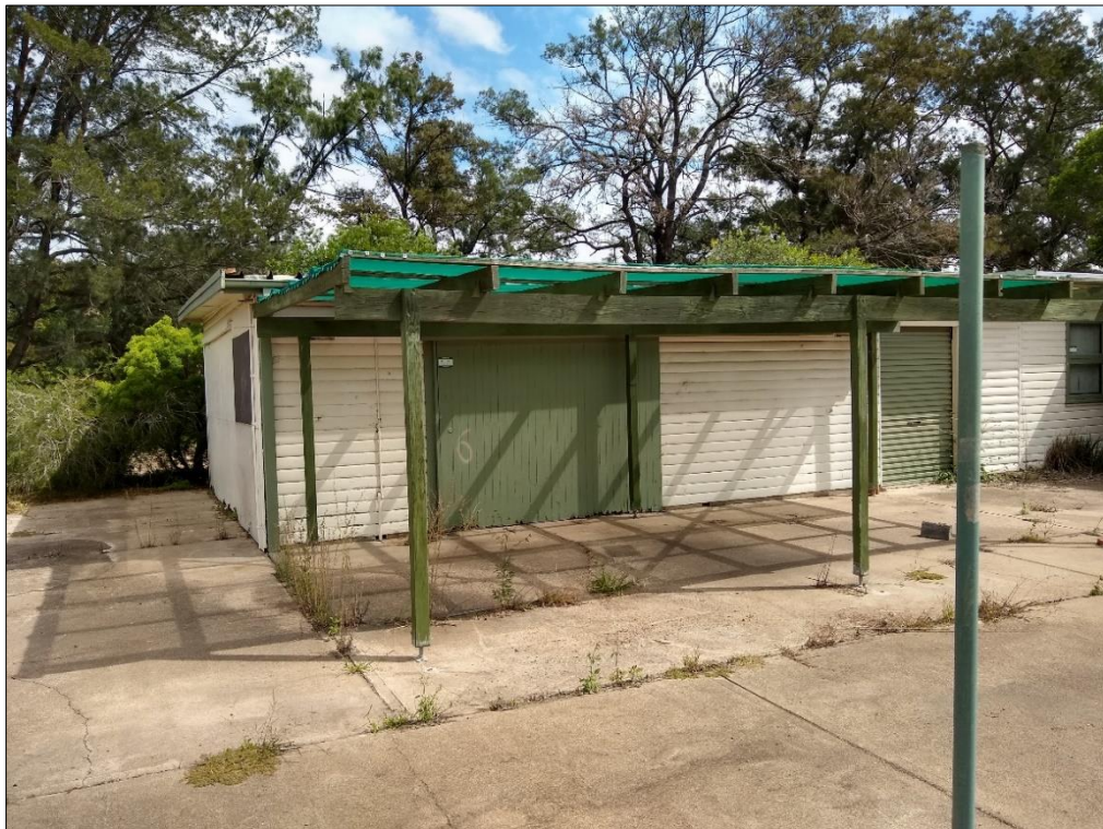
Figure 30: Typical surface area along north western face of Building 6.
