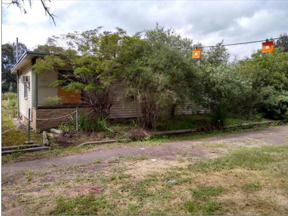
Figure 29: Garden bed located along the western face of Building 6.
