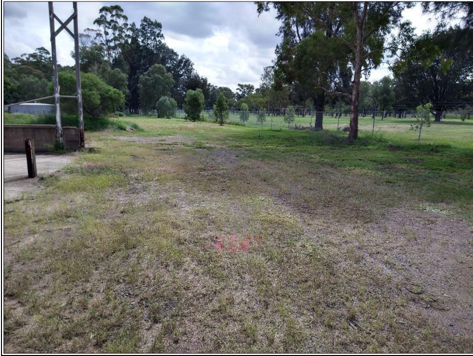
Figure 5: Area of buried asphalt access track, north of the Building 5, looking west.
