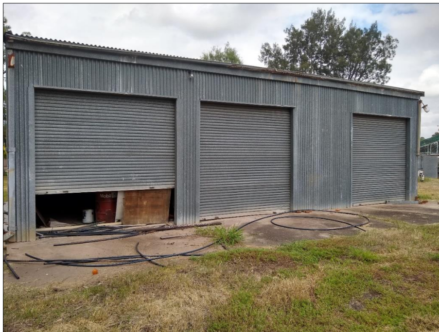
Figure 24: Concrete pavements located along the north western face of Building 9.
