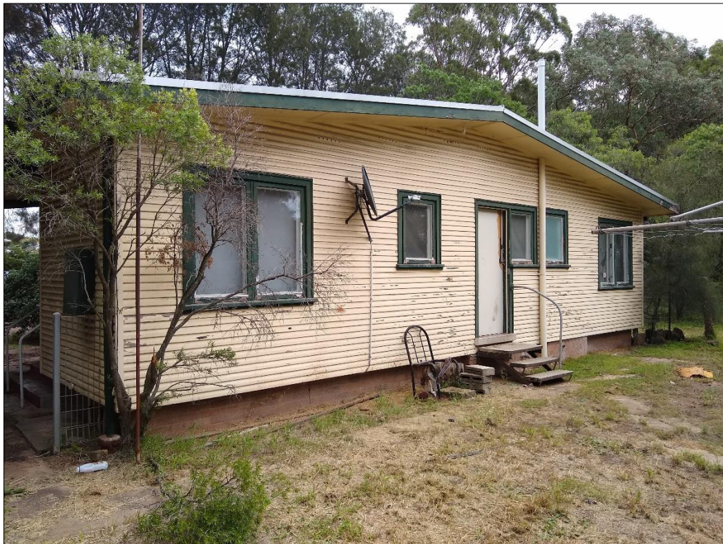
Figure 34: Surface area along the eastern face of Building 1.
