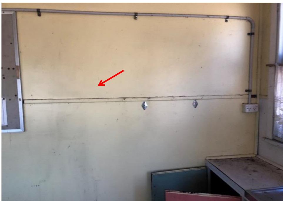
Photograph 55: Rear Office, internal , walls, yellow paint, lead paint (>0.1% lead w/w).
