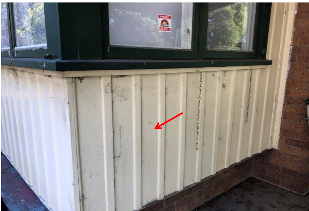
Photograph 3: Residential Dwelling, external , walls, fibre cement sheet, asbestos detected by analysis.
