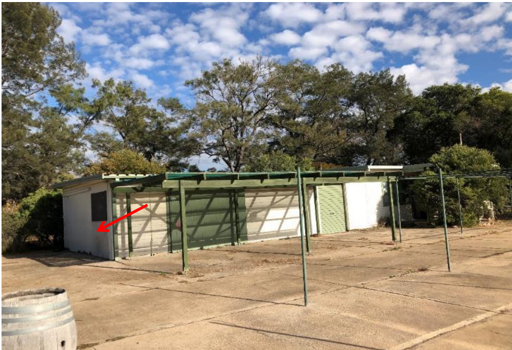
Photograph 36: Front Office, external, walls, south end, fibre cement sheet, no asbestos detected by analysis.
