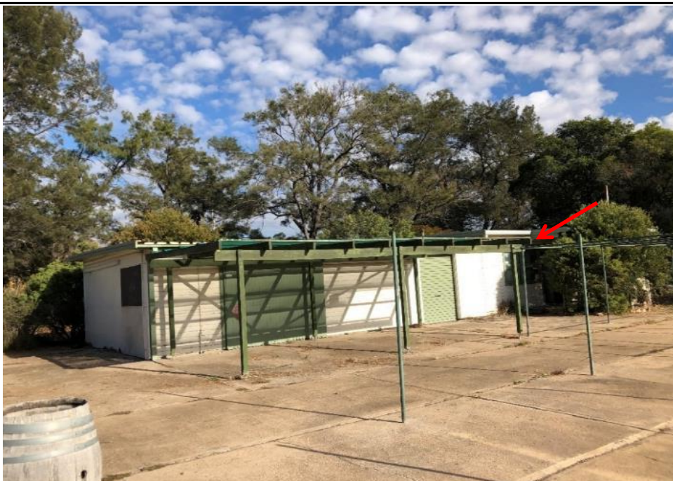
Photograph 47: Front Office, external, eaves to north, fibre cement sheet, no asbestos detected by analysis.
