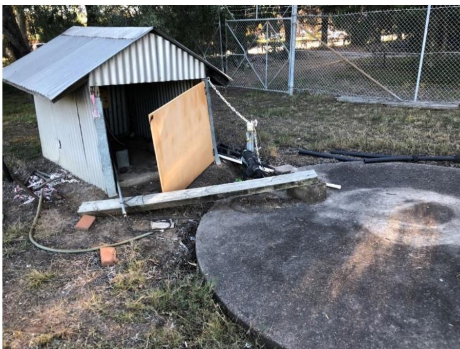
Photograph 20: Concrete water tank (in ground).
