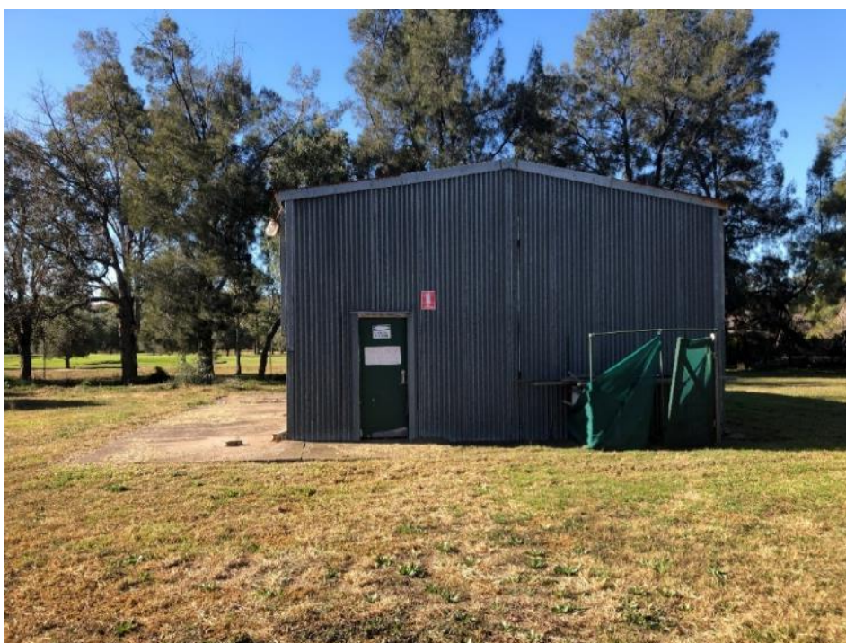
Photograph 62: Machinery and HAZMCHM shed.
