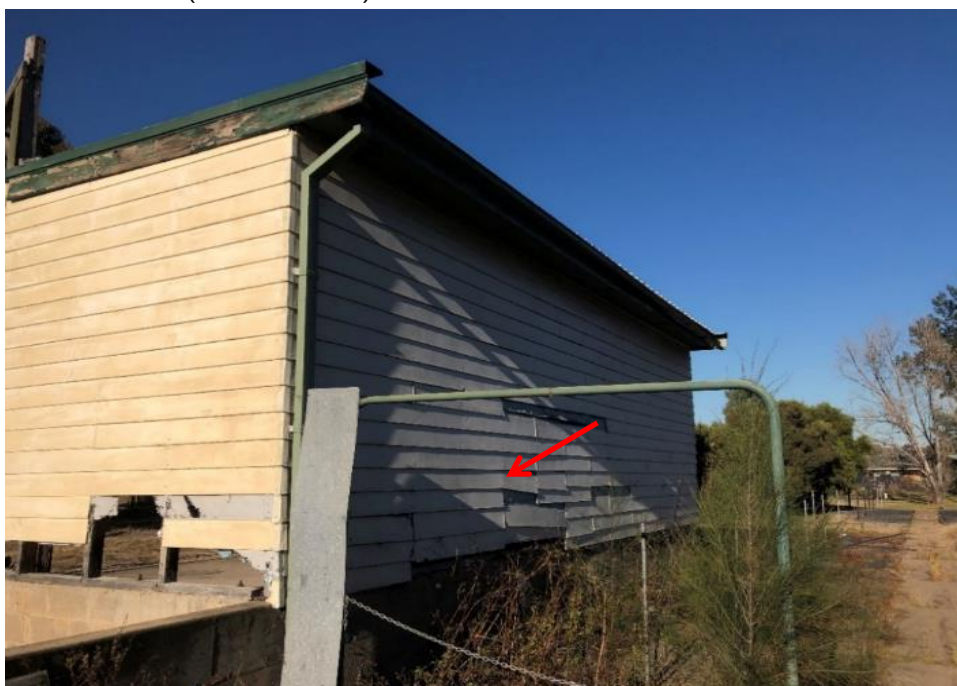
Photograph 23: Potting shed, external , corrugated sheet metal, green paint, lead paint (>0.1% lead w/w).
