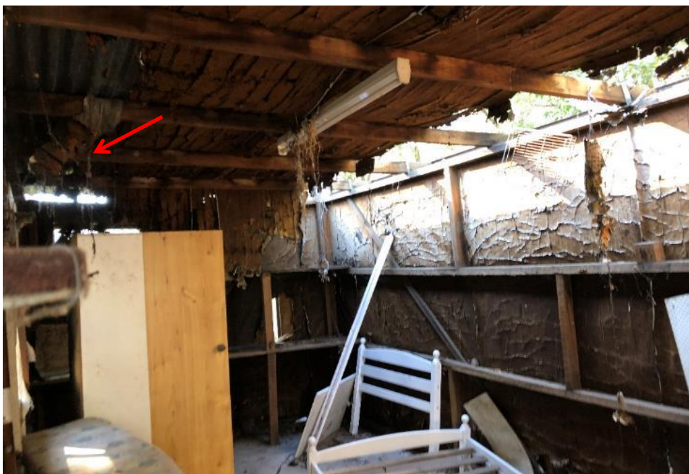
Photograph 18: Rear Shed, roof, insulation blanket, insulation, SMF (assumed).
