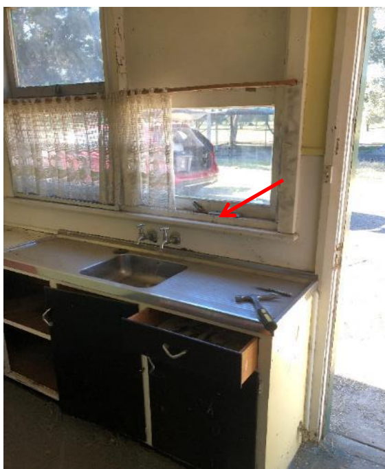
Photograph 55: Rear Office, internal , walls, yellow paint, lead paint (>0.1% lead w/w).
