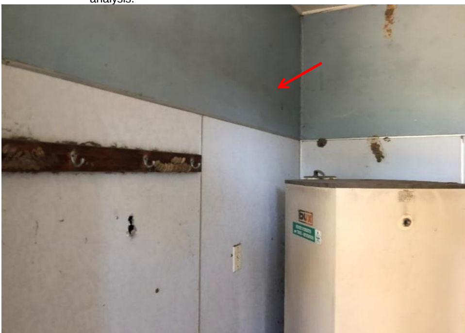
Photograph 57: Rear Office, internal , walls, fibre cement sheet, asbestos detected by analysis.
