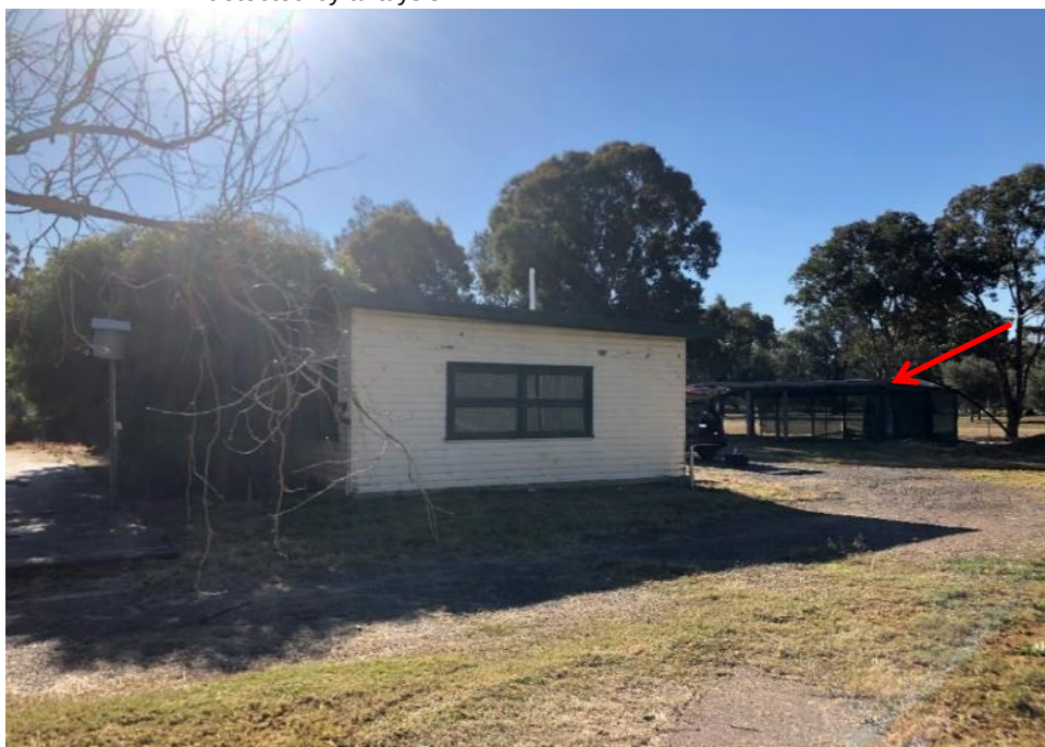
Photograph 47: Front Office, external, eaves to north, fibre cement sheet, no asbestos detected by analysis.
