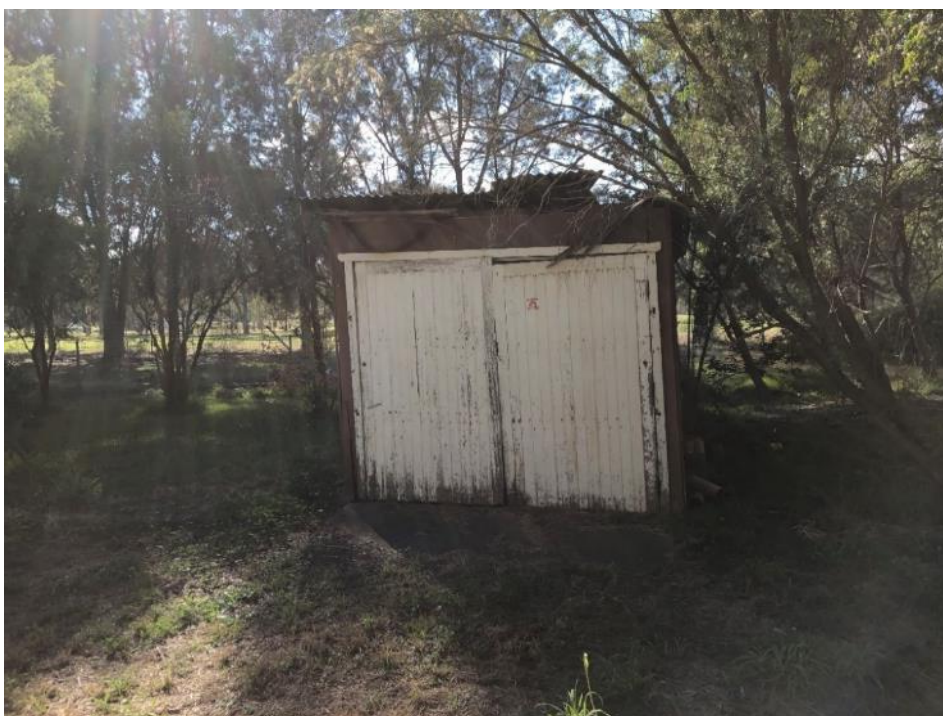
Photograph 17: Timber shed to rear of residential dwelling.
