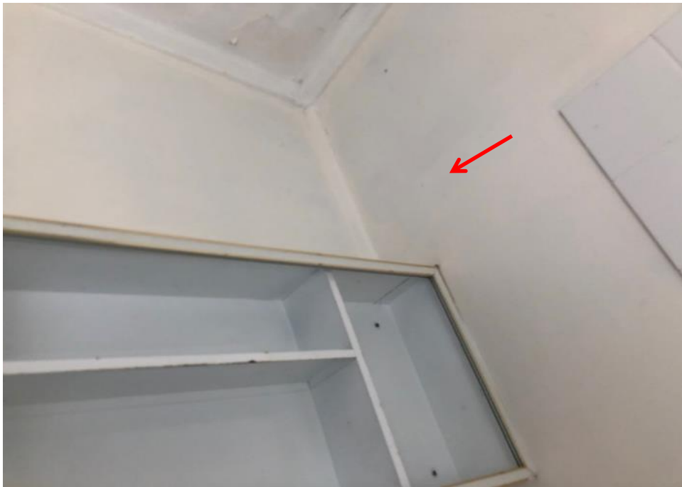
Photograph 11: Residential Dwelling, internal , walls to laundry, fibre cement sheet, no asbestos detected by analysis.
