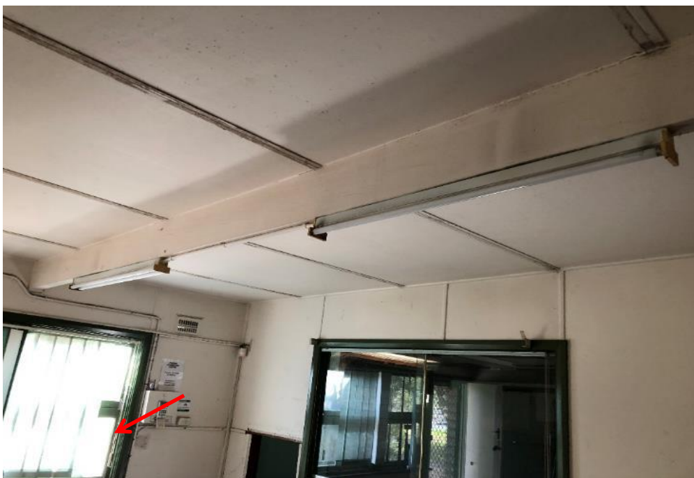
Photograph 45: Front Office, internal , windows and architraves, green paint, non-lead paint (≤0.1% lead w/w).
