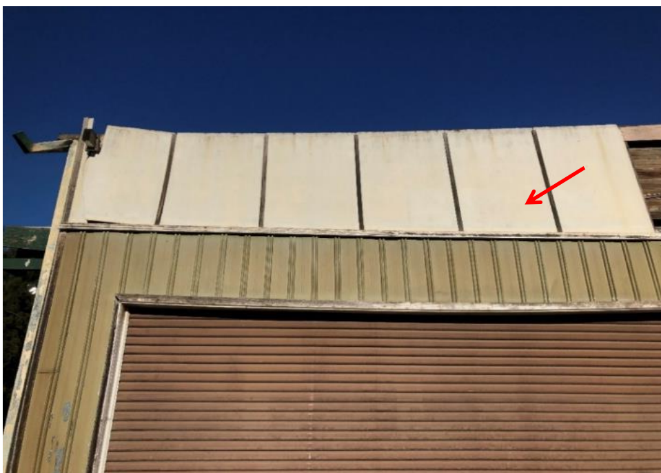
Photograph 25: Potting shed, external , walls, fibre cement sheet, no asbestos detected by analysis.
