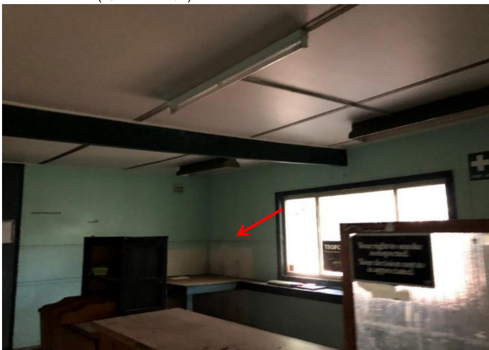
Photograph 45: Front Office, internal , windows and architraves, green paint, non-lead paint (≤0.1% lead w/w).
