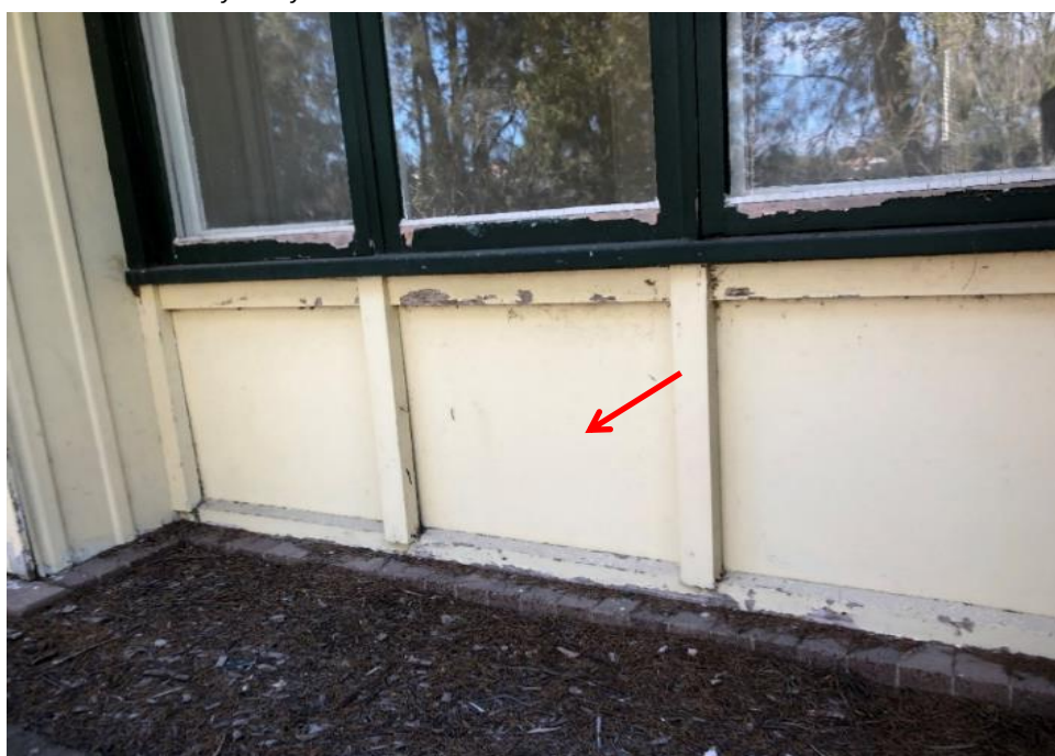
Photograph 3: Residential Dwelling, external , walls, fibre cement sheet, asbestos detected by analysis.
