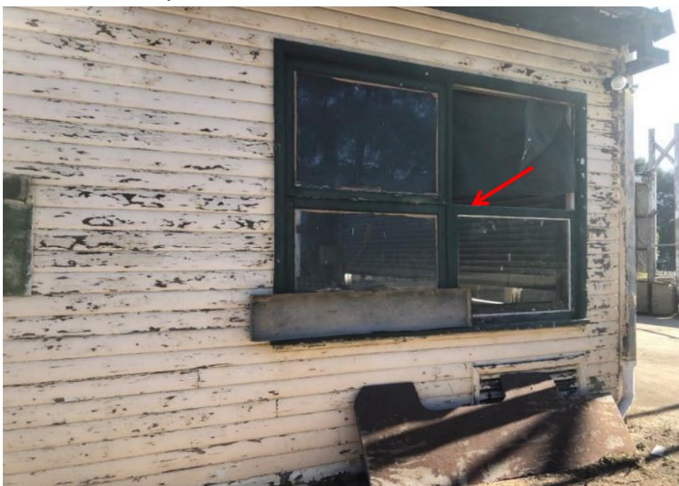
Photograph 25: Potting shed, external , walls, fibre cement sheet, no asbestos detected by analysis.
