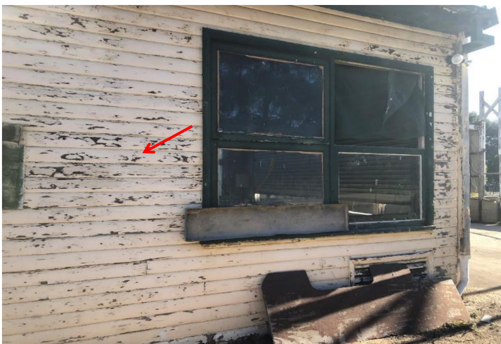
Photograph 22: Potting shed, external , walls, cream paint, lead paint (>0.1% lead w/w).
