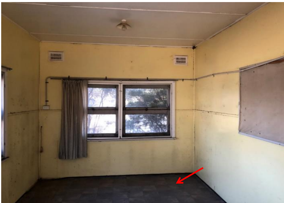
Photograph 54: Rear Office, internal , floors, vinyl floor sheet, no asbestos detected by analysis.
