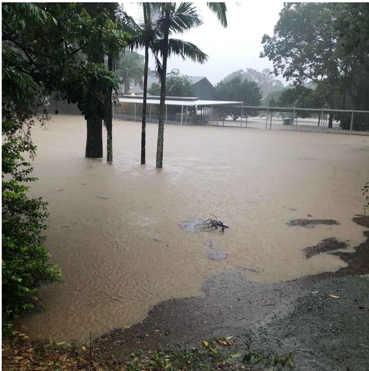
MEPS site and buildings flood impacted
