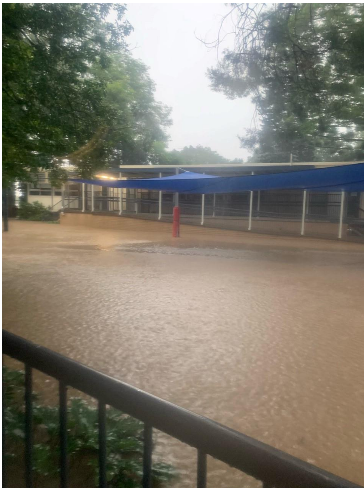
MEPS main site flood impacted
