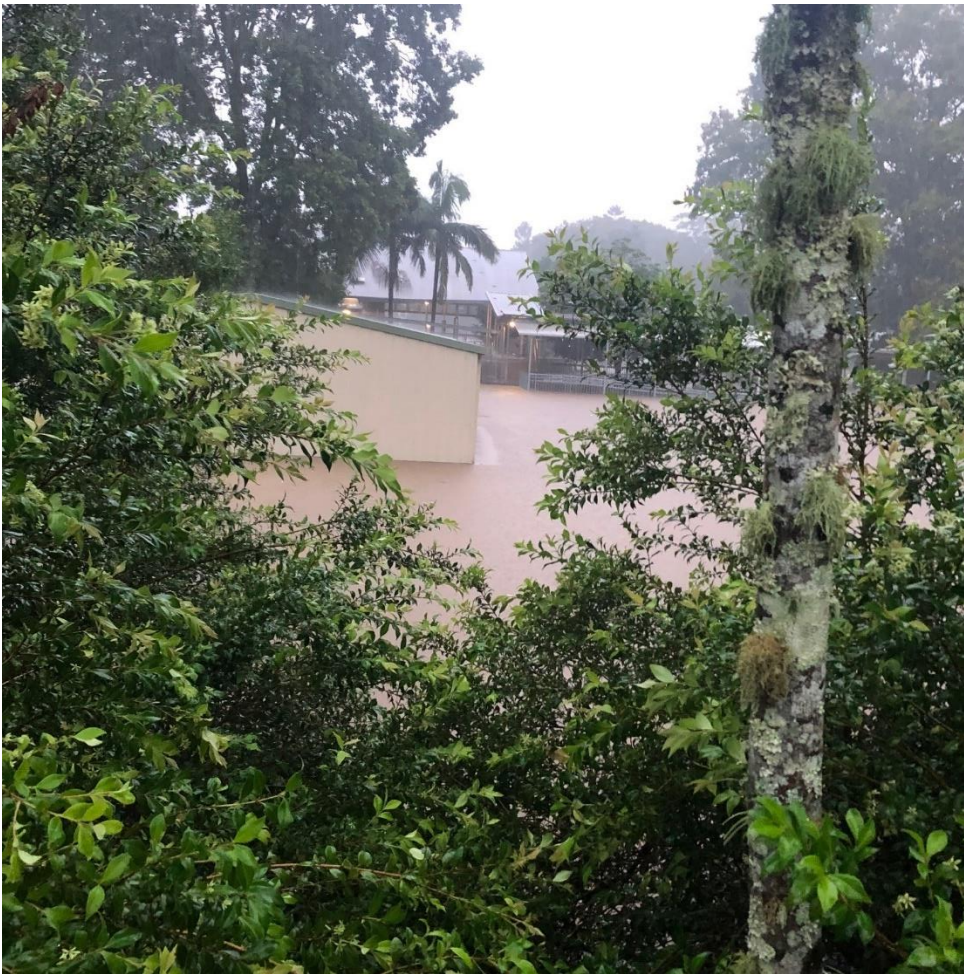
MEPS site and buildings flood impacted
