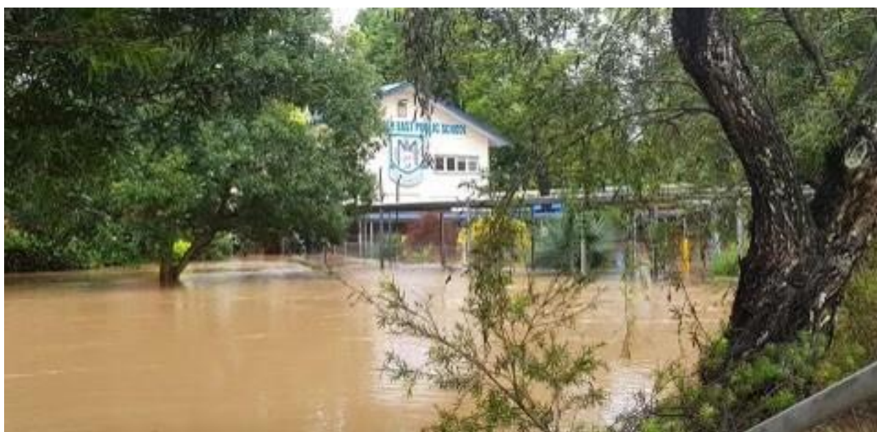
MEPS site and buildings flood impacted
