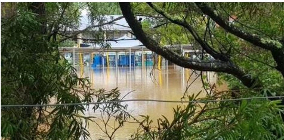
MEPS building flood impacted
