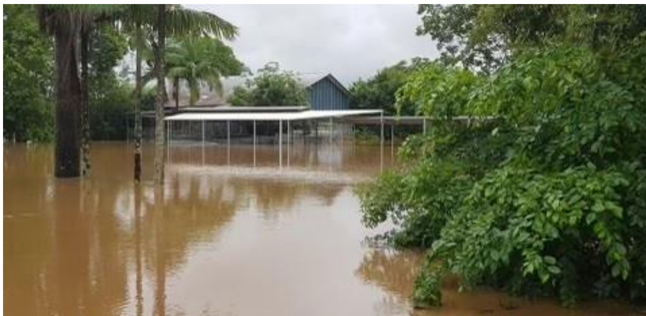
MEPS site and buildings flood impacted
