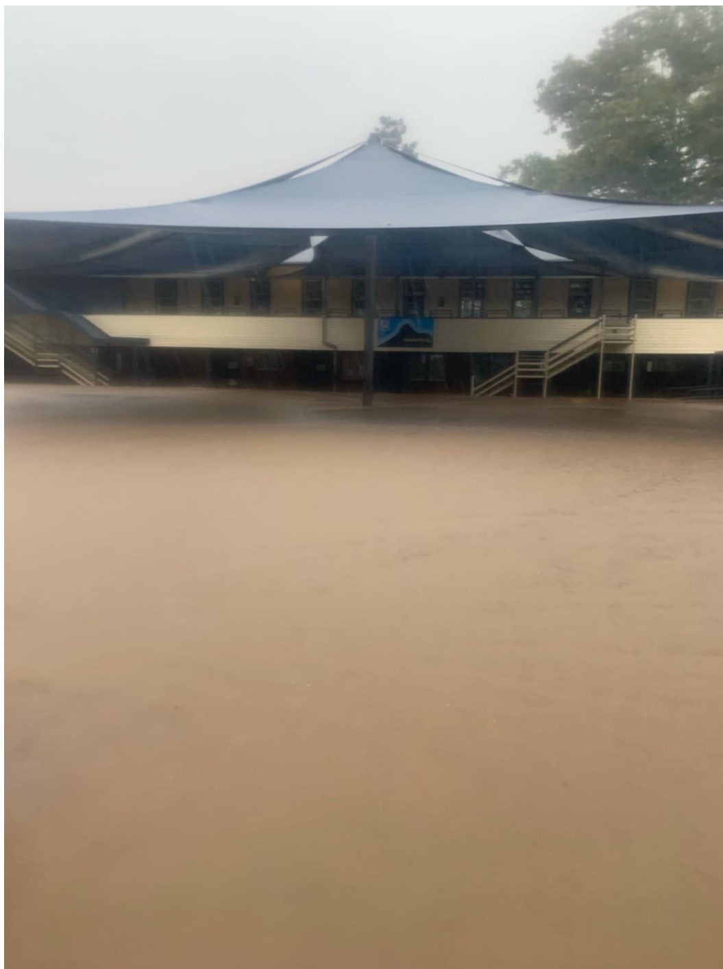
MEPS building flood impacted
