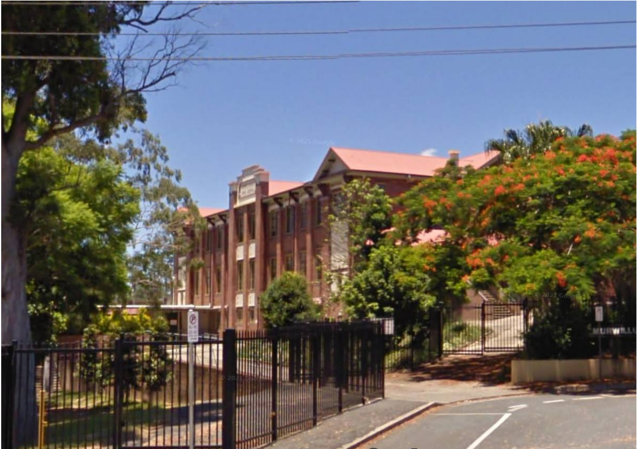
View 1 - View towards building A from existing drop off on Riverview Streets - Existing Image
