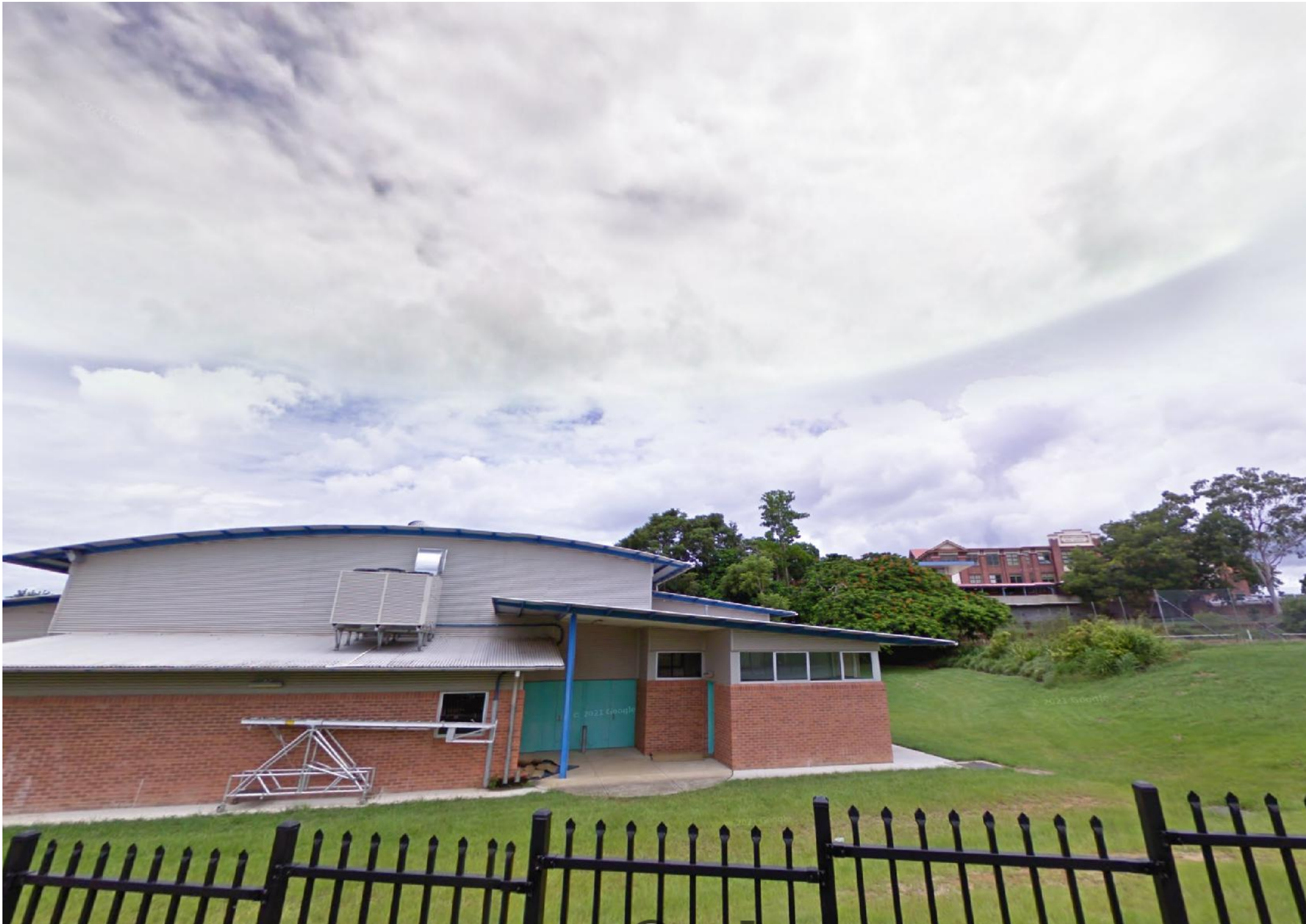
View 5 - View south towards existing building A from neighbouring lot, 84B Riverview Street - Existing Image
