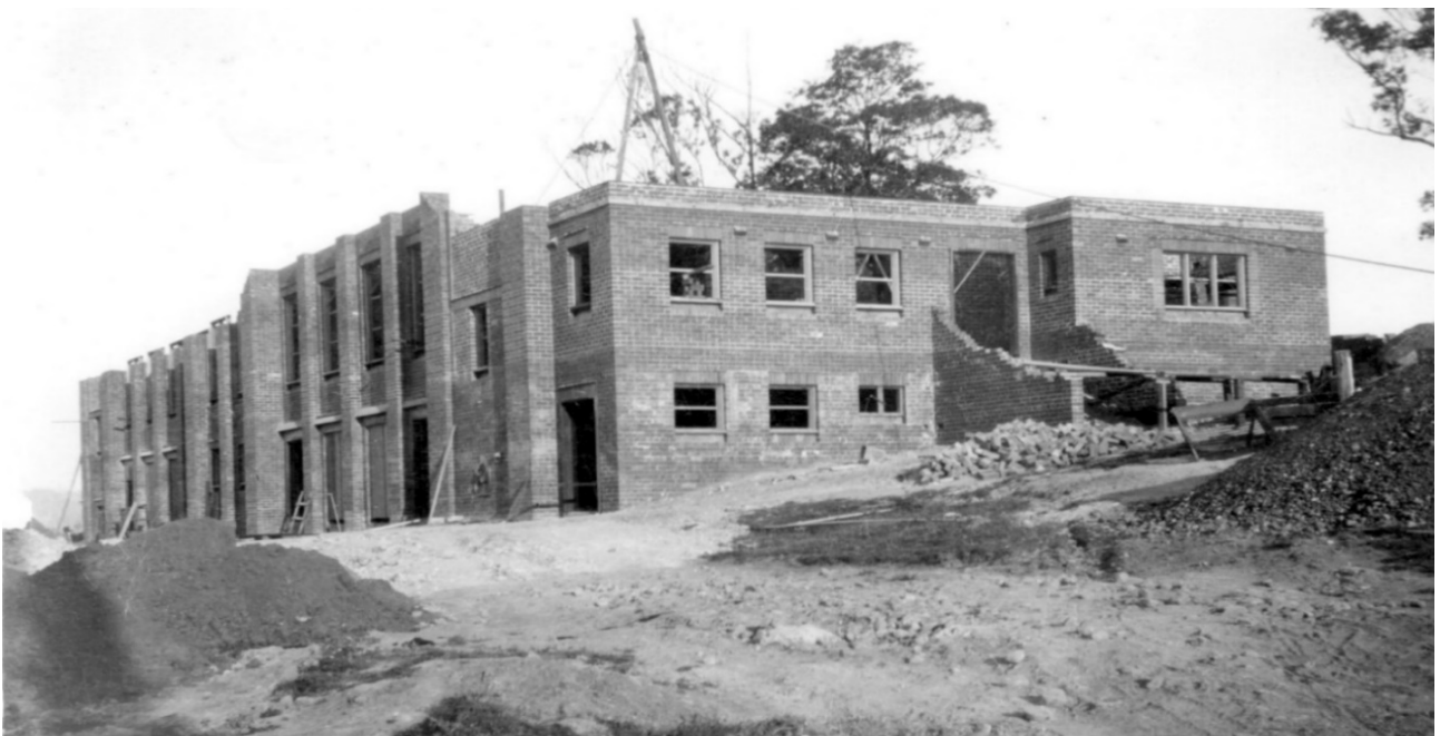
Plate 3.3 Construction of Murwillumbah High School with lower floors c. 1928. Source: M12-33, Tweed Regional Museum archives. Photographer Unknown.
