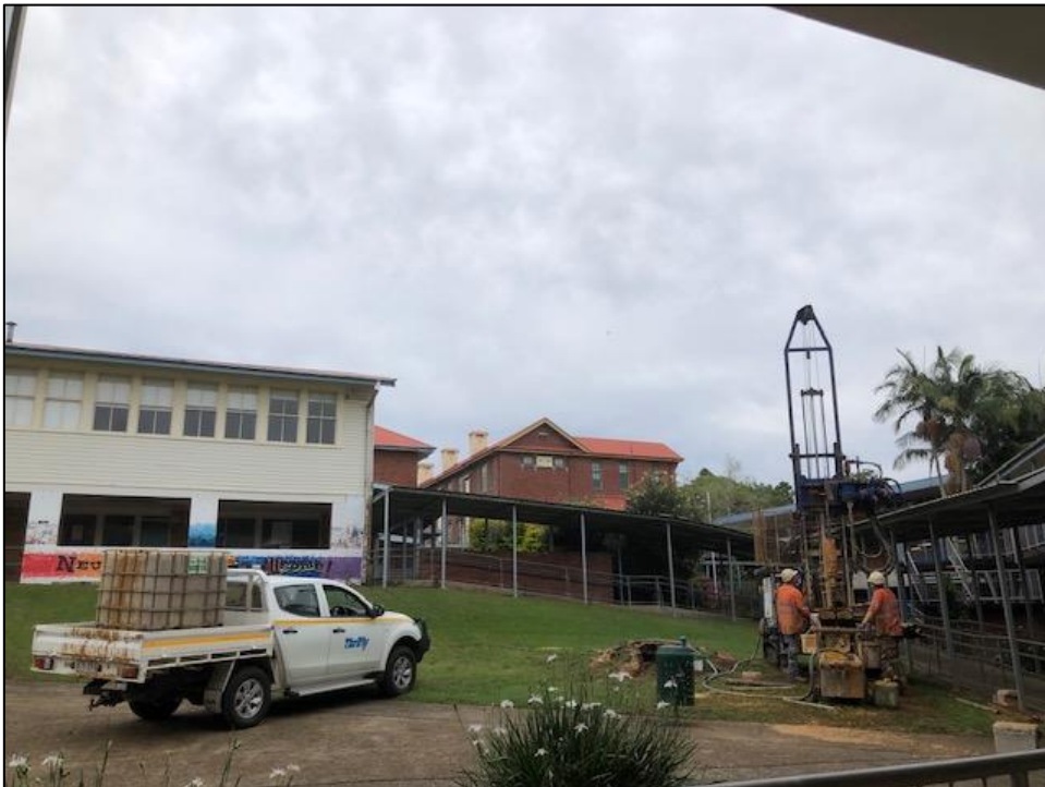
Figure 3: Typical site conditions during investigation looking west at drill rig set up at Bore 105.
