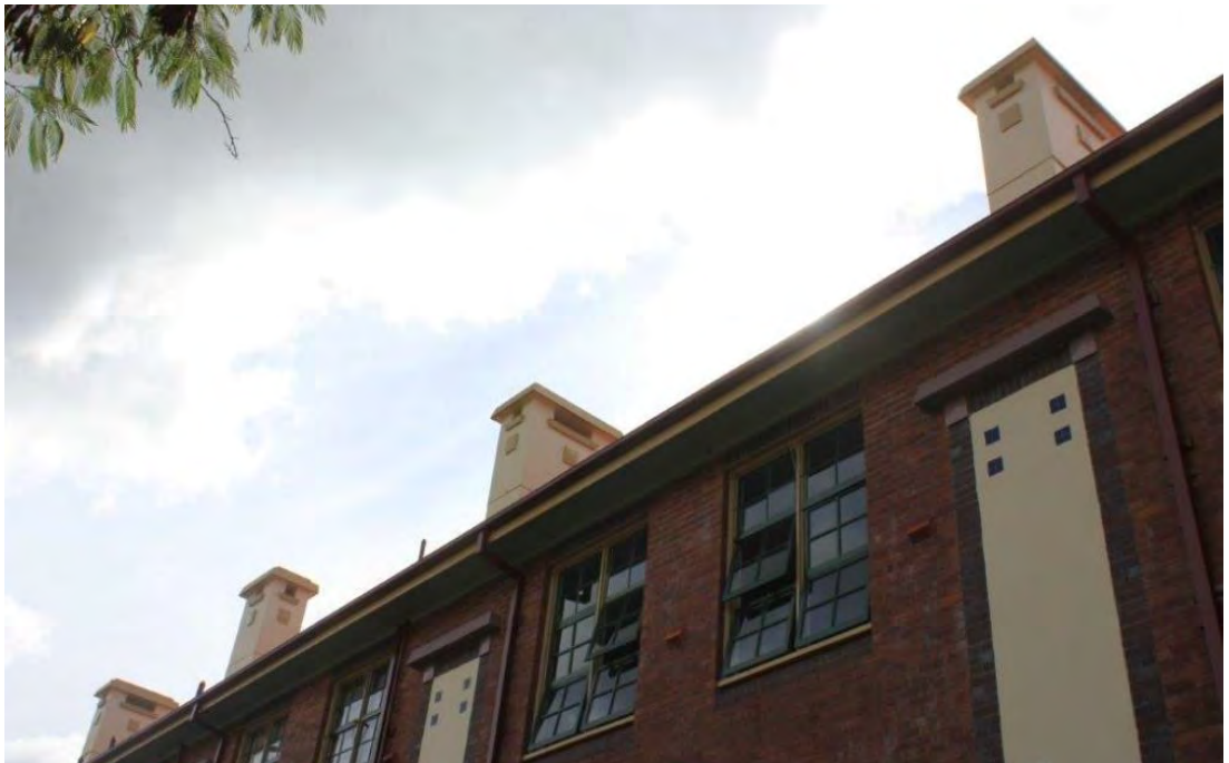
Plate 5.11 View of Block A south elevation and chimney shafts. Source: EMM 2021.
