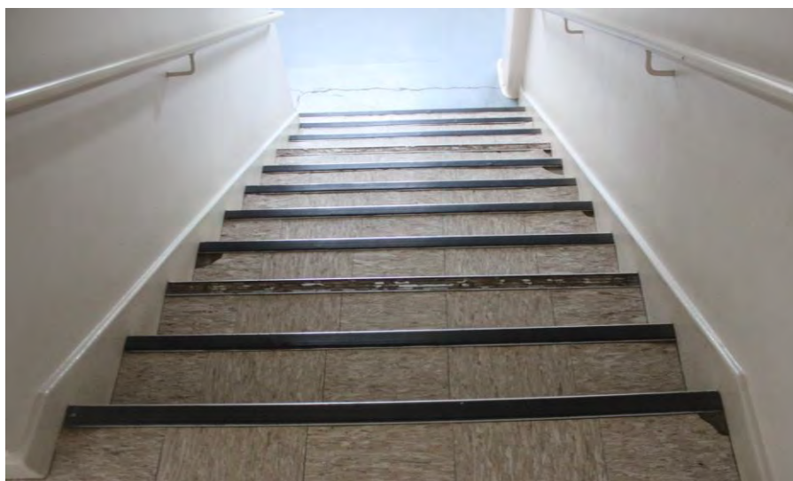
Plate 9.6 Western Block A stairway with vinyl flooring. Source: EMM 2021.
