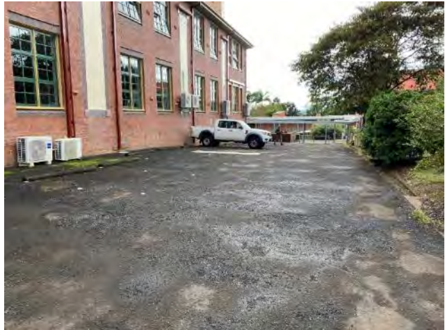
Plate 7.6 Asphalt car parking zone to south of Block A. Source: EMM 2021.
