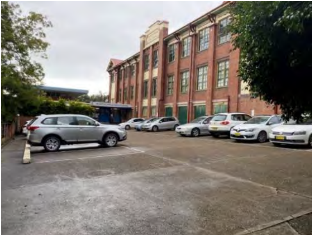
Plate 7.5 Asphalt car parking zone to north of Block A. Source: EMM 2021.
