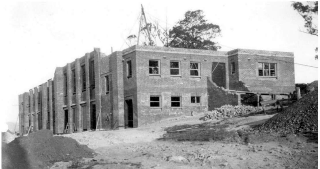
Plate 4.6 Construction of Murwillumbah High School with lower floors c. 1928. Source: M12-33, Tweed Regional Museum archives. Source: Tweed Regional Museum Archives (unknown photographer).
