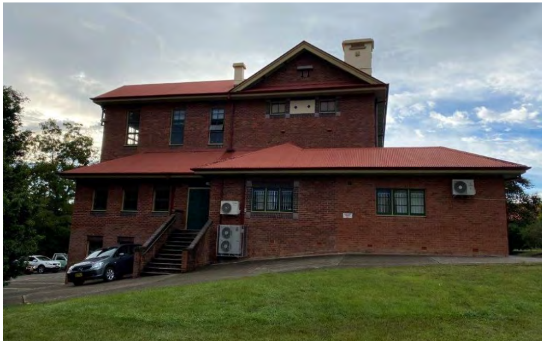
Plate 5.9 View of the Block A western elevation and entry way indicating change in elevation from north to south. Source: EMM 2021.
