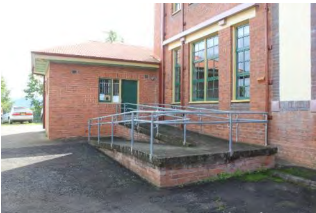
Plate 7.3 Disabled access ramp to extension. Source: EMM 2021.
