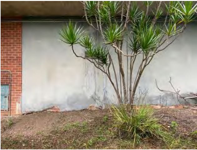
Plate 7.7 Mid-twentieth century extension. Source: EMM 2021.
