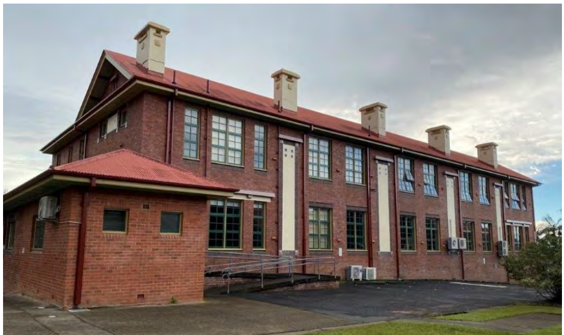
Plate 5.8 View of the Block A south elevation. Source: EMM 2021.
