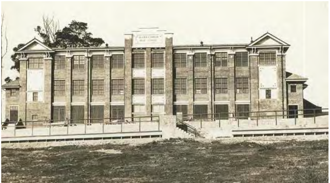
Plate 4.8 Murwillumbah High School building at the finalisation of its construction c. 1929 showing original features including timber batten gates (highlighted in blue) for entryways to the basement level. Source: M19-17, Tweed Regional Museum archives. Photographer Unknown.
