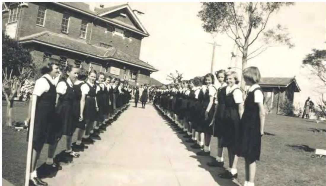
Plate 4.11 Pathway leading to the Block A building c.1950 indicating original paved floor finish and the now demolished boys closet block to the foreground (rear right). Source: M19-27, Tweed Regional Museum archives. Photographer Unknown.
