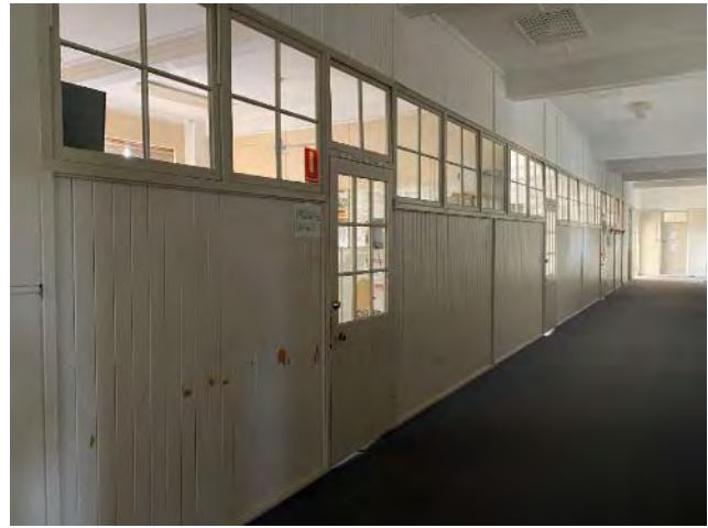
Plate 5.27 Level 2 – main hallway and later partition wall. Source: EMM 2021.
