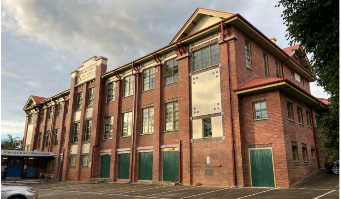
Plate 5.5 View of the Block A facade (north elevation). Source: EMM 2021.
