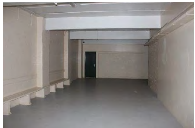
Plate 5.17 Ground Level - eastern vacant space. Source: EMM 2021.
