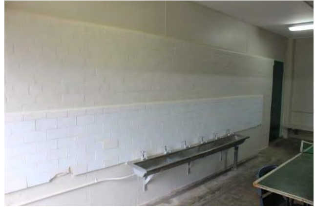
Plate 5.15 Ground Level - Storage partition wall. Source: EMM 2021.
