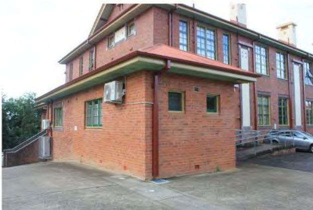
Plate 7.1 Mid-twentieth century extension. Source: EMM 2021.
