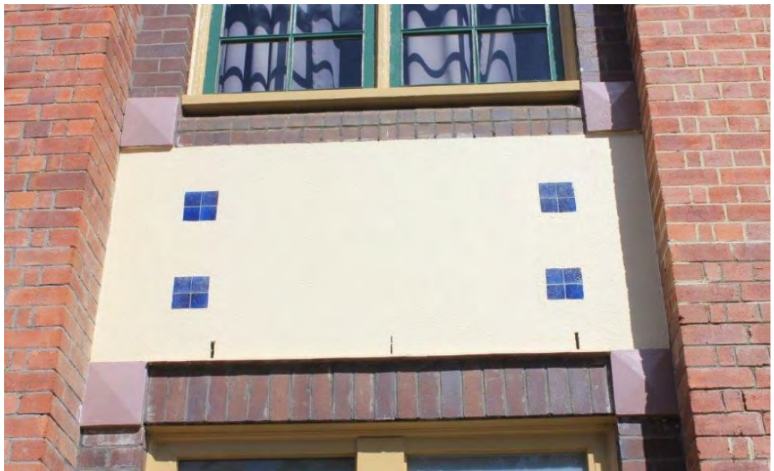
Plate 5.7 View of facade detail to north elevation. Source: EMM 2021.
