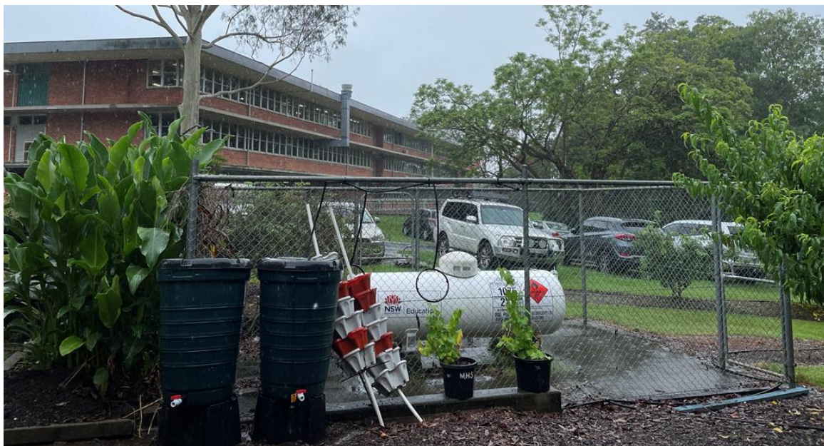
Figure 7 Existing Bulk LPG Tank Compound
