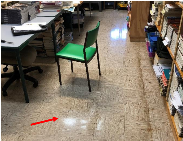
Photo 10: Building A - Asbestos vinyl floor tiles to AR1005
