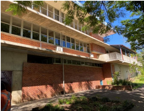
Photo 16: Building E overview
