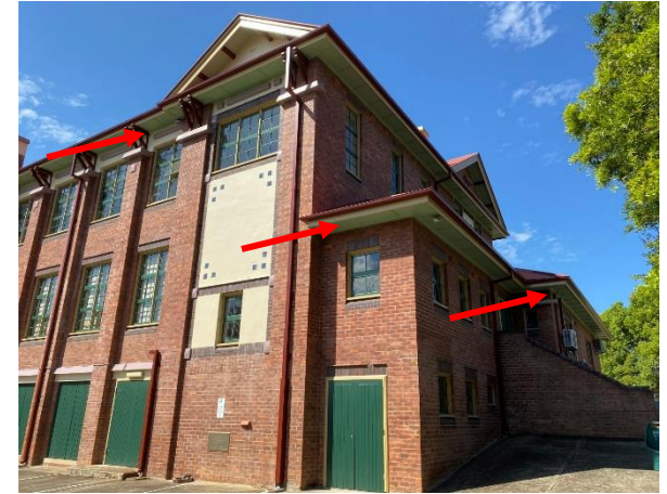
Photo 3: Building A – Asbestos flat sheet eaves to all levels and faces
