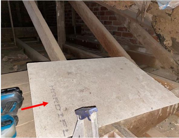
Photo 13: Building A - Assumed ACM access hatch to ceiling space from AR1007
