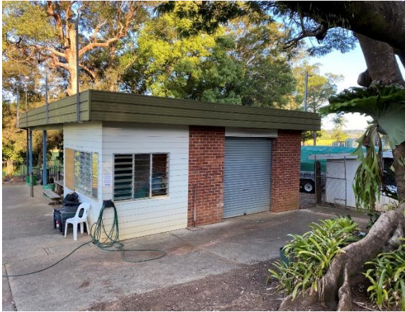
Photo 31: Building AY overview
