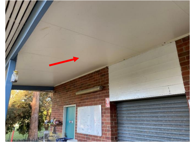
Photo 33: Building AY – Asbestos flat sheet ceiling lining to AYR0001
