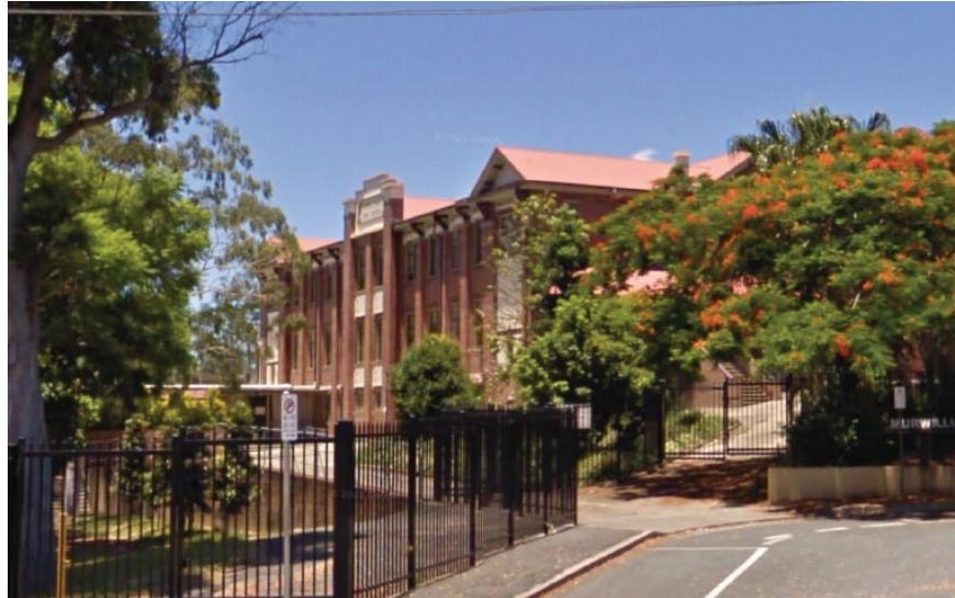
Figure 50 Current View 1 (photo)
