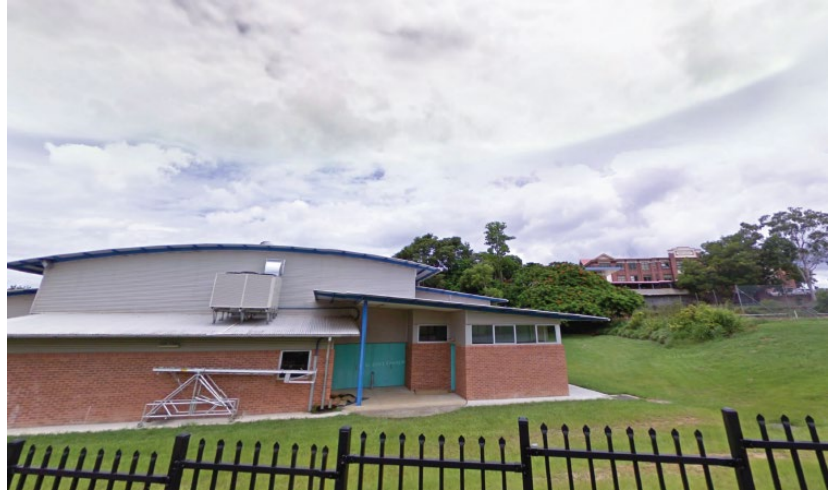
Figure 63 Current View 5 (photo)
