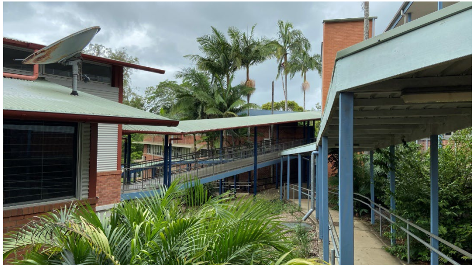
Figure 14 View of typical covered walkway between existing buildings H and S. Source: Architectus
