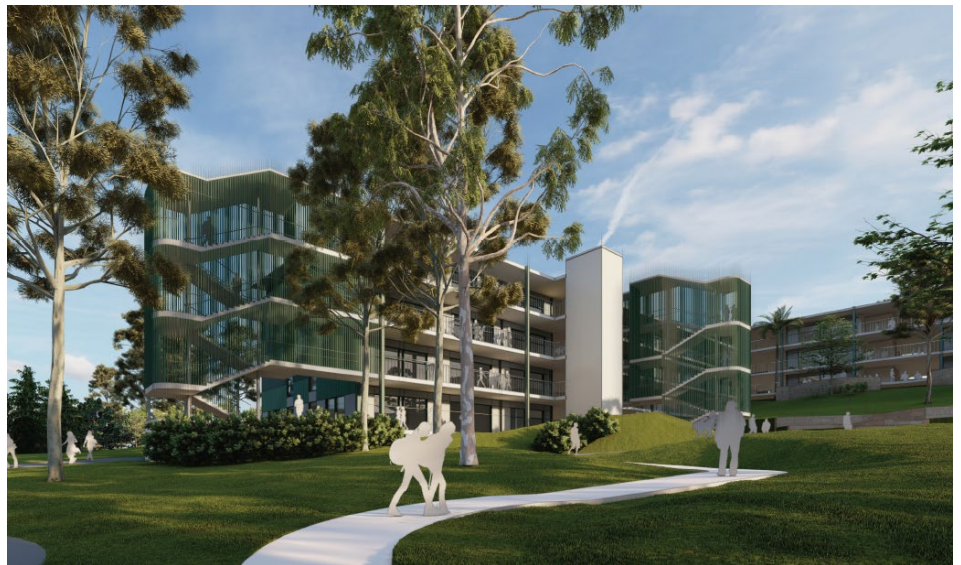
Figure 30 North elevation of Building 4 viewed from the assembly area. Source: Architectus
