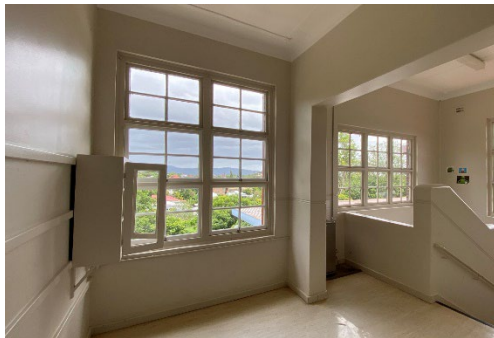
Figure 27 Block A interiors Source: Architectus
