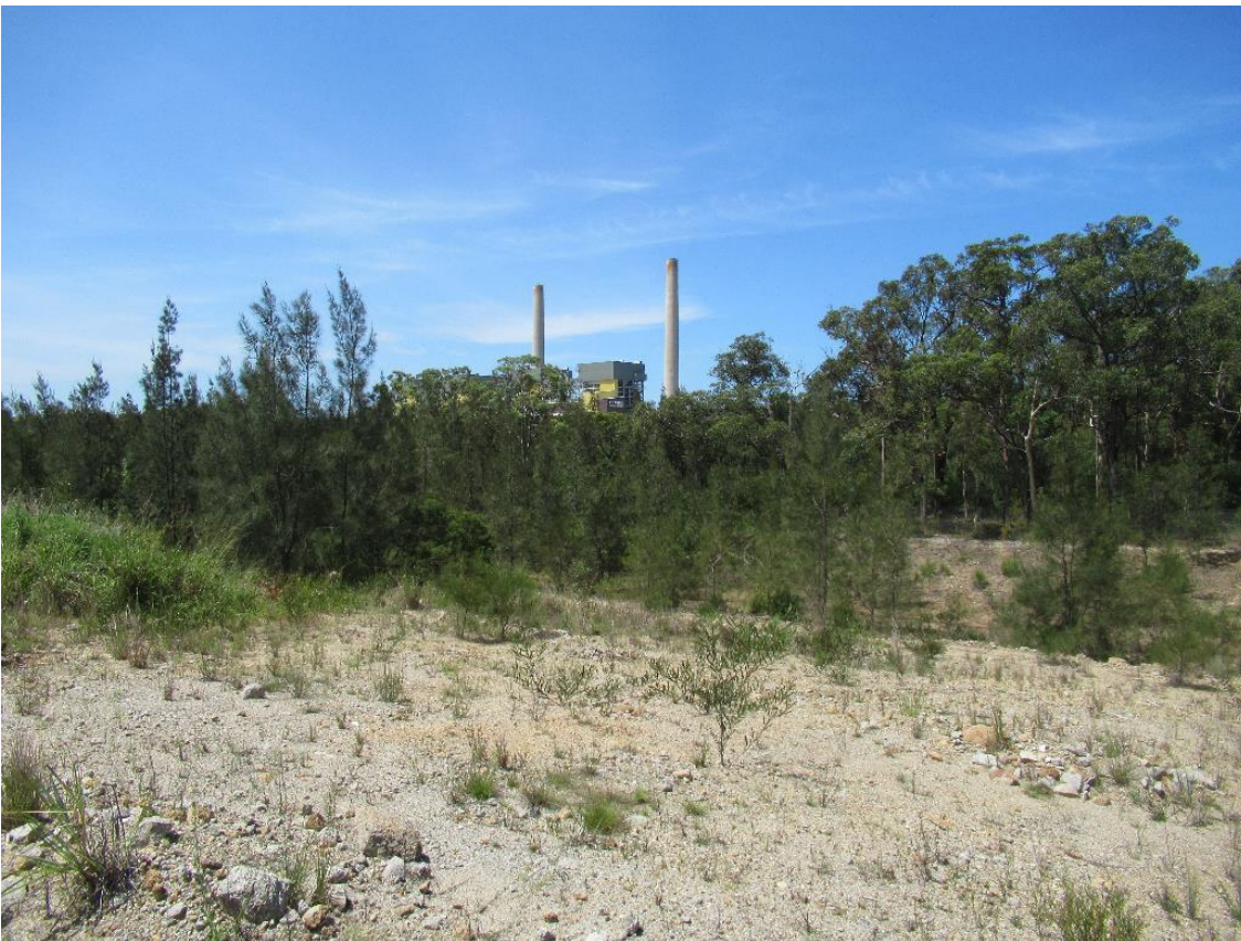
Photo 3-3: BESS compound area from centre looking north to EPS
