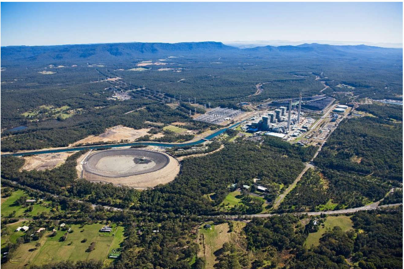
Photo 1-1: Aerial view of Origin landholding from above Lake Eraring (south east)
