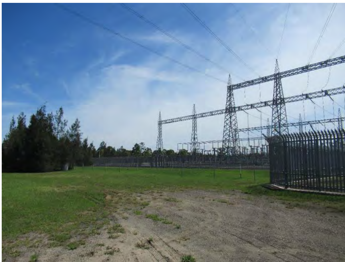
Photo 3-2: View of vacant gantry at TransGrid switchyard
