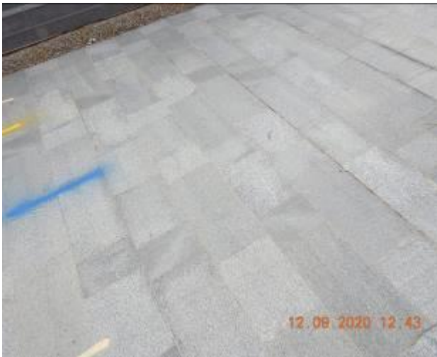
Figure 39 – Hairline cracking and efflorescence through footpath pavement
