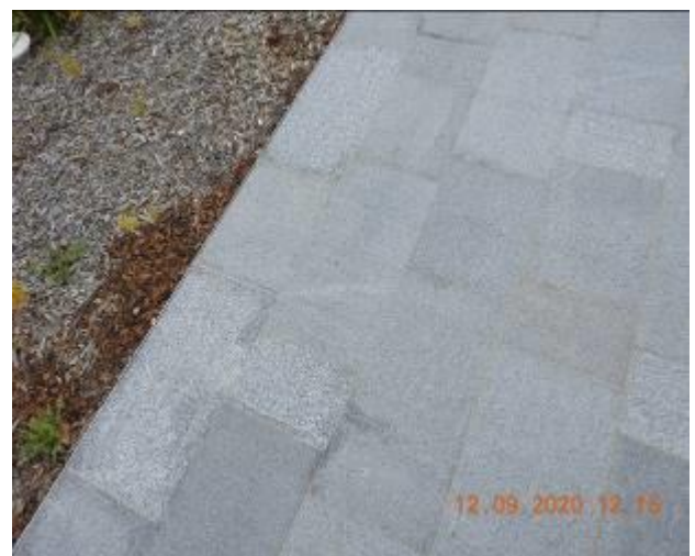
Figure 905 – Efflorescence and crack propagation through footpath pavement
