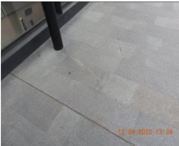
Figure 2076 – Hairline crack propagation through floor tiles
