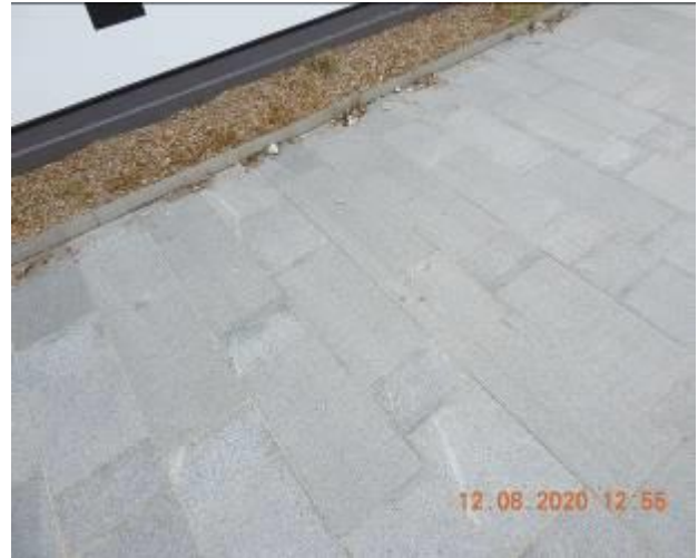
Figure 750 – Efflorescence, hairline crack propagation and loss of material through footpath pavement
