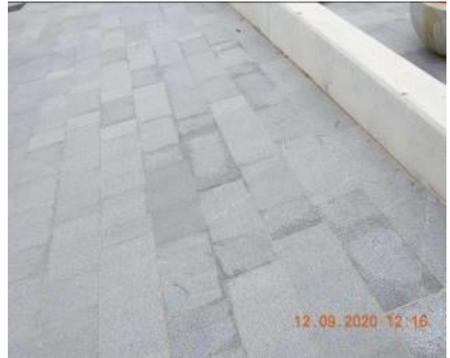
Figure 925 – Hairline crack propagation through footpath pavement
