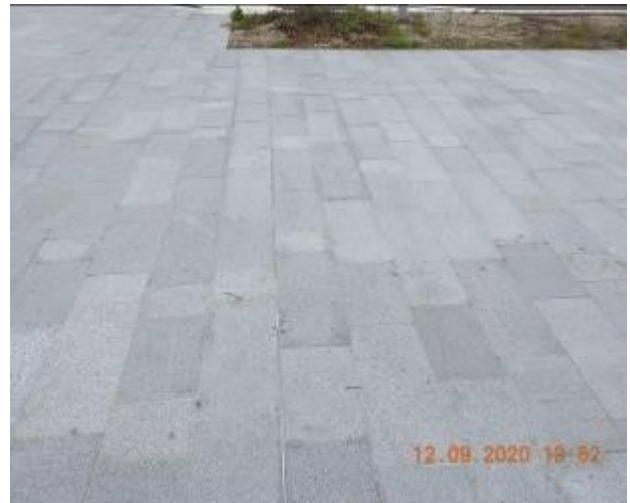
Figure 2459 – Hairline crack propagation through walkway floor
