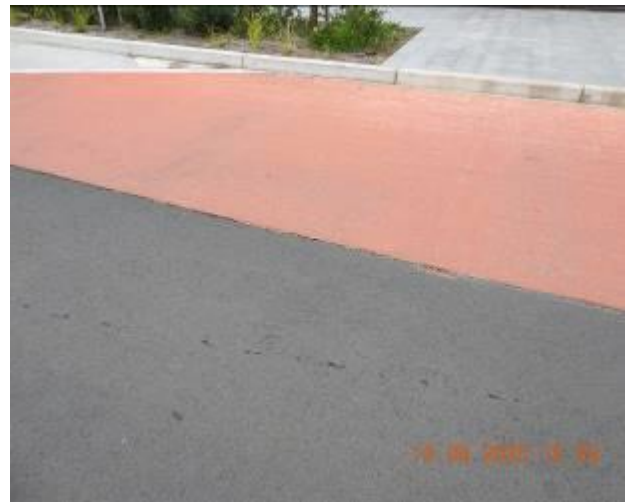
Figure 614 – Crack propagation and loss of material through road surface
