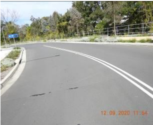
Figure 1445 – Evidence of patchwork through road surface
