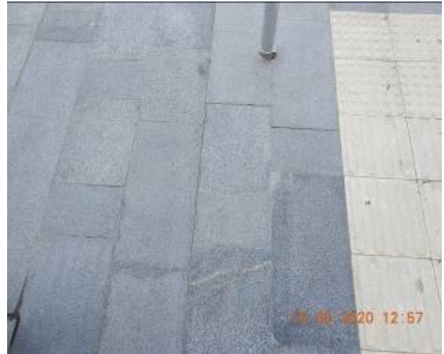
Figure 774 – Hairline crack propagation and loss of material through footpath pavement
