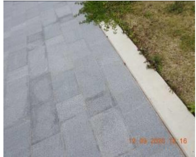
Figure 919 – Crack propagation through footpath pavement
