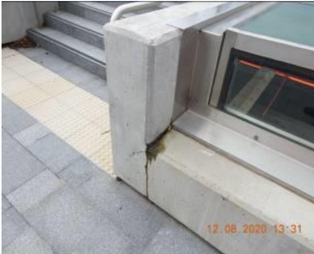
Figure 2008 – Crack propagation through retaining wall
