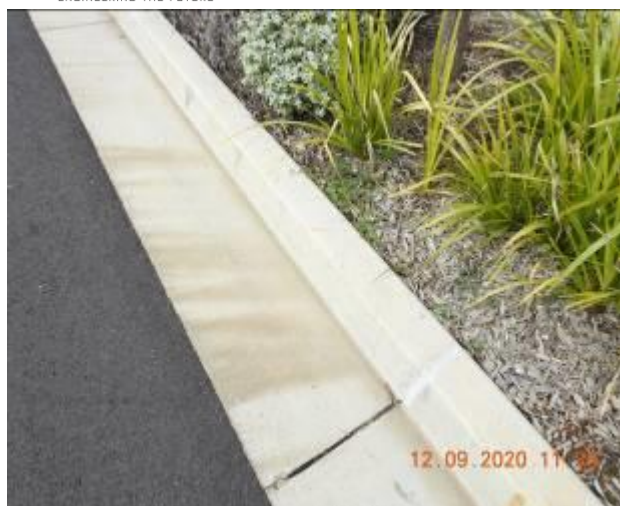
Figure 1263 – Hairline crack propagation through kerb
