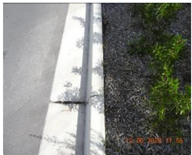
Figure 1786 – Crack propagation and loss of material through kerb and gutter
