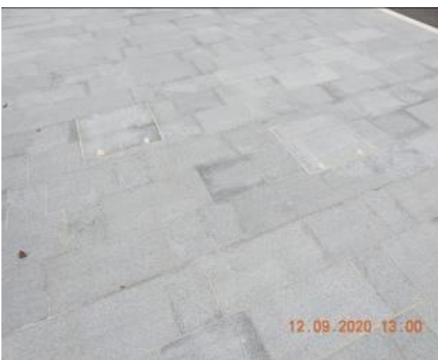
Figure 269 – Hairline cracking and efflorescence through footpath pavement
