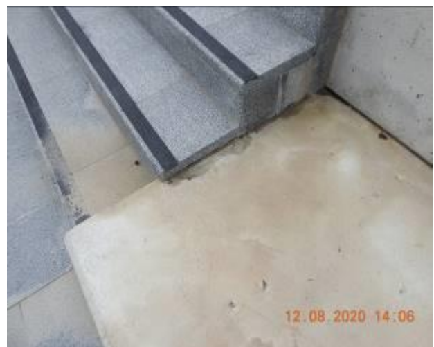
Figure 2218 – Efflorescence through staircase floor
