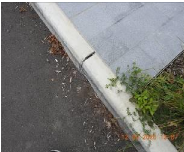
Figure 411 – Crack propagation and loss of material through kerb
