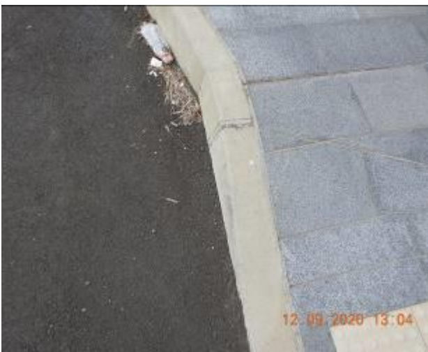
Figure 353 – Crack propagation through kerb
