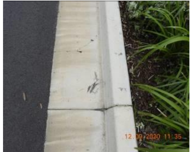
Figure 1204 – Crack propagation and loss of material through kerb and gutter
