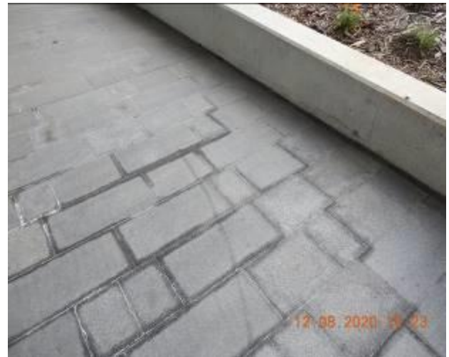
Figure 1957 – Efflorescence, crack propagation and loss of material through floor tiles
