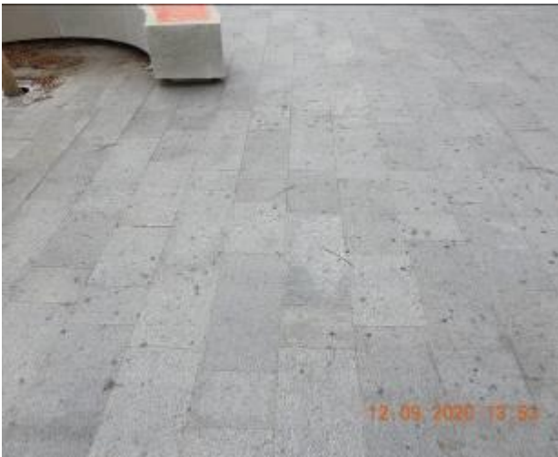
Figure 2482 – Hairline crack propagation through walkway floor
