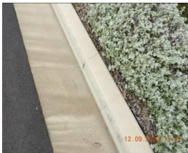
Figure 1249 – Crack propagation and loss of material through kerb and gutter
