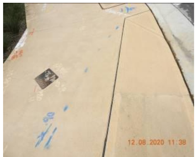
Figure 1648 – Crack propagation through footpath pavement
