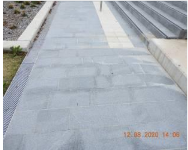
Figure 2220 – Hairline crack propagation through walkway floor
