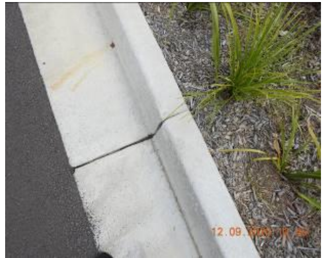
Figure 100 – Crack propagation and loss of material through kerb and gutter
