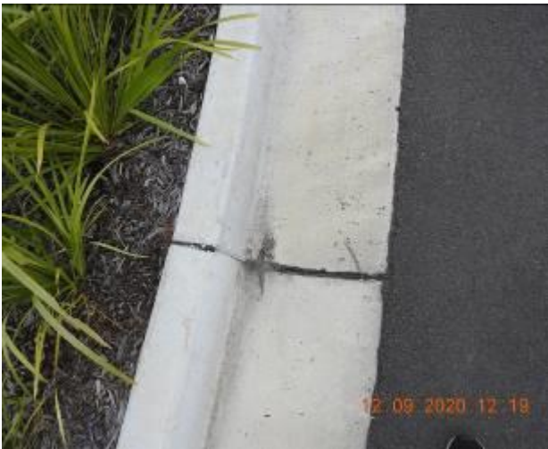
Figure 962 – Crack propagation and loss of material through kerb and gutter
