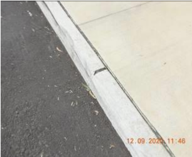
Figure 1359 – Loss of material through kerb
