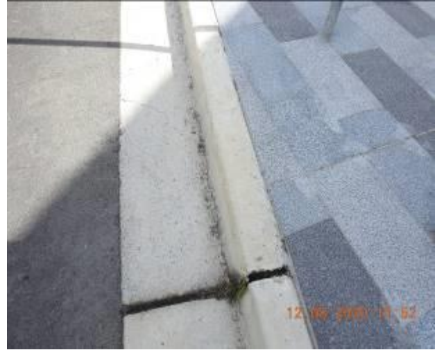
Figure 1746 – Crack propagation and loss of material through kerb and gutter
