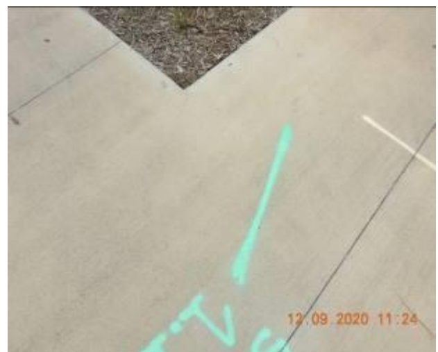
Figure 1082 – Crack propagation through footpath pavement
