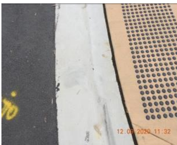
Figure 1165 – Crack propagation through layback and gutter
