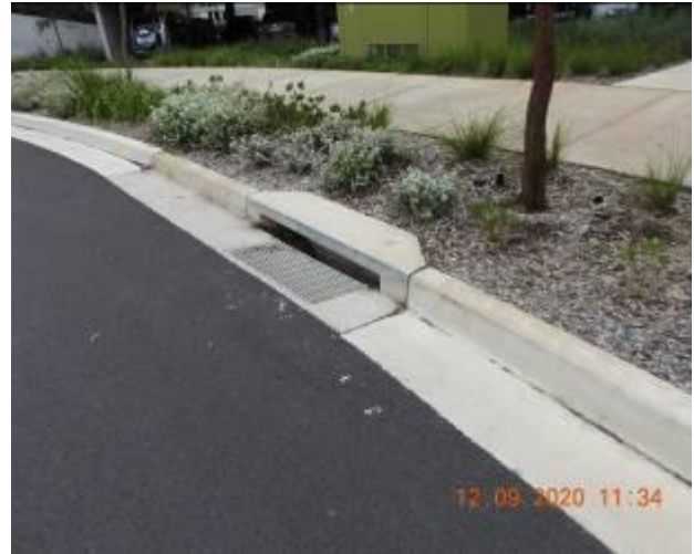
Figure 1186 – General condition of stormwater inlet pit/ Loss of material through kerb
