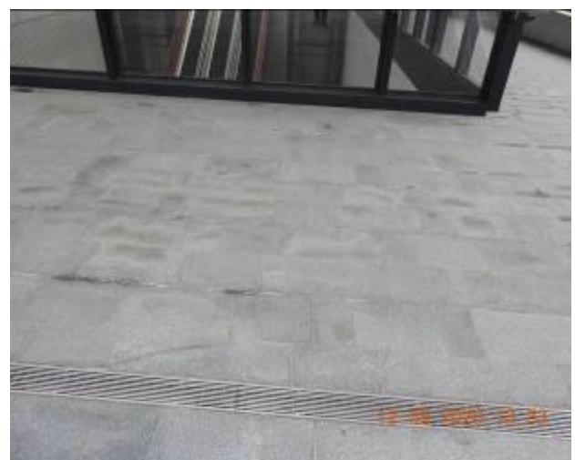
Figure 2031 – Efflorescence and hairline crack propagation through floor tiles
