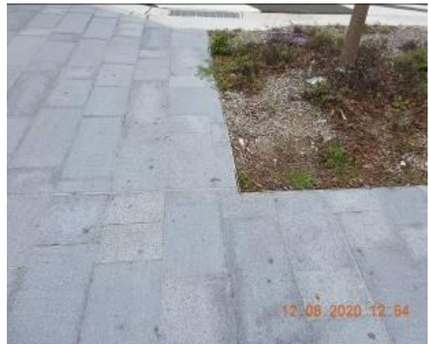
Figure 734 – Crack propagation and loss of material through footpath pavement
