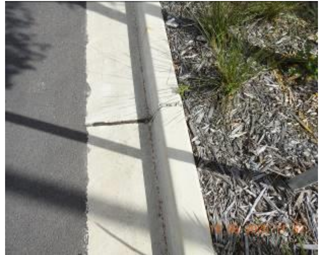
Figure 1730 – Crack propagation and loss of material through kerb and gutter
