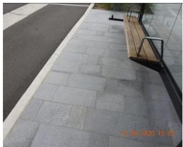
Figure 318 – Hairline cracking and efflorescence through footpath pavement
