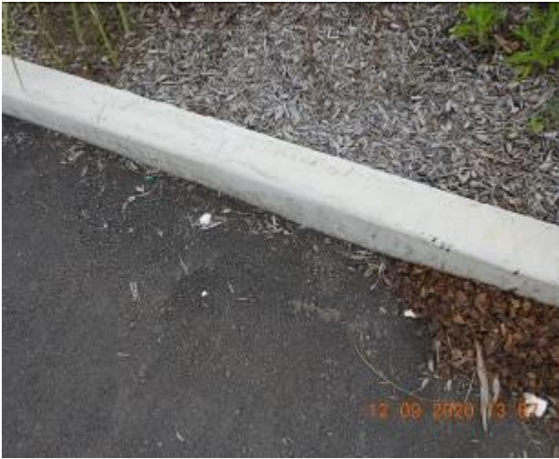
Figure 415 – Crack propagation through kerb
