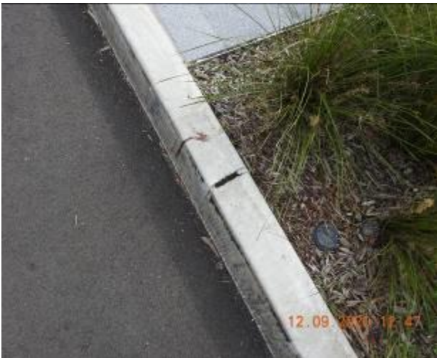
Figure 135 – Crack propagation through kerb
