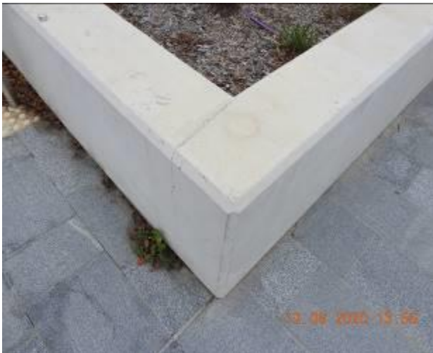
Figure 2143 – Crack propagation through retaining wall
