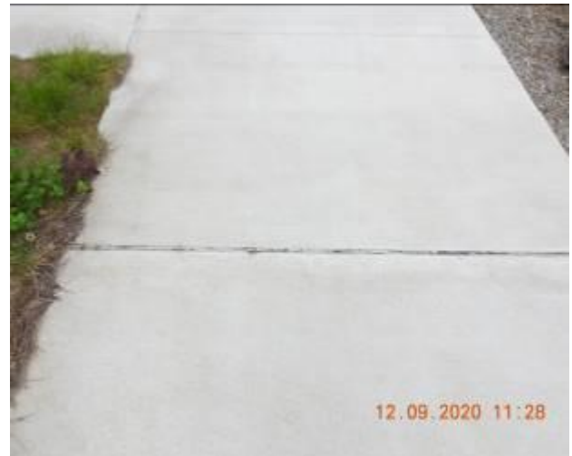
Figure 1128 – Loss of material through footpath pavement
