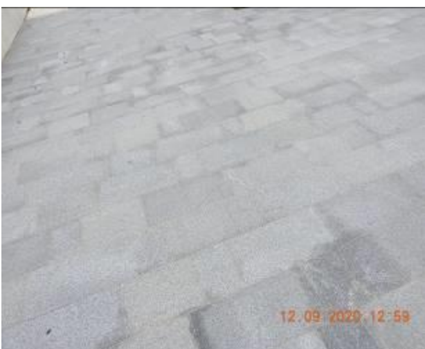
Figure 257 – Hairline cracking and efflorescence through footpath pavement
