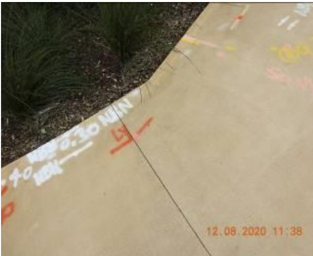
Figure 1651 – Separation through footpath pavement
