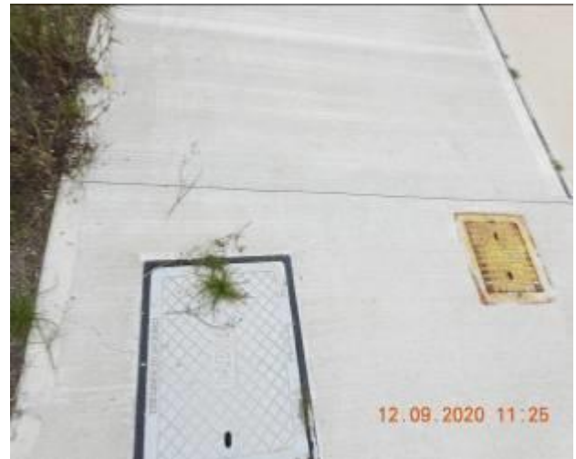
Figure 1098 – Crack propagation through footpath pavement
