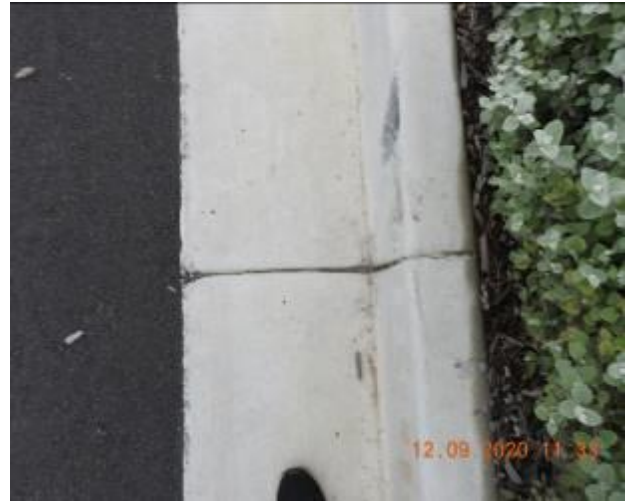
Figure 1180 – Crack propagation and loss of material through kerb and gutter
