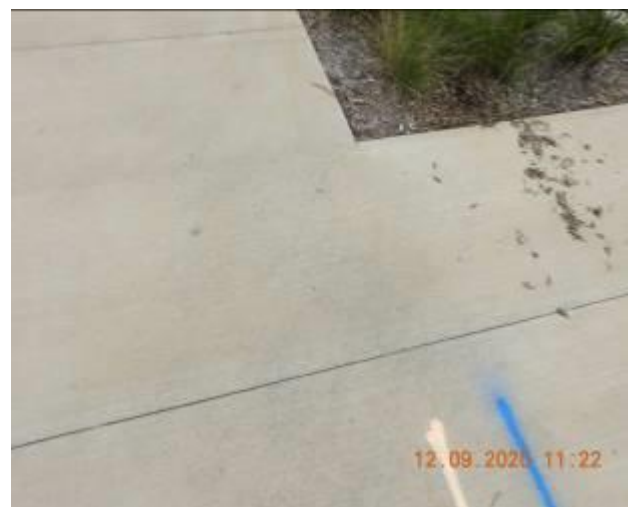
Figure 1064 – Hairline crack propagation through footpath pavement
