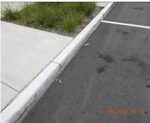
Figure 976 – Loss of material through kerb
