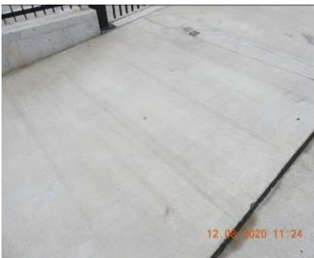
Figure 1539 – Loss of material through driveway pavement
