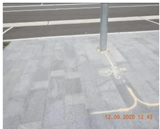
Figure 54 – Hairline cracking and efflorescence through footpath pavement
