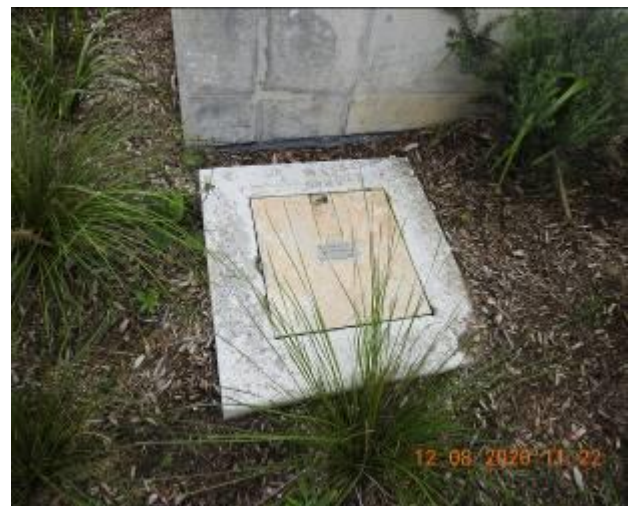
Figure 1526 – Loss of material through service pit pavement
