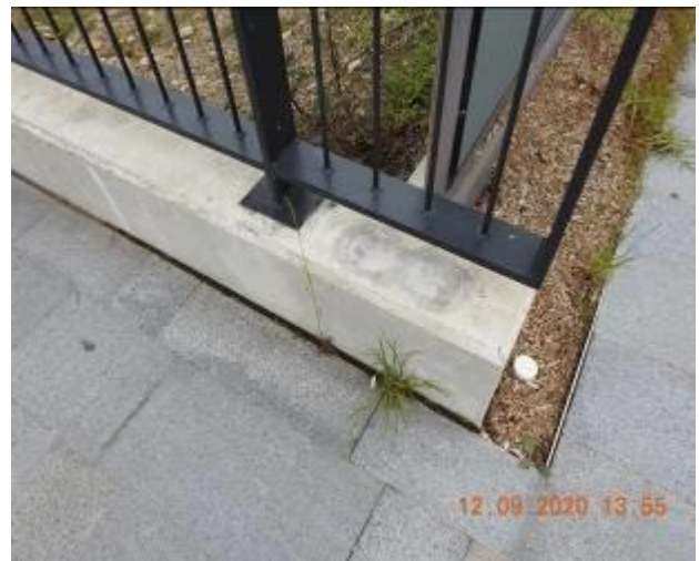
Figure 2513 – Evidence of patchwork through boundary wall
