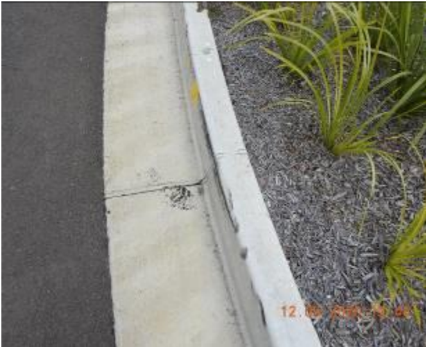
Figure 91 – Crack propagation and loss of material through gutter
