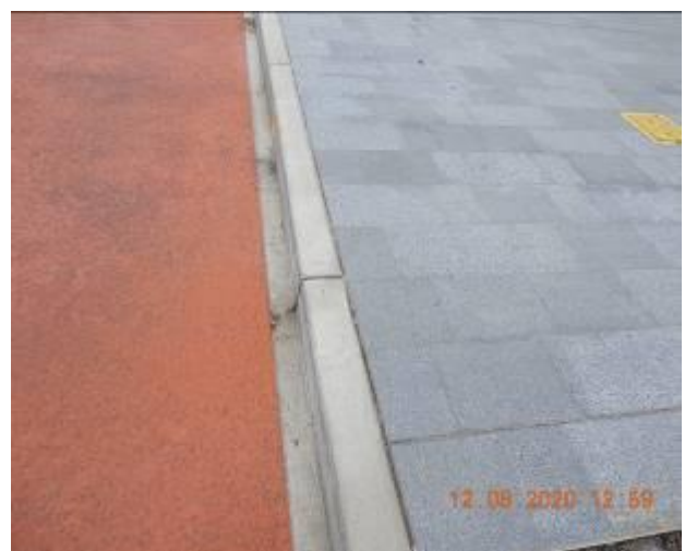
Figure 802 – Hairline crack propagation and evidence of patchwork through kerb
