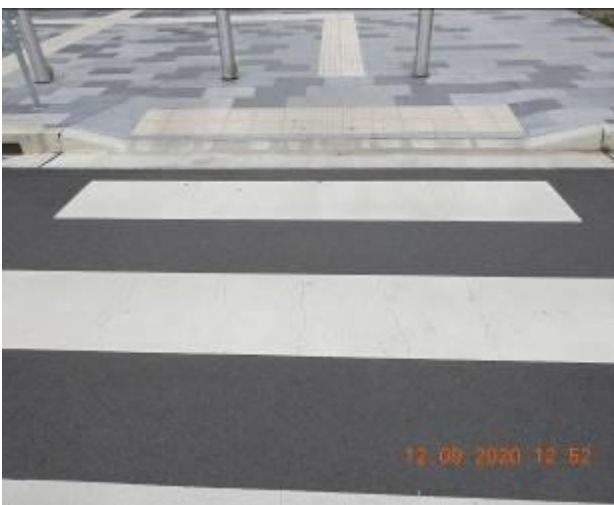
Figure 189 – Crack propagation through road surface
