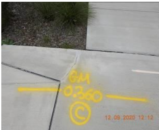
Figure 878 – Crack propagation and loss of material through footpath pavement
