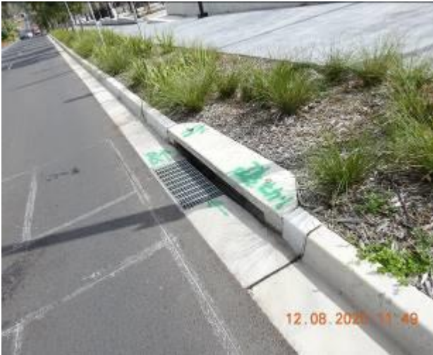
Figure 1697 – General condition of stormwater inlet pit/Loss of material through kerb
