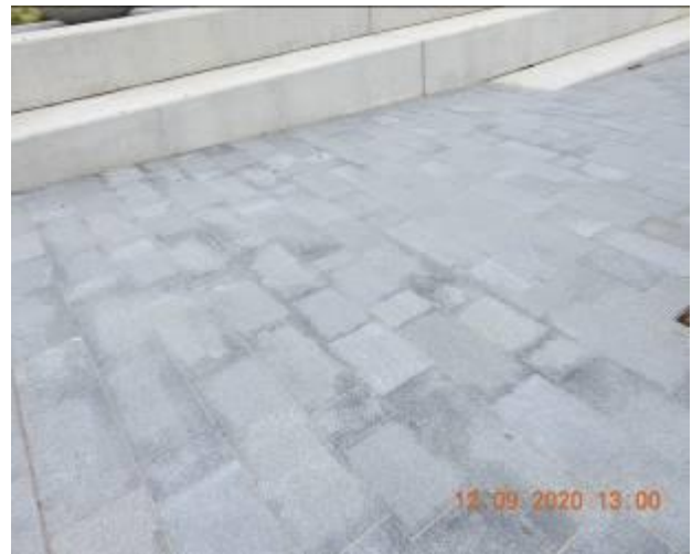
Figure 262 – Hairline cracking and efflorescence through footpath pavement
