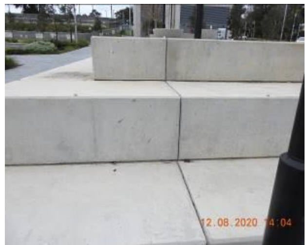
Figure 2206 – Separation through retaining wall
