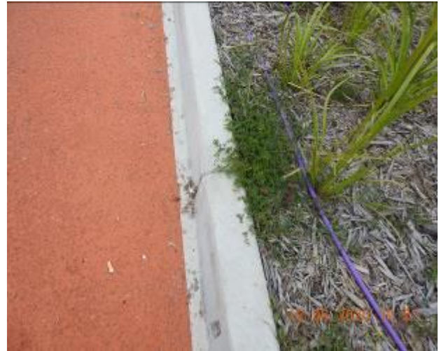
Figure 570 – Crack propagation and loss of material through kerb
