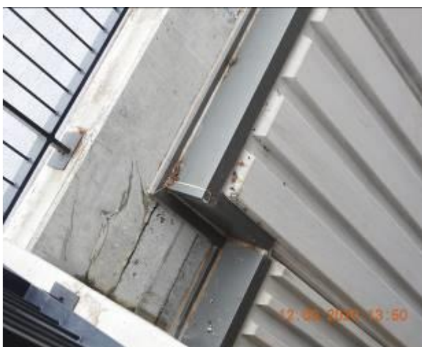
Figure 2436 – Crack propagation and loss of material through external wall
