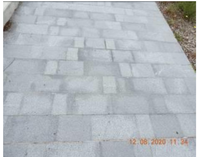
Figure 1622 – Crack propagation and loss of material through footpath pavement
