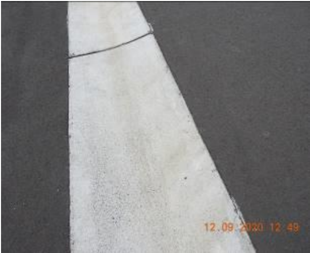
Figure 121 – Crack propagation through gutter
