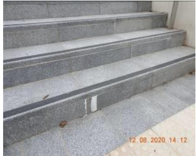
Figure 2292 – Efflorescence, crack propagation and loss of material through staircase floor
