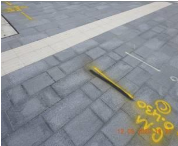
Figure 511 – Loss of material through footpath pavement
