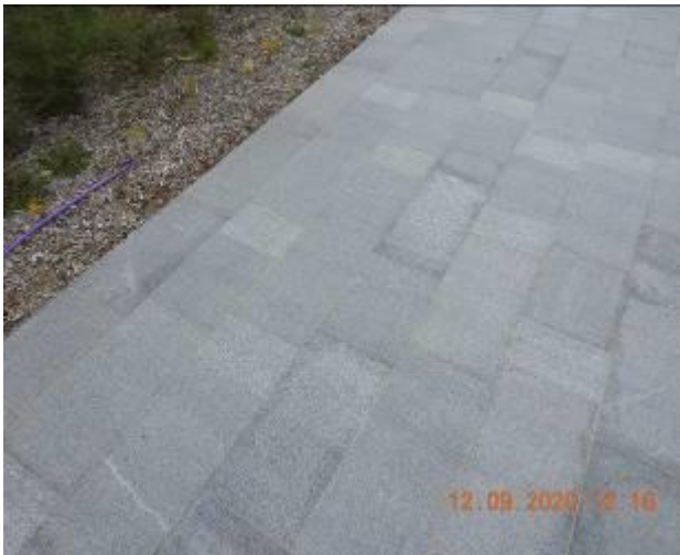
Figure 920 – Hairline crack propagation through footpath pavement
