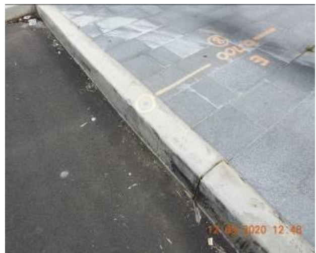
Figure 150 – Crack propagation and loss of material through kerb
