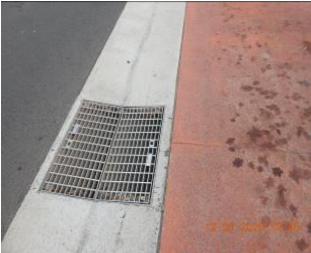
Figure 623 – Evidence of patchwork, crack propagation and loss of material through road surface
