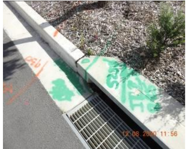
Figure 1794 – Loss of material through kerb
