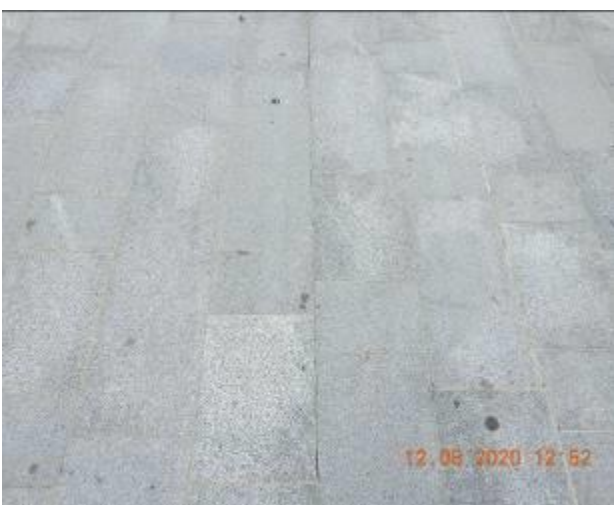
Figure 723 – Efflorescence, hairline crack propagation and loss of material through footpath pavement
