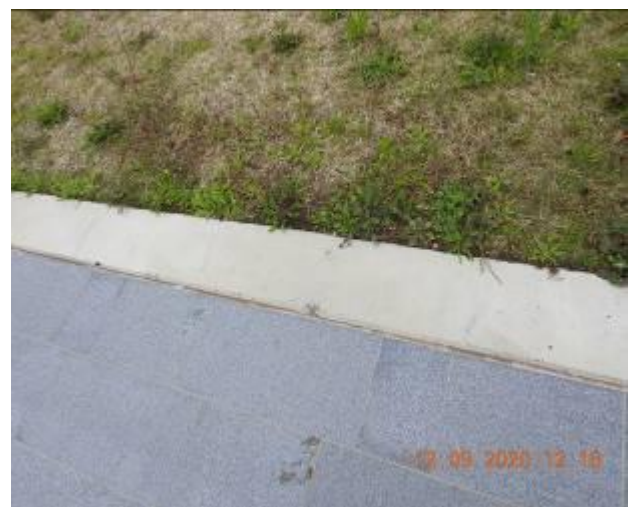
Figure 911 – Crack propagation and loss of material through footpath pavement
