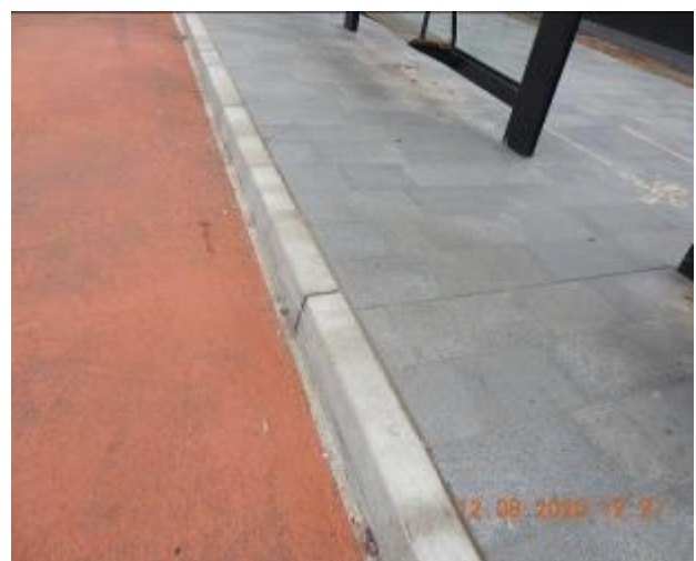
Figure 574 – Evidence of patchwork crack propagation and loss of material through kerb
