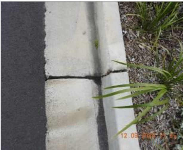
Figure 1211 – Loss of material through kerb
