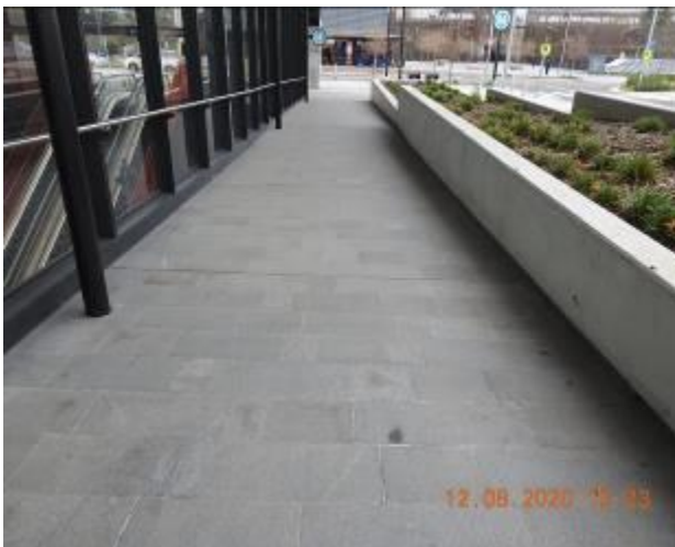
Figure 1958 – Efflorescence through floor tiles
