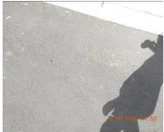
Figure 1410 – Loss of material through road surface
