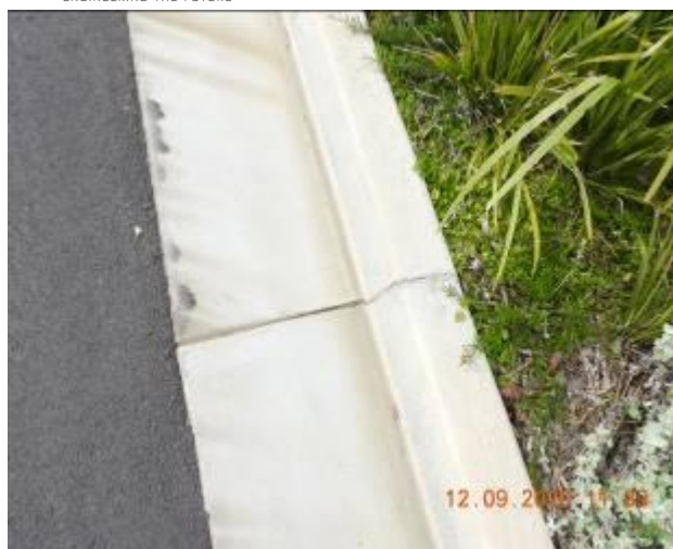
Figure 1281 – Crack propagation and loss of material through kerb and gutter
