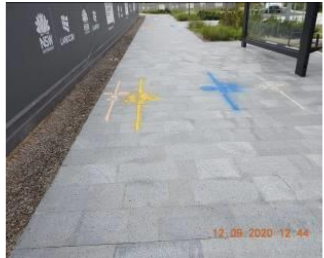
Figure 70 – Hairline cracking and efflorescence through footpath pavement
