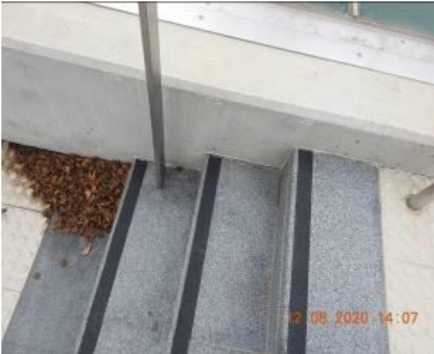
Figure 2231 – Separation through staircase floor
