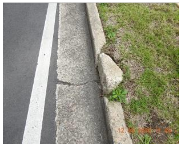
Figure 1672 – Crack propagation and loss of material through kerb and gutter
