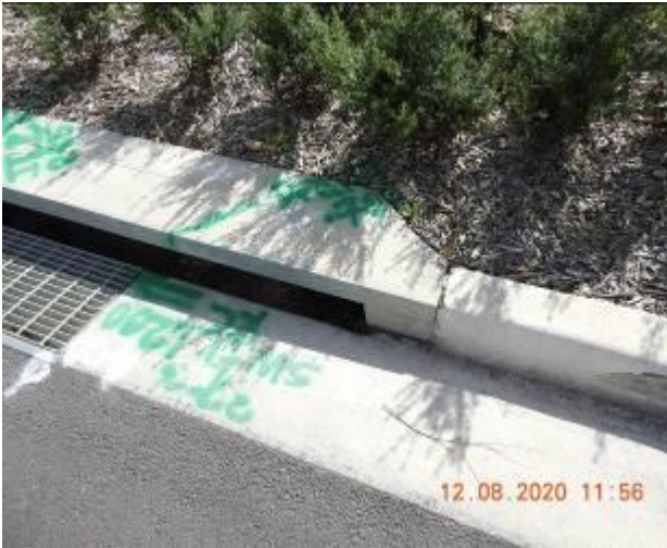
Figure 1793 – Loss of material through kerb
