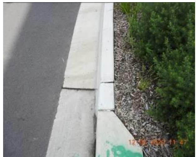
Figure 1684 – Loss of material through kerb and gutter
