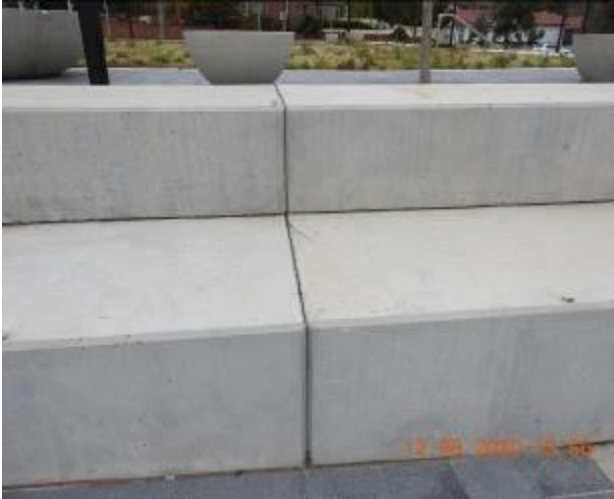
Figure 2135 – Separation through retaining wall
