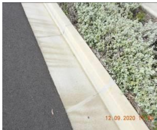
Figure 1268 – Crack propagation and loss of material through kerb and gutter
