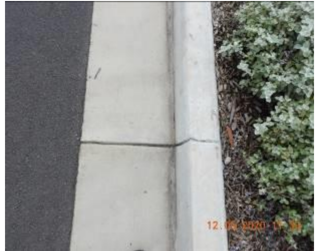
Figure 1222 – Crack propagation and loss of material through kerb and gutter
