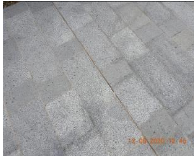
Figure 76 – Hairline cracking and efflorescence through footpath pavement
