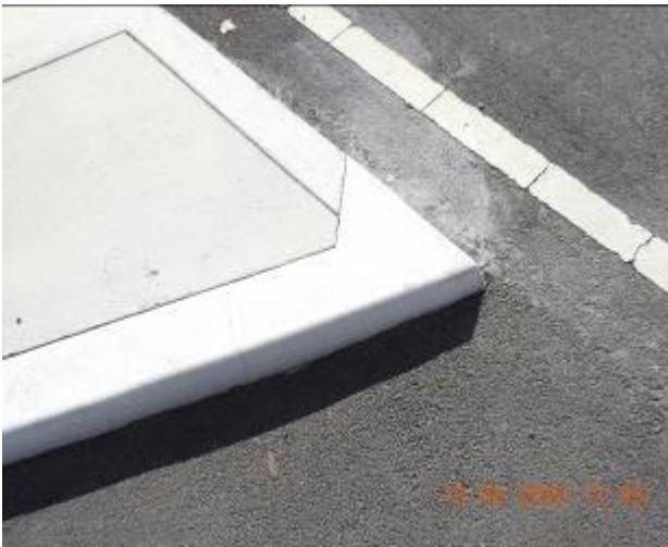
Figure 1807 – Crack propagation through traffic island pavement
