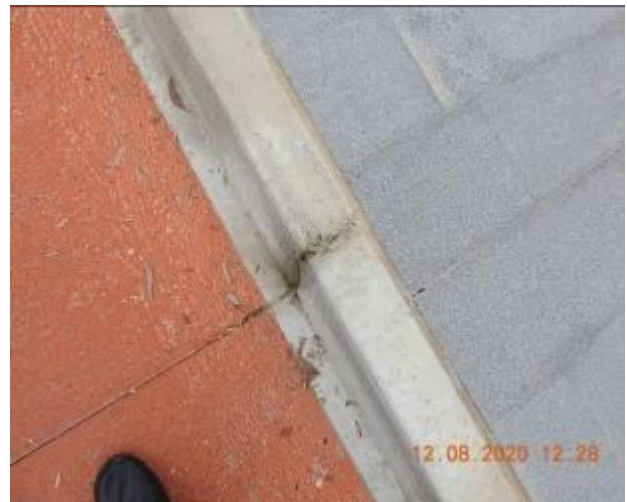
Figure 584 – Crack propagation and loss of material through kerb
