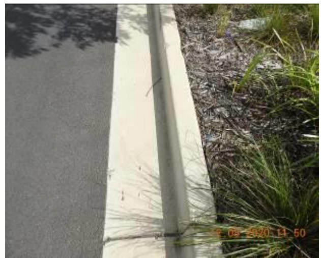
Figure 1708 – Loss of material through kerb and gutter
