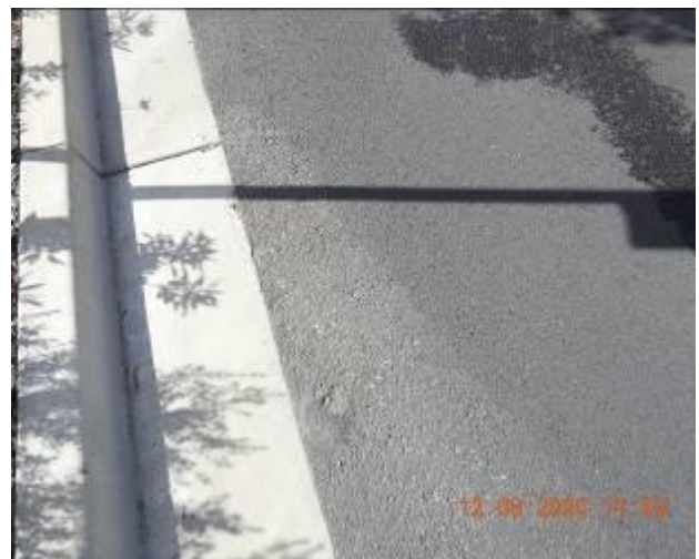
Figure 1816 – Evidence of patchwork through road surface
