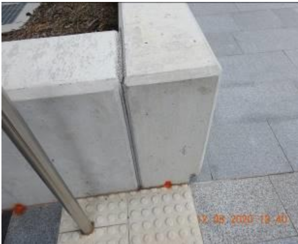
Figure 2088 – Crack propagation through retaining wall
