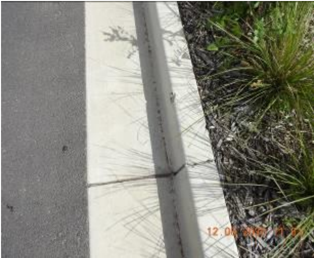
Figure 1729 – Crack propagation and loss of material through kerb and gutter
