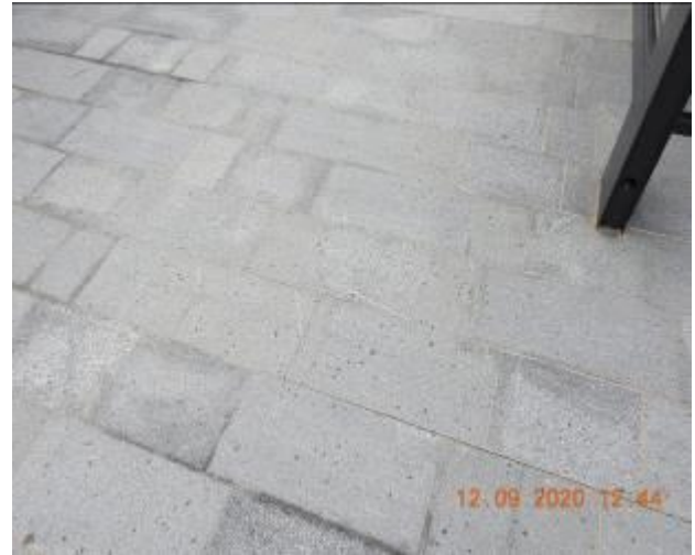
Figure 68 – Hairline cracking and efflorescence through footpath pavement
