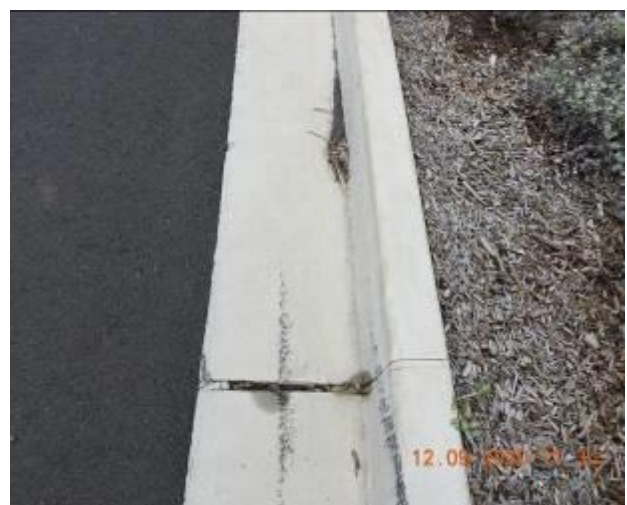
Figure 1184 – Crack propagation and loss of material through kerb and gutter
