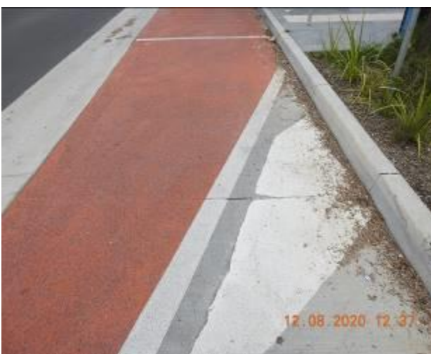
Figure 609 – Paint flaking and loss of material through road surface
