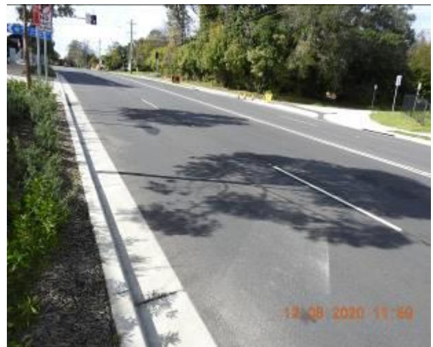
Figure 1814 – Loss of material through road surface
