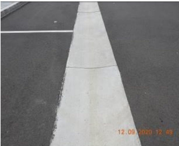
Figure 165 – Crack propagation and loss of material through gutter
