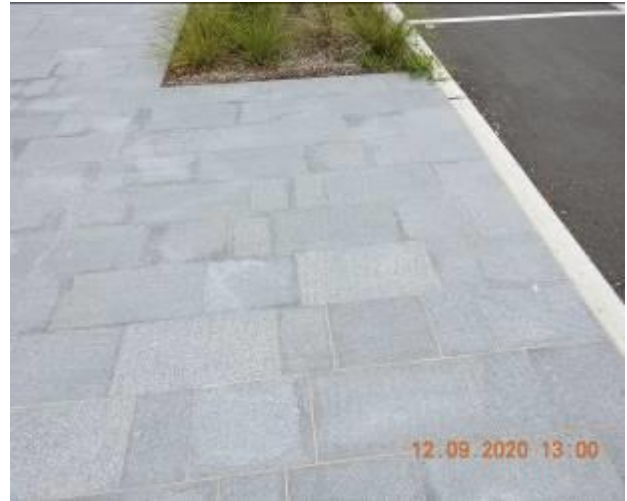
Figure 272 – Hairline cracking and efflorescence through footpath pavement
