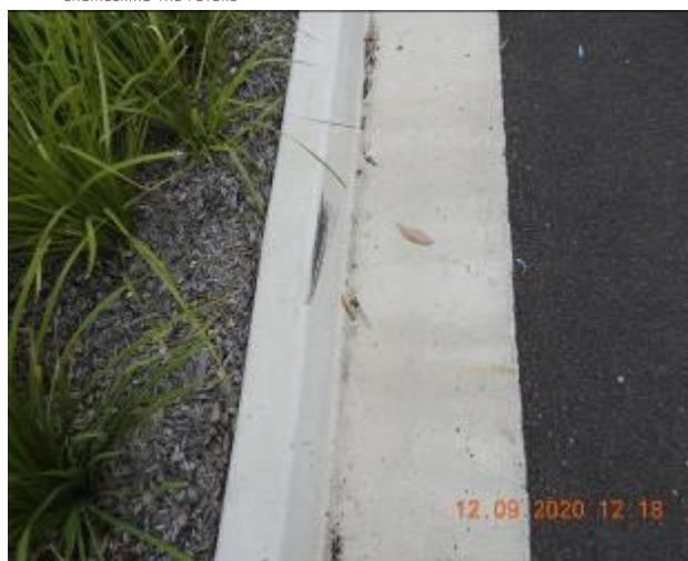
Figure 942 – Hairline crack propagation through kerb
