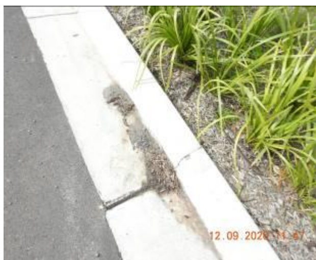
Figure 1375 – Crack propagation and loss of material through kerb and gutter
