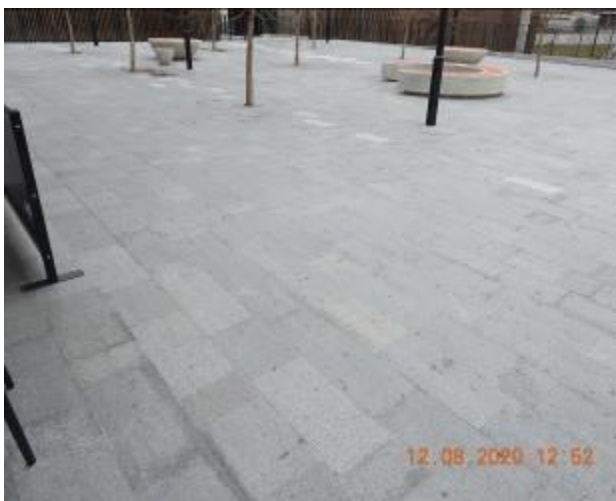
Figure 717 – Efflorescence, hairline crack propagation and loss of material through footpath pavement
