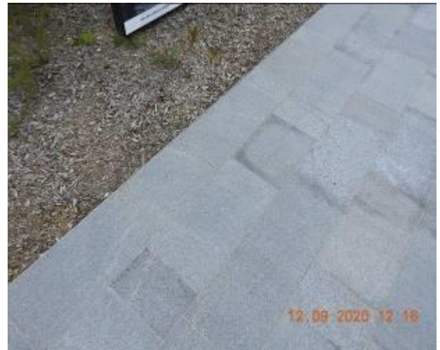
Figure 915 – Hairline crack propagation through footpath pavement
