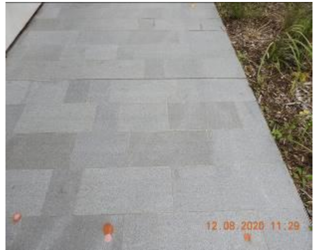
Figure 1586 – Efflorescence and hairline crack propagation through footpath pavement
