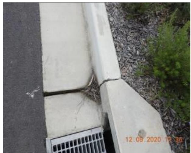
Figure 1220 – Loss of material through kerb
