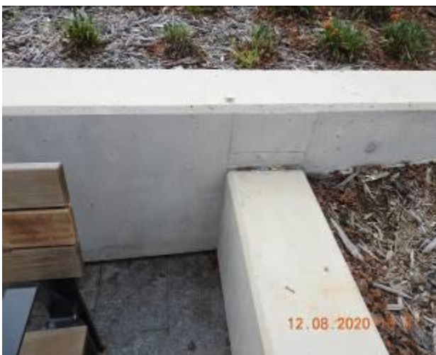
Figure 2012 – Crack propagation and loss of material through retaining wall
