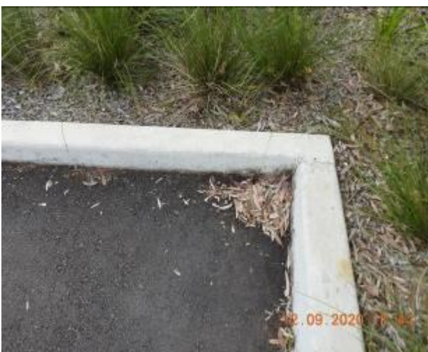
Figure 1345 – Crack propagation and loss of material through kerb
