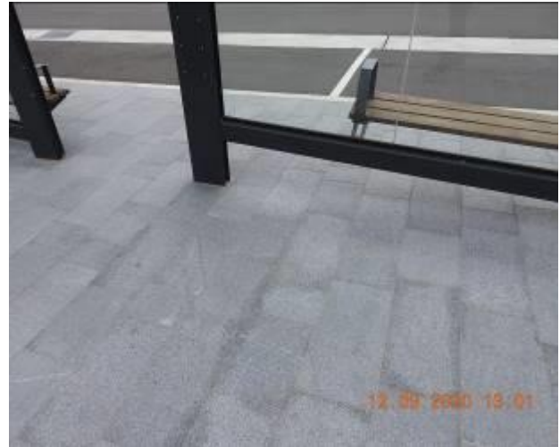
Figure 296 – Hairline cracking and efflorescence through footpath pavement
