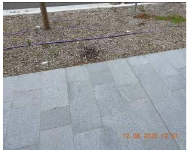
Figure 712 – Efflorescence, crack propagation and loss of material through footpath pavement
