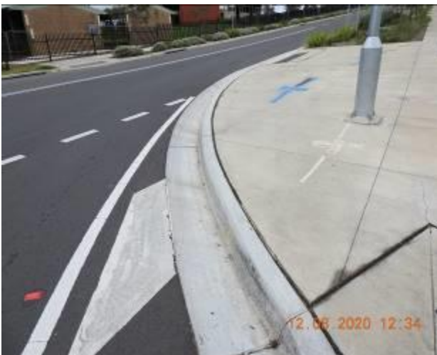
Figure 597 – Crack propagation and loss of material through kerb and gutter
