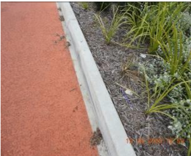
Figure 811 – Hairline crack propagation and evidence of patchwork through kerb
