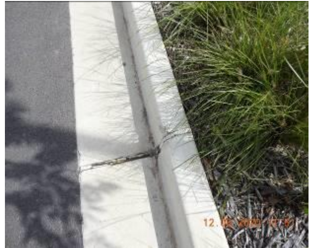
Figure 1722 – Crack propagation and loss of material through kerb and gutter
