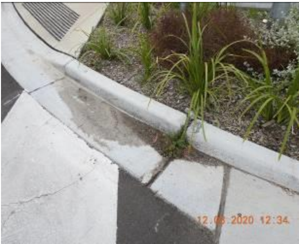
Figure 595 – Crack propagation and loss of material through kerb and gutter
