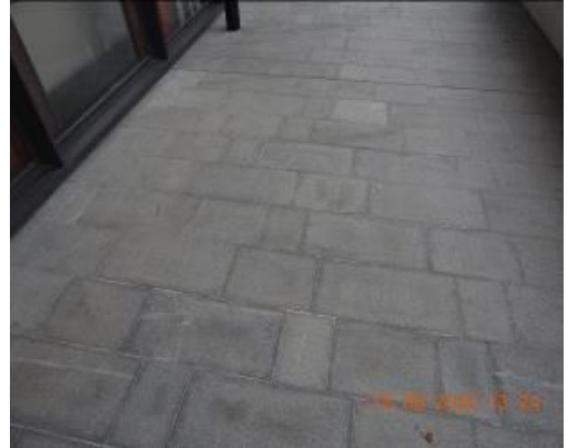
Figure 1967 – Efflorescence and hairline crack propagation through floor tiles
