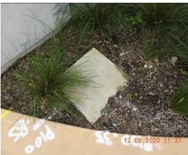
Figure 1647 – Crack propagation and loss of material through service pit pavement
