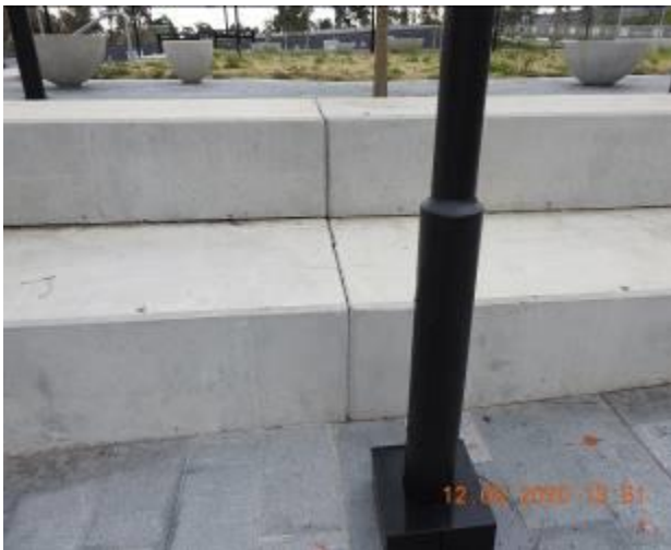
Figure 2113 – Separation through retaining wall
