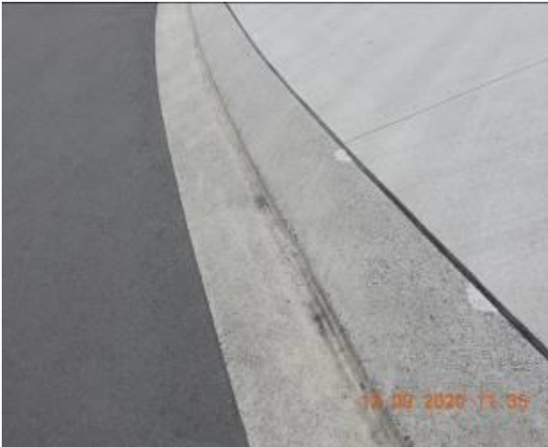
Figure 1215 – Evidence of patchwork through layback
