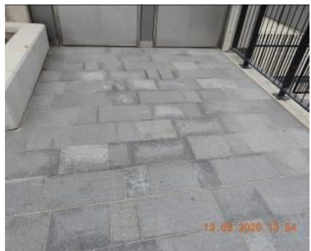
Figure 2503 – Hairline crack propagation through walkway floor
