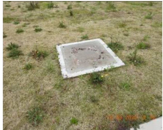
Figure 921 – Crack propagation and loss of material through service pit pavement
