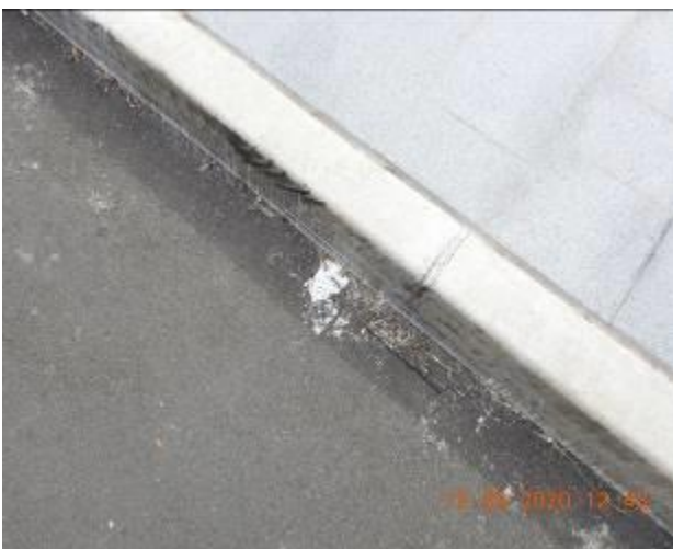
Figure 143 – Crack propagation through kerb
