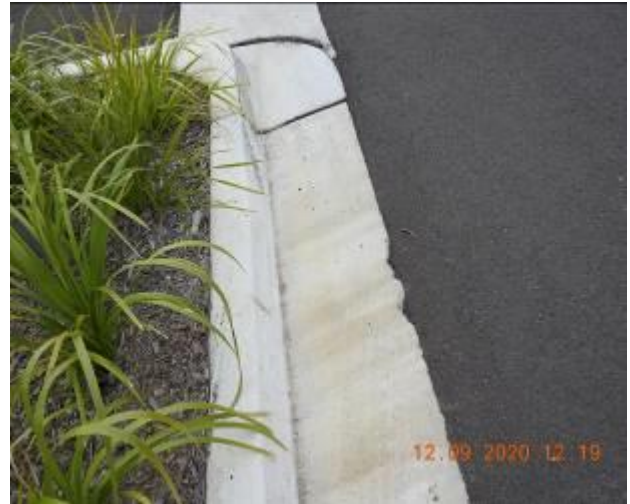
Figure 973 – Loss of material through gutter
