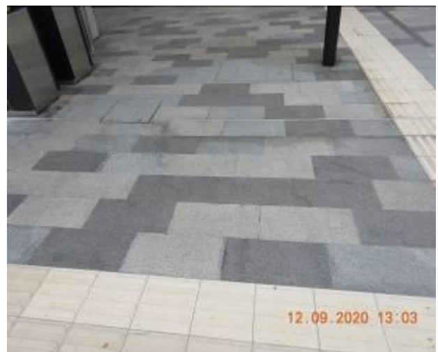
Figure 336 – Hairline cracking and efflorescence through footpath pavement
