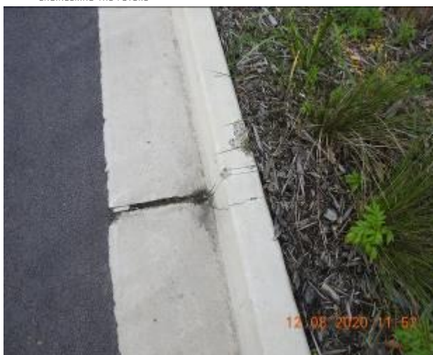
Figure 1733 – Crack propagation and loss of material through kerb and gutter
