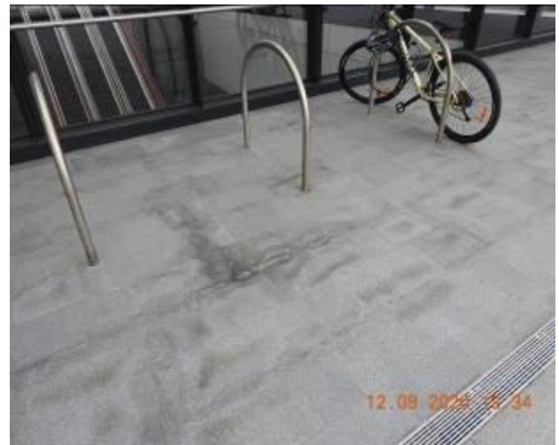
Figure 2041 – Efflorescence, crack propagation and loss of material through floor tiles
