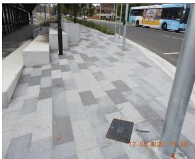
Figure 1575 – Loss of material through footpath pavement
