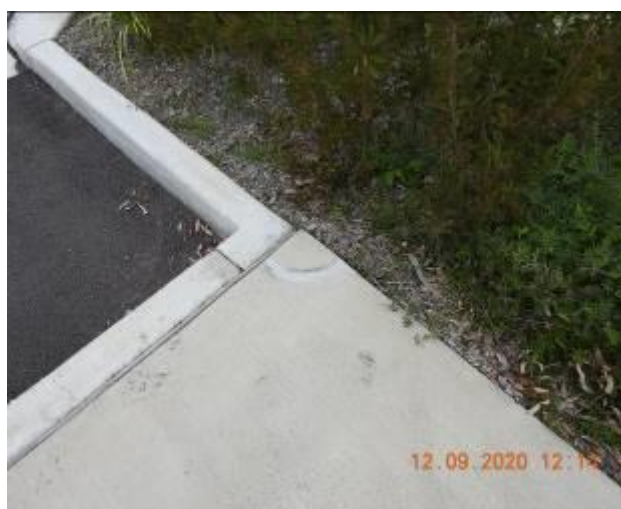
Figure 892 – Hairline Crack propagation and evidence of patchwork through footpath pavement
