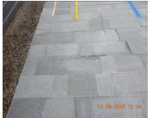
Figure 58 – Hairline cracking and efflorescence through footpath pavement
