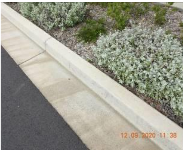
Figure 1253 – Hairline crack propagation through kerb
