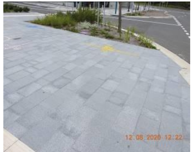
Figure 506 – Loss of material through footpath pavement
