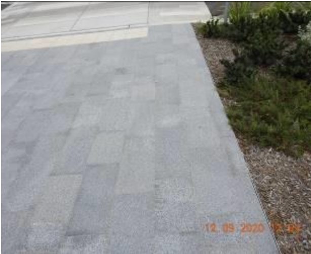
Figure 259 – Hairline cracking and efflorescence through footpath pavement
