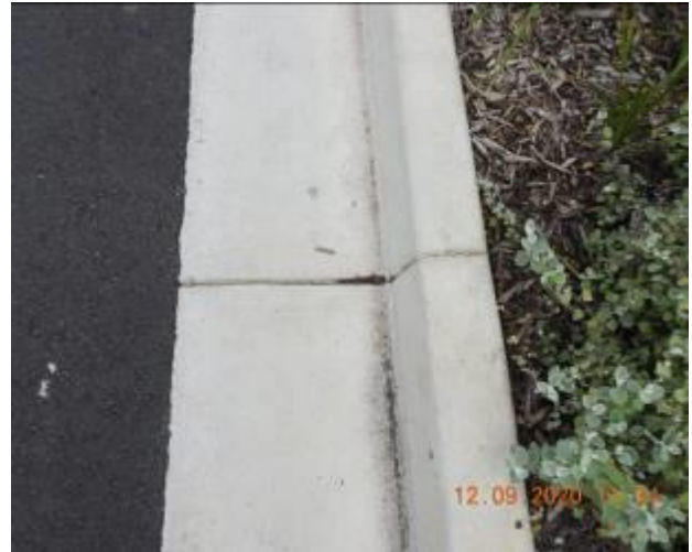
Figure 1192 – Crack propagation and loss of material through kerb and gutter
