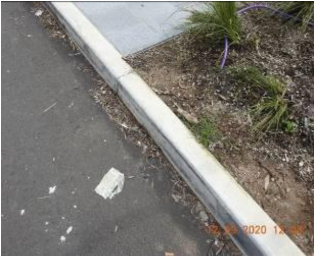
Figure 145 – Crack propagation through kerb
