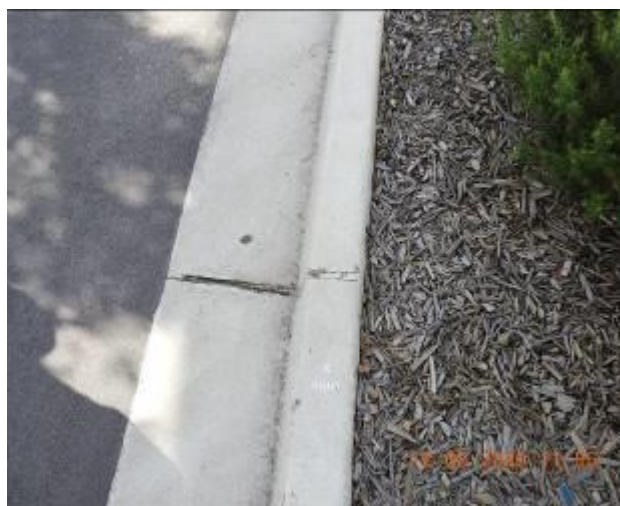
Figure 1789 – Crack propagation and loss of material through kerb and gutter
