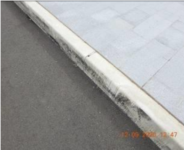
Figure 109 – Loss of material through kerb
