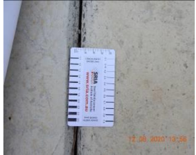
Figure 2136 – Separation through retaining wall Approx. 4mm in width
