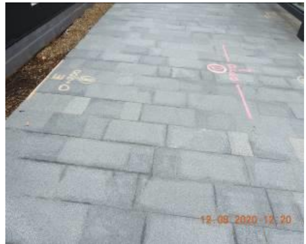
Figure 488 – Hairline crack propagation through footpath pavement
