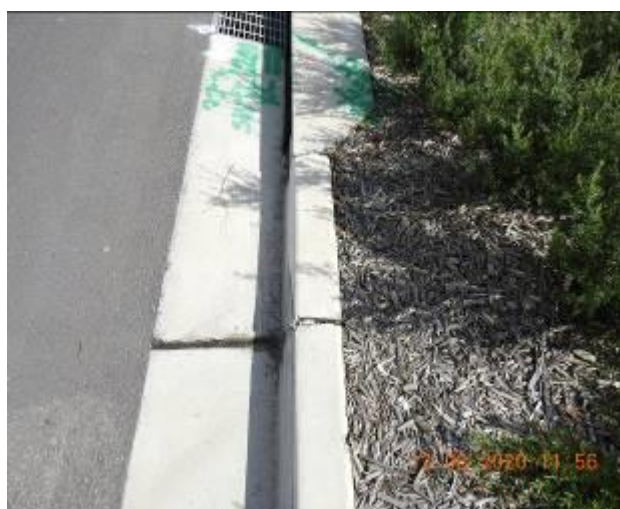
Figure 1791 – Loss of material through kerb and gutter
