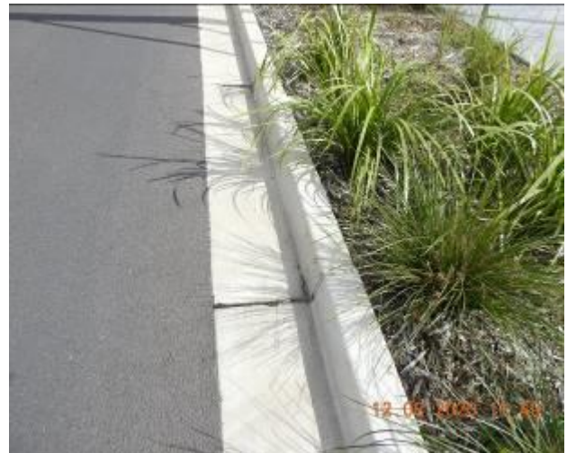
Figure 1700 – Loss of material through kerb and gutter
