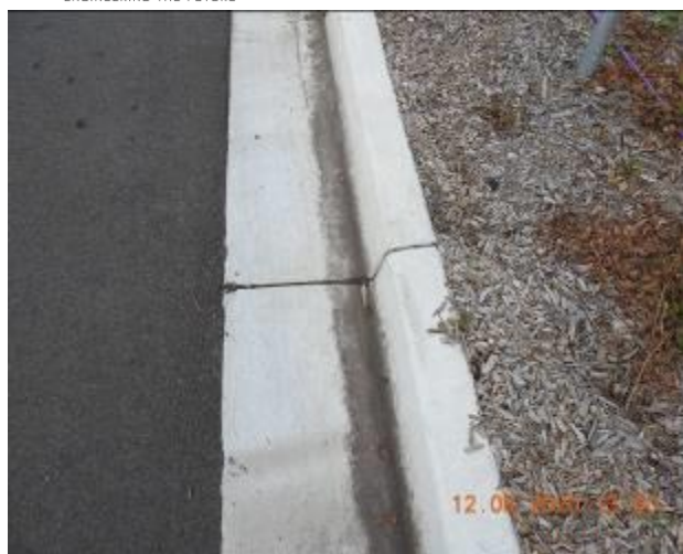
Figure 839 – Crack propagation and loss of material through kerb and gutter
