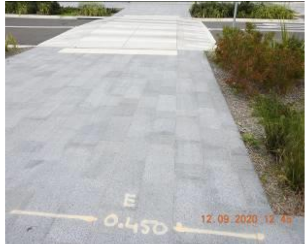
Figure 80 – Hairline cracking and efflorescence through footpath pavement
