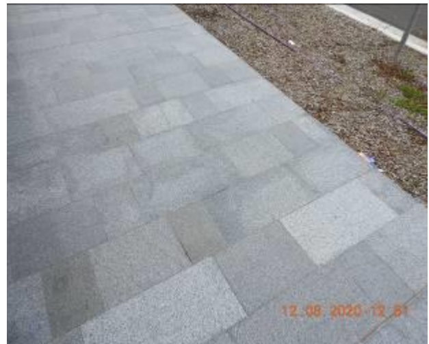
Figure 710 – Loss of material through footpath pavement
