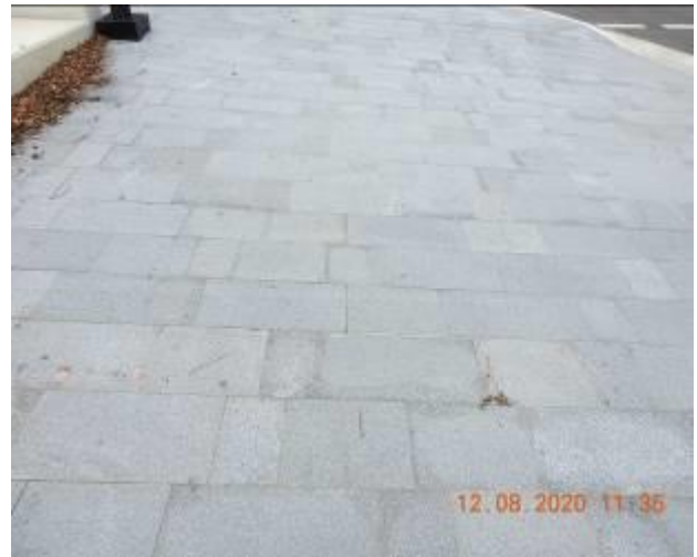
Figure 1628 – Crack propagation and loss of material through footpath pavement
