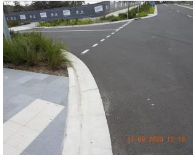
Figure 955 – General condition of layback and gutter
