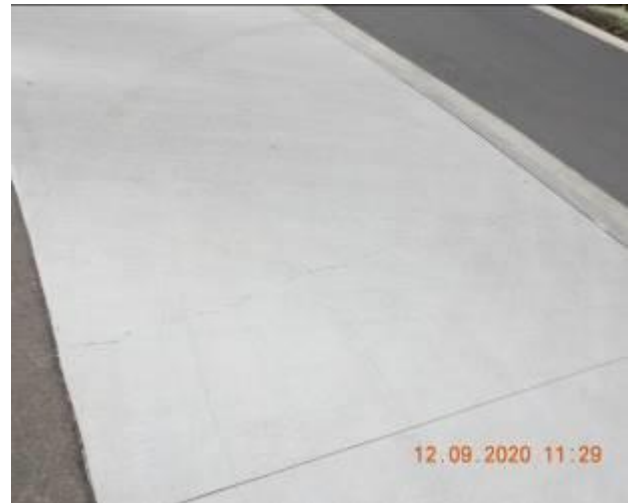
Figure 1134 – Crack propagation and loss of material through driveway pavement
