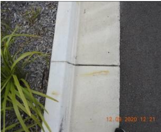
Figure 998 – Crack propagation and loss of material through kerb and gutter
