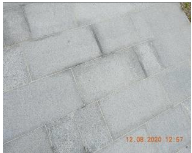
Figure 778 – Loss of material through footpath pavement
