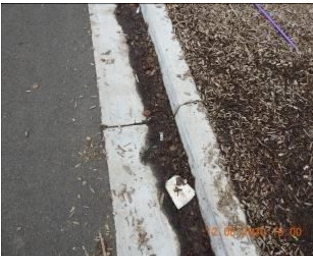
Figure 831 – Crack propagation and loss of material through kerb and gutter
