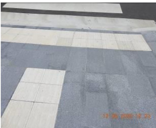
Figure 513 – Crack propagation and loss of material through footpath pavement
