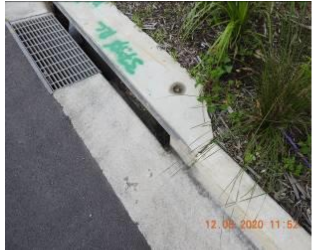
Figure 1740 – Loss of material through kerb
