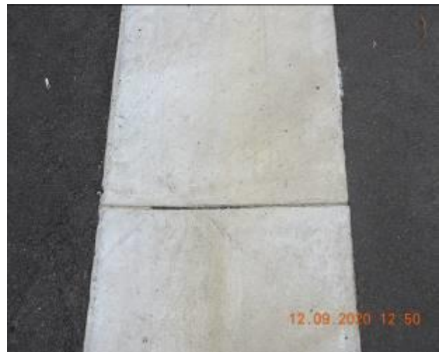
Figure 126 – Crack propagation and loss of material through gutter
