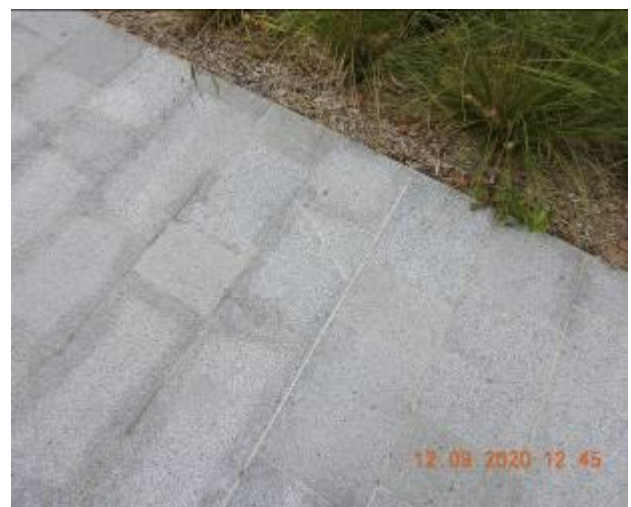
Figure 84 – Hairline cracking and efflorescence through footpath pavement
