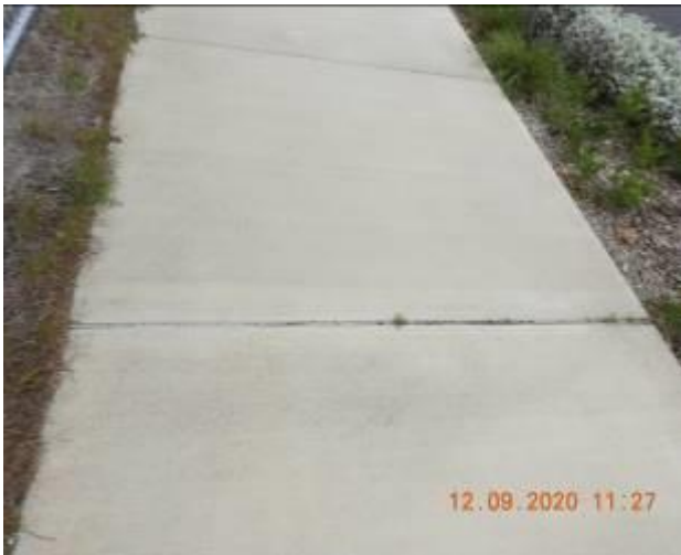
Figure 1115 – Loss of material through footpath pavement
