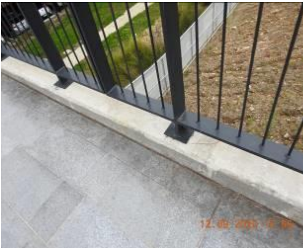
Figure 2518 – Loss of material through boundary wall
