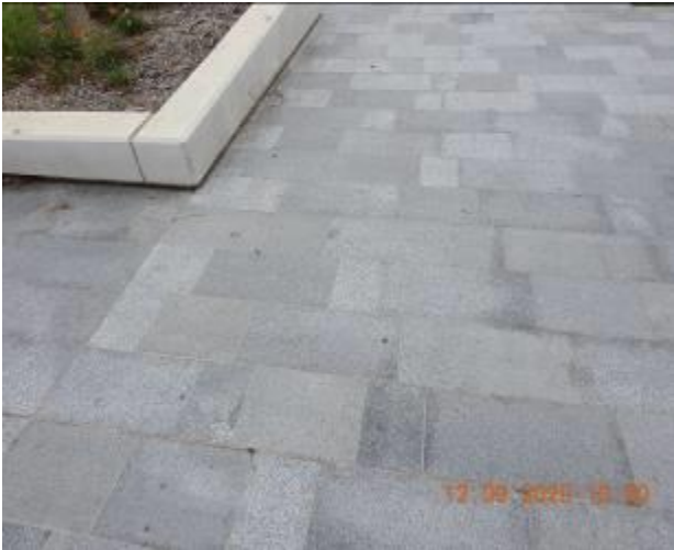
Figure 283 – Hairline cracking and efflorescence through footpath pavement
