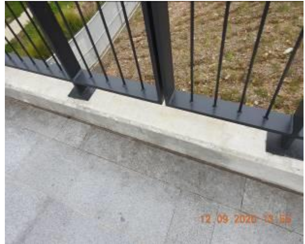
Figure 2517 – Crack propagation through boundary wall
