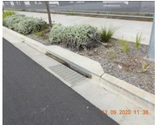
Figure 1258 – General condition of stormwater inlet pit/Loss of material through curb
