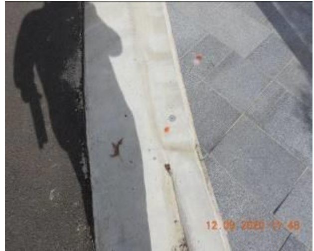
Figure 1692 – Crack propagation through layback and gutter
