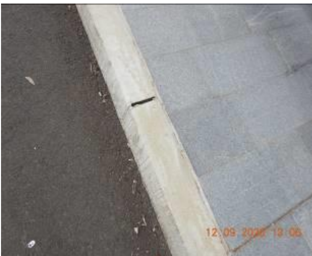
Figure 389 – Crack propagation and loss of material through kerb
