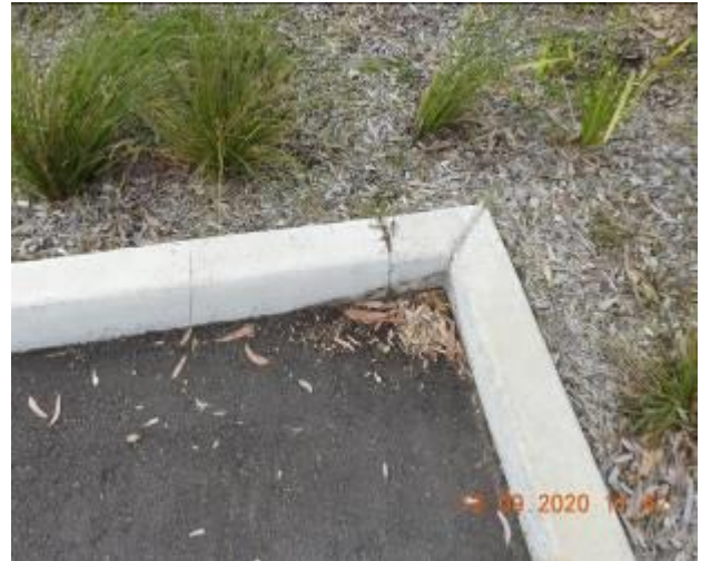
Figure 1324 – Crack propagation and loss of material through kerb
