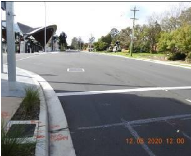
Figure 1825 – Loss of material and evidence of patchwork through road surface
