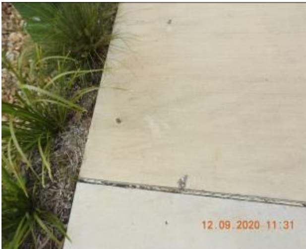
Figure 1157 – Loss of material through footpath pavement
