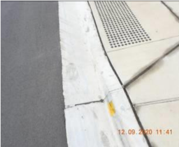
Figure 1305 – Crack propagation and loss of material through kerb and gutter
