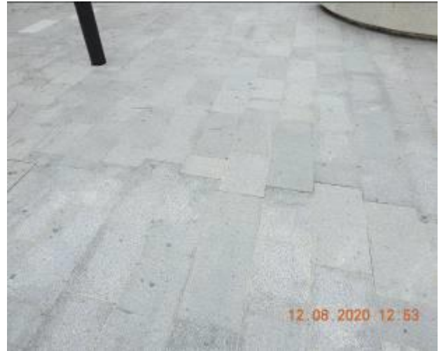
Figure 726 – Efflorescence, hairline crack propagation and loss of material through footpath pavement
