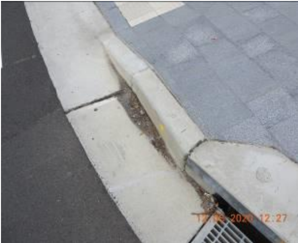
Figure 563 – Evidence of patchwork, crack propagation and loss of material through kerb and gutter
