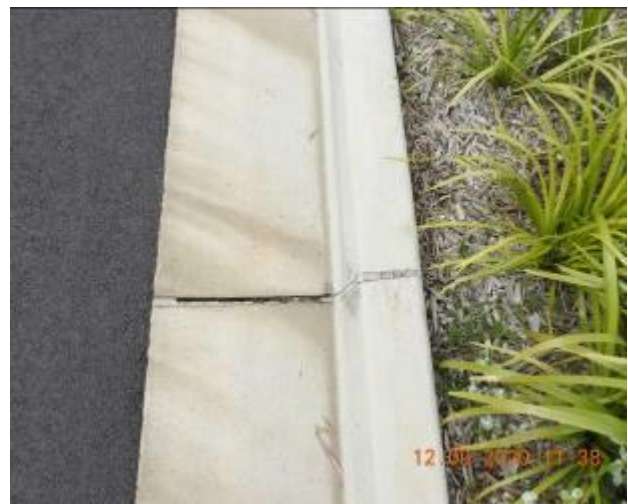
Figure 1256 – Loss of material through kerb and gutter
