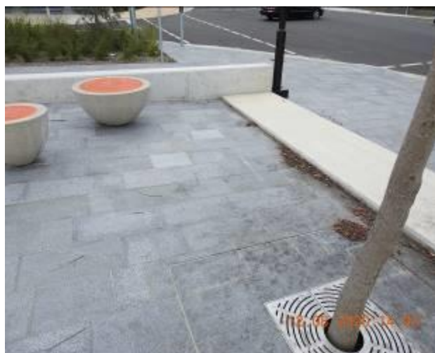
Figure 2185 – Loss of material through walkway floor
