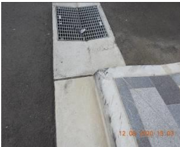
Figure 347 – Crack propagation through kerb
