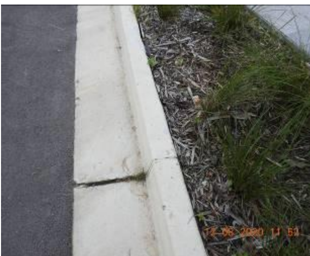
Figure 1743 – Crack propagation and loss of material through kerb and gutter
