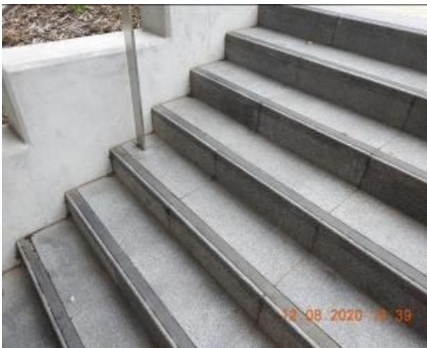
Figure 2084 – Separation through staircase pavement
