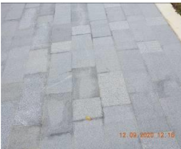
Figure 916 – Crack propagation and loss of material through footpath pavement
