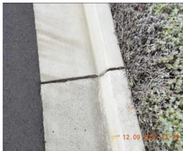
Figure 1274 – Loss of material through kerb and gutter
