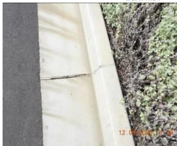
Figure 1282 – Crack propagation and loss of material through kerb and gutter
