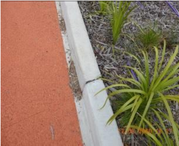
Figure 569 – Loss of material through kerb
