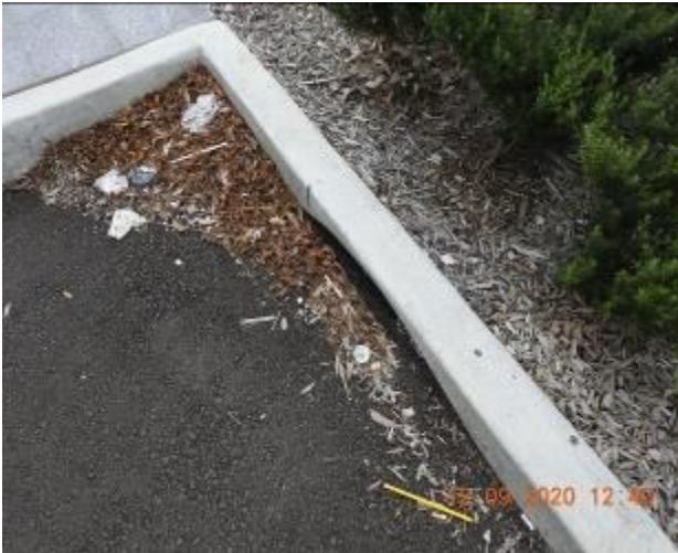
Figure 103 – Crack propagation through kerb
