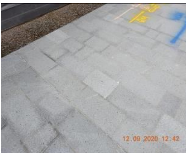
Figure 29 – Hairline cracking and efflorescence through footpath pavement
