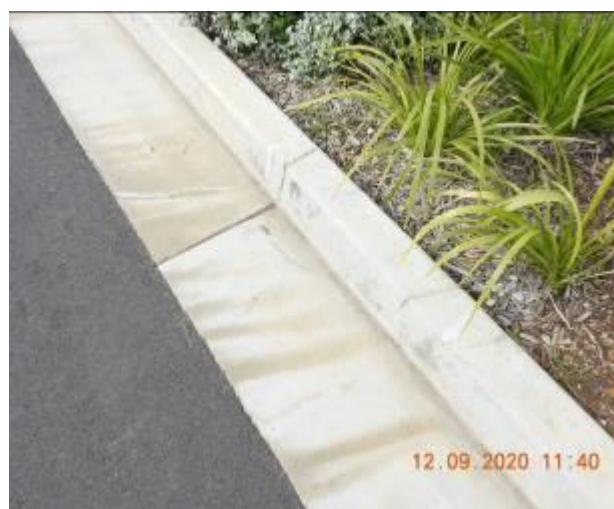
Figure 1286 – Crack propagation and loss of material through kerb and gutter
