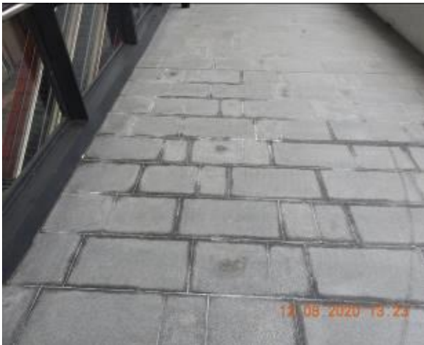
Figure 1956 – Efflorescence, crack propagation and loss of material through floor tiles
