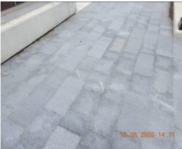
Figure 2281 – Efflorescence and crack propagation through walkway floor
