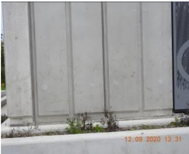
Figure 2314 – Evidence of patchwork through external wall
