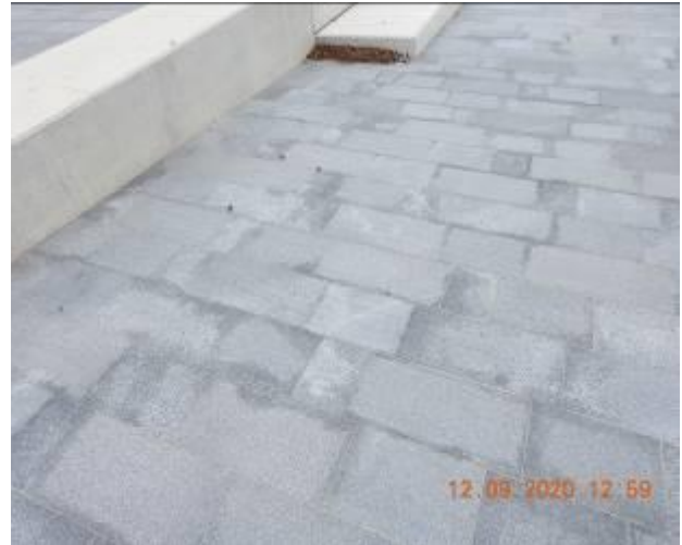
Figure 254 – Hairline cracking and efflorescence through footpath pavement
