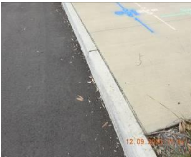
Figure 1343 – Loss of material through kerb
