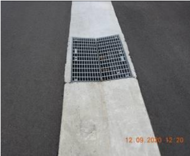
Figure 990 – Loss of material through gutter
