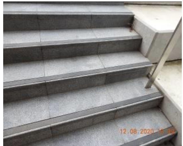
Figure 2083 – Separation through staircase pavement
