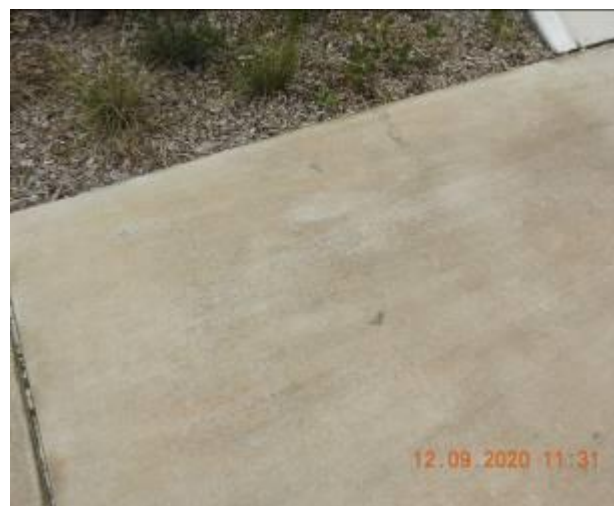
Figure 1152 – Loss of material through driveway pavement
