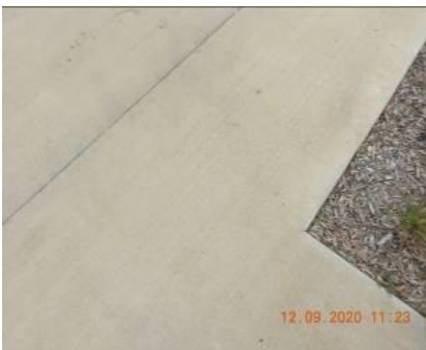
Figure 1075 – Hairline crack propagation through footpath pavement
