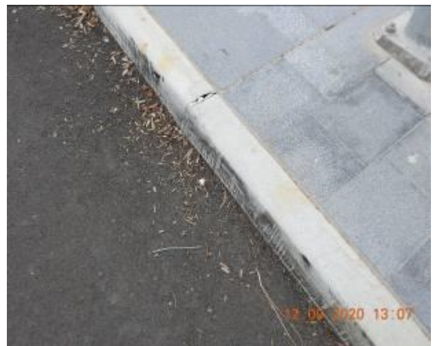
Figure 408 – Crack propagation and loss of material through kerb
