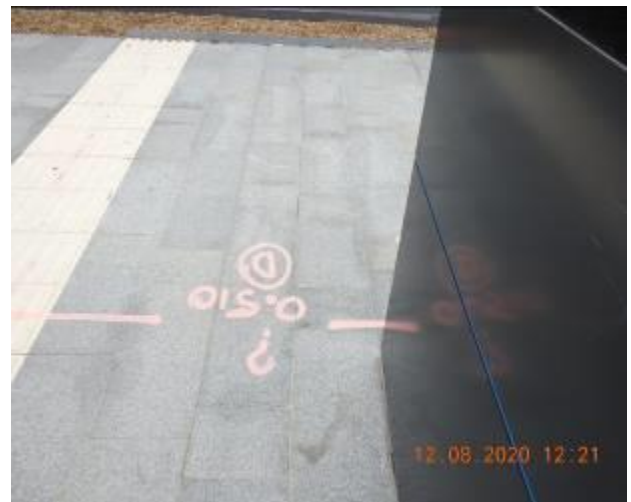
Figure 496 – Loss of material through footpath pavement
