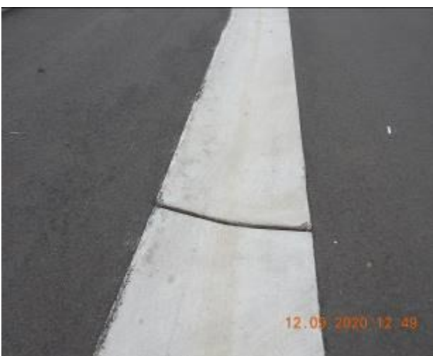
Figure 167 – Crack propagation and loss of material through gutter
