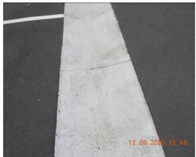
Figure 120 – Crack propagation through gutter
