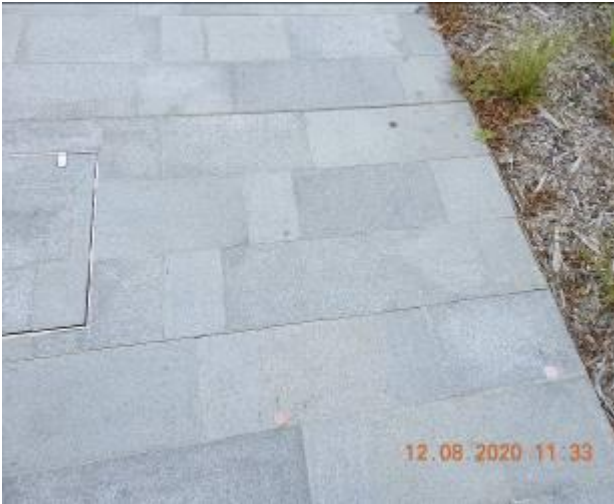
Figure 1607 – Crack propagation and loss of material through footpath pavement
