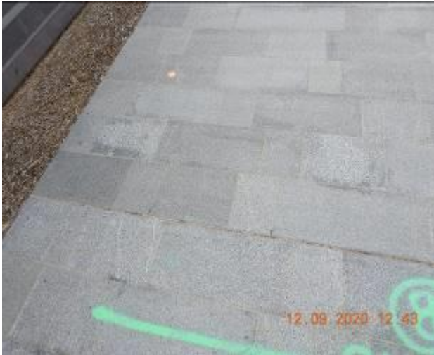
Figure 43 – Hairline cracking and efflorescence through footpath pavement
