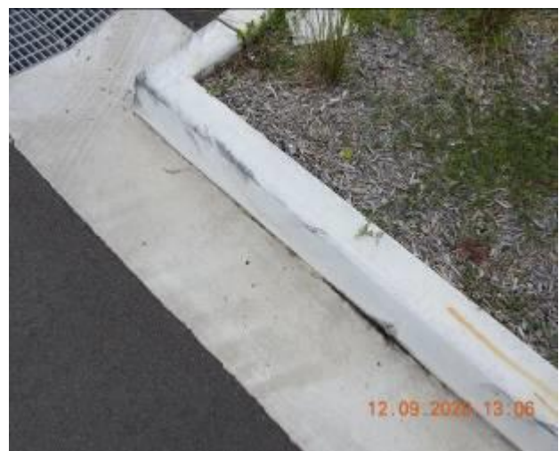
Figure 384 – Crack propagation through kerb
