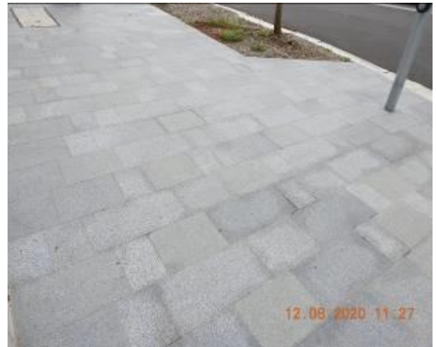
Figure 1568 – Loss of material through footpath pavement
