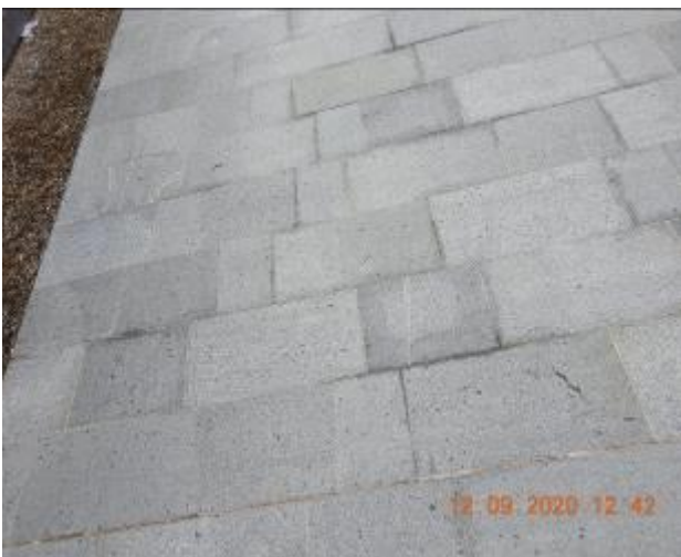
Figure 17 – Efflorescence through footpath pavement
