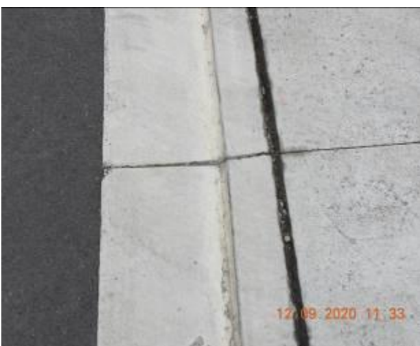
Figure 1177 – Loss of material through layback and gutter
