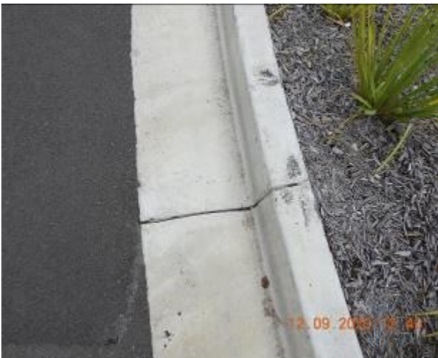
Figure 93 – Crack propagation through kerb
