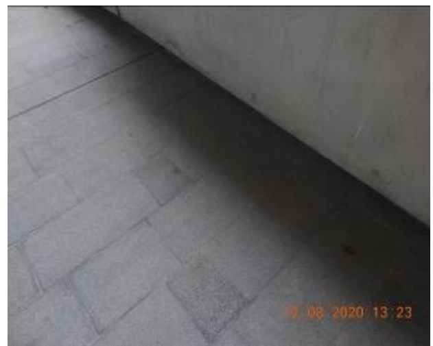
Figure 1963 – Efflorescence through floor tiles
