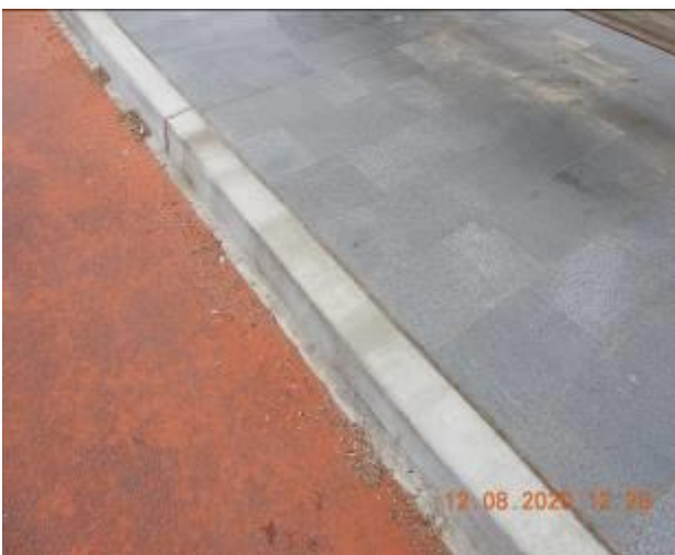
Figure 577 – Evidence of patchwork, crack propagation and loss of material through kerb
