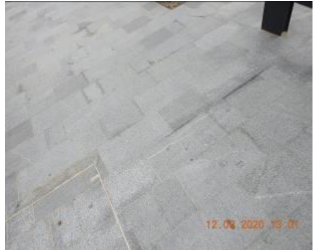
Figure 302 – Hairline cracking and efflorescence through footpath pavement
