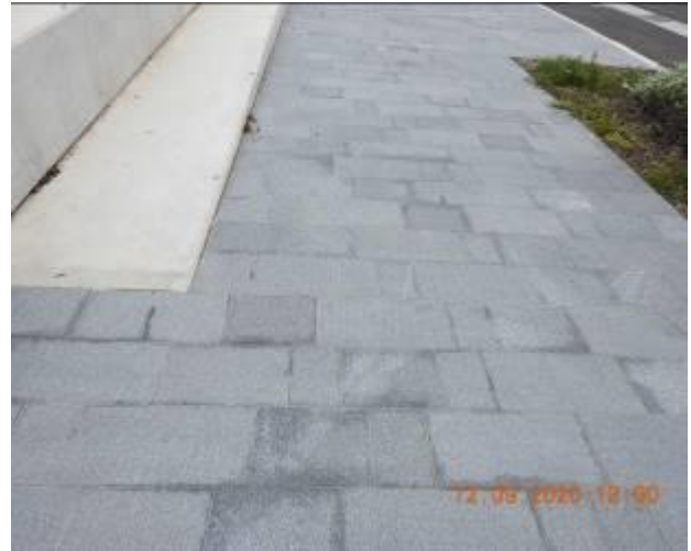
Figure 266 – Hairline cracking and efflorescence through footpath pavement
