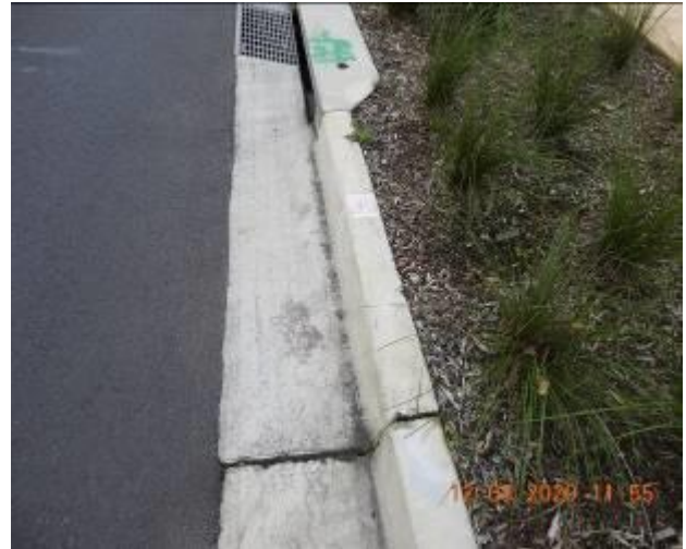
Figure 1764 – Loss of material through kerb and gutter
