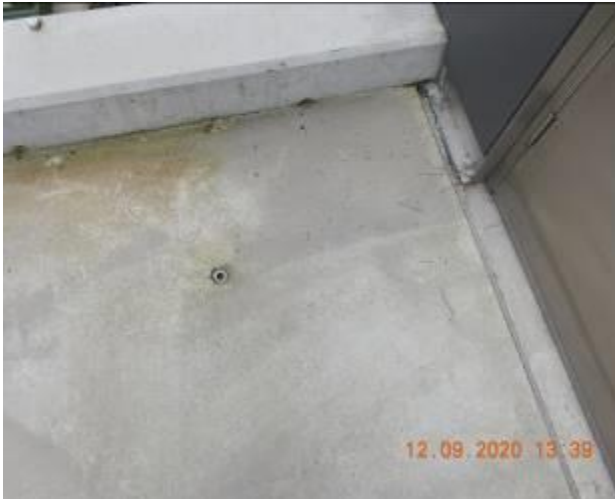
Figure 2402 – Loss of material through walkway pavement
