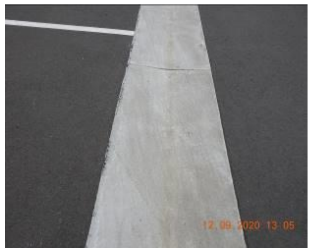
Figure 372 – Crack propagation through gutter
