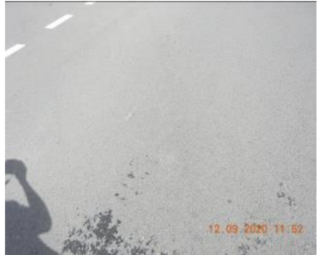
Figure 1420 – Loss of material through road surface
