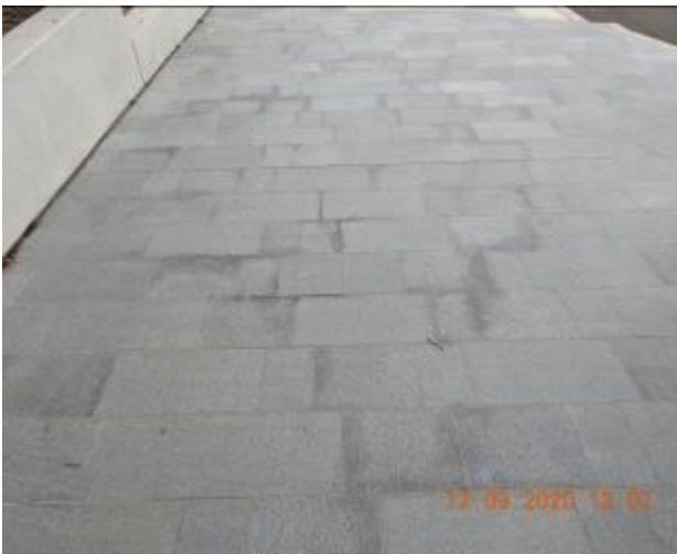
Figure 321 – Hairline cracking and efflorescence through footpath pavement
