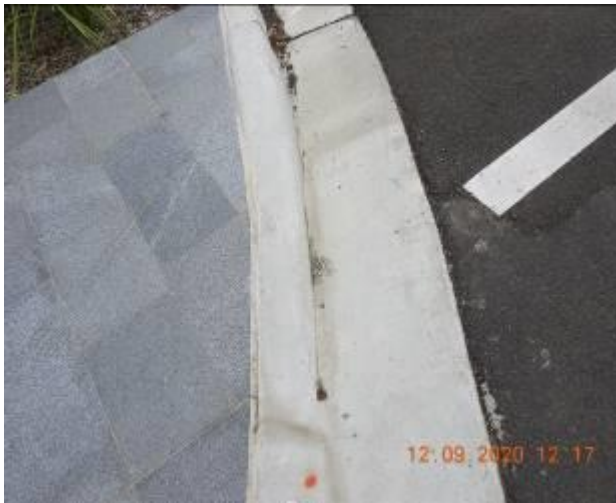
Figure 938 – Crack propagation and loss of material through layback and gutter
