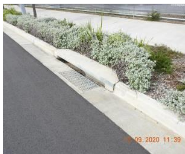
Figure 1272 – General condition of stormwater inlet pit/ Loss of material through kerb
