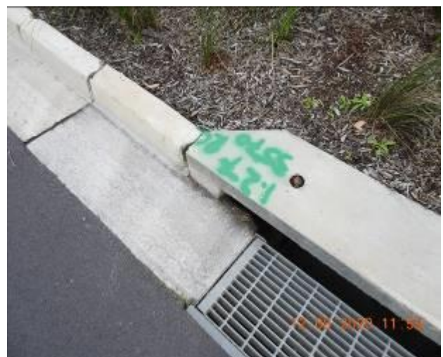
Figure 1768 – Loss of material through kerb and gutter
