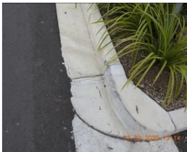
Figure 429 – Evidence of patchwork, crack propagation and loss of material through kerb and gutter
