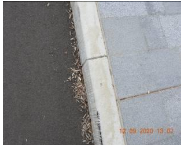
Figure 400 – Crack propagation through kerb
