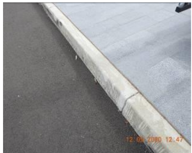
Figure 108 – Crack propagation through kerb
