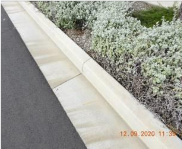
Figure 1275 – Crack propagation and loss of material through kerb and gutter
