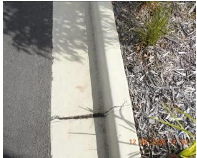
Figure 1712 – Loss of material through kerb and gutter
