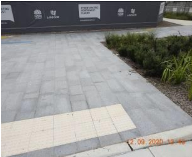
Figure 81 – Hairline cracking and efflorescence through footpath pavement
