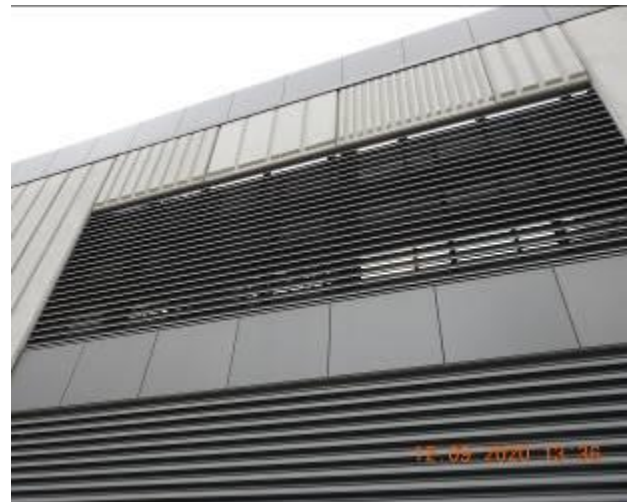
Figure 2375 – Loss of material through external wall
