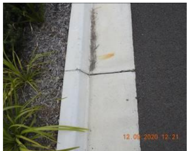
Figure 1001 – Crack propagation and loss of material through kerb and gutter
