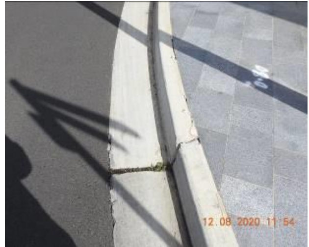
Figure 1758 – Crack propagation and loss of material through kerb and gutter
