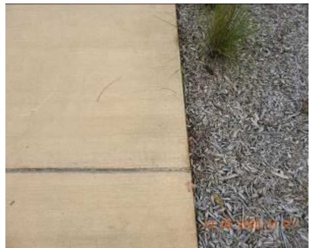
Figure 1520 – Loss of material through footpath pavement
