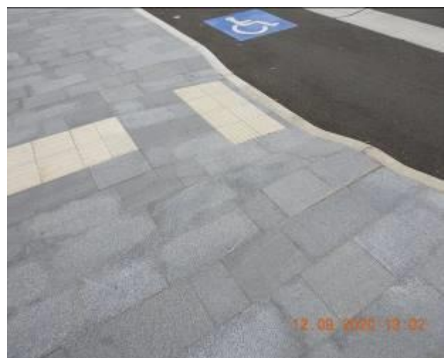
Figure 324 – Hairline cracking and efflorescence through footpath pavement
