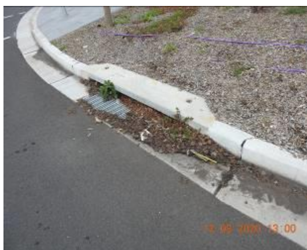
Figure 841 – General condition of stormwater inlet pit
