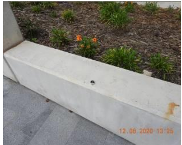
Figure 1981 – Loss of material through retaining wall
