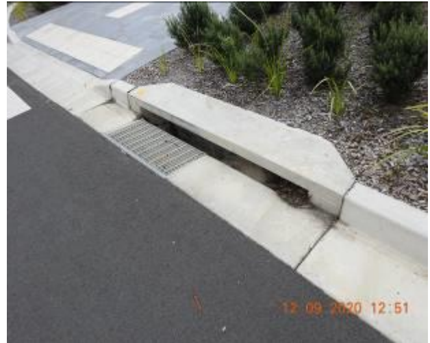
Figure 176 – General condition of kerb inlet pit and stormwater inlet pit
