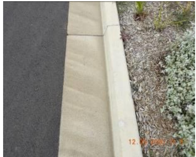
Figure 1242 – Evidence of patchwork through kerb
