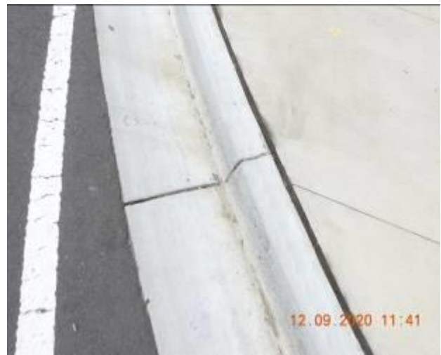
Figure 1302 – Crack propagation and loss of material through kerb
