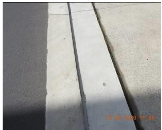
Figure 1774 – Loss of material through layback
