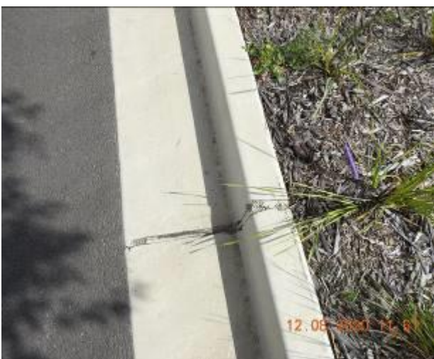
Figure 1725 – Crack propagation and loss of material through kerb and gutter
