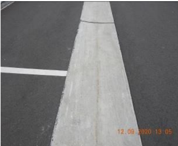
Figure 375 – Crack propagation through gutter
