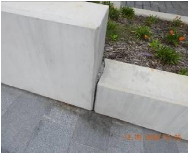
Figure 1984 – Loss of material through retaining wall
