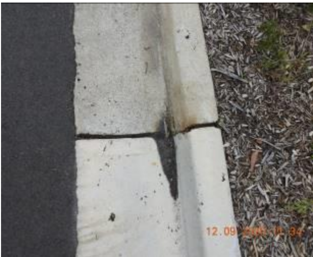
Figure 1199 – Loss of material through kerb and gutter
