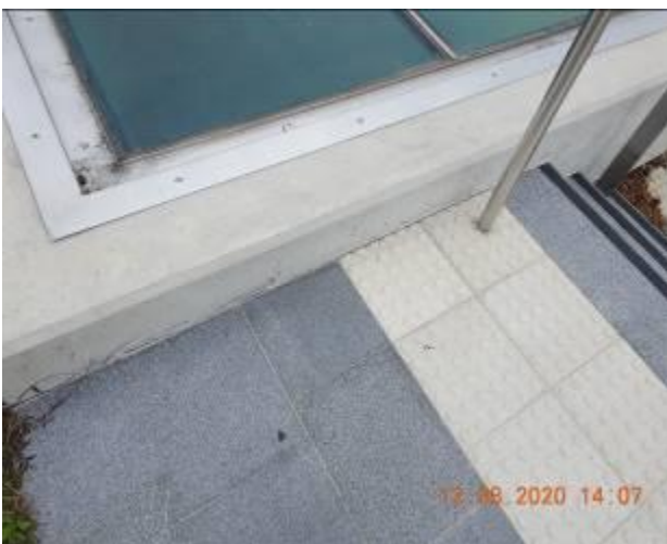
Figure 2229 – Separation through staircase floor
