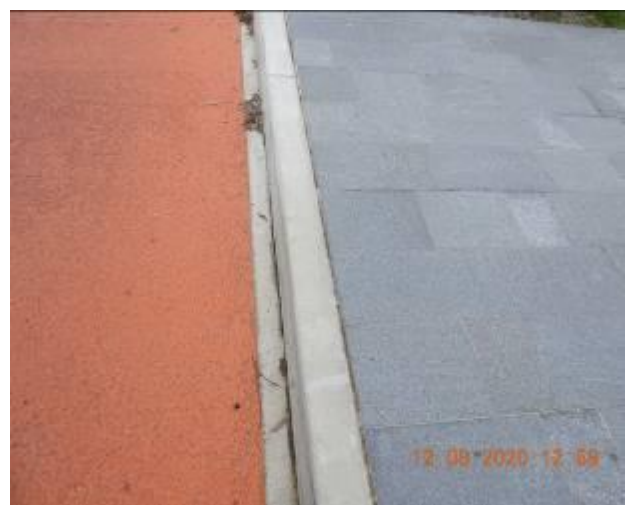
Figure 808 – Hairline crack propagation and evidence of patchwork through kerb
