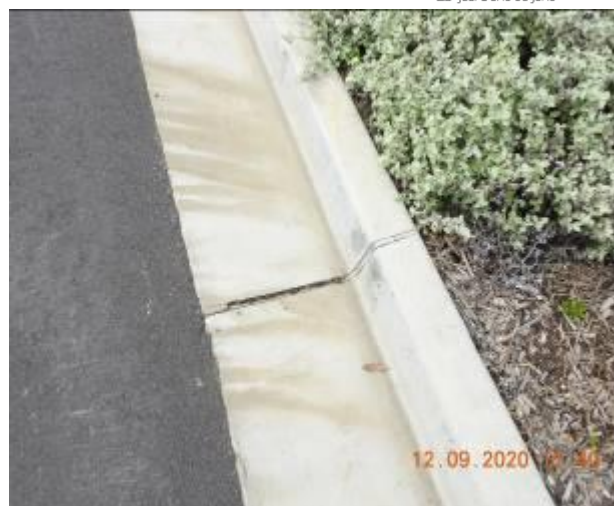
Figure 1288 – Crack propagation and loss of material through kerb and gutter
