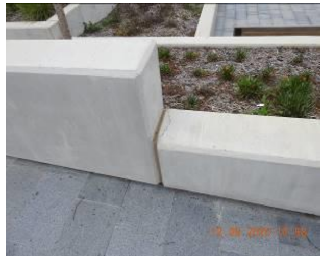
Figure 2152 – Crack propagation and loss of material through retaining wall
