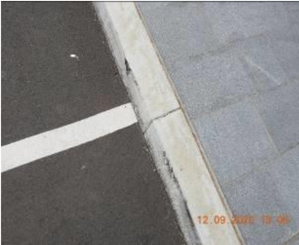
Figure 391 – Crack propagation through kerb
