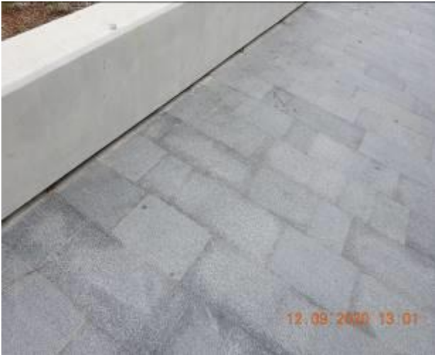
Figure 295 – Hairline cracking and efflorescence through footpath pavement
