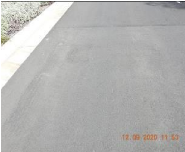
Figure 1433 – Loss of material through road surface
