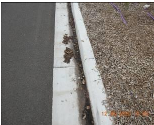
Figure 835 – Crack propagation and loss of material through kerb and gutter
