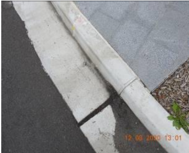
Figure 845 – Crack propagation and loss of material through kerb
