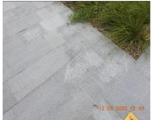
Figure 50 – Hairline cracking and efflorescence through footpath pavement
