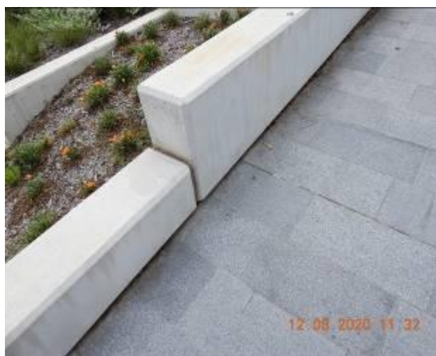
Figure 1603 – Crack propagation through showground retaining wall
