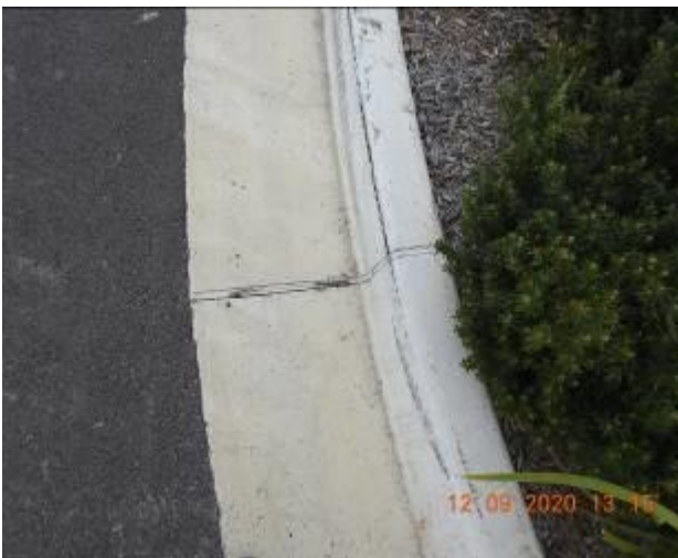
Figure 441 – Crack propagation through kerb and gutter
