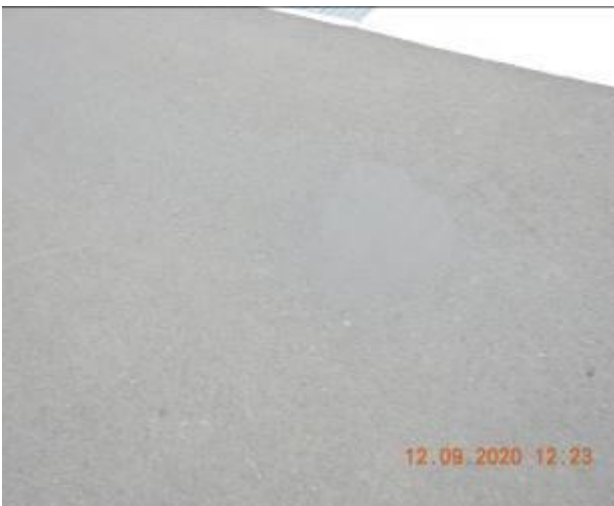
Figure 1016 – Evidence of patchwork through road surface
