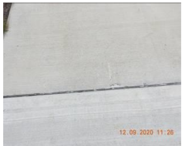
Figure 1100 – Loss of material through footpath pavement
