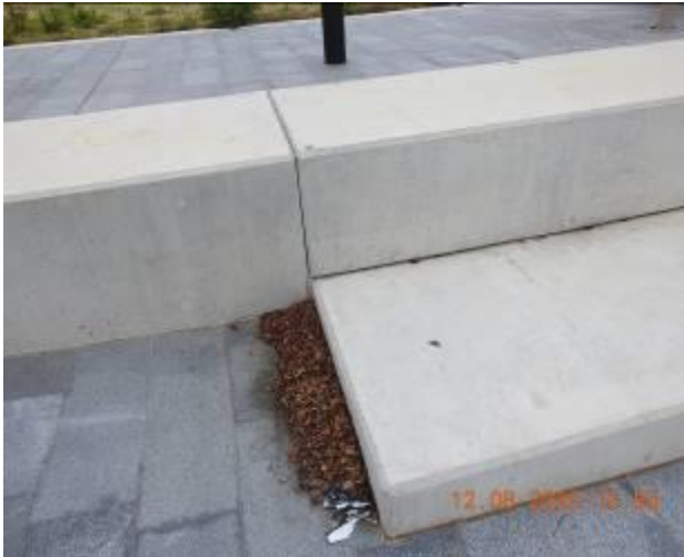
Figure 2129 – Separation through retaining wall
