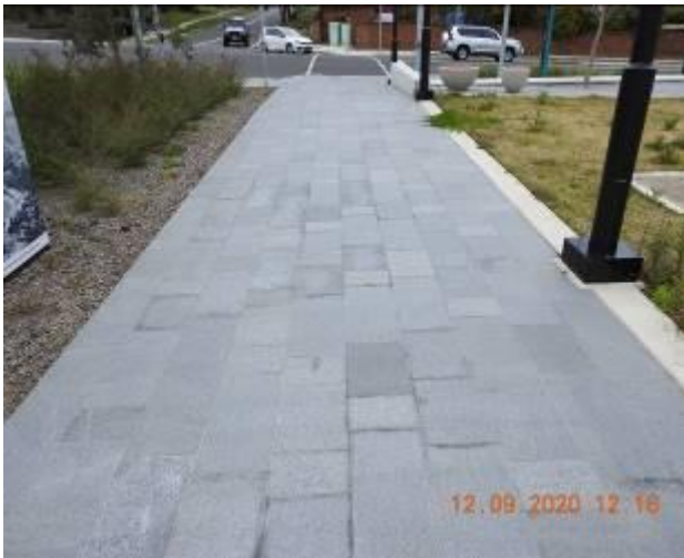
Figure 914 – Loss of material through footpath pavement
