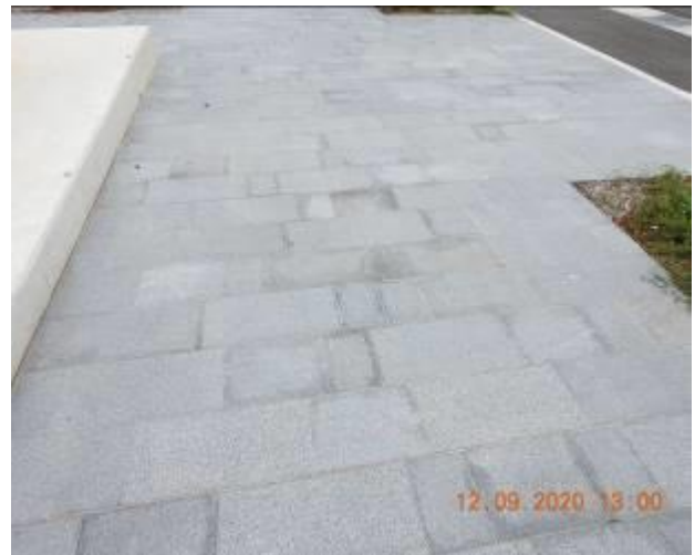
Figure 268 – Hairline cracking and efflorescence through footpath pavement
