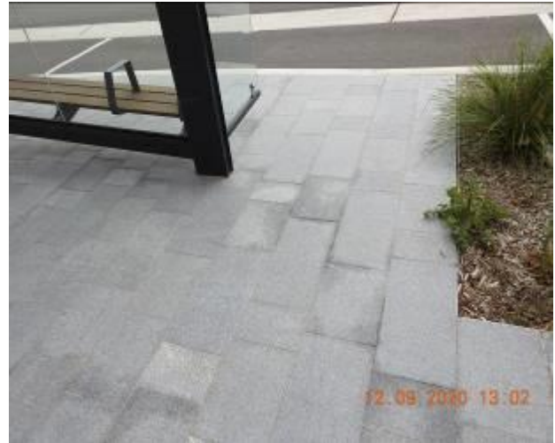
Figure 314 – Hairline cracking and efflorescence through footpath pavement
