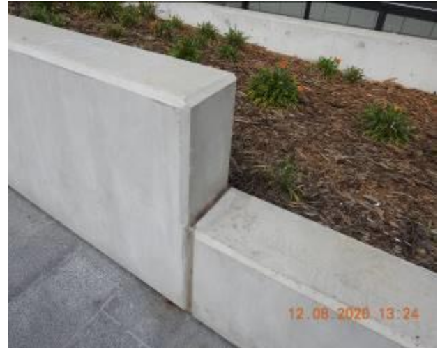
Figure 1979 – Crack propagation and loss of material through retaining wall
