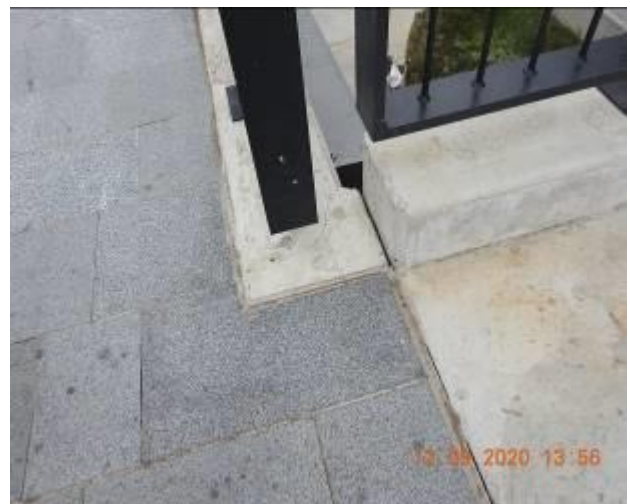
Figure 2527 – Crack propagation through boundary wall
