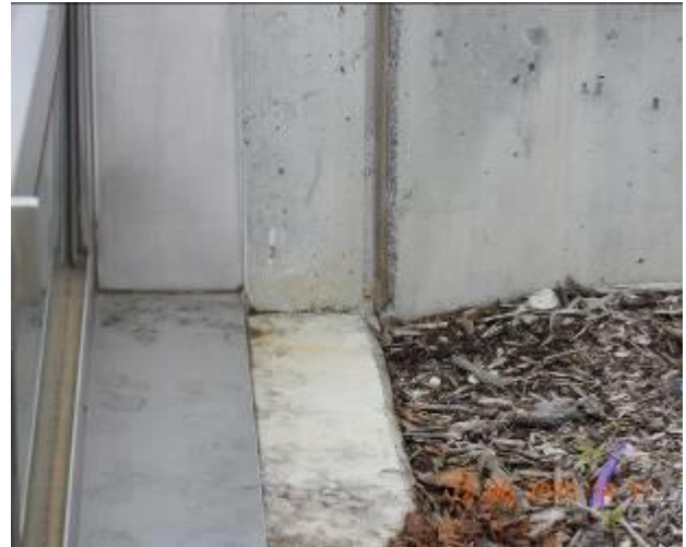
Figure 2274 – Crack propagation and loss of material through retaining wall
