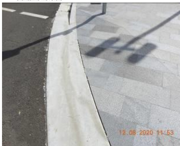
Figure 1751 – Loss of material through layback
