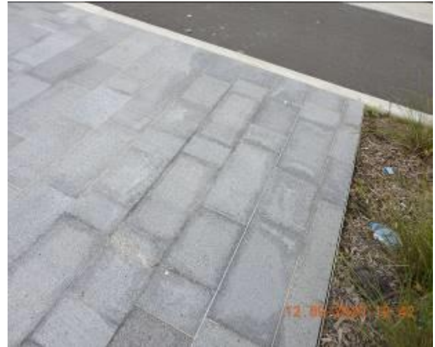
Figure 20 – Hairline cracking and efflorescence through footpath pavement
