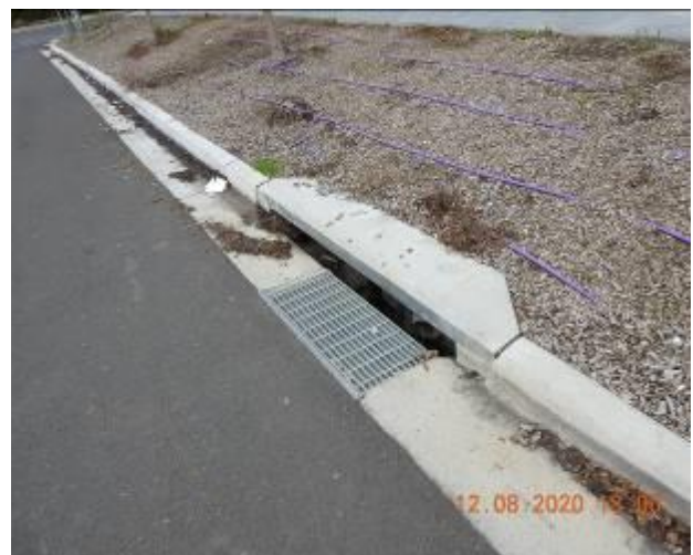
Figure 826 – General condition of stormwater inlet pit
