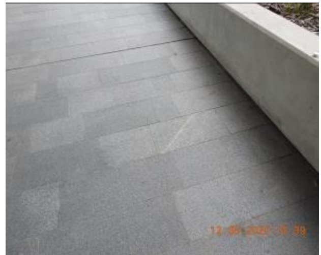
Figure 2077 – Hairline crack propagation through floor tiles
