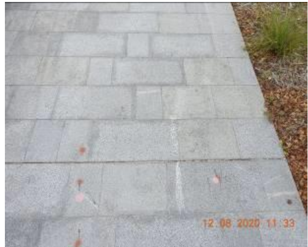
Figure 1610 – Efflorescence and hairline crack propagation through footpath pavement
