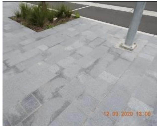
Figure 280 – Hairline cracking and efflorescence through footpath pavement
