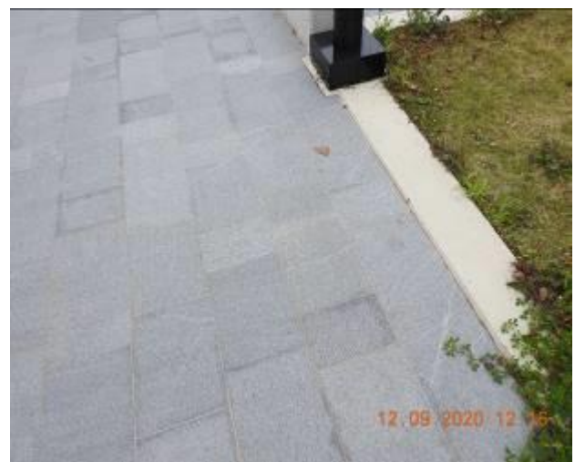
Figure 923 – Efflorescence and crack propagation through footpath pavement
