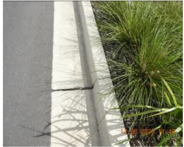
Figure 1704 – Crack propagation and loss of material through kerb and gutter
