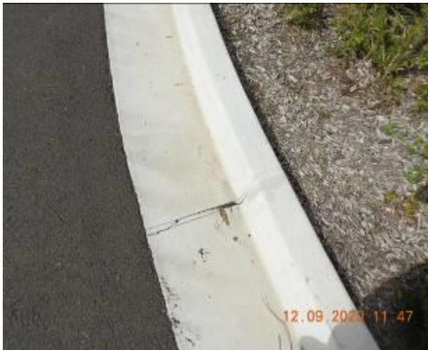
Figure 1379 – Crack propagation and loss of material through kerb and gutter
