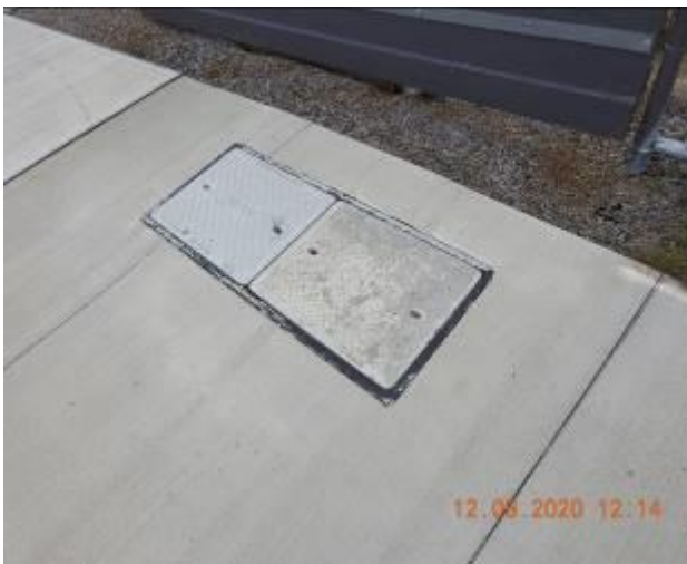
Figure 896 – Loss of material through service pit pavement
