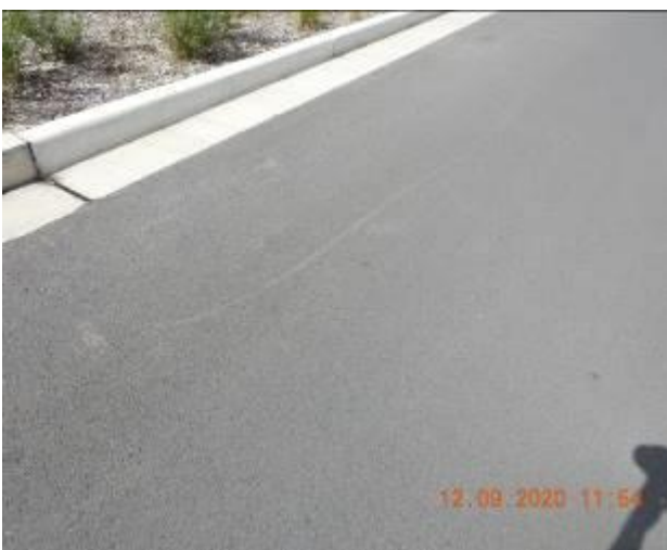
Figure 1447 – Loss of material through road surface
