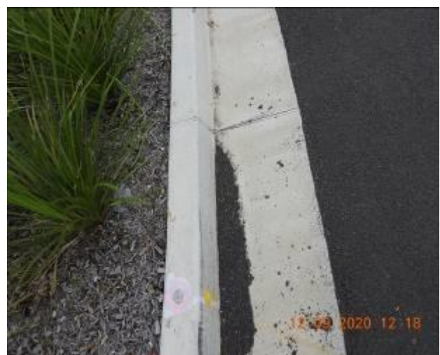
Figure 941 – Crack propagation and loss of material through kerb and gutter
