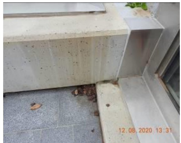
Figure 2007 – Loss of material through retaining wall
