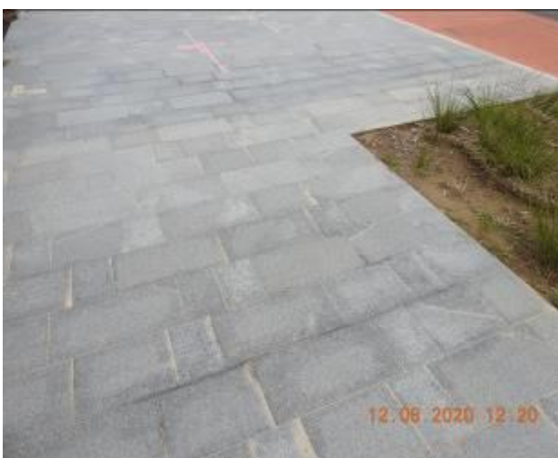
Figure 483 – Efflorescence and crack propagation through footpath pavement
