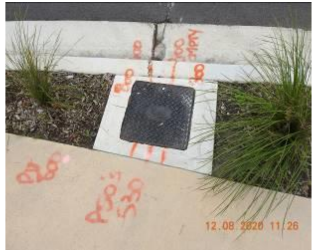
Figure 1562 – Crack propagation and loss of material through service pit pavement
