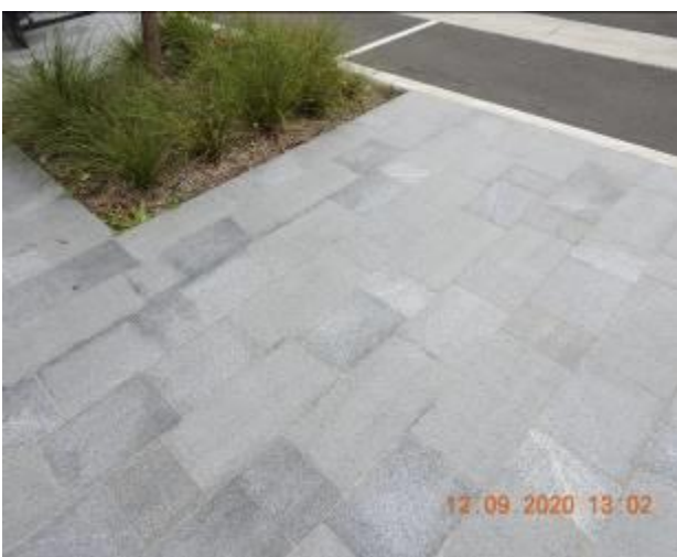
Figure 311 – Hairline cracking and efflorescence through footpath pavement
