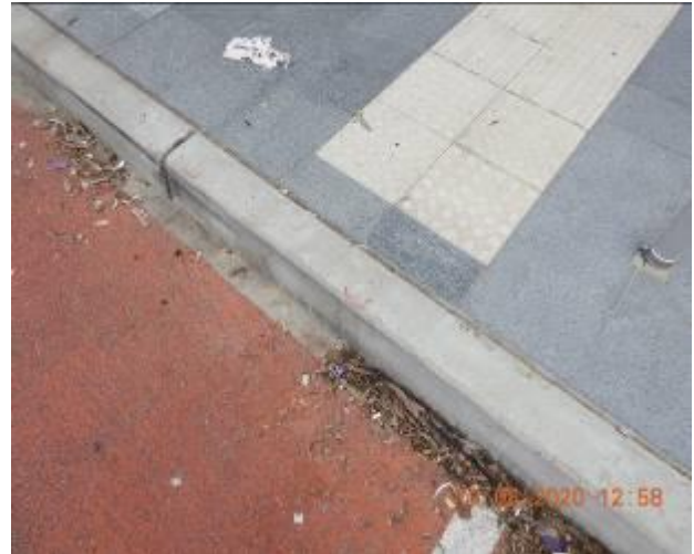
Figure 792 – Evidence of patchwork, crack propagation and loss of material through kerb
