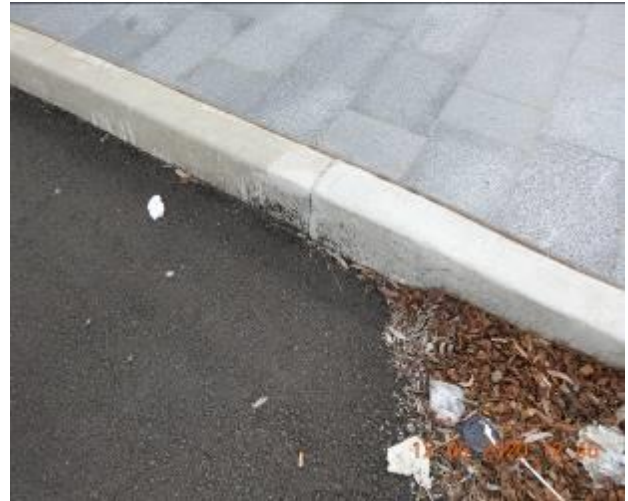
Figure 104 – Evidence of patchwork through kerb
