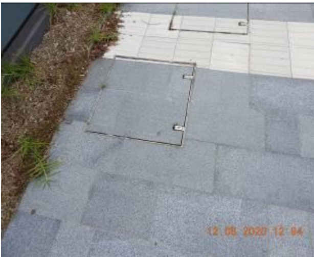
Figure 739 – Loss of material through service pit pavement
