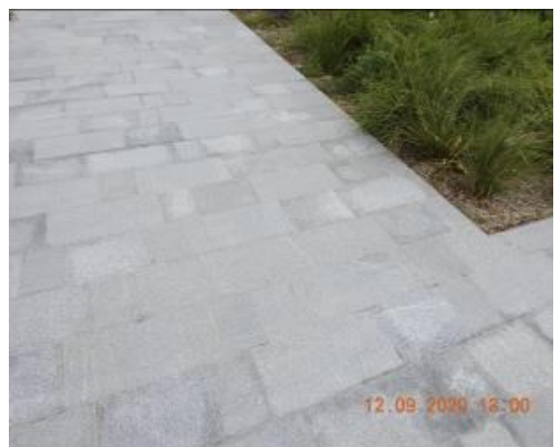
Figure 264 – Hairline cracking and efflorescence through footpath pavement
