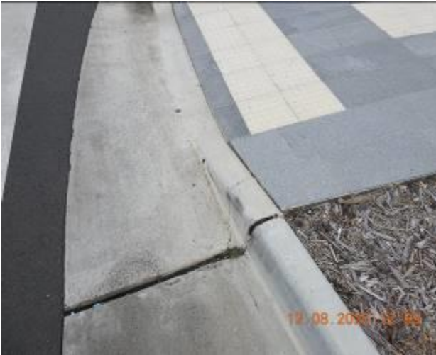
Figure 815 – Crack propagation and loss of material through kerb and gutter
