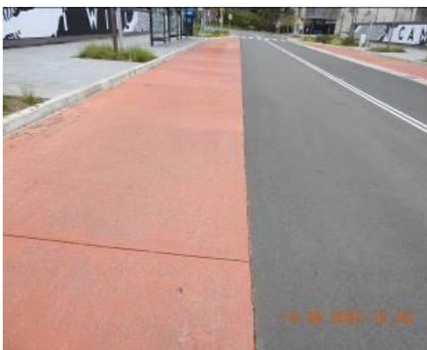
Figure 615 – Crack propagation and loss of material through road surface
