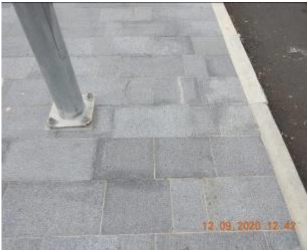
Figure 21 – Hairline cracking and efflorescence through footpath pavement
