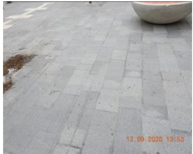
Figure 2477 – Hairline crack propagation through walkway floor
