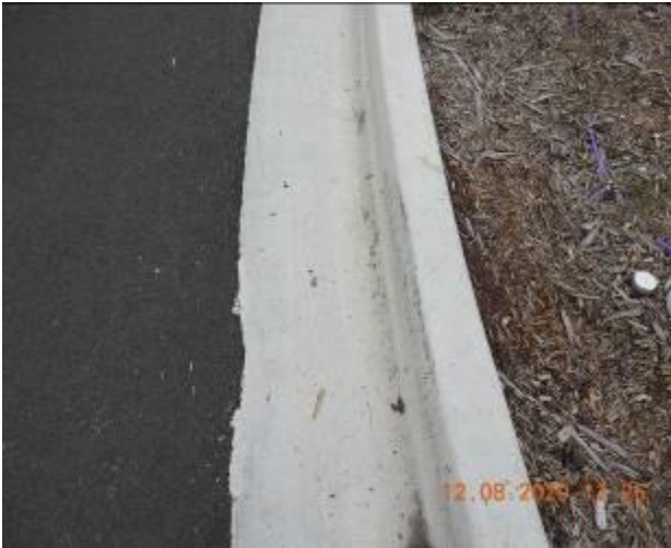
Figure 539 – Evidence of patchwork and hairline crack propagation through kerb and gutter
