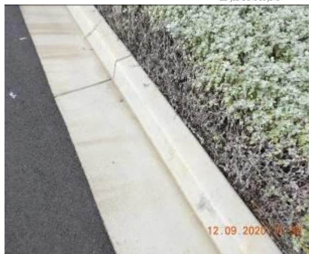
Figure 1264 – Crack propagation through kerb
