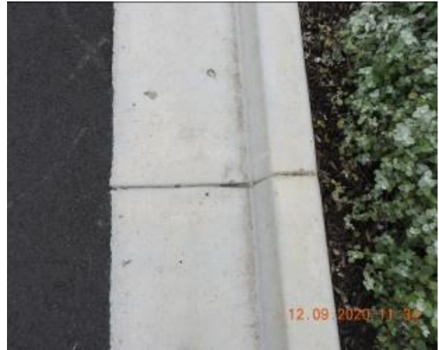
Figure 1198 – Crack propagation and loss of material through kerb and gutter
