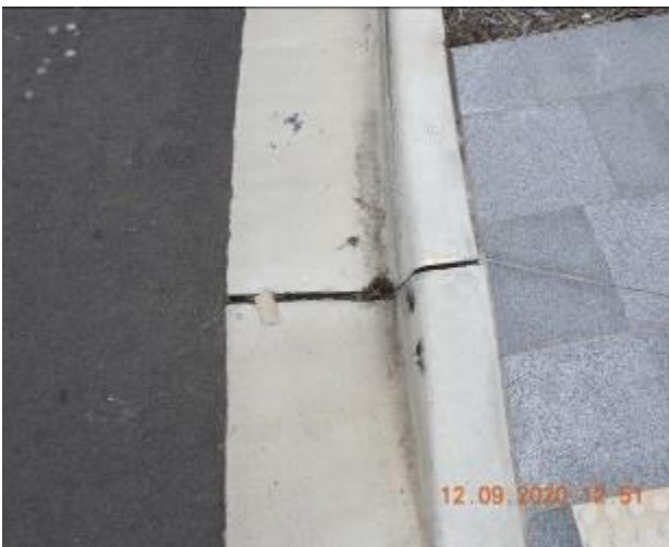
Figure 179 – Loss of material through kerb
