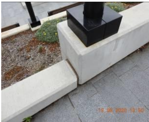
Figure 2101 – Crack propagation and loss of material through retaining wall
