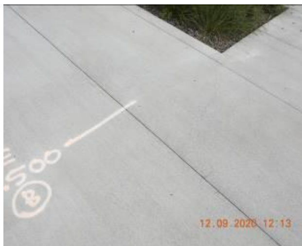
Figure 890 – Crack propagation through footpath pavement
