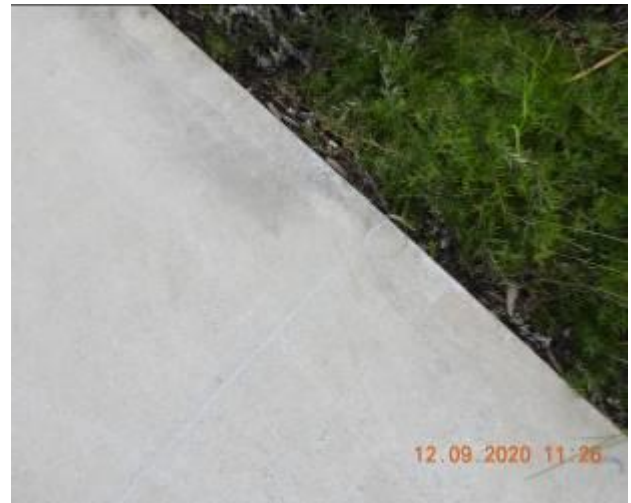
Figure 1104 – Crack propagation through footpath pavement
