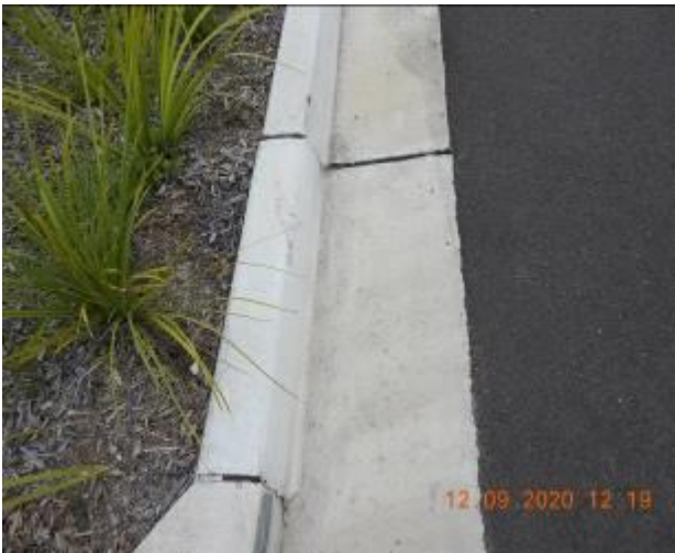
Figure 968 – Loss of material through kerb
