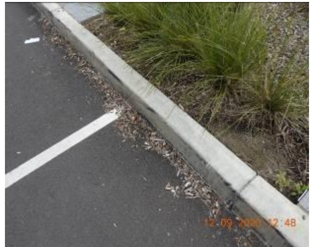
Figure 148 – Crack propagation through kerb
