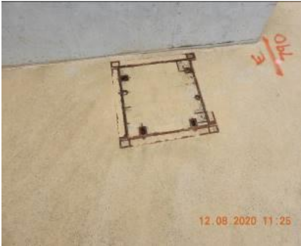
Figure 1547 – Loss of material through service pit pavement
