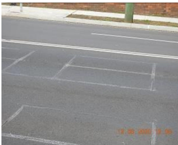
Figure 1849 – Evidence of patchwork and loss of material through road surface
