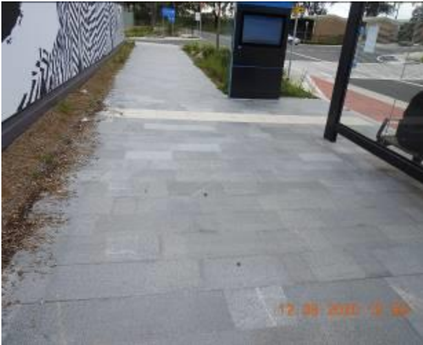
Figure 767 – Hairline crack propagation through footpath pavement
