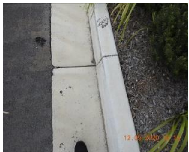
Figure 438 – Crack propagation and loss of material through kerb and gutter
