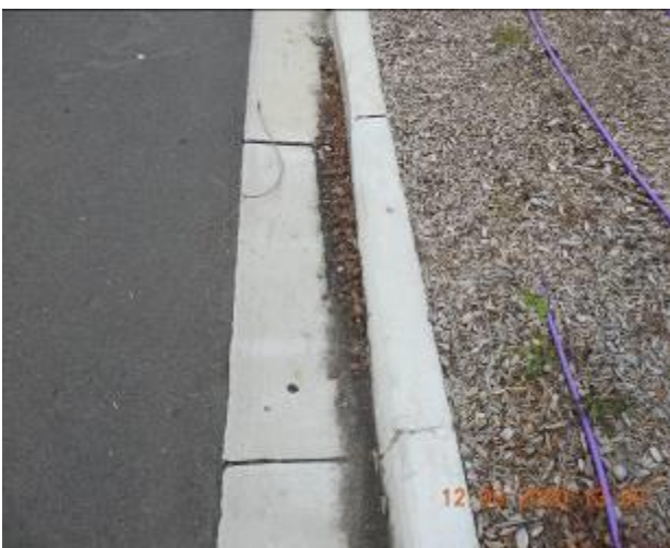
Figure 825 – Crack propagation and loss of material through kerb and gutter
