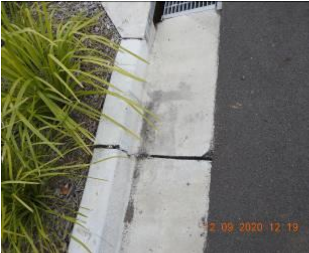
Figure 966 – Crack propagation and loss of material through kerb and gutter
