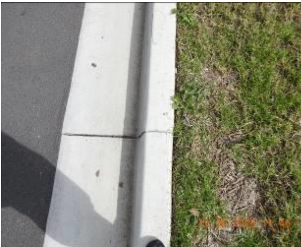
Figure 1675 – Crack propagation and loss of material through kerb and gutter
