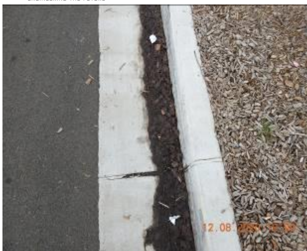
Figure 833 – Crack propagation and loss of material through kerb and gutter
