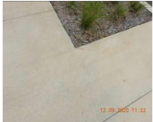
Figure 1062 – Hairline crack propagation through footpath pavement
