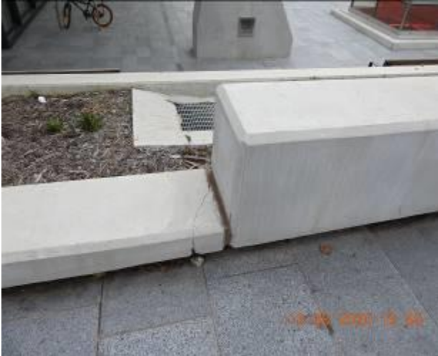
Figure 2098 – Crack propagation and loss of material through retaining wall
