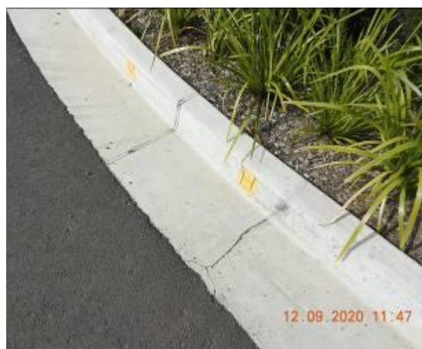
Figure 1376 – Crack propagation and loss of material through kerb and gutter
