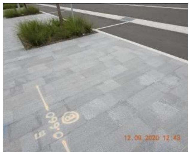
Figure 36 – Hairline cracking and efflorescence through footpath pavement
