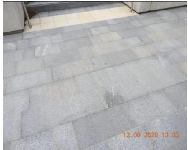
Figure 2035 – Crack propagation and loss of material through floor tiles
