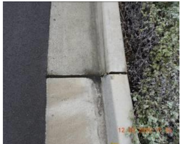
Figure 1206 – Loss of material through kerb and gutter
