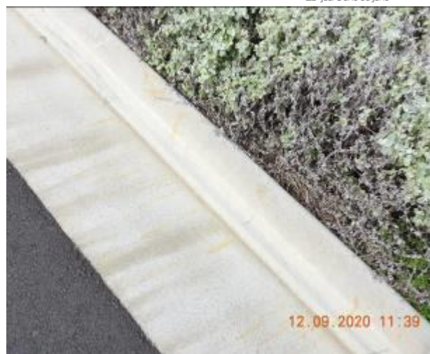
Figure 1270 – Hairline crack propagation through kerb
