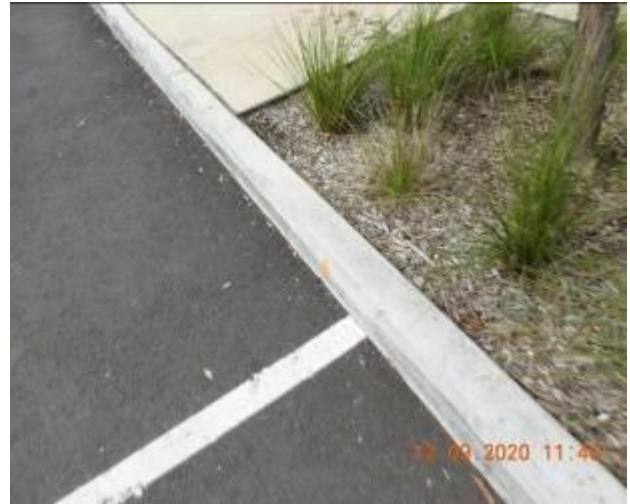
Figure 1360 – Crack propagation through kerb
