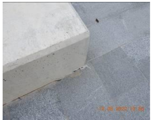
Figure 2140 – Loss of material through retaining wall
