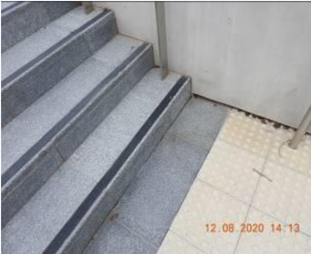
Figure 2303 – Crack propagation and loss of material through staircase floor
