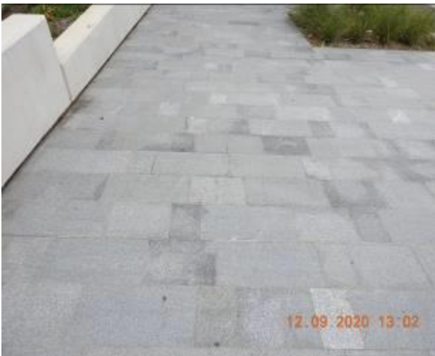
Figure 309 – Hairline cracking and efflorescence through footpath pavement
