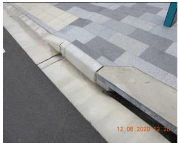
Figure 554 – Crack propagation and loss of material through kerb
