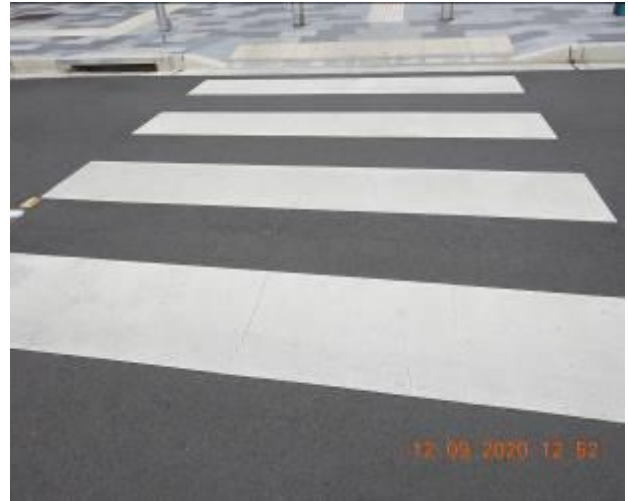
Figure 188 – Crack propagation through road surface
