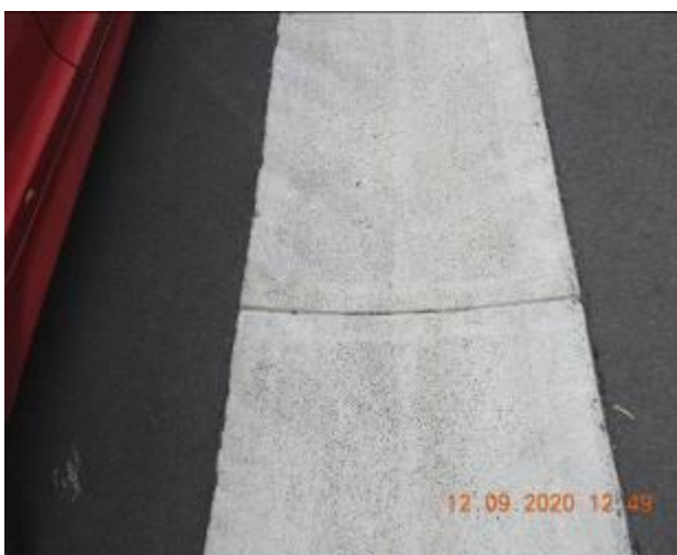
Figure 173 – Evidence of patchwork through gutter
