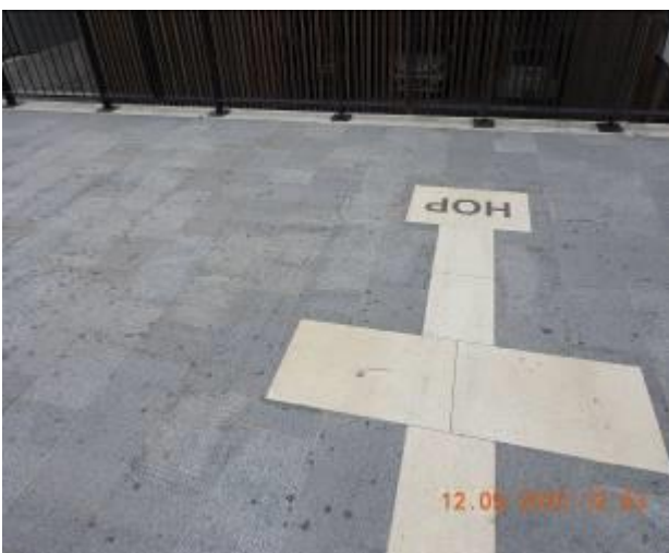
Figure 2472 – Hairline crack propagation through walkway floor
