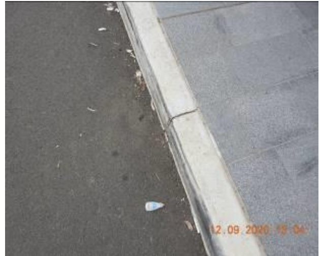
Figure 356 – Crack propagation through kerb
