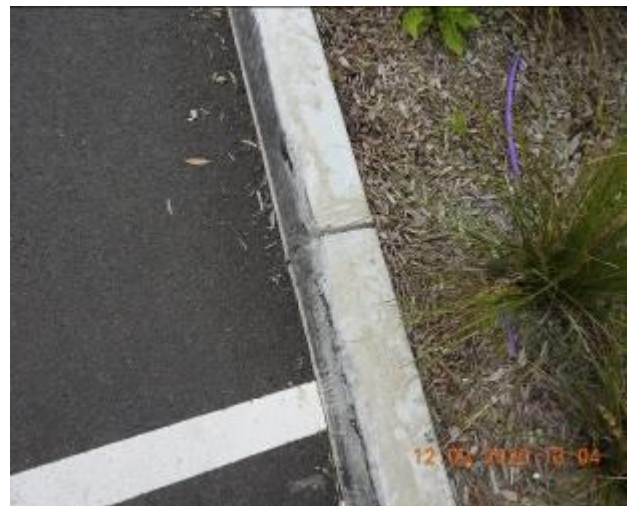
Figure 364 – Crack propagation through kerb
