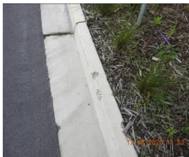
Figure 1738 – Loss of material through kerb and gutter
