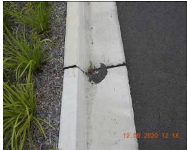
Figure 951 – Crack propagation and loss of material through kerb
