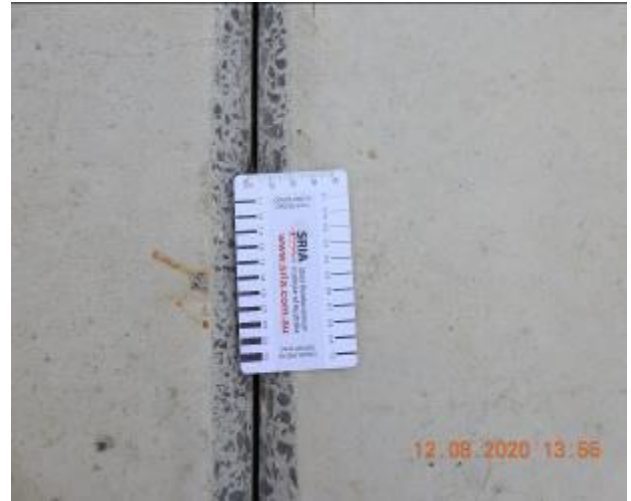
Figure 2130 – Separation through retaining wall Approx. 3mm in width
