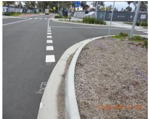
Figure 548 – Evidence of patchwork through gutter
