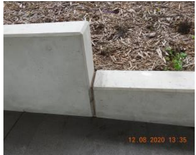
Figure 2053 – Crack propagation and loss of material through retaining wall
