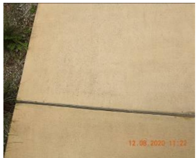
Figure 1522 – Separation through footpath pavement
