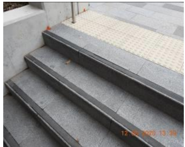
Figure 2085 – Separation through staircase pavement
