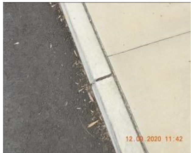
Figure 1322 – Loss of material through kerb
