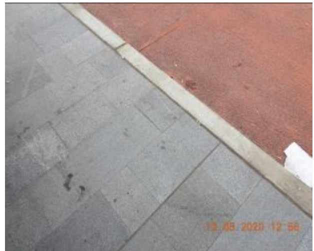
Figure 770 – Hairline crack propagation through footpath pavement
