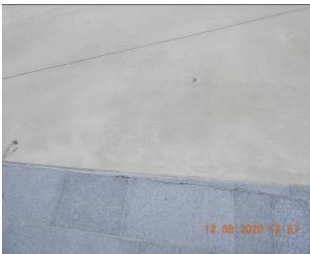
Figure 781 – Crack propagation and loss of material through footpath pavement
