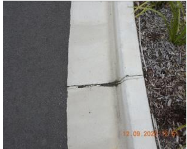
Figure 182 – Crack propagation and loss of material through kerb and gutter
