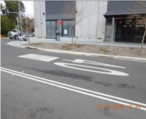
Figure 677 – Evidence of patchwork through road surface
