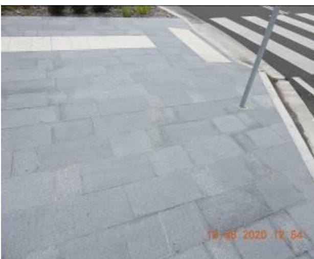
Figure 735 – Crack propagation and loss of material through footpath pavement
