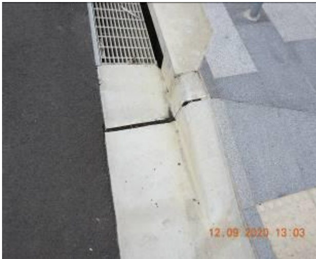
Figure 343 – Crack propagation and loss of material through kerb and gutter
