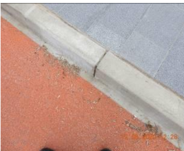
Figure 585 – Evidence of patchwork and loss of material through kerb
