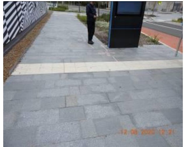
Figure 494 – Loss of material through footpath pavement
