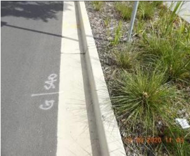
Figure 1705 – Loss of material through kerb
