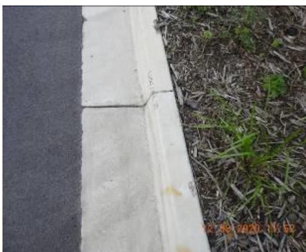
Figure 1737 – Loss of material through kerb
