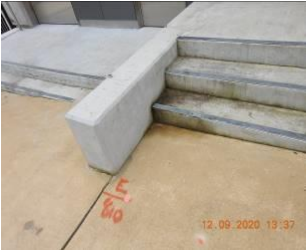
Figure 2390 – Crack propagation and loss of material through staircase pavement
