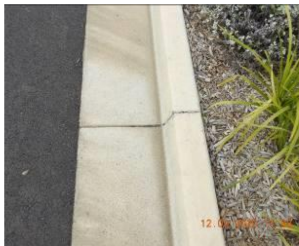
Figure 1250 – Crack propagation and loss of material through kerb and gutter
