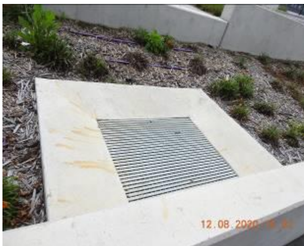
Figure 2018 – General condition of stormwater inlet pit
