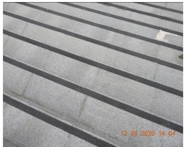
Figure 2200 – Loss of material through staircase floor
