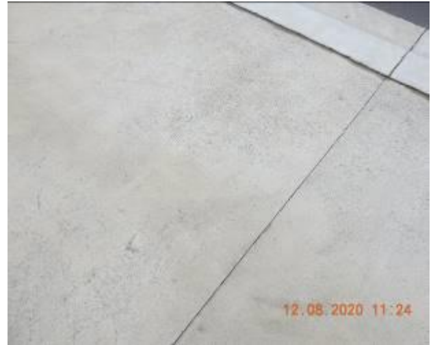
Figure 1542 – Loss of material through driveway pavement
