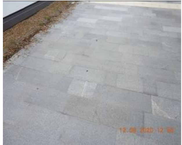
Figure 768 – Hairline crack propagation through footpath pavement
