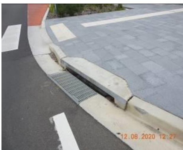
Figure 561 – General condition of stormwater inlet pit
