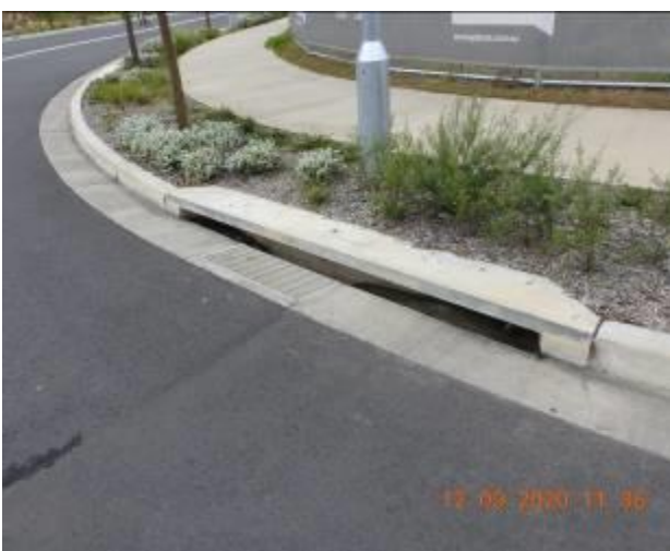
Figure 1231 – General condition of stormwater inlet pit/Crack propagation and loss of material through kerb and gutter
