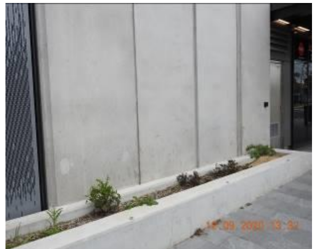
Figure 2323 – Evidence of patchwork through external wall
