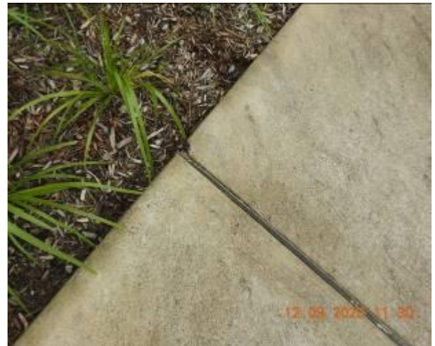
Figure 1140 – Loss of material through footpath pavement
