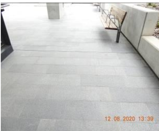
Figure 2078 – Hairline crack propagation through floor tiles
