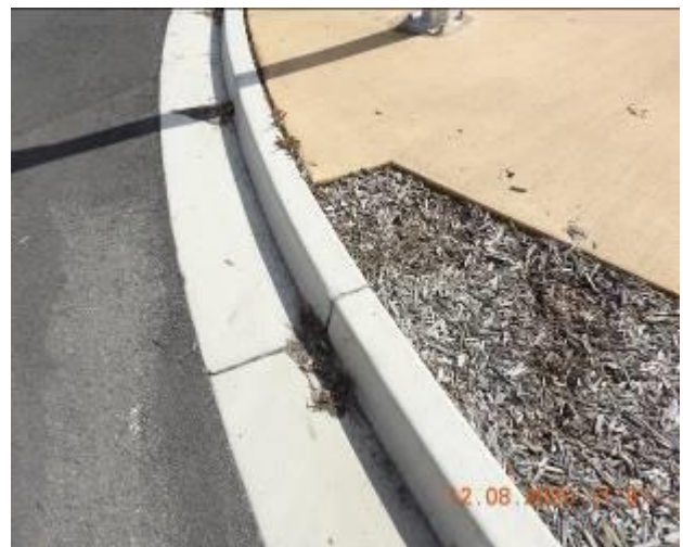
Figure 1798 – Crack propagation and loss of material through kerb
