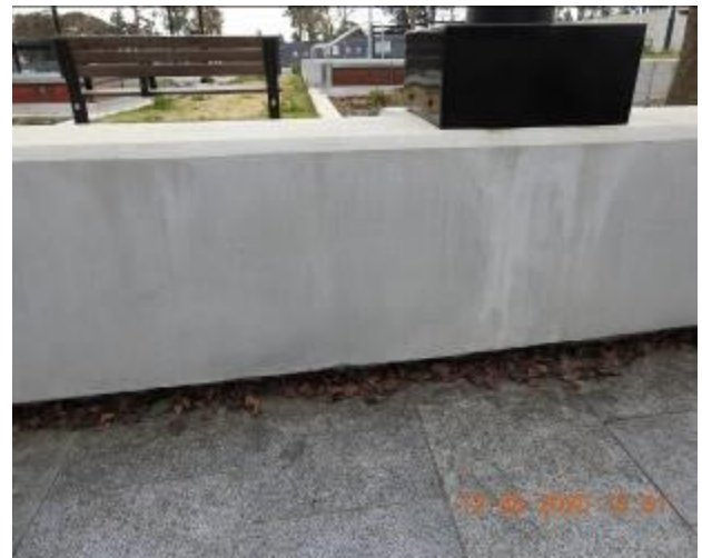
Figure 2108 – Hairline crack propagation through retaining wall
