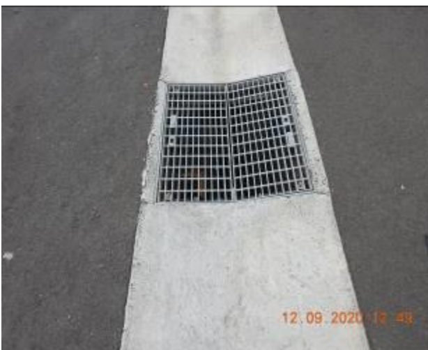
Figure 161 – General condition of stormwater inlet pit and crack propagation through gutter
