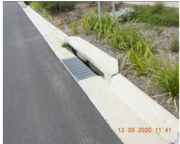
Figure 1308 – General condition of stormwater inlet pit/ Loss of material through kerb
