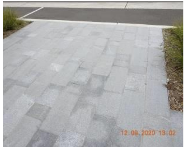
Figure 310 – Hairline cracking and efflorescence through footpath pavement
