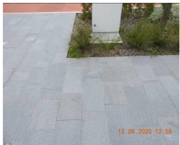
Figure 754 – Loss of material through footpath pavement
