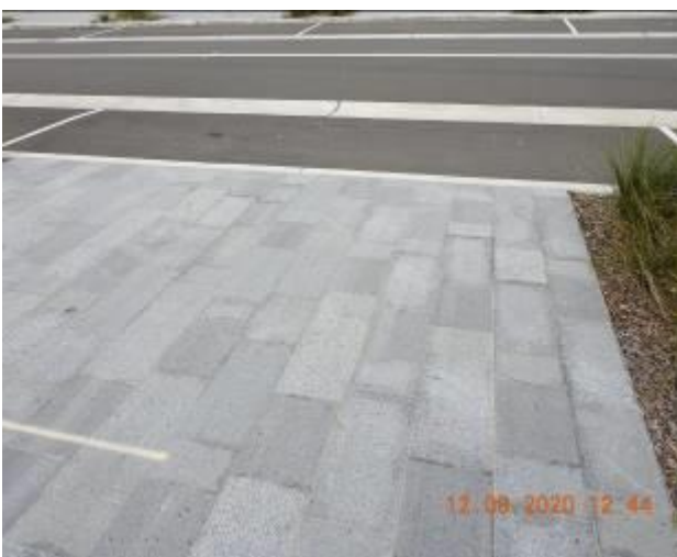
Figure 59 – Hairline cracking and efflorescence through footpath pavement
