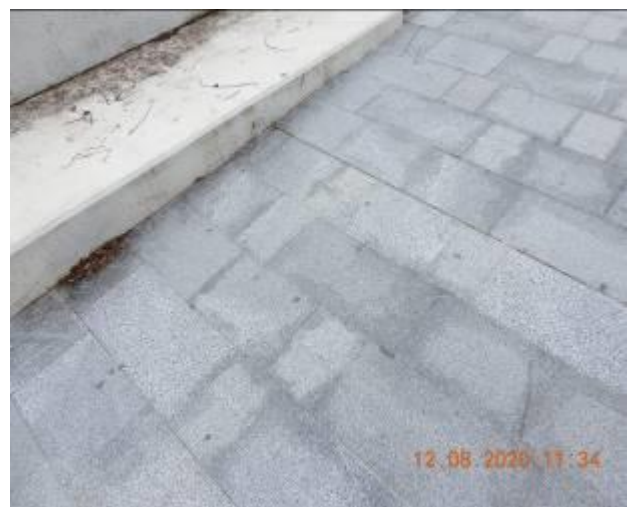
Figure 1624 – Crack propagation and loss of material through footpath pavement
