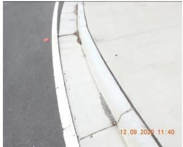
Figure 1296 – Crack propagation and loss of material through kerb and gutter
