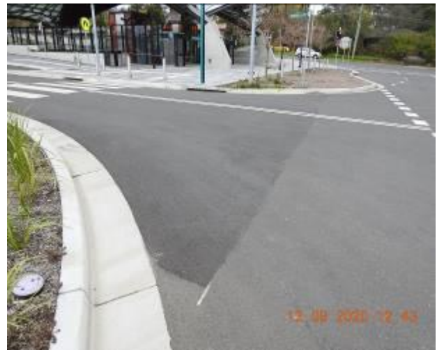
Figure 662 – Evidence of patchwork through road surface
