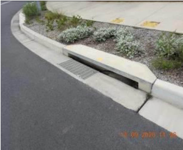
Figure 1227 – General condition of stormwater inlet pit
