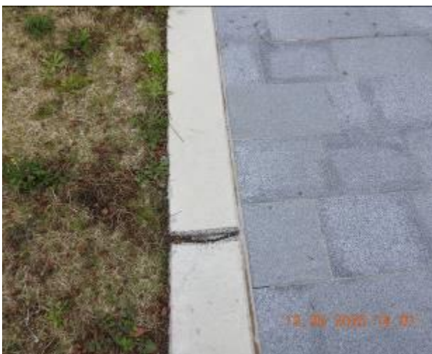
Figure 2163 – Loss of material through retaining wall
