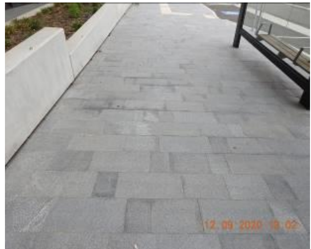
Figure 316 – Hairline cracking and efflorescence through footpath pavement
