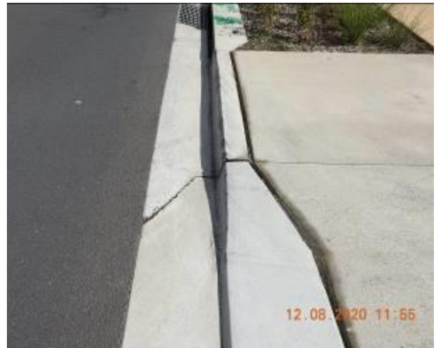
Figure 1778 – Loss of material through kerb and gutter
