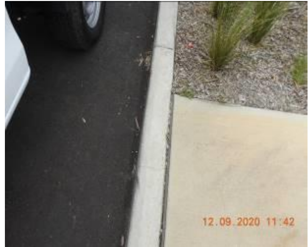
Figure 1318 – Crack propagation through kerb
