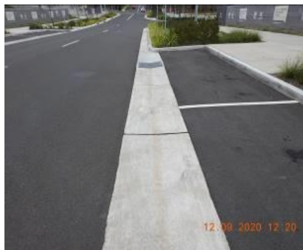
Figure 989 – Loss of material through gutter/General condition of stormwater inlet pit
