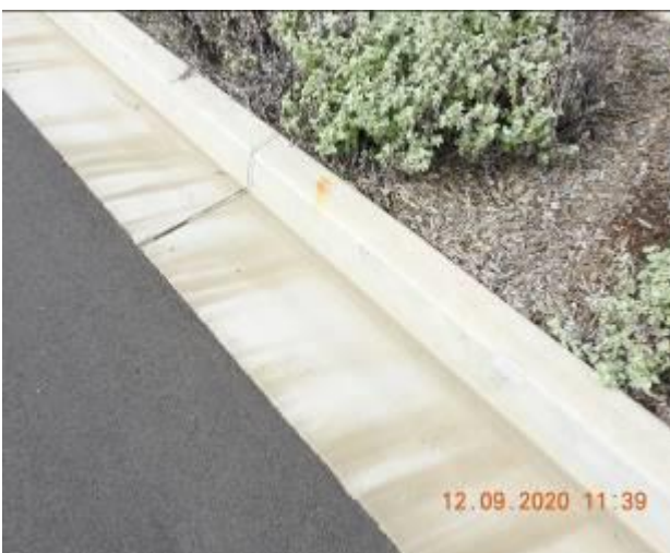
Figure 1279 – Evidence of patchwork and loss of material through kerb and gutter
