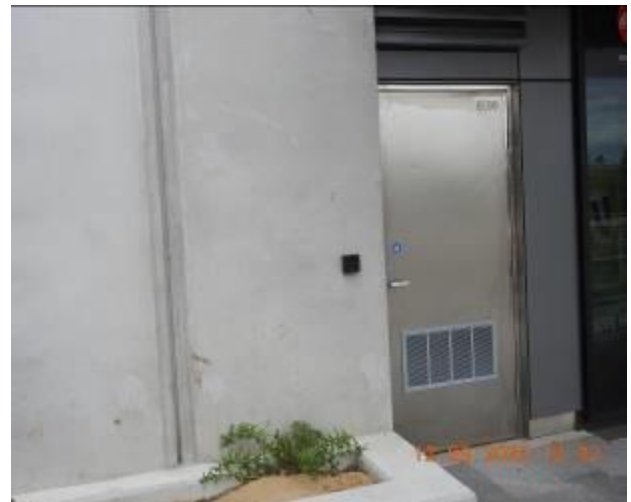
Figure 2327 – Evidence of patchwork through external wall
