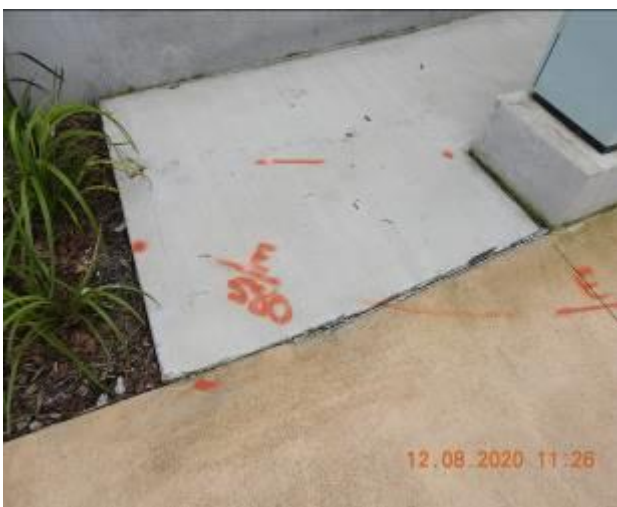
Figure 1557 – Crack propagation and loss of material through footpath pavement
