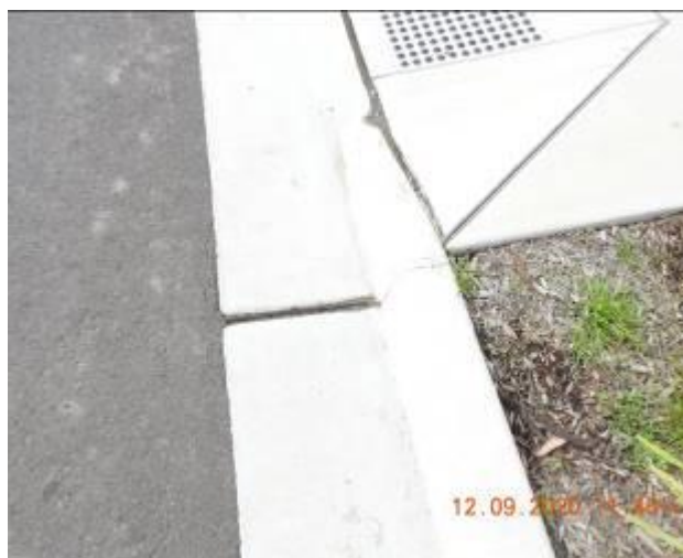
Figure 1373 – Crack propagation and loss of material through kerb and gutter
