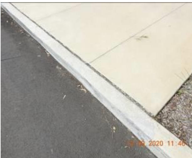
Figure 1363 – Evidence of patchwork through kerb
