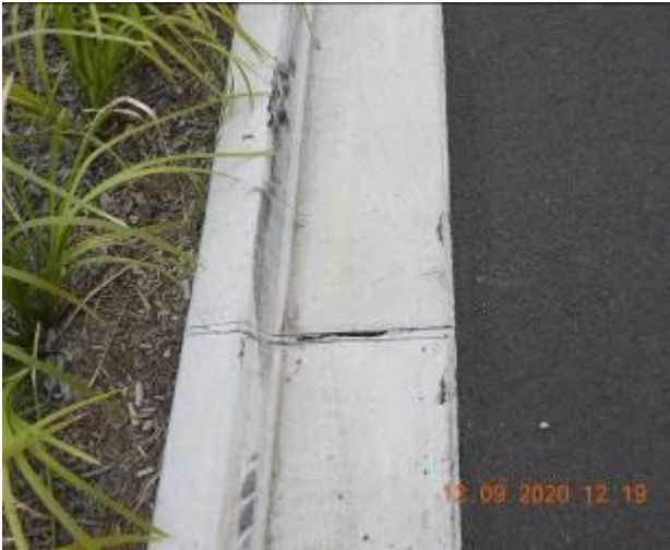
Figure 972 – Crack propagation and loss of material through kerb and gutter
