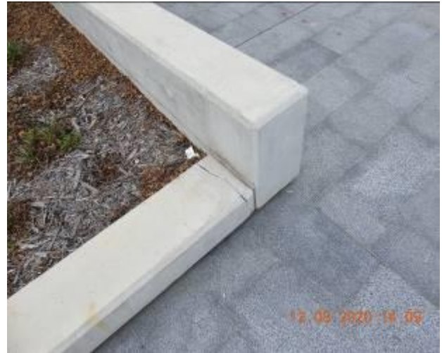
Figure 2262 – Crack propagation and loss of material through retaining wall
