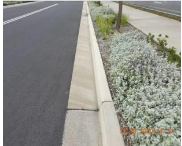
Figure 1240 – General condition of kerb and gutter
