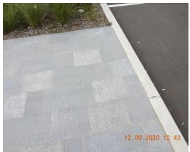
Figure 48 – Hairline cracking and efflorescence through footpath pavement
