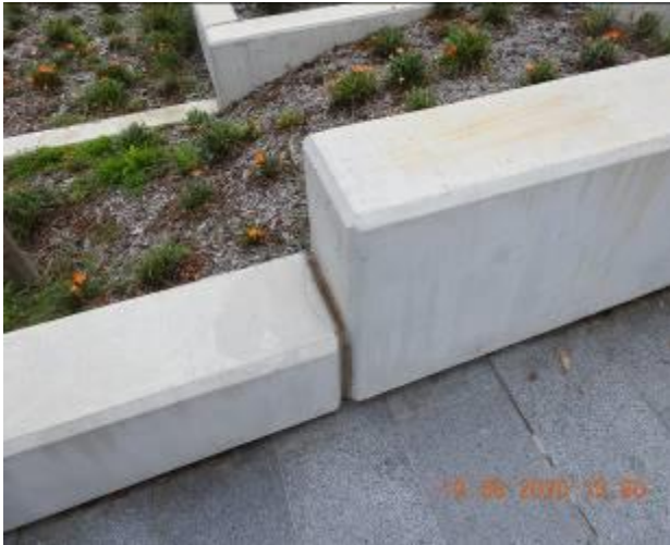
Figure 2105 – Crack propagation through retaining wall
