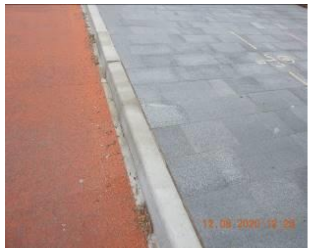
Figure 578 – Evidence of patchwork, crack propagation and loss of material through kerb
