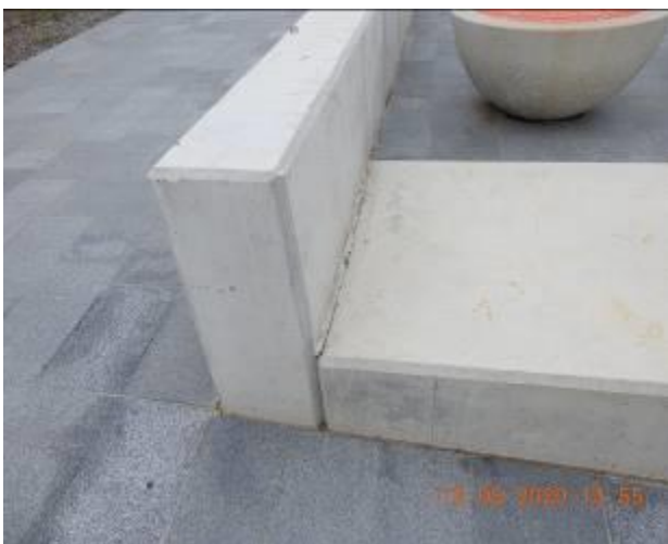
Figure 2127 – Crack propagation and loss of material through retaining wall
