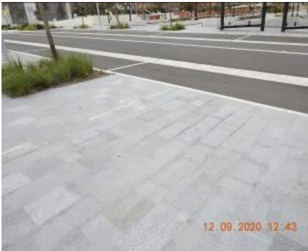
Figure 45 – Hairline cracking and efflorescence through footpath pavement
