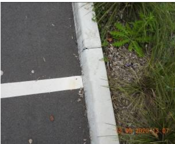
Figure 401 – Crack propagation through kerb
