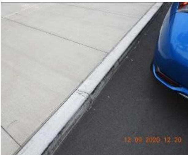
Figure 980 – Crack propagation and loss of material through kerb
