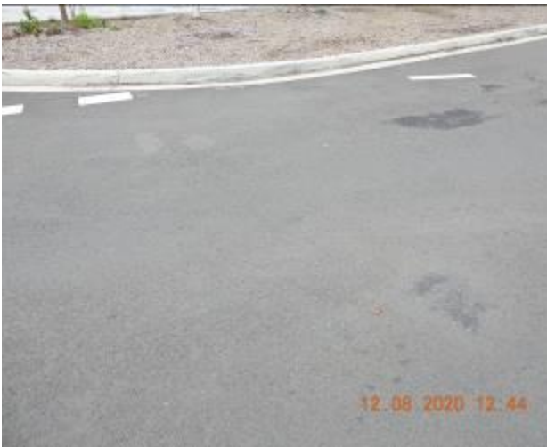
Figure 673 – Evidence of patchwork through road surface
