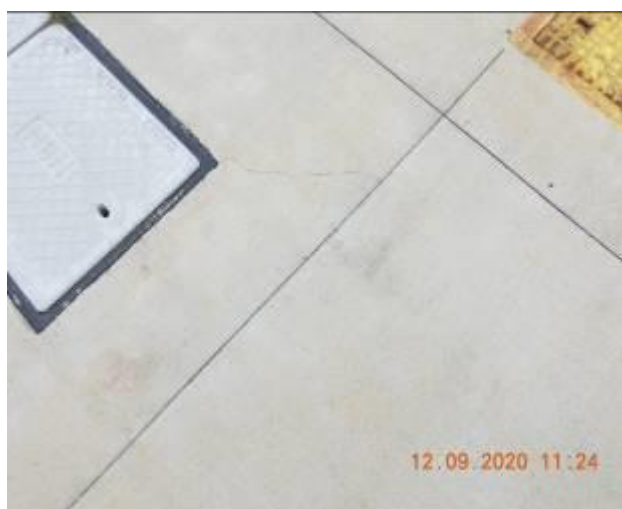
Figure 1087 – Crack propagation and loss of material through footpath pavement
