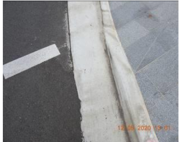
Figure 846 – Evidence of patchwork and loss of material through gutter
