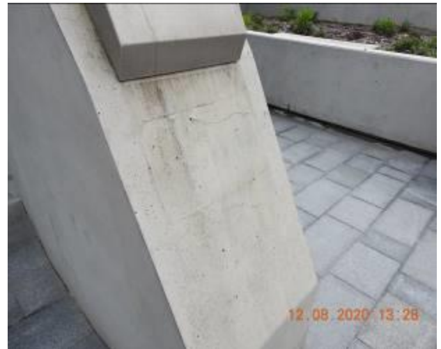
Figure 1987 – Crack propagation and loss of material through external wall
