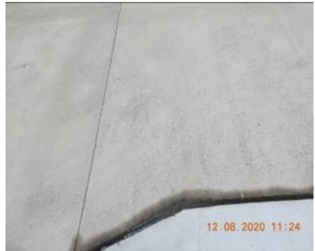
Figure 1538 – Crack propagation and loss of material through driveway pavement
