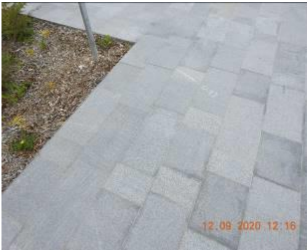
Figure 926 – Hairline crack propagation through footpath pavement
