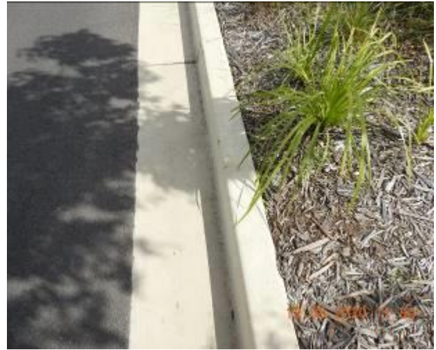
Figure 1710 – Loss of material through kerb and gutter
