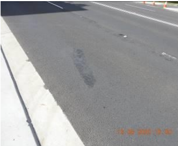
Figure 1819 – Evidence of patchwork through road surface
