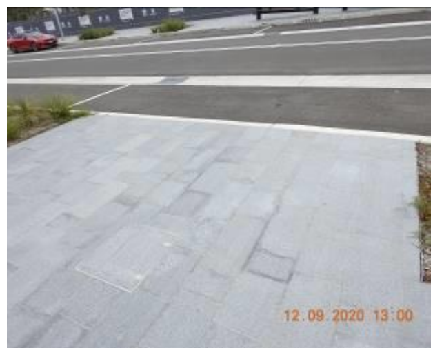
Figure 270 – Hairline cracking and efflorescence through footpath pavement
