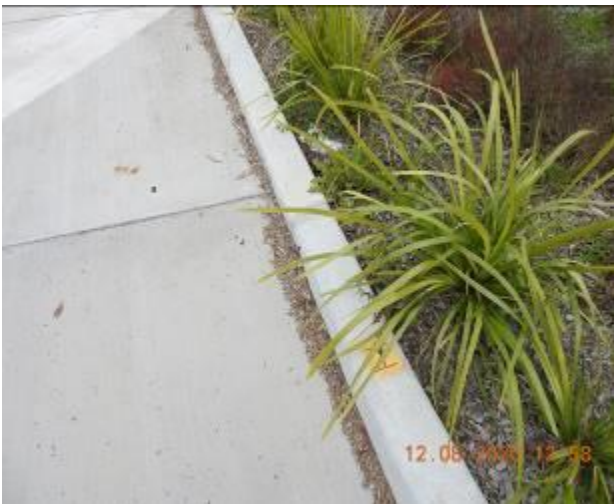
Figure 787 – Evidence of patchwork crack propagation and loss of material through kerb
