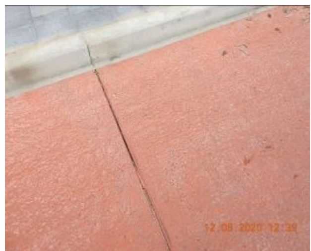
Figure 616 – Crack propagation and loss of material through road surface
