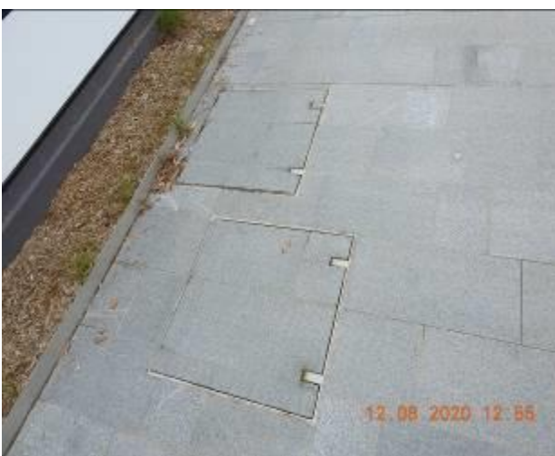
Figure 753 – Loss of material through service pit pavement
