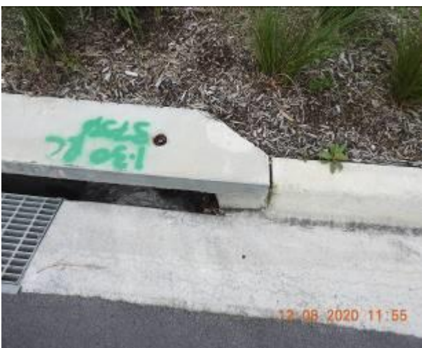
Figure 1767 – Loss of material through kerb
