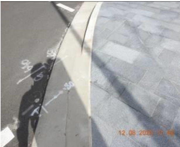
Figure 1693 – Crack propagation through layback and gutter
