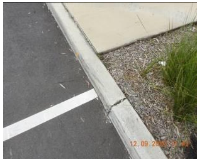
Figure 1340 – Loss of material through kerb
