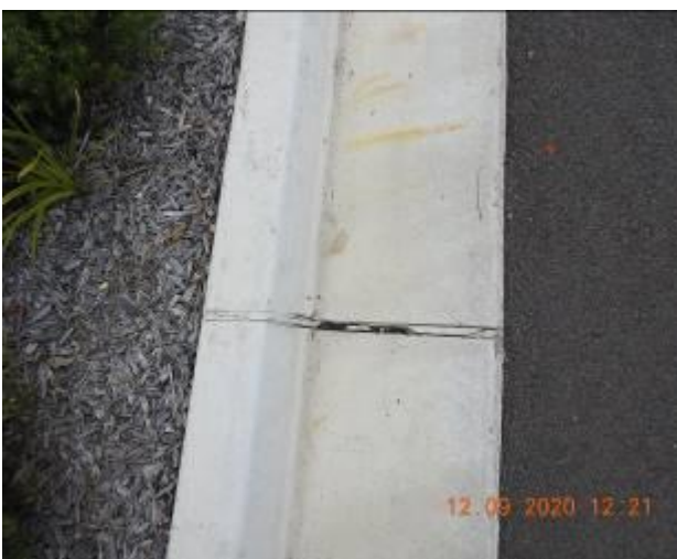
Figure 1000 – Crack propagation and loss of material through kerb and gutter
