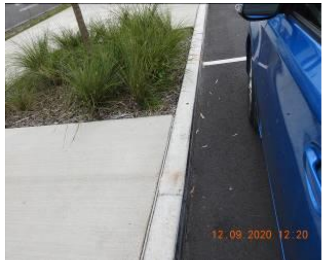
Figure 981 – Evidence of patchwork and Loss of material through kerb
