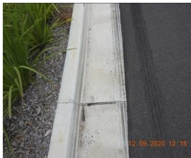
Figure 945 – Crack propagation and loss of material through kerb and gutter
