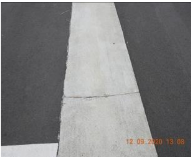
Figure 423 – Loss of material through gutter
