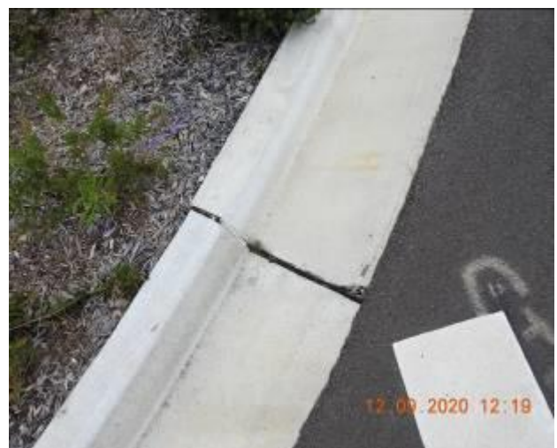
Figure 959 – Crack propagation and loss of material through kerb and gutter
