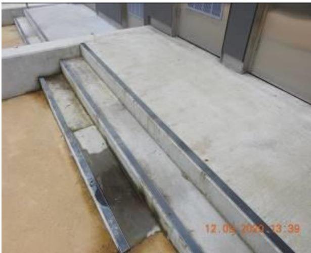
Figure 2404 – Loss of material through steps pavement
