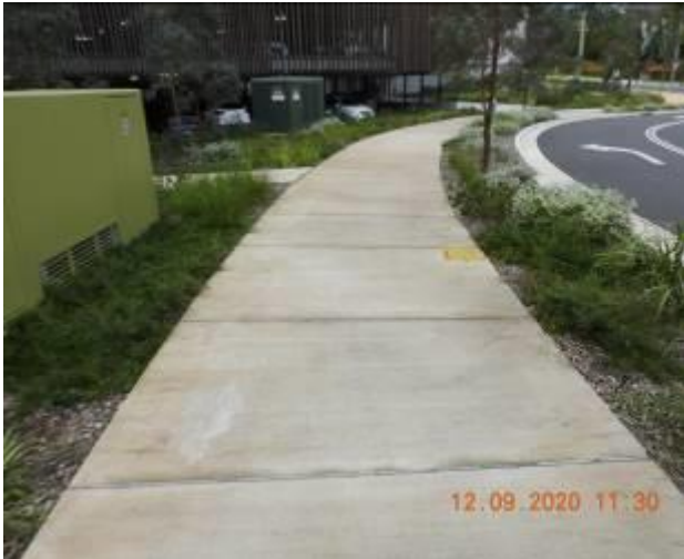
Figure 1143 – Loss of material through footpath pavement
