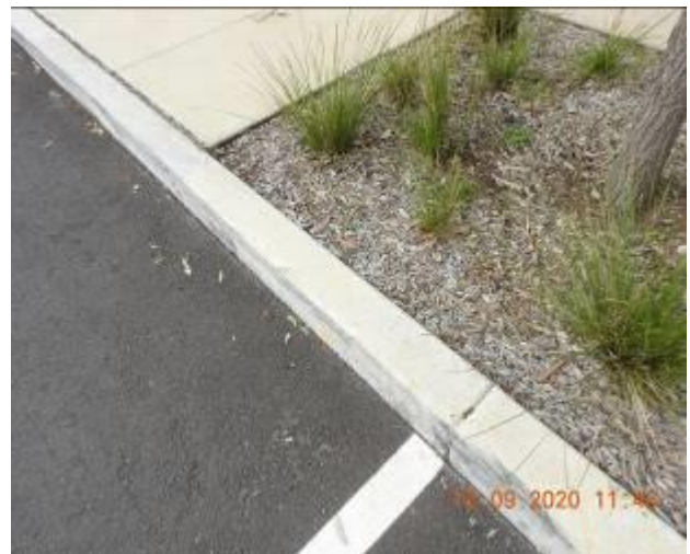
Figure 1362 – Loss of material through kerb
