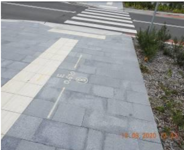
Figure 505 – Hairline crack propagation and loss of material through
