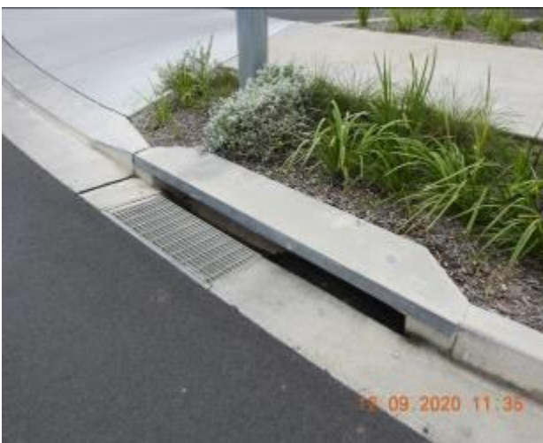
Figure 1213 – General condition of stormwater inlet pit/ Loss of material through kerb and gutter
