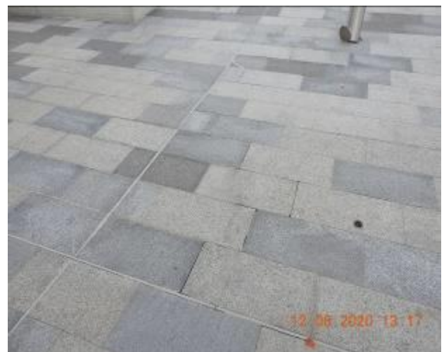
Figure 1923 – Crack propagation and loss of material through floor tiles
