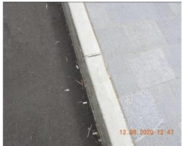
Figure 132 – Crack propagation through kerb
