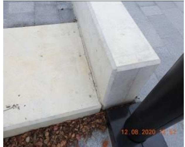
Figure 2118 – Crack propagation and loss of material through retaining wall
