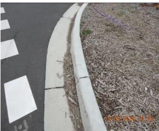
Figure 549 – Loss of material through kerb and gutter
