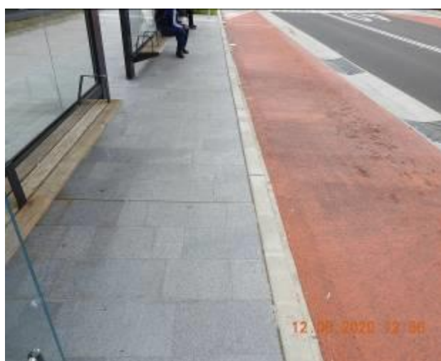
Figure 765 – Efflorescence and hairline crack propagation through footpath pavement
