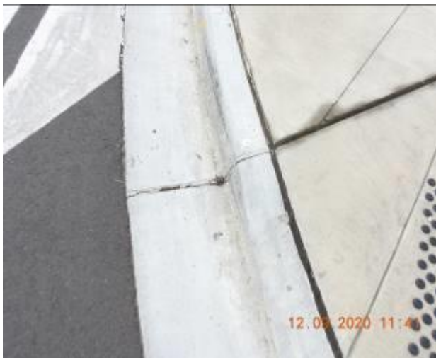
Figure 1301 – Crack propagation and loss of material through kerb and gutter
