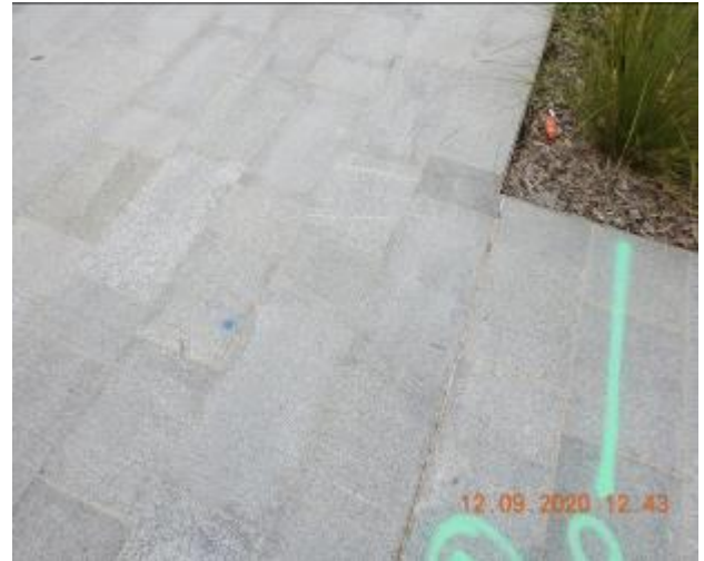
Figure 44 – Hairline cracking and efflorescence through footpath pavement
