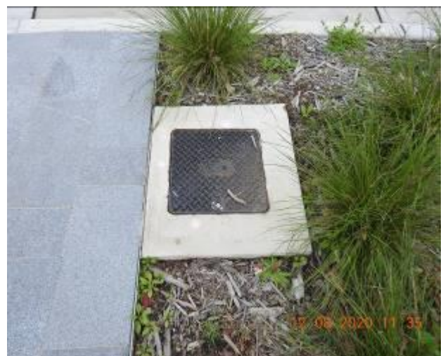
Figure 1630 – Loss of material through service pit pavement
