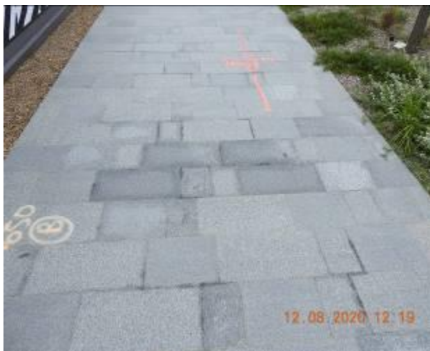
Figure 475 – Loss of material through footpath pavement
