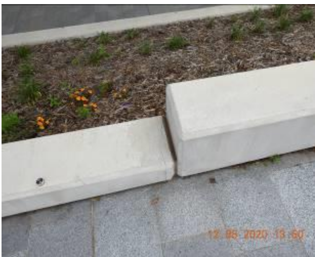
Figure 2096 – Crack propagation through retaining wall
