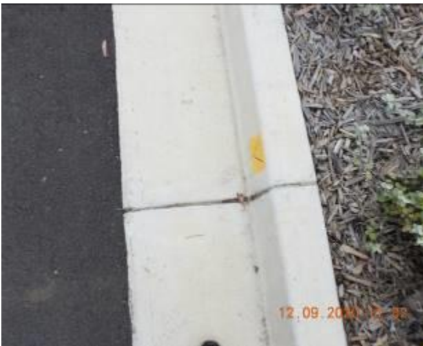
Figure 1169 – Crack propagation and loss of material through kerbs and gutter
