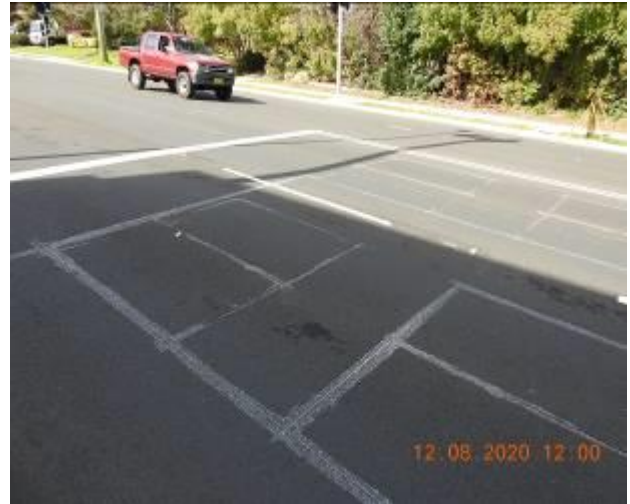
Figure 1824 – Loss of material and evidence of patchwork through road surface
