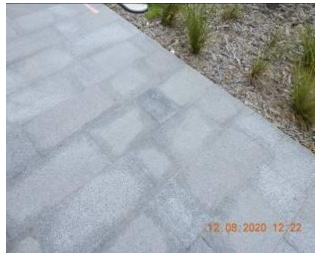
Figure 500 – Loss of material through footpath pavement
