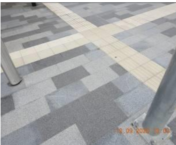
Figure 335 – Hairline cracking and efflorescence through footpath pavement
