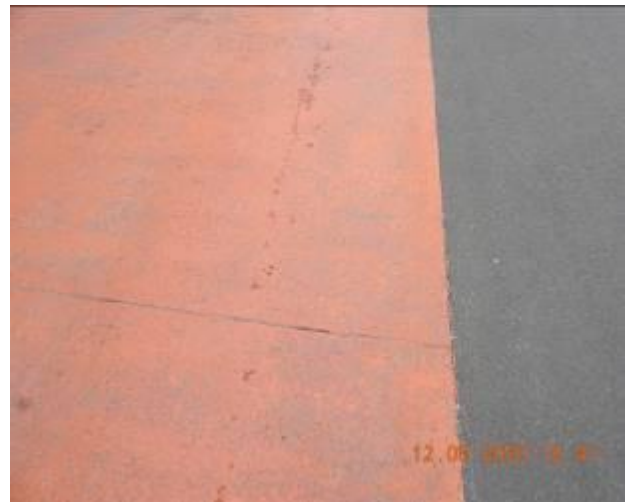
Figure 638 – Crack propagation and loss of material through road surface
