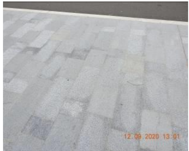
Figure 286 – Hairline cracking and efflorescence through footpath pavement
