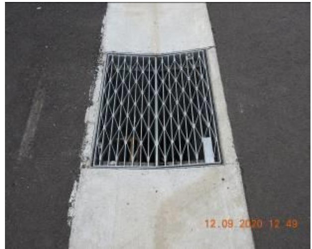
Figure 124 – General condition of stormwater inlet pit and Crack propagation through gutter
