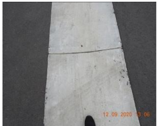
Figure 396 – Crack propagation through gutter
