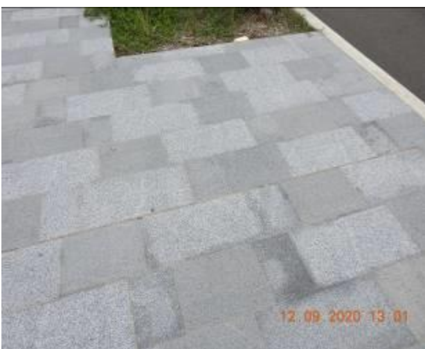
Figure 287 – Hairline cracking and efflorescence through footpath pavement
