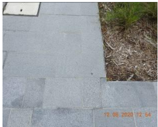
Figure 742 – Loss of material through footpath pavement
