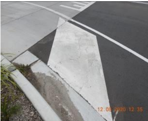
Figure 601 – Crack propagation and loss of material through road surface
