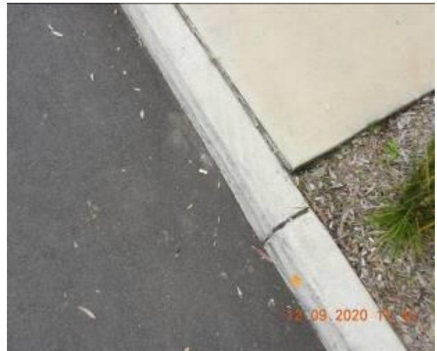
Figure 1338 – Loss of material through kerb
