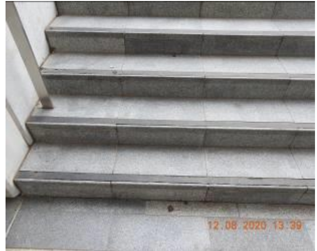
Figure 2081 – Separation through staircase pavement
