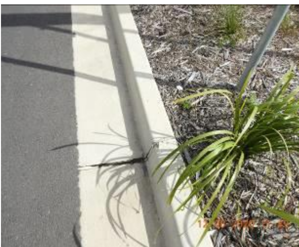
Figure 1701 – Loss of material through kerb and gutter
