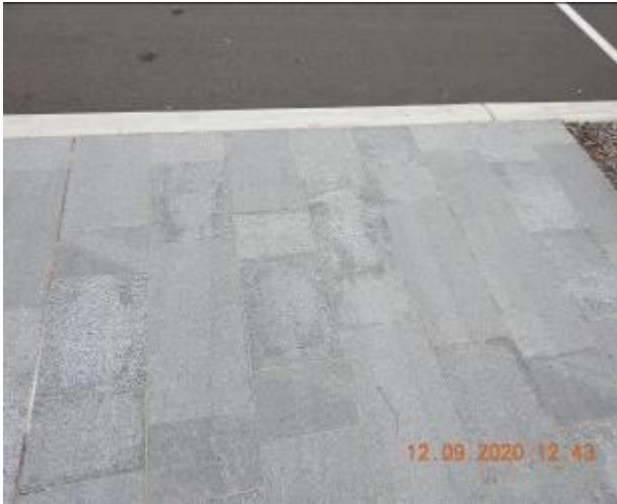
Figure 37 – Hairline cracking and efflorescence through footpath pavement
