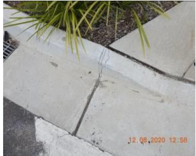
Figure 786 – Crack propagation and loss of material through kerb and gutter
