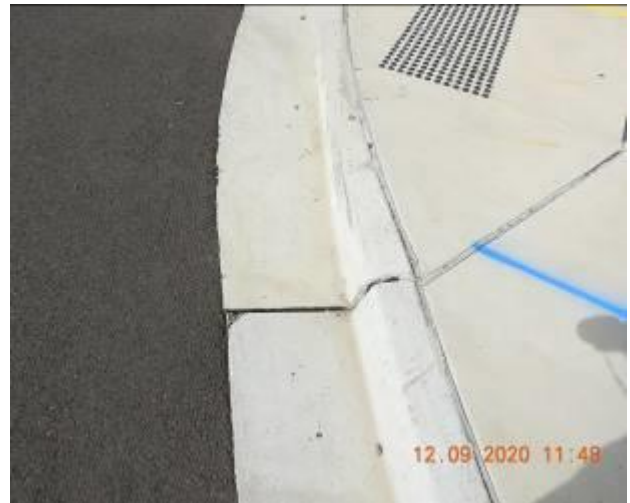
Figure 1380 – Crack propagation and loss of material through kerb and gutter
