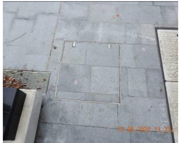
Figure 1616 – Loss of material through service pit
