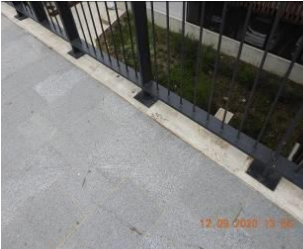
Figure 2528 – Evidence of patchwork through boundary wall
