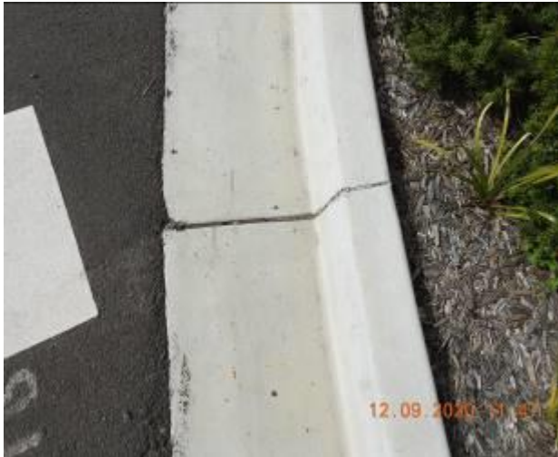
Figure 1377 – Crack propagation and loss of material through kerb and gutter
