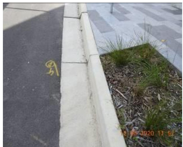
Figure 1744 – Evidence of patchwork through kerb
