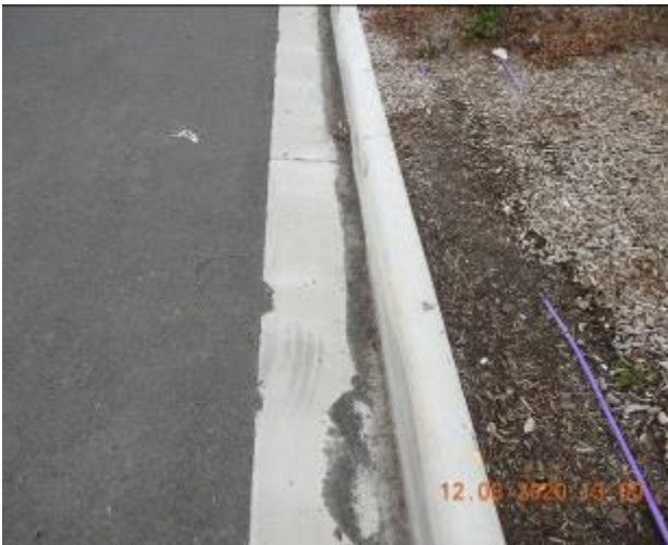
Figure 823 – Loss of material through gutter
