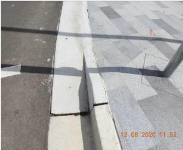
Figure 1747 – Crack propagation and loss of material through kerb and gutter
