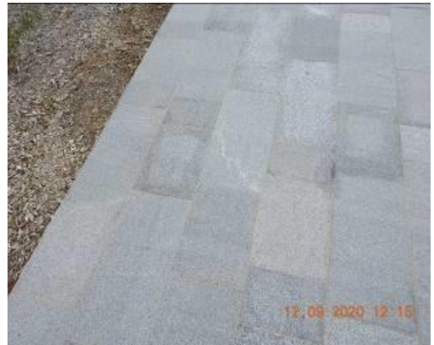
Figure 909 – Crack propagation and loss of material through footpath pavement
