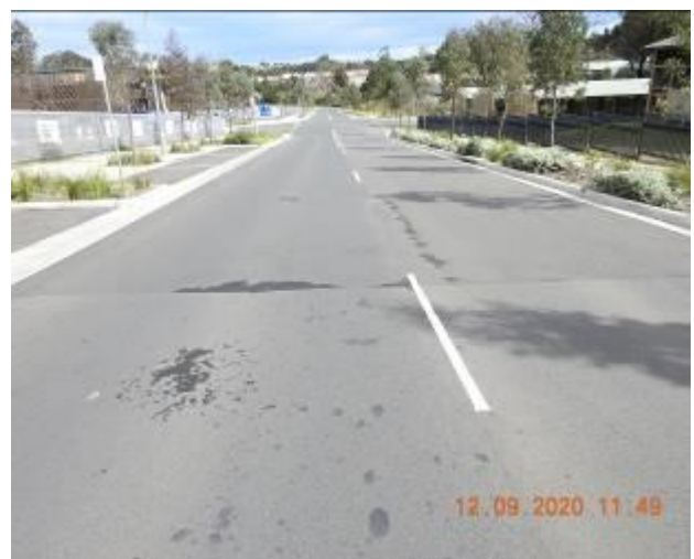
Figure 1394 – Evidence of patchwork through road surface
