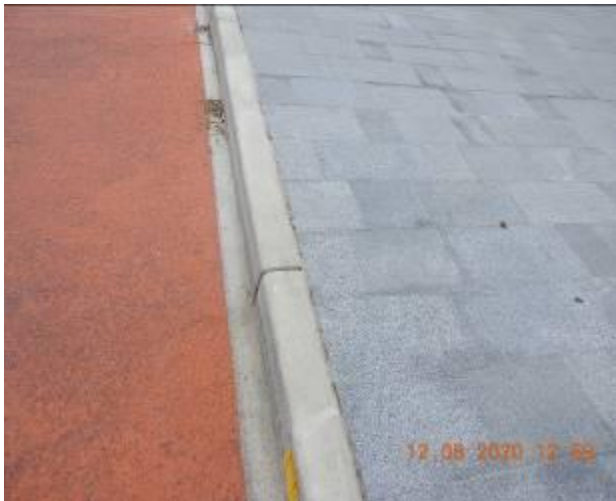
Figure 803 – Evidence of patchwork, hairline crack propagation and loss of material through kerb
