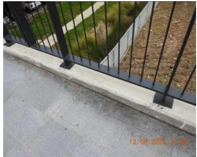
Figure 2519 – Crack propagation and loss of material through boundary wall
