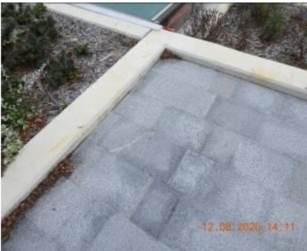
Figure 2275 – Efflorescence and crack propagation through walkway floor and retaining wall
