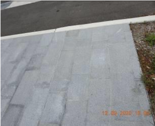
Figure 271 – Hairline cracking and efflorescence through footpath pavement
