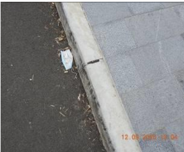
Figure 363 – Crack propagation and loss of material through kerb
