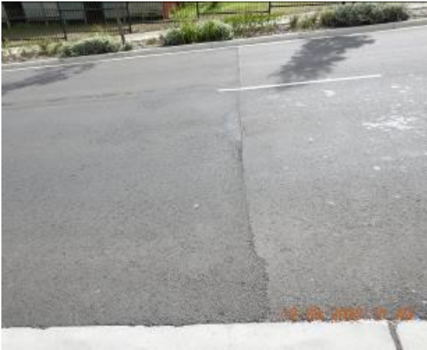
Figure 1395 – Loss of material and evidence of patchwork through road surface
