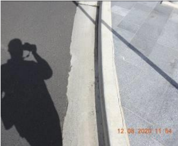
Figure 1757 – Loss of material through kerb and gutter
