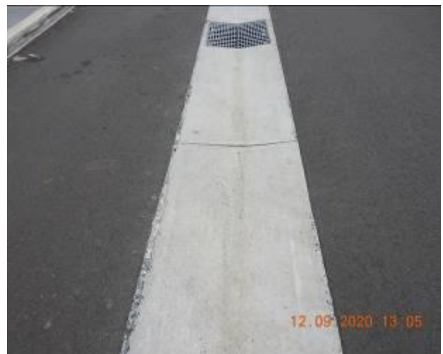
Figure 378 – Crack propagation and loss of material through gutter
