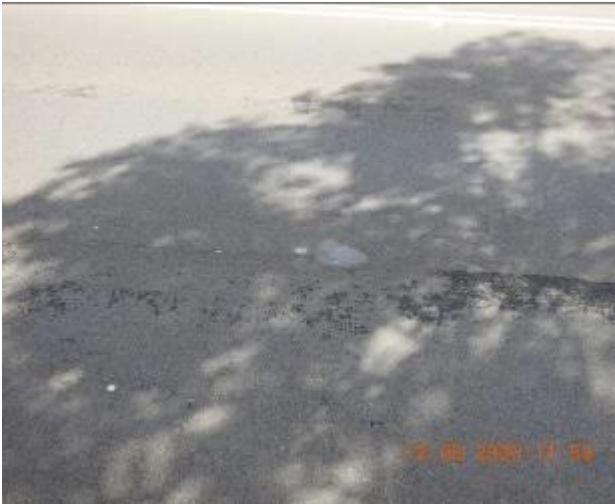
Figure 1817 – Evidence of patchwork through road surface
