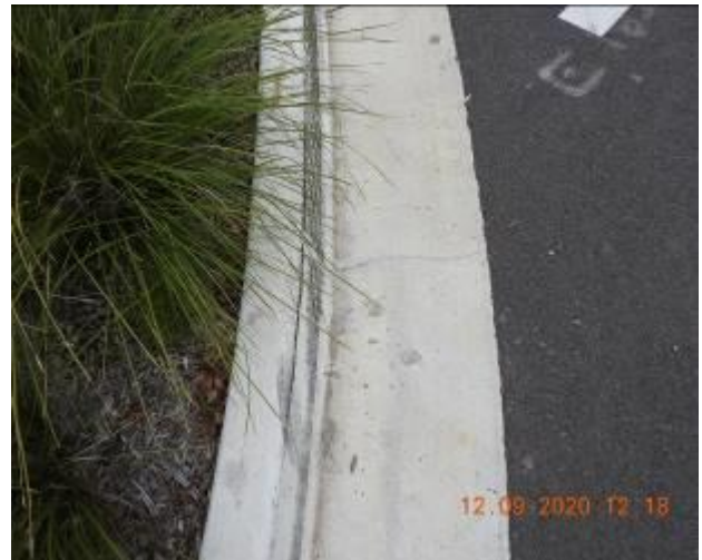
Figure 957 – Crack propagation and loss of material through kerb and gutter
