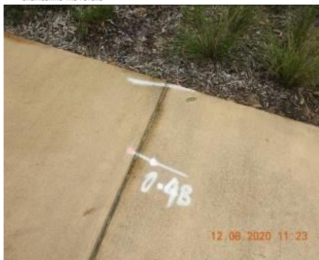
Figure 1529 – Loss of material through footpath pavement
