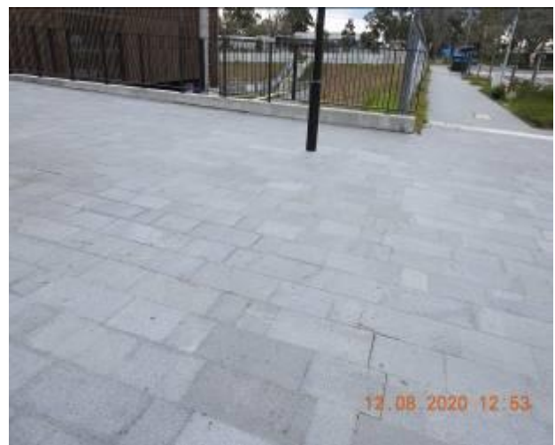
Figure 730 – Efflorescence, hairline crack propagation and loss of material through footpath pavement
