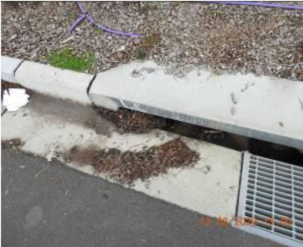
Figure 827 – Loss of material through kerb
