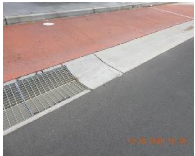
Figure 620 – Crack propagation and loss of material through road surface
