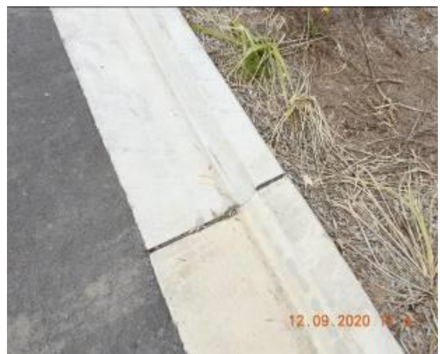
Figure 1310 – Loss of material through kerb and gutter
