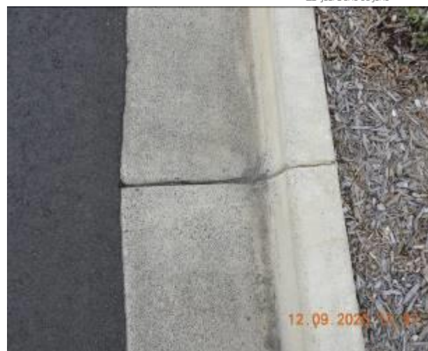
Figure 1234 – Crack propagation and loss of material through kerb and gutter
