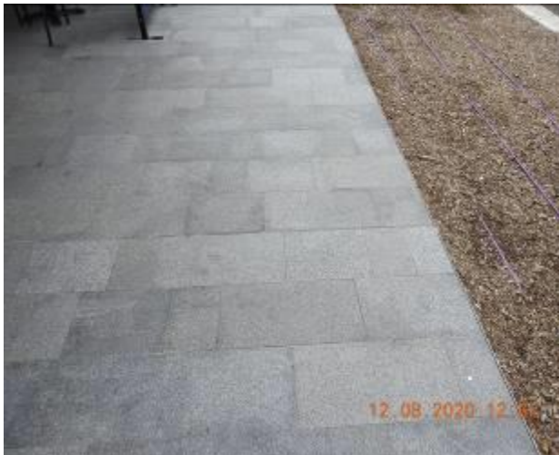
Figure 713 – Efflorescence, crack propagation and loss of material through footpath pavement
