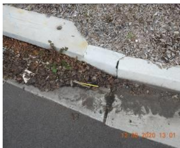
Figure 842 – Crack propagation and loss of material through kerb and gutter
