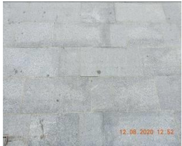
Figure 722 – Efflorescence, hairline crack propagation and loss of material through footpath pavement
