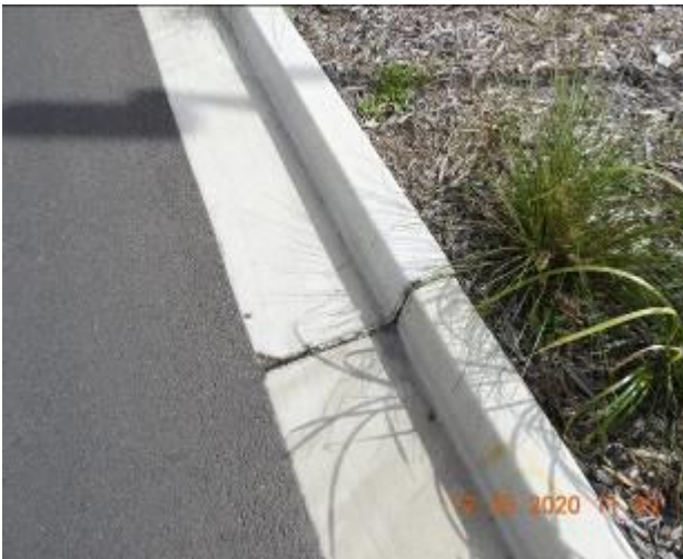
Figure 1699 – Loss of material through kerb and gutter
