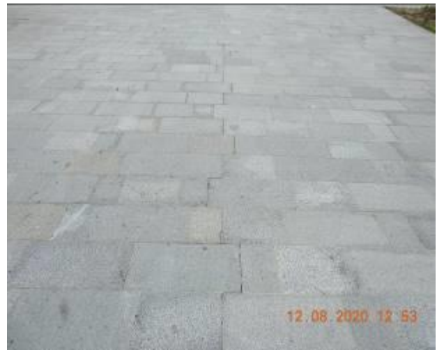
Figure 728 – Efflorescence, hairline crack propagation and loss of material through footpath pavement
