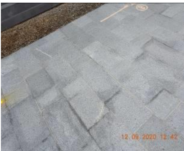
Figure 23 – Hairline cracking and efflorescence through footpath pavement
