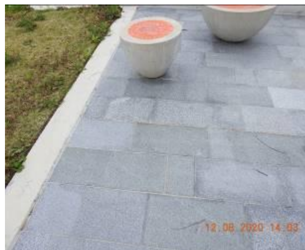
Figure 2186 – Hairline crack propagation through walkway floor
