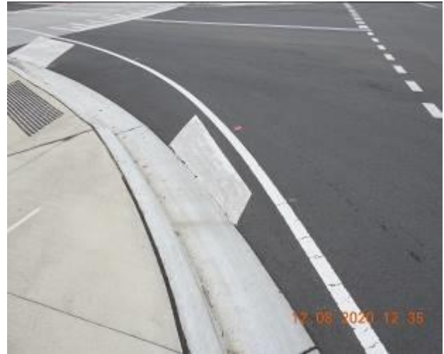
Figure 600 – Crack propagation and loss of material through road surface
