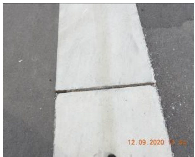
Figure 1352 – Loss of material through gutter
