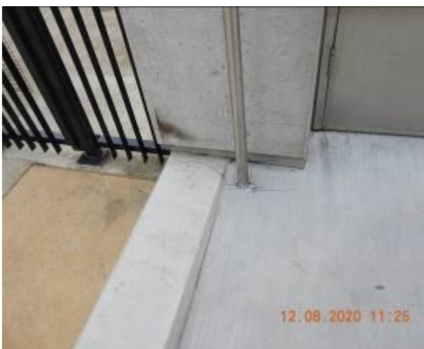
Figure 1551 – Crack propagation and loss of material through steps pavement
