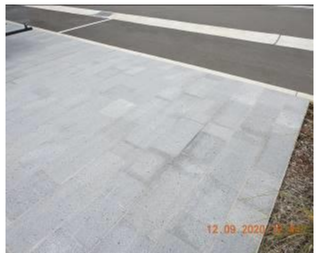
Figure 66 – Hairline cracking and efflorescence through footpath pavement
