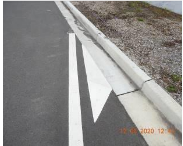
Figure 666 – Crack propagation and loss of material through road surface
