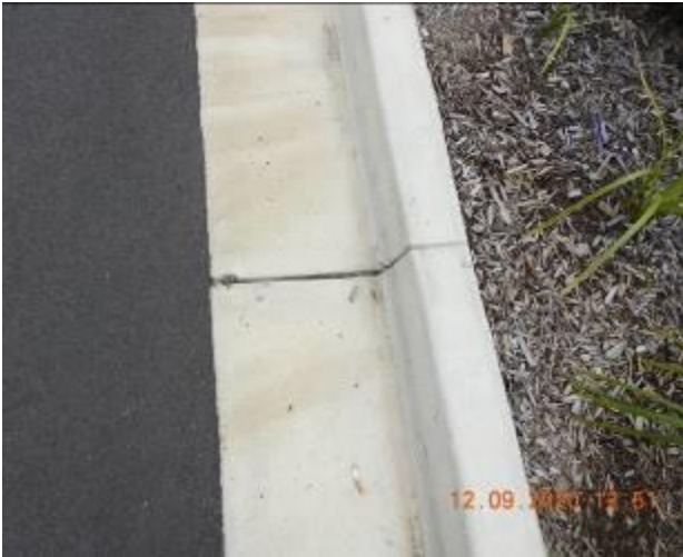
Figure 175 – Loss of material through gutter
