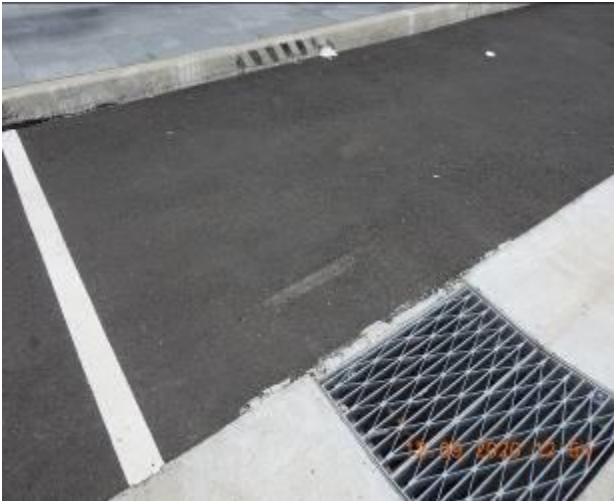
Figure 217 – Loss of material through road surface
