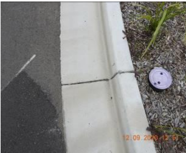
Figure 183 – Crack propagation through kerb
