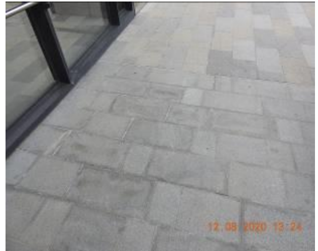
Figure 1969 – Efflorescence and loss of material through floor tiles
