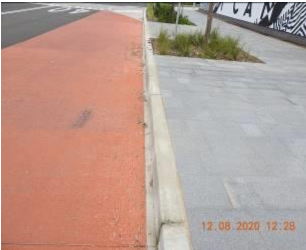
Figure 583 – Evidence of patchwork and hairline crack propagation through kerb
