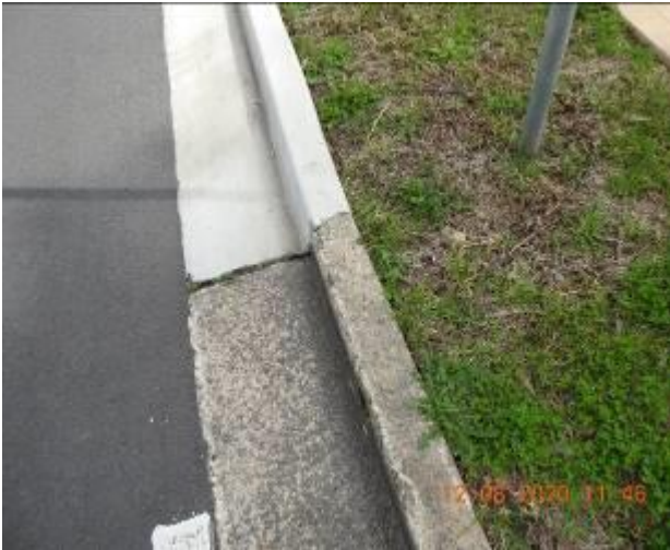
Figure 1673 – Loss of material through kerb and gutter
