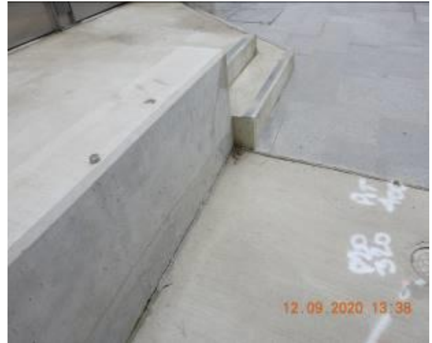
Figure 2397 – Crack propagation and loss of material through retaining wall
