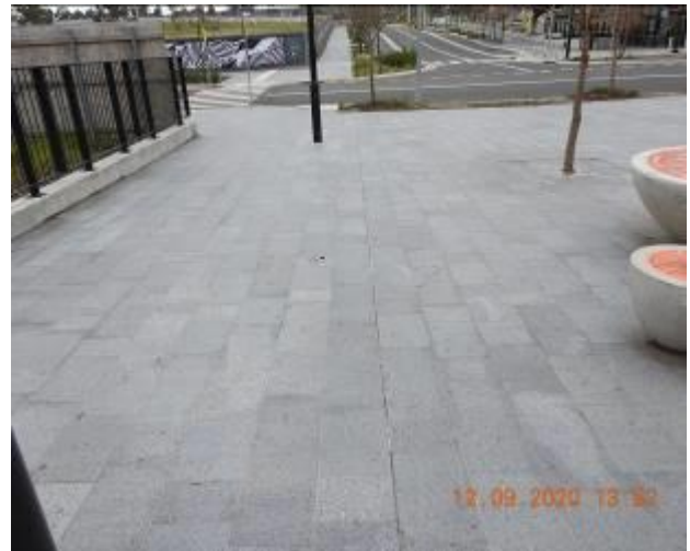
Figure 2453 – Hairline crack propagation through walkway floor
