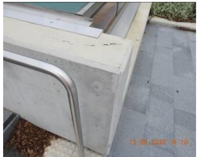
Figure 2272 – Crack propagation and loss of material through retaining wall
