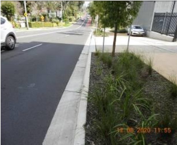
Figure 1769 – General condition of kerb and gutter
