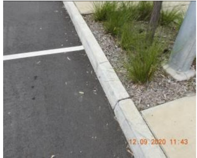
Figure 1342 – Loss of material through kerb
