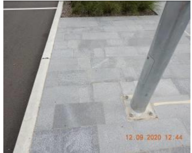
Figure 56 – Hairline cracking and efflorescence through footpath pavement
