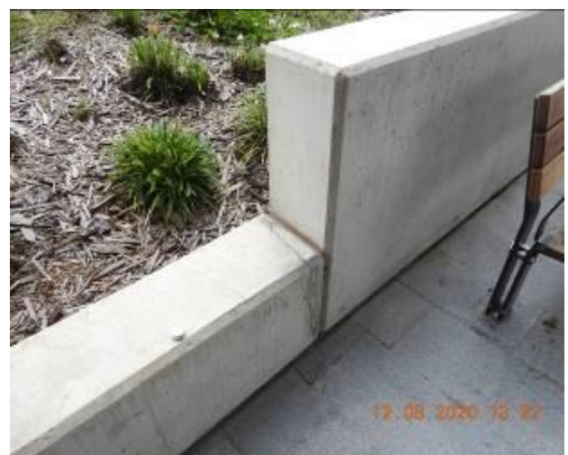
Figure 1953 – Crack propagation and loss of material through retaining wall
