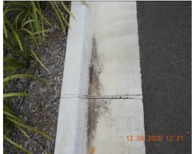
Figure 1003 – Crack propagation and loss of material through kerb and gutter
