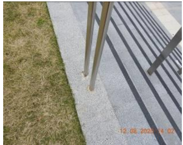
Figure 2174 – Loss of material through retaining
