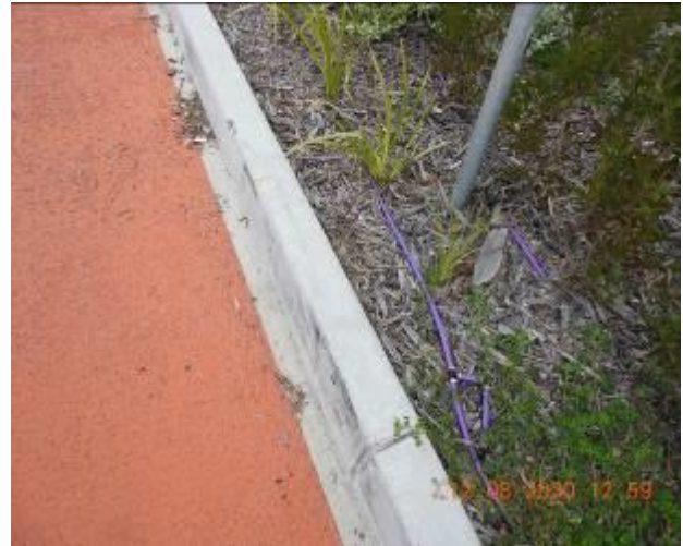
Figure 810 – Evidence of patchwork, crack propagation and loss of material through kerb
