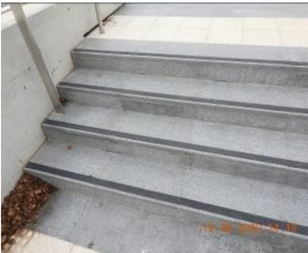
Figure 2269 – Loss of material through staircase floor
