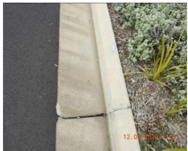
Figure 1244 – Crack propagation and loss of material through kerb and gutter
