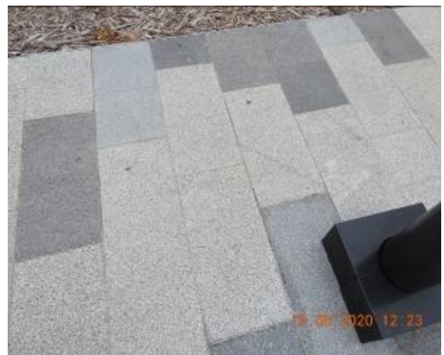
Figure 524 – Loss of material through footpath pavement
