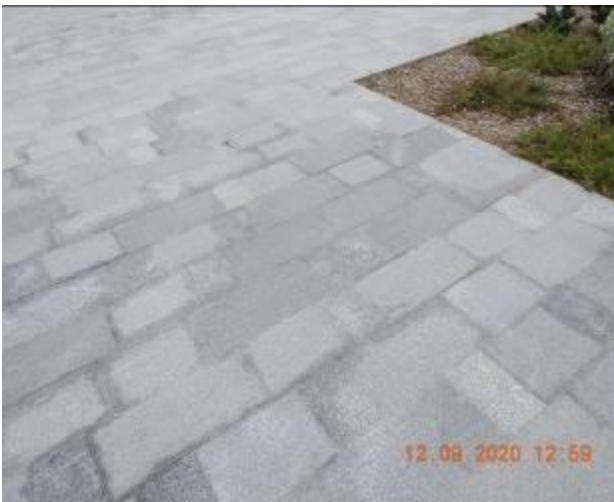
Figure 255 – Hairline cracking and efflorescence through footpath pavement
