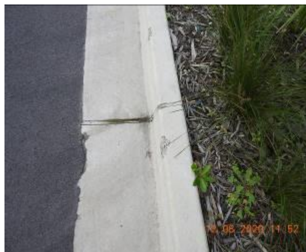
Figure 1736 – Crack propagation and loss of material through kerb and gutter
