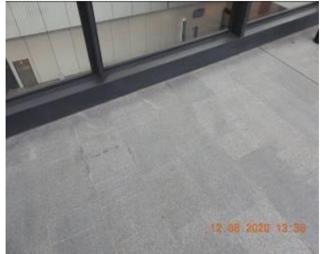
Figure 2075 – Hairline crack propagation through floor tiles
