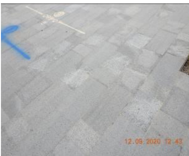
Figure 35 – Hairline cracking and efflorescence through footpath pavement
