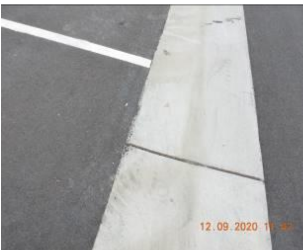
Figure 1327 – Loss of material through gutter
