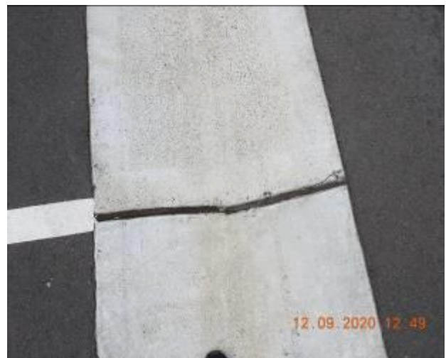
Figure 172 – Crack propagation through gutter
