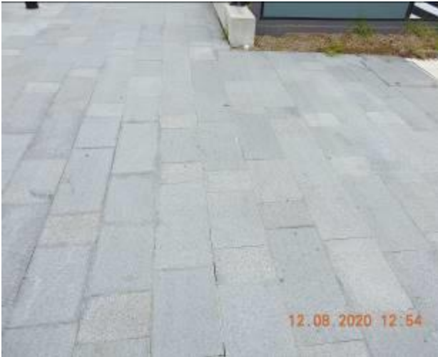
Figure 737 – Crack propagation and loss of material through footpath pavement
