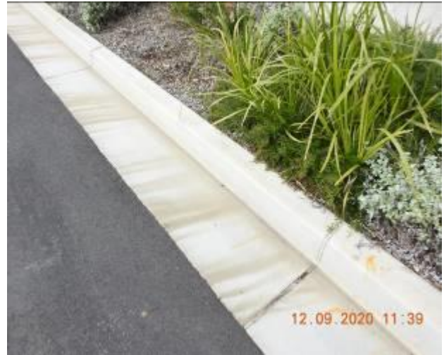
Figure 1276 – Loss of material through gutter
