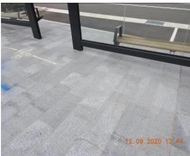
Figure 71 – Hairline cracking and efflorescence through footpath pavement
