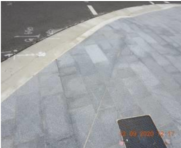
Figure 932 – Hairline crack propagation through footpath pavement
