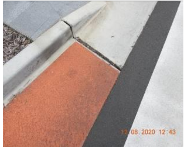
Figure 660 – Crack propagation and loss of material through road surface
