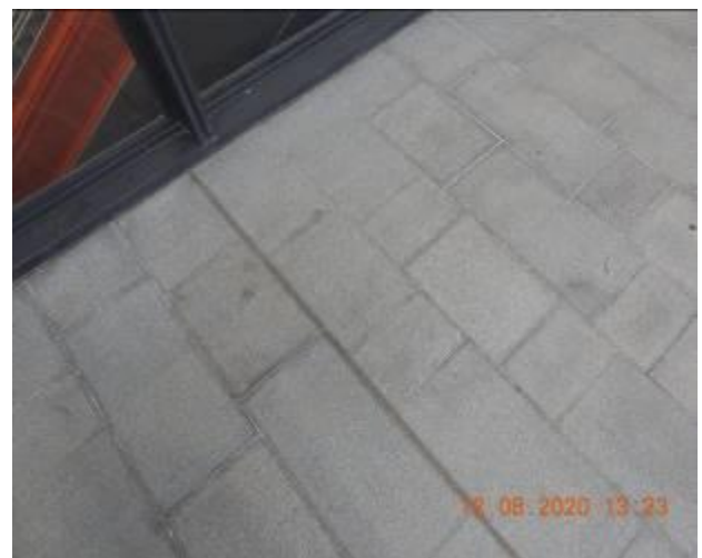
Figure 1965 – Efflorescence through floor tiles
