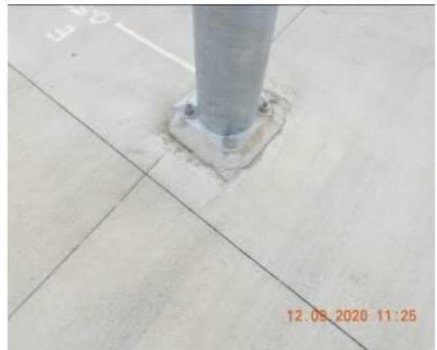
Figure 1092 – Crack propagation and loss of material through lamp post foundation
