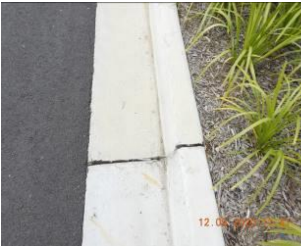
Figure 1313 – Crack propagation and loss of material through kerb and gutter
