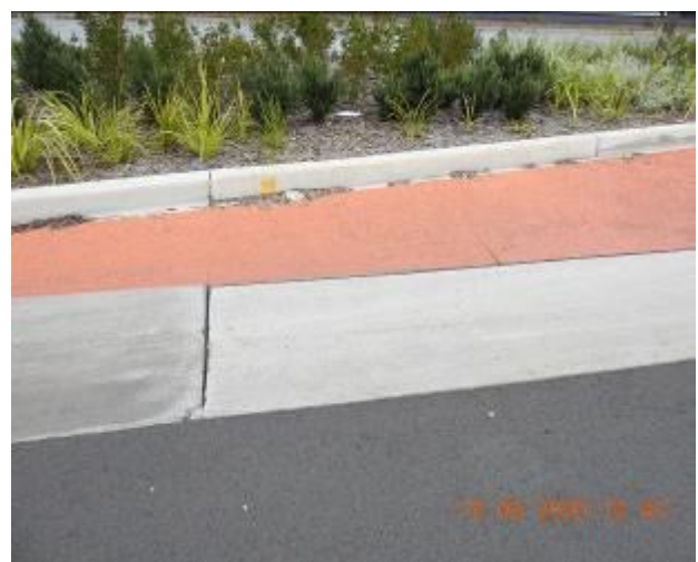
Figure 652 – Crack propagation and loss of material through road surface
