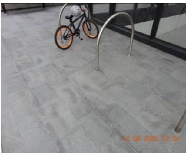
Figure 2042 – Efflorescence, crack propagation and loss of material through floor tiles
