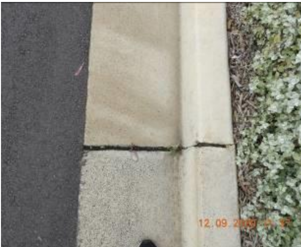
Figure 1241 – Crack propagation and loss of material through kerb and gutter
