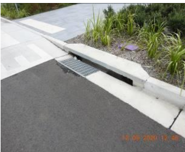
Figure 95 – General condition of kerb inlet pit
