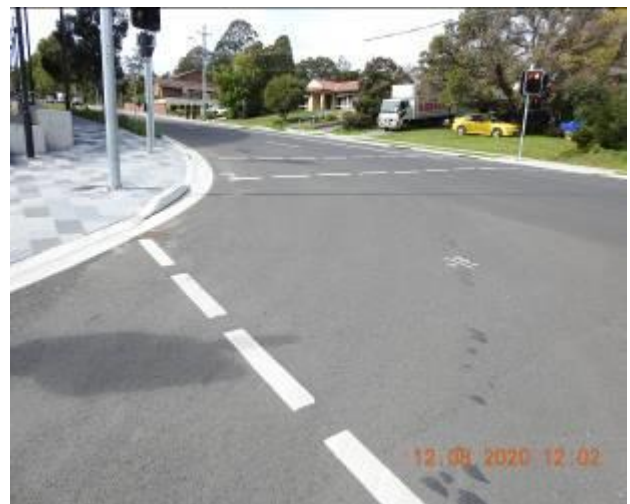
Figure 1834 – Evidence of patchwork through road surface
