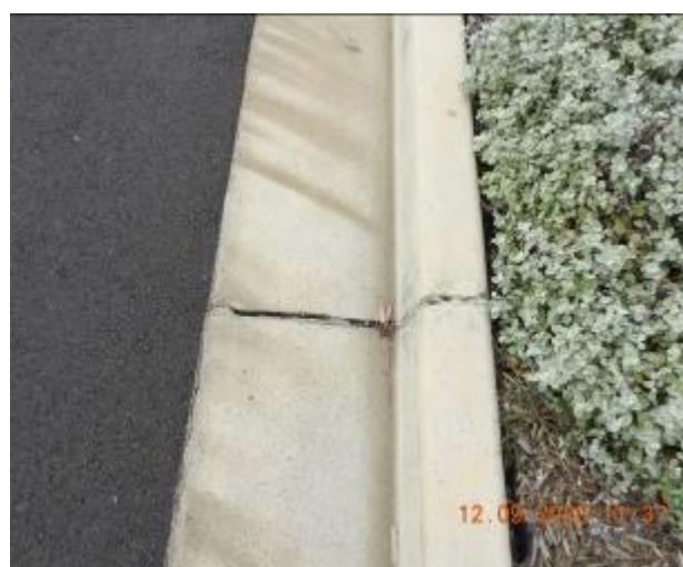
Figure 1248 – Crack propagation and loss of material through kerb and gutter
