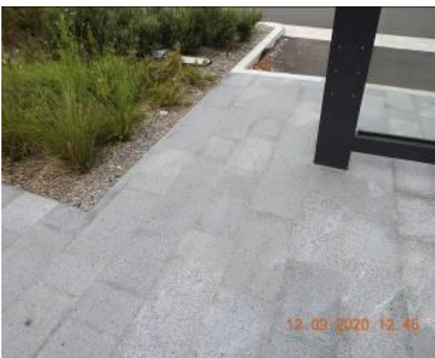
Figure 77 – Hairline cracking and efflorescence through footpath pavement
