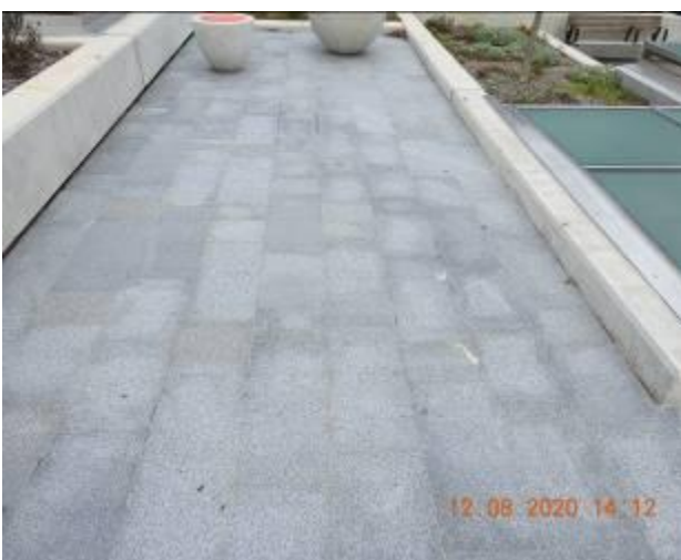
Figure 2295 – Efflorescence and crack propagation through walkway floor
