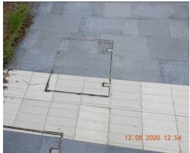
Figure 740 – Crack propagation and loss of material through service pit pavement
