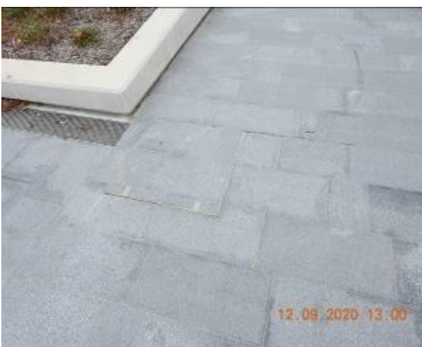
Figure 275 – Hairline cracking and efflorescence through footpath pavement
