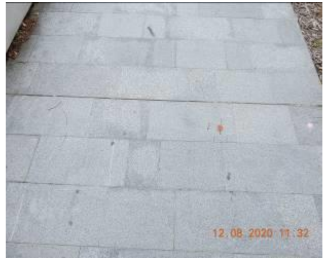
Figure 1598 – Efflorescence, hairline crack propagation and loss of material through footpath pavement
