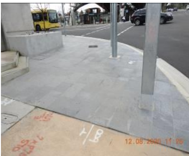
Figure 1563 – Loss of material through footpath pavement
