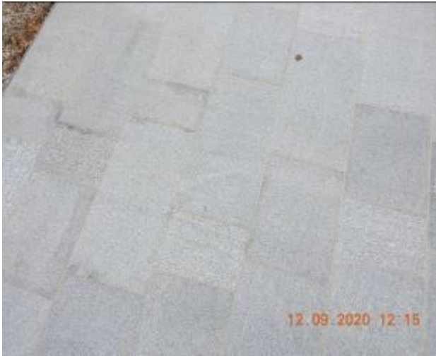
Figure 906 – Crack propagation and loss of material through footpath pavement
