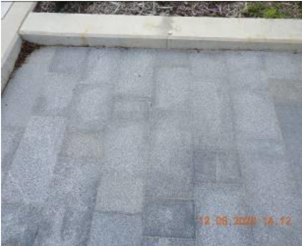
Figure 2291 – Hairline crack propagation and loss of material through walkway floor
