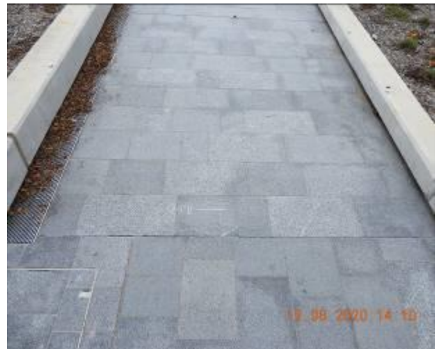
Figure 2264 – Crack propagation and loss of material through walkway floor
