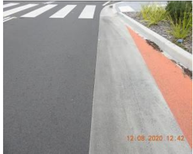
Figure 654 – Separation through road surface
