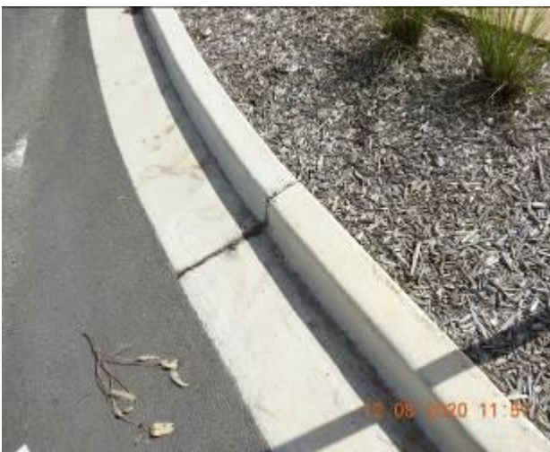
Figure 1797 – Loss of material through kerb
