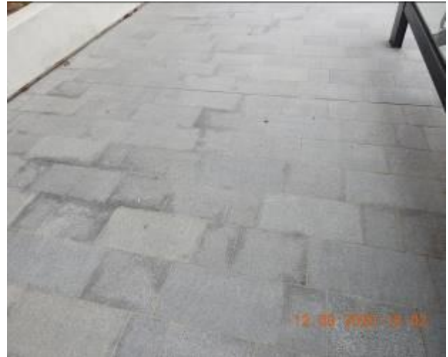
Figure 320 – Hairline cracking and efflorescence through footpath pavement
