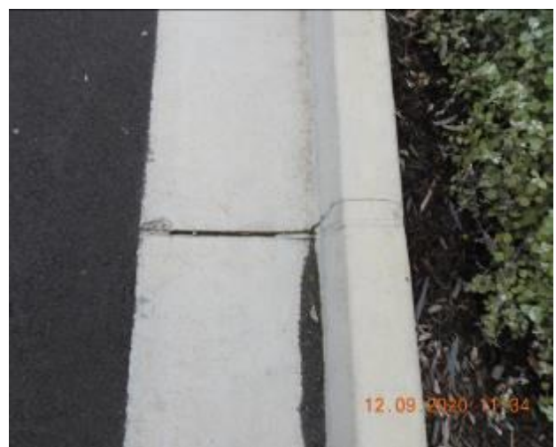
Figure 1196 – Crack propagation and loss of material through kerb and gutter
