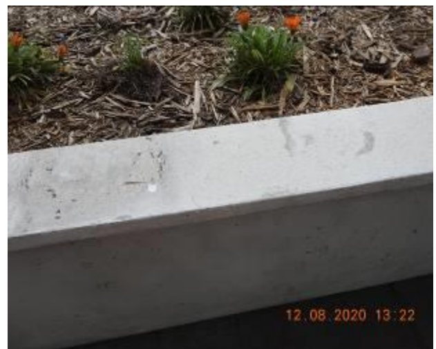
Figure 1945 – Crack propagation and loss of material through retaining wall
