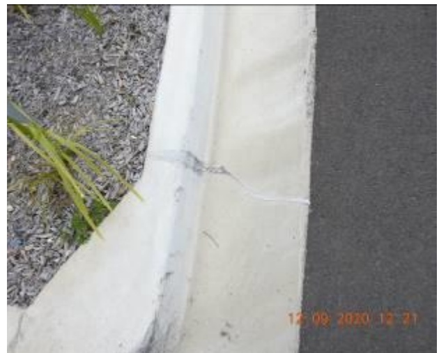
Figure 993 – Evidence of patchwork and crack propagation through kerb and gutter
