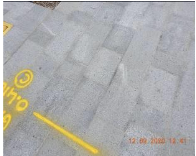
Figure 4 – Crack propagation and efflorescence through footpath pavement
