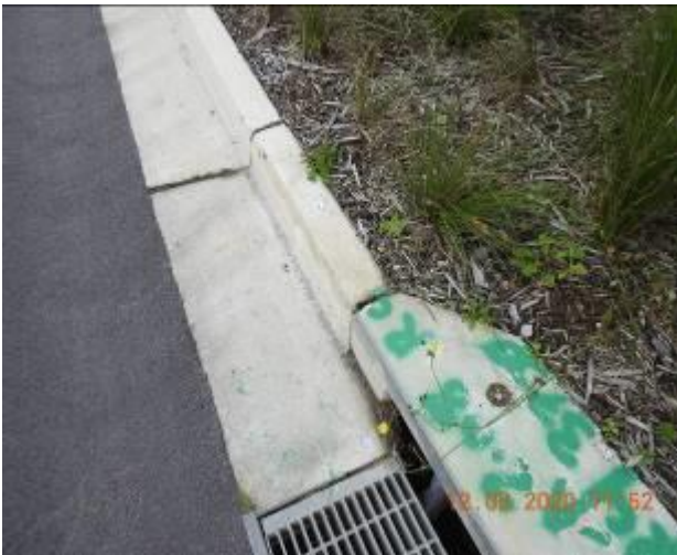
Figure 1741 – Crack propagation and loss of material through kerb
