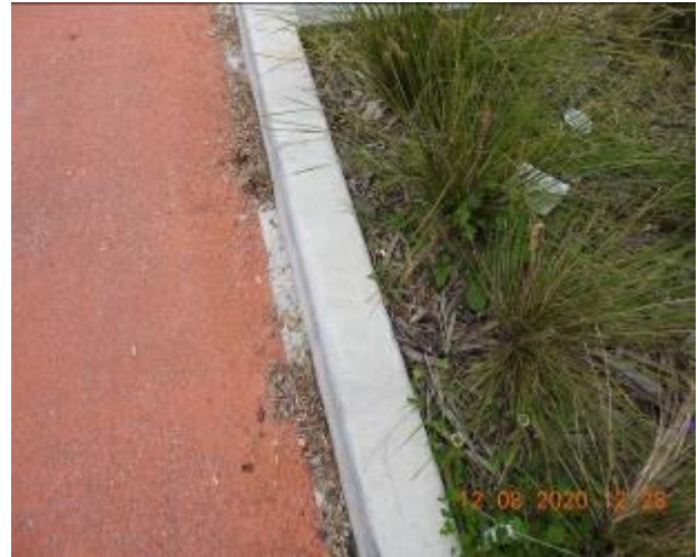
Figure 582 – Evidence of patchwork and hairline crack propagation through kerb
