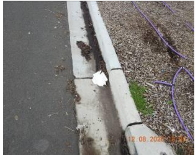
Figure 828 – Loss of material through kerb and gutter
