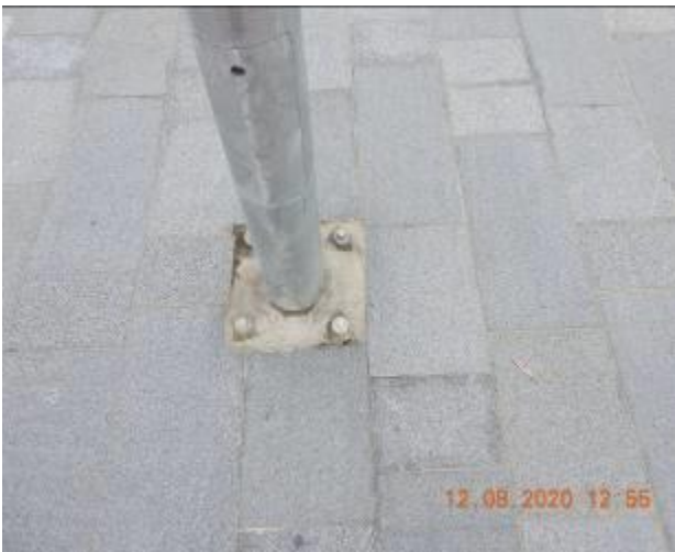
Figure 757 – Loss of material through lamp post foundation
