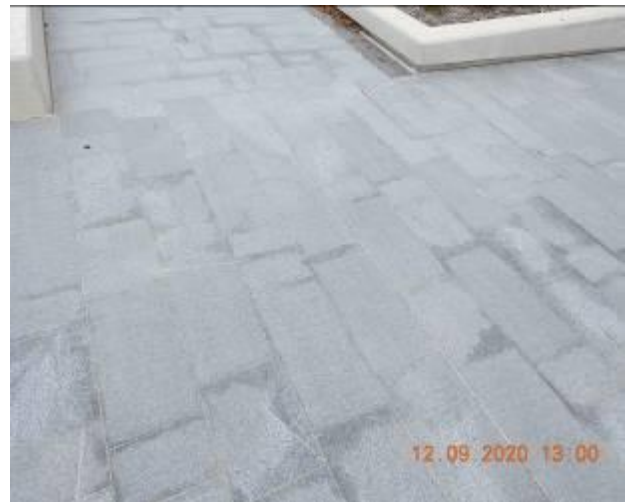
Figure 274 – Hairline cracking and efflorescence through footpath pavement
