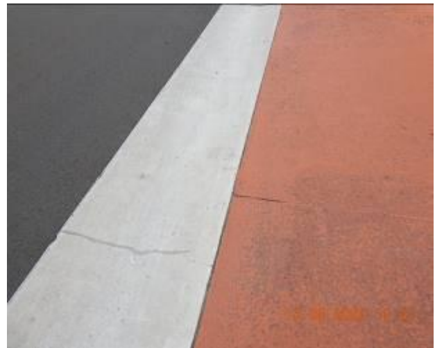
Figure 644 – Evidence of patchwork, hairline crack propagation and loss of material through road surface
