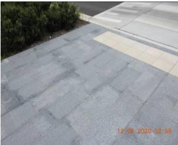
Figure 261 – Hairline cracking and efflorescence through footpath pavement
