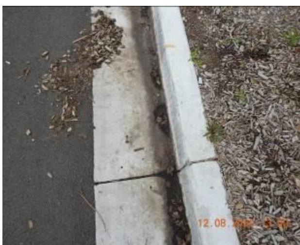
Figure 837 – Crack propagation and loss of material through kerb and gutter
