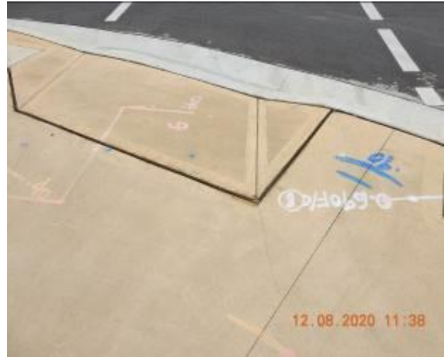
Figure 1650 – Crack propagation and loss of material through footpath pavement
