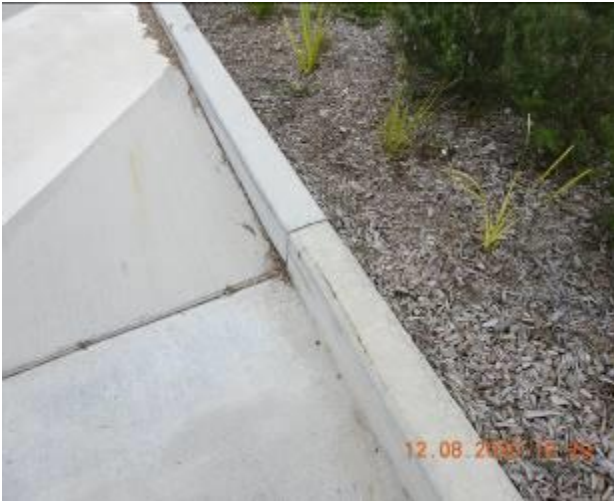
Figure 593 – Loss of material through kerb
