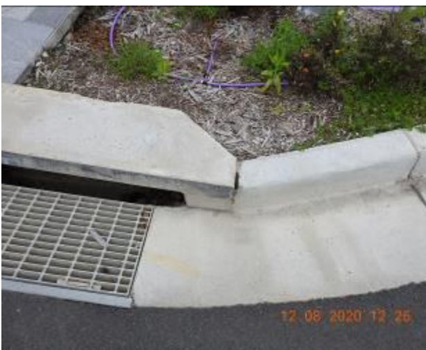
Figure 553 – Crack propagation and loss of material through kerb
