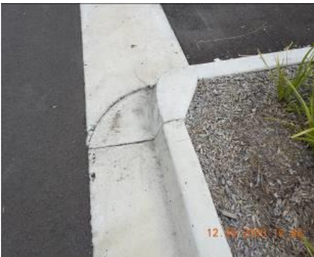
Figure 101 – Crack propagation and loss of material through kerb and gutter
