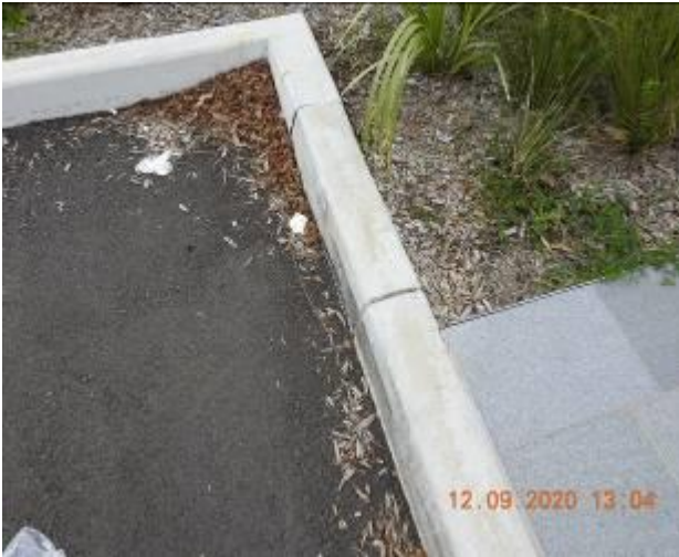
Figure 367 – Crack propagation through kerb
