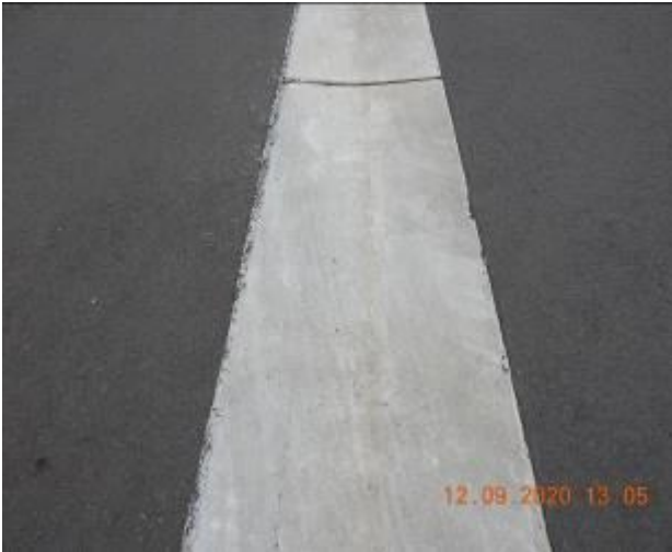
Figure 373 – Crack propagation through gutter
