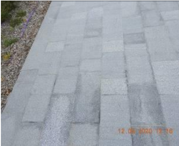
Figure 918 – Crack propagation and loss of material through footpath pavement
