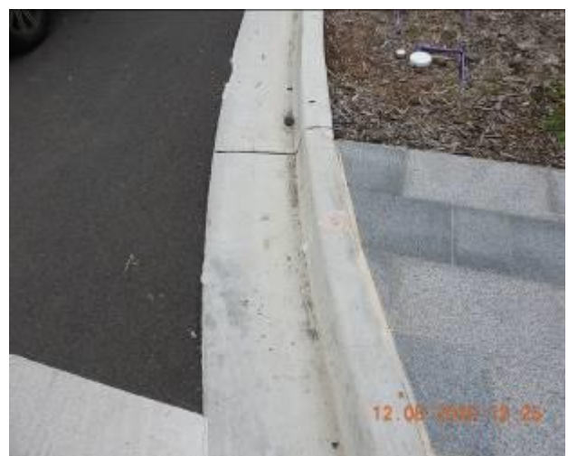
Figure 538 – Crack propagation and loss of material through kerb and gutter
