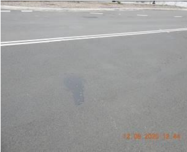
Figure 671 – Evidence of patchwork through road surface
