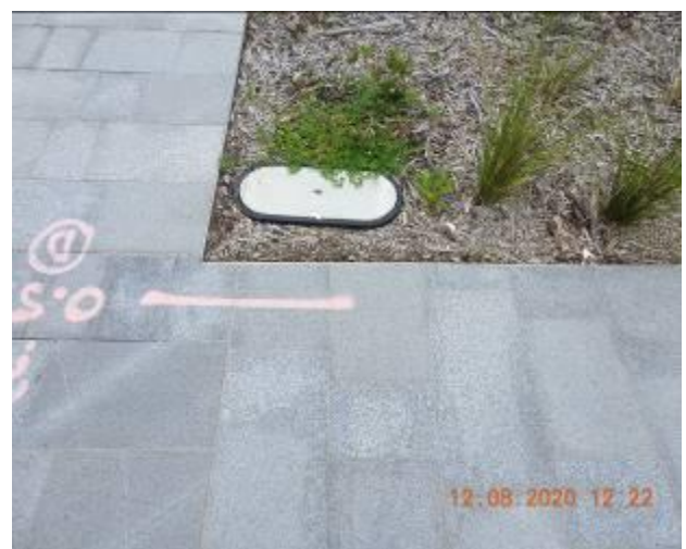
Figure 502 – Hairline crack propagation through footpath pavement/ General condition of service pit
