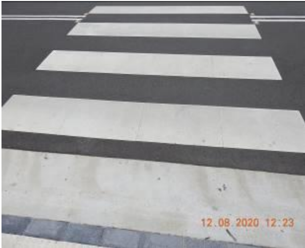
Figure 515 – Crack propagation and loss of material through road surface
