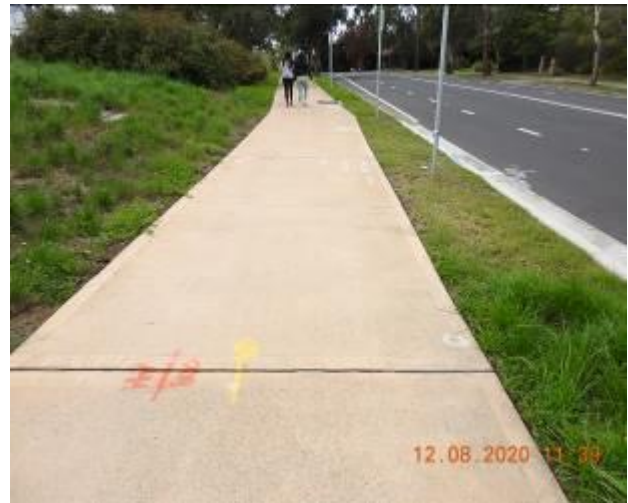
Figure 1664 – Loss of material through footpath pavement
