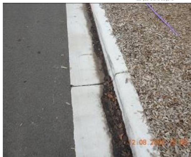
Figure 834 – Loss of material through kerb and gutter
