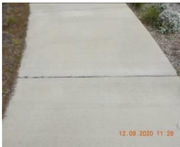
Figure 1121 – Crack propagation and loss of material through footpath pavement
