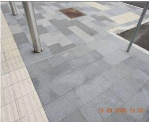
Figure 329 – Hairline cracking and efflorescence through footpath pavement
