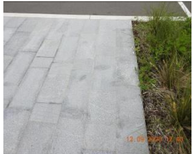
Figure 46 – Hairline cracking and efflorescence through footpath pavement
