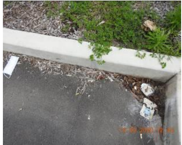
Figure 152 – Evidence of patchwork through kerb
