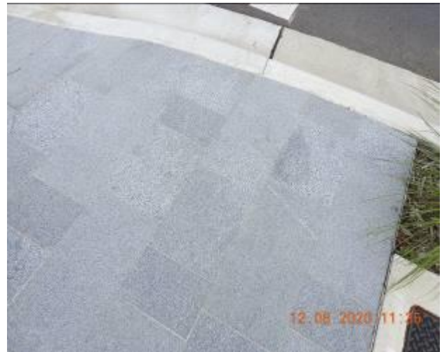
Figure 1632 – Hairline crack propagation through footpath pavement
