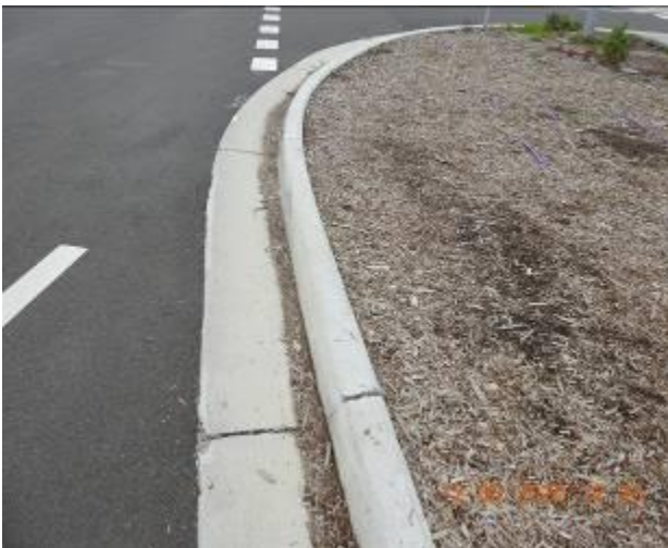
Figure 547 – Evidence of patchwork and loss of material through kerb and gutter
