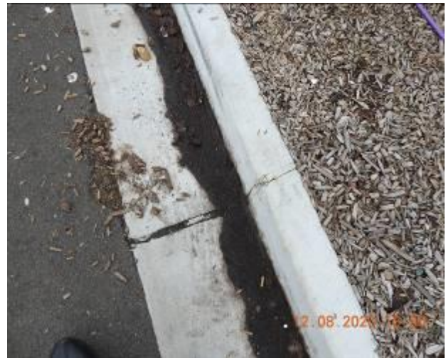
Figure 830 – Crack propagation and loss of material through kerb and gutter
