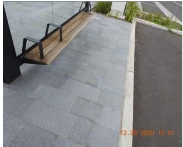
Figure 298 – Hairline cracking and efflorescence through footpath pavement
