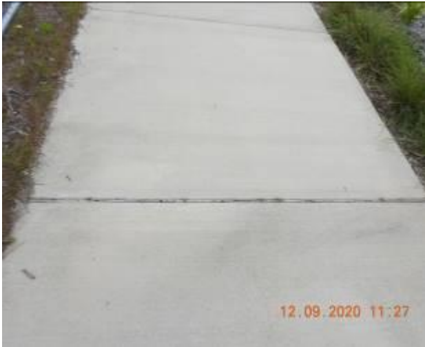
Figure 1113 – Loss of material through footpath pavement
