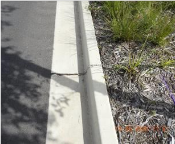
Figure 1727 – Crack propagation and loss of material through kerb and gutter
