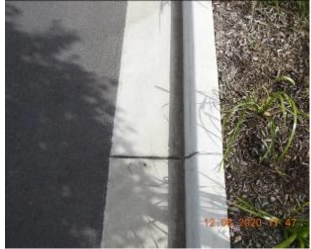
Figure 1680 – Crack propagation and loss of material through kerb and gutter
