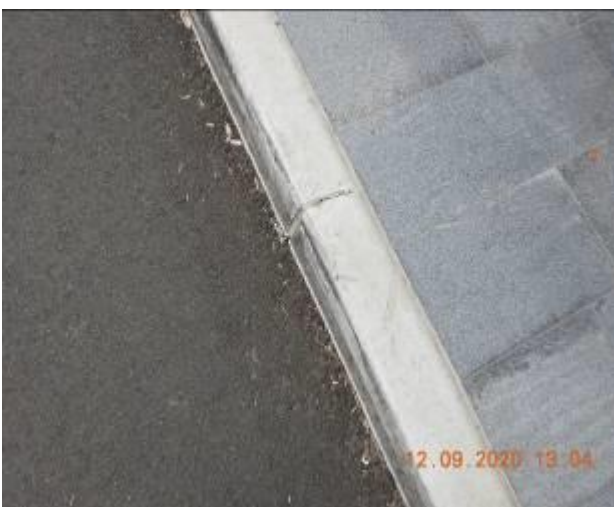
Figure 359 – Crack propagation and loss of material through kerb
