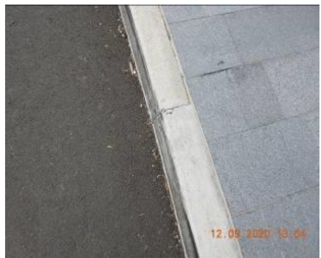
Figure 360 – Crack propagation through kerb
