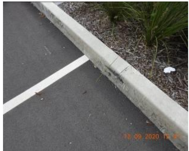
Figure 114 – Crack propagation through kerb
