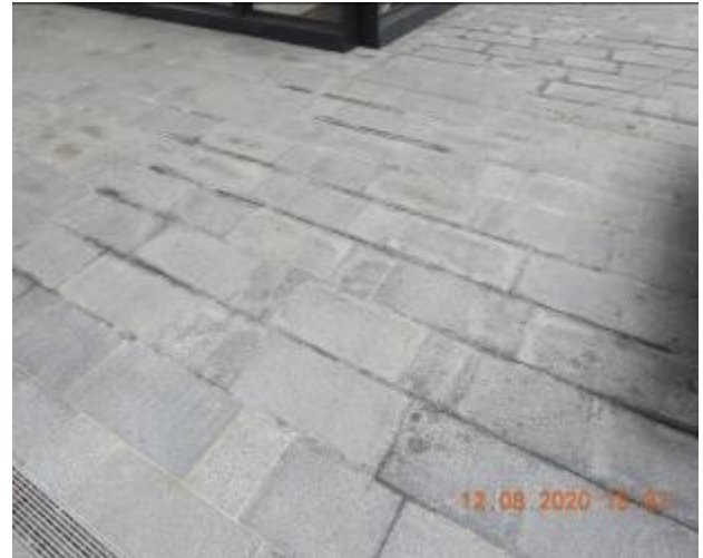
Figure 2021 – Efflorescence and loss of material through floor tiles
