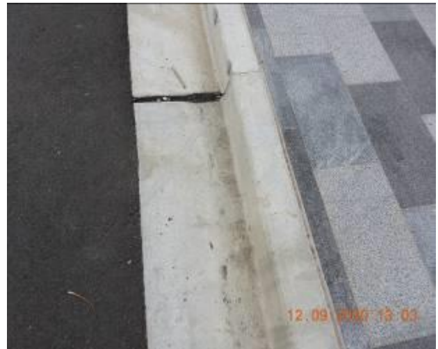
Figure 346 – Evidence of patchwork through gutter
