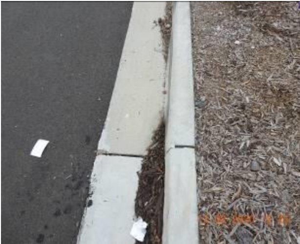
Figure 545 – Crack propagation and loss of material through kerb and gutter
