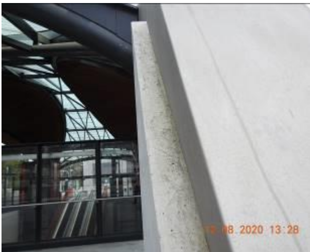
Figure 1988 – Hairline crack propagation and loss of material through external wall
