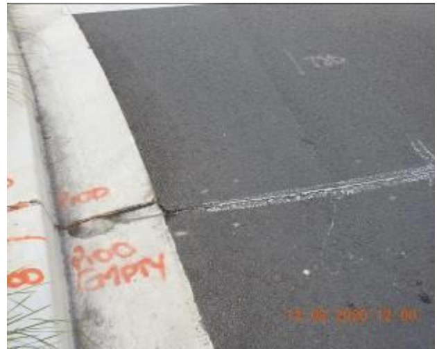
Figure 1826 – Loss of material through road surface
