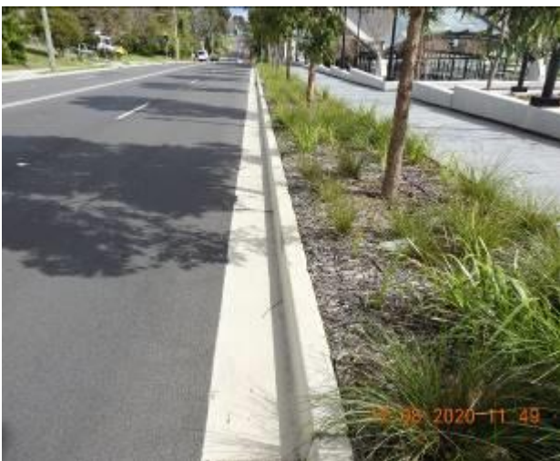
Figure 1707 – Loss of material through kerb
