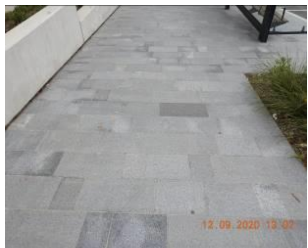
Figure 312 – Hairline cracking and efflorescence through footpath pavement
