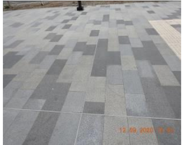
Figure 338 – Hairline cracking and efflorescence through footpath pavement
