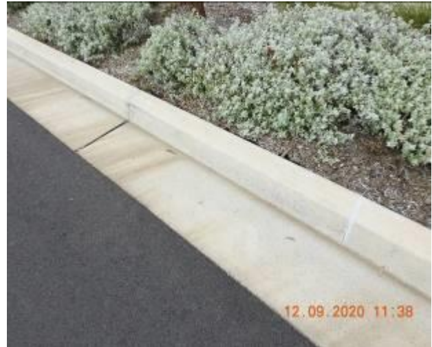
Figure 1252 – Hairline crack propagation through kerb
