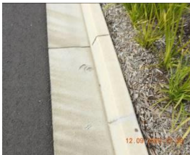
Figure 1267 – Crack propagation and loss of material through kerb and gutter
