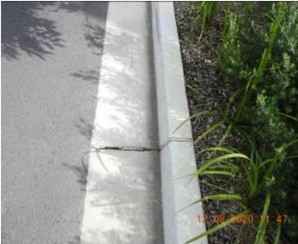
Figure 1681 – Crack propagation and loss of material through kerb and gutter
