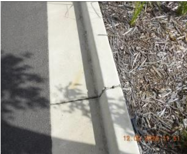
Figure 1717 – Crack propagation and loss of material through kerb and gutter
