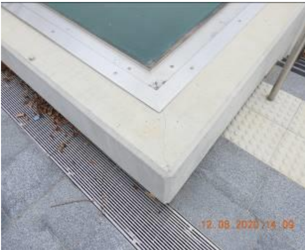
Figure 2257 – Crack propagation through retaining wall
