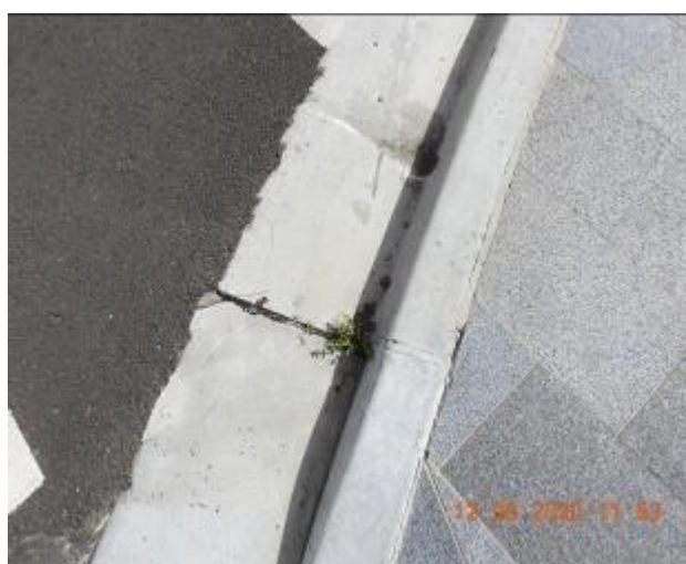
Figure 1753 – Evidence of patchwork and loss of material through kerb and gutter
