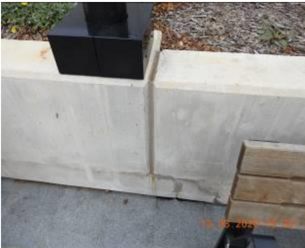
Figure 1998 – Crack propagation and loss of material through retaining wall
