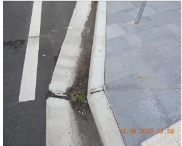
Figure 816 – Crack propagation and loss of material through kerb and gutter
