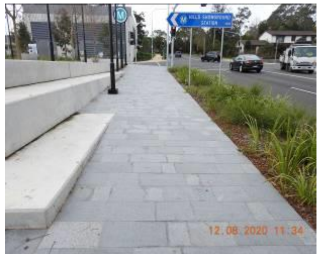
Figure 1618 – Efflorescence and hairline crack propagation through footpath pavement
