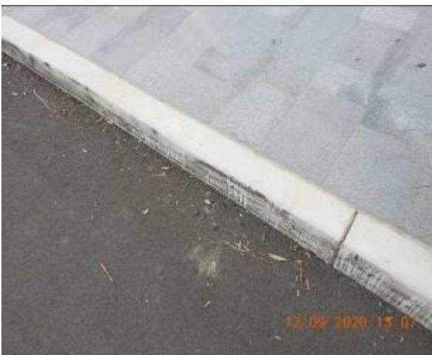
Figure 407 – Crack propagation through kerb
