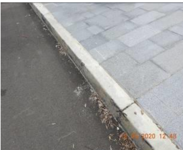
Figure 149 – Crack propagation through kerb
