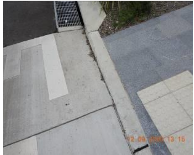
Figure 434 – Crack propagation and loss of material through layback
