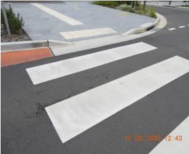
Figure 659 – Crack propagation and loss of material through road surface
