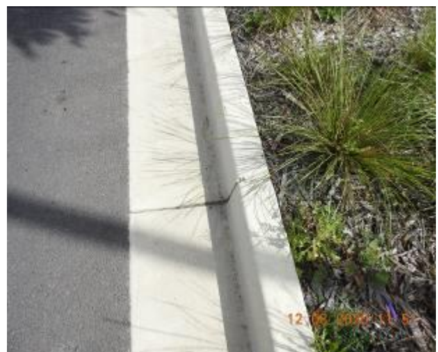
Figure 1726 – Crack propagation and loss of material through kerb and gutter
