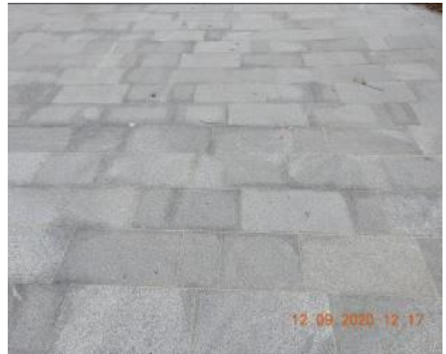
Figure 933 – Hairline crack propagation through footpath pavement
