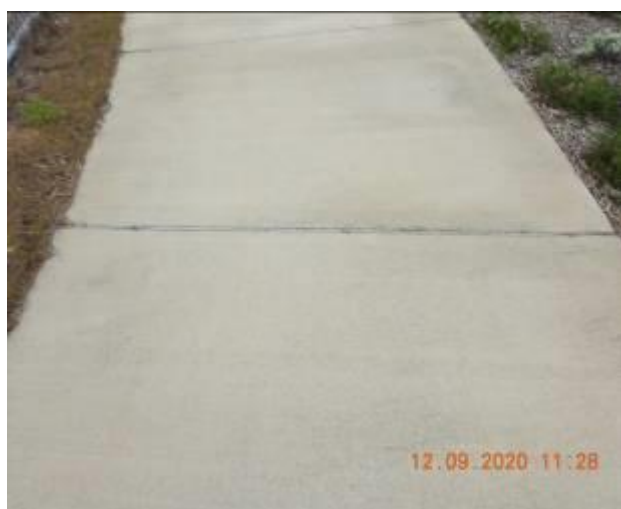
Figure 1123 – Loss of material through footpath pavement
