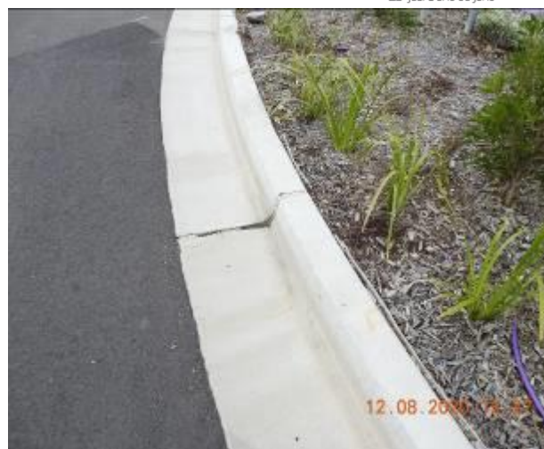
Figure 558 – Crack propagation and loss of material through kerb and gutter
