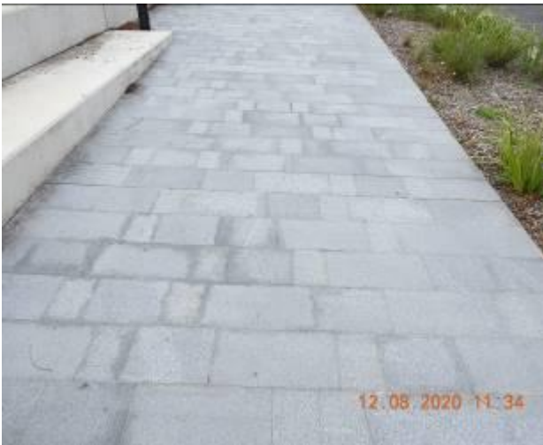
Figure 1621 – Hairline crack propagation through footpath pavement
