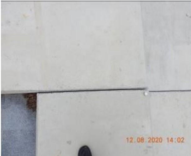
Figure 2177 – Separation through retaining wall
