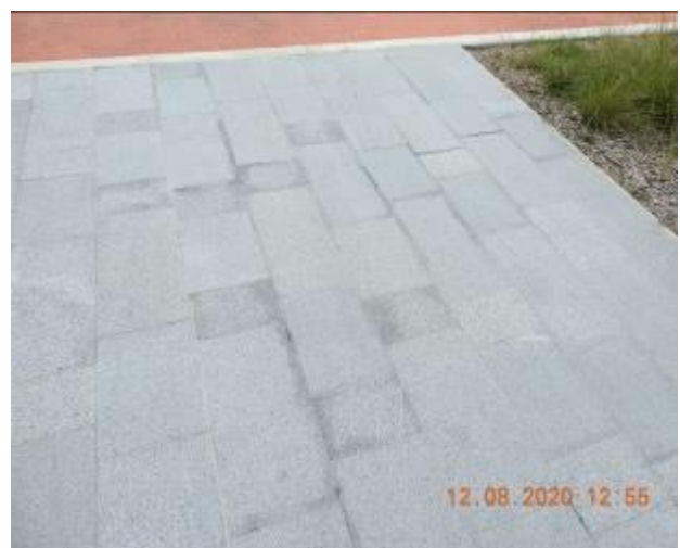
Figure 760 – Crack propagation and loss of material through footpath pavement
