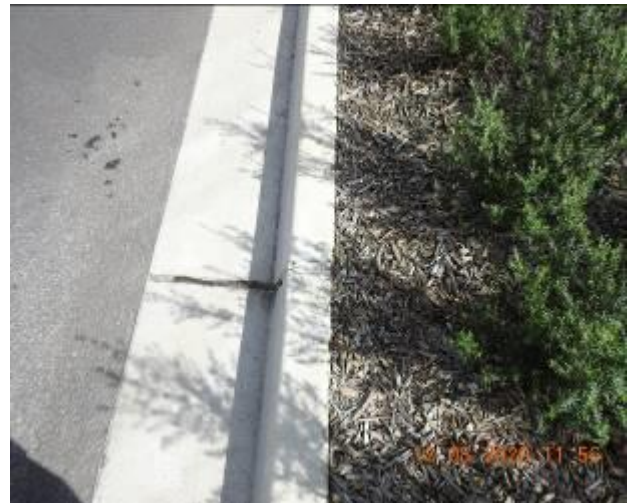
Figure 1784 – Crack propagation and loss of material through kerb and gutter
