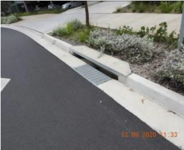
Figure 1173 – General condition of stormwater inlet pit/ Loss of material through kerb
