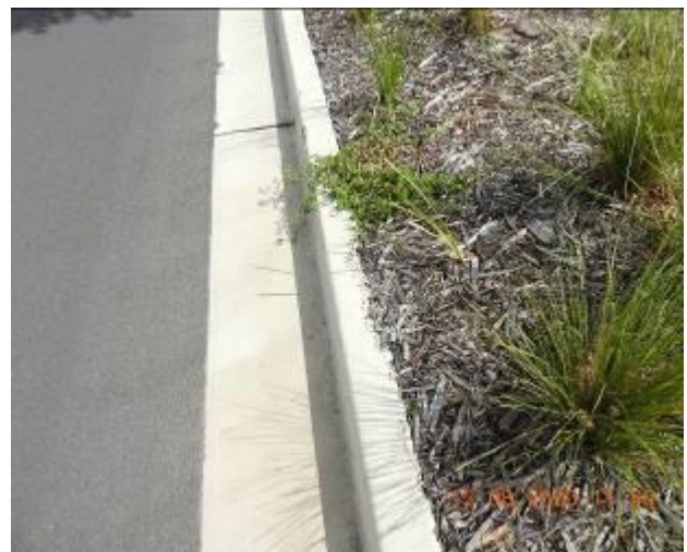
Figure 1714 – Loss of material through gutter
