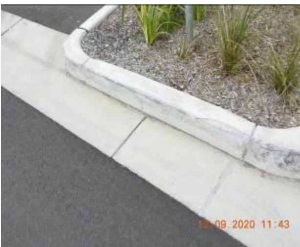
Figure 1333 – Crack propagation through kerb
