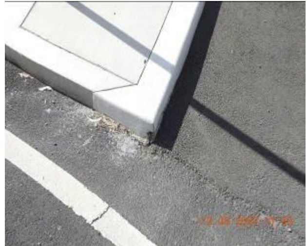
Figure 1806 – Loss of material through traffic island pavement
