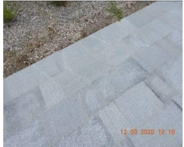
Figure 913 – Hairline crack propagation through footpath pavement
