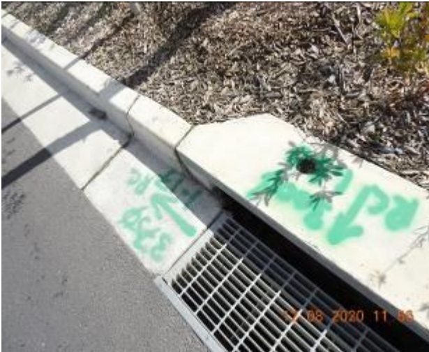
Figure 1781 – Crack propagation and loss of material through kerb
