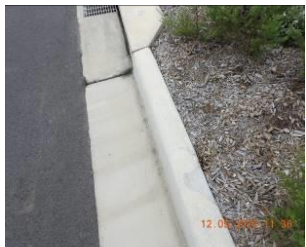
Figure 1226 – Evidence of patchwork and loss of material through kerb and gutter
