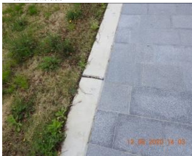
Figure 2183 – Loss of material through retaining wall
