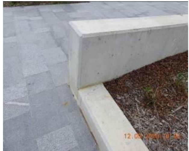
Figure 2246 – Separation through retaining wall
