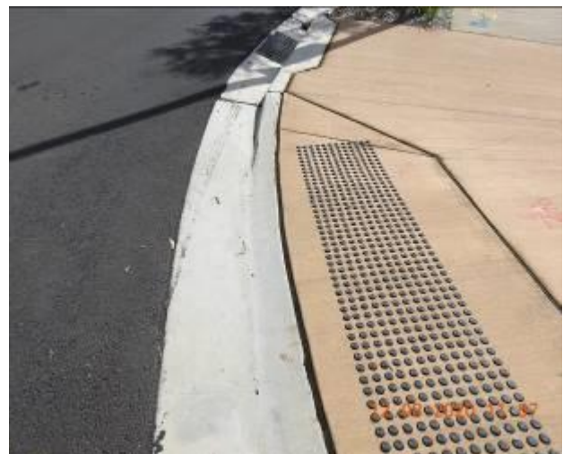
Figure 1802 – Crack propagation through layback and gutter
