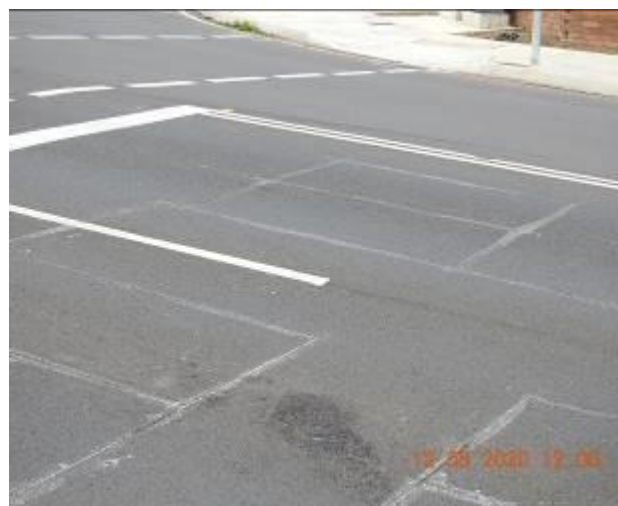
Figure 1850 – Evidence of patchwork and loss of material through road surface
