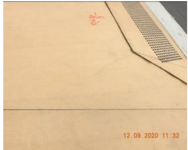
Figure 1162 – Crack propagation through footpath pavement
