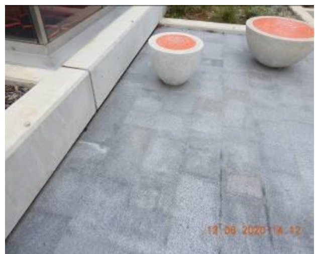
Figure 2296 – Efflorescence and crack propagation through walkway floor
