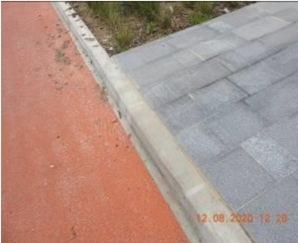
Figure 587 – Evidence of patchwork and hairline cracking through kerb
