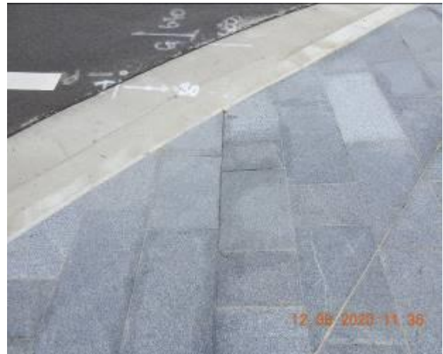
Figure 1640 – Crack propagation and loss of material through footpath pavement
