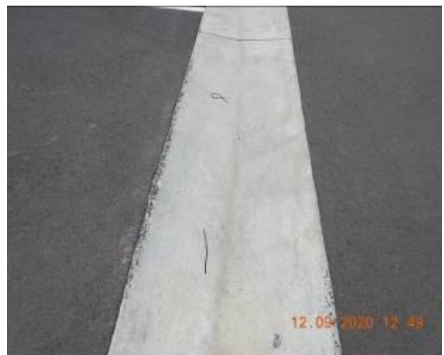
Figure 162 – Loss of material through gutter
