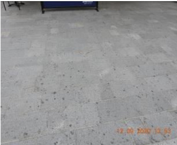
Figure 2488 – Hairline crack propagation through walkway floor
