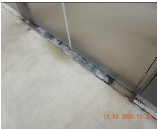
Figure 2400 – Loss of material through walkway pavement
