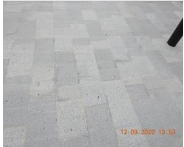
Figure 2475 – Hairline crack propagation through walkway floor
