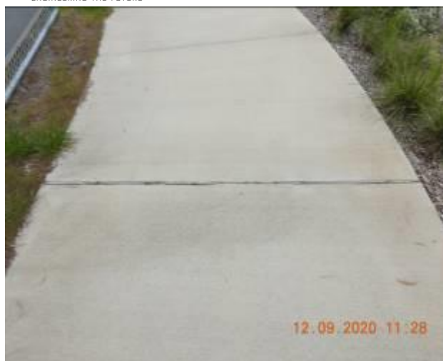
Figure 1119 – Crack propagation and loss of material through footpath pavement
