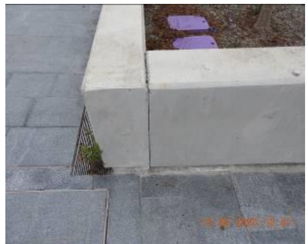
Figure 2146 – Separation through retaining wall
