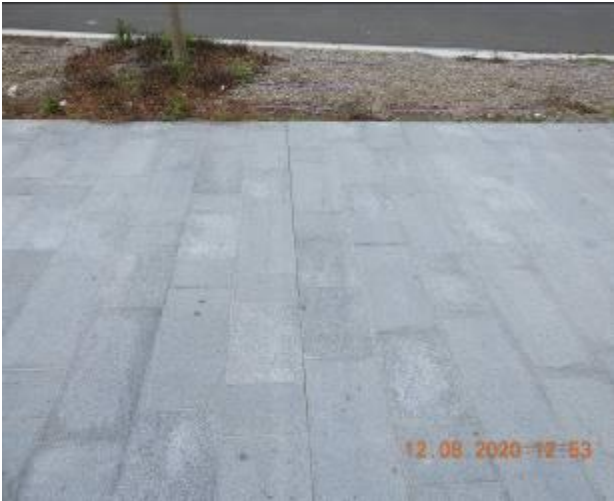
Figure 725 – Efflorescence, hairline crack propagation and loss of material through footpath pavement
