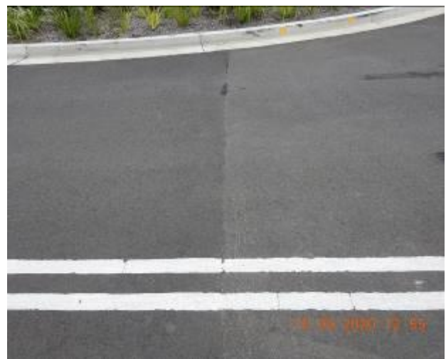
Figure 226 – Loss of material through road surface
