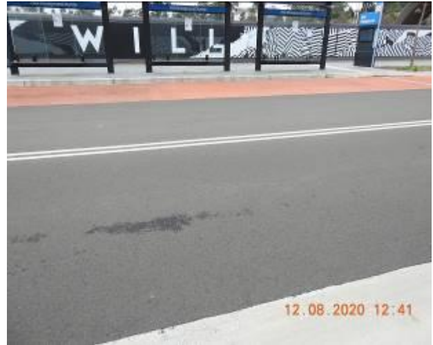
Figure 636 – Crack propagation and loss of material through road surface
