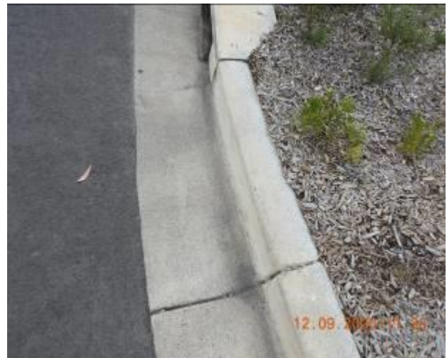
Figure 1230 – Loss of material through kerb and gutter
