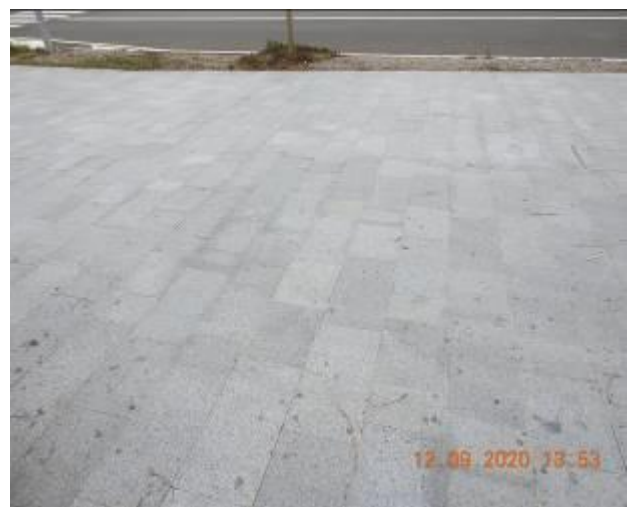
Figure 2485 – Hairline crack propagation through walkway floor
