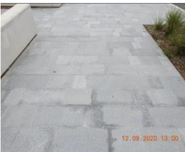
Figure 281 – Hairline cracking and efflorescence through footpath pavement
