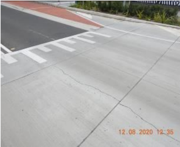
Figure 605 – Crack propagation and loss of material through road surface ramp
