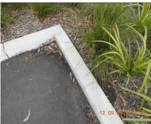
Figure 1357 – Evidence of patchwork through kerb
