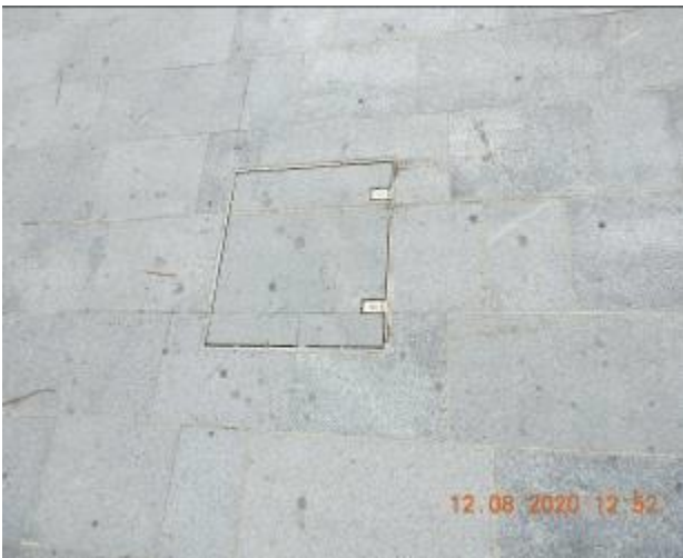
Figure 721 – Loss of material through service pit
