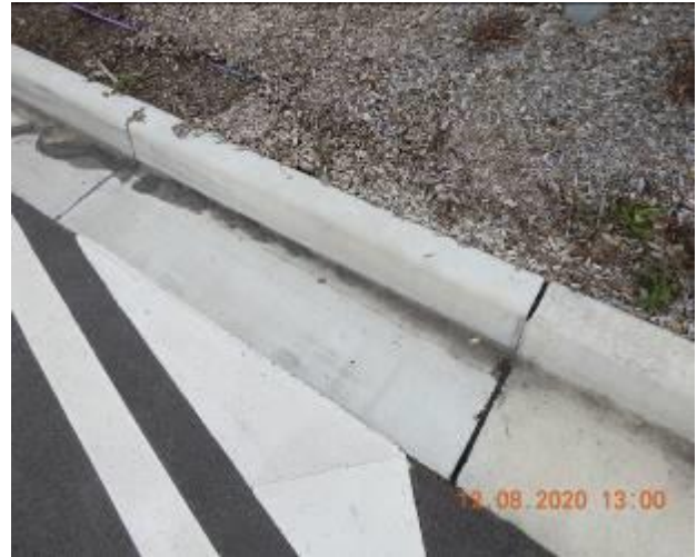
Figure 822 – Loss of material through kerb
