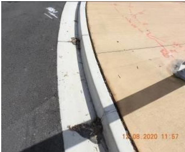
Figure 1799 – Evidence of patchwork, crack propagation and loss of material through kerb
