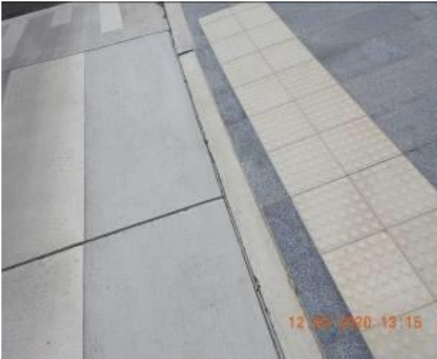
Figure 433 – Crack propagation and loss of material through layback
