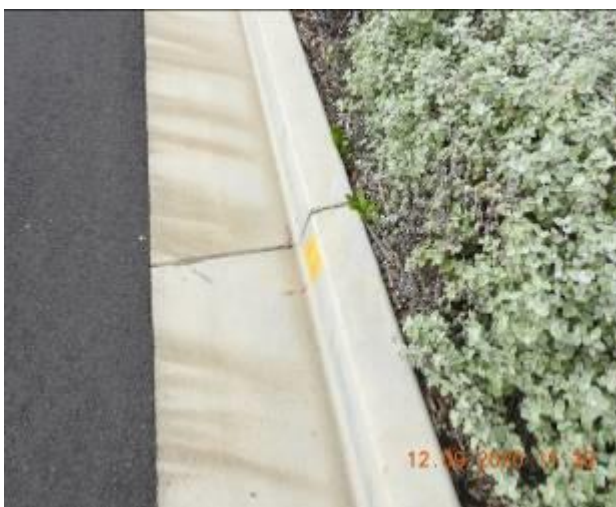
Figure 1261 – Crack propagation and loss of material through curb and gutter
