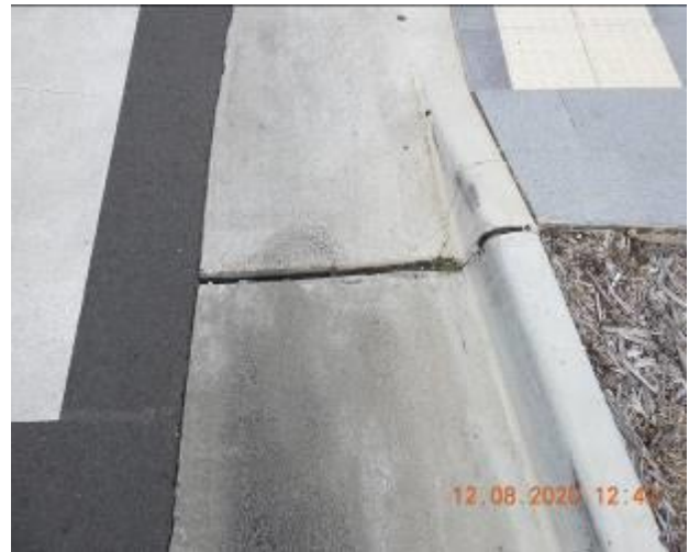
Figure 656 – Crack propagation and loss of material through gutter
