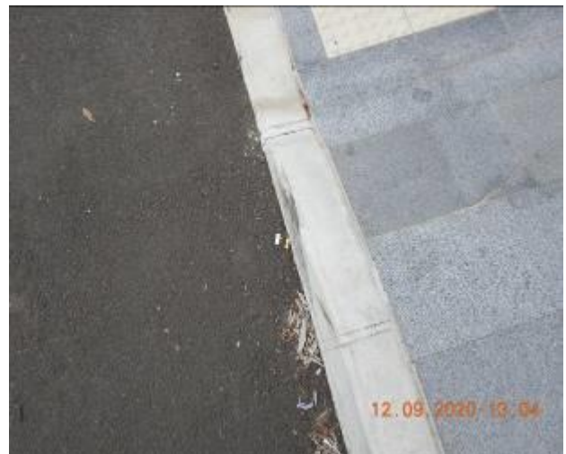
Figure 352 – Crack propagation through kerb
