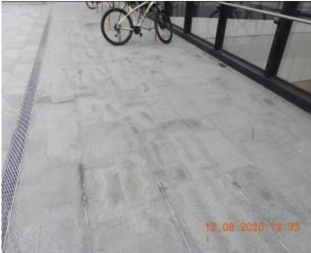
Figure 2032 – Efflorescence and loss of material through floor tiles
