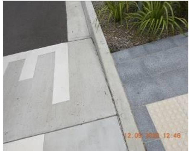
Figure 98 – Crack propagation through layback
