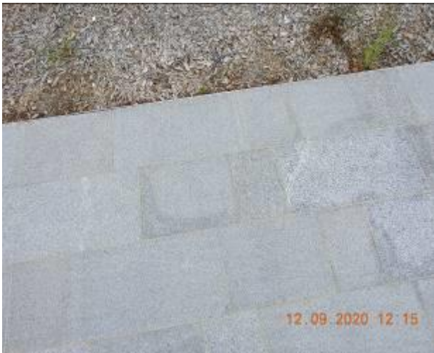
Figure 908 – Crack propagation and loss of material through footpath pavement
