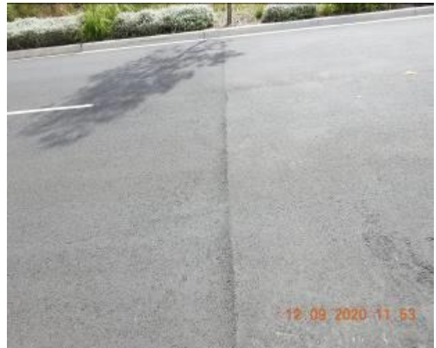
Figure 1434 – Evidence of patchwork through road surface
