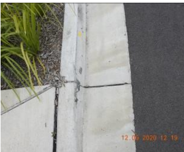
Figure 964 – Crack propagation and loss of material through kerb and gutter
