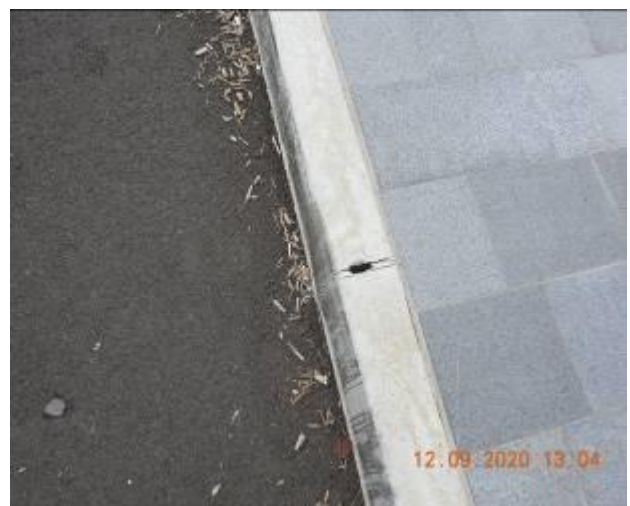
Figure 366 – Loss of material through kerb
