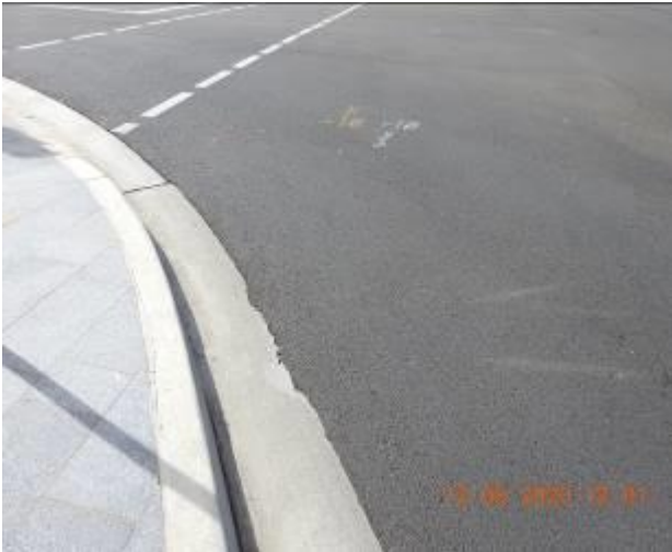
Figure 1829 – Loss of material through road surface
