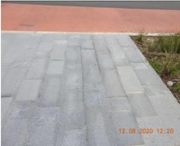
Figure 485 – Loss of material through footpath pavement
