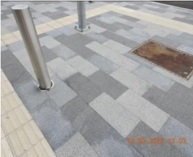
Figure 331 – Hairline cracking and efflorescence through footpath pavement
