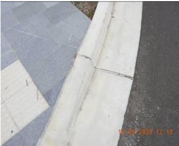
Figure 956 – Crack propagation and loss of material through kerb and gutter
