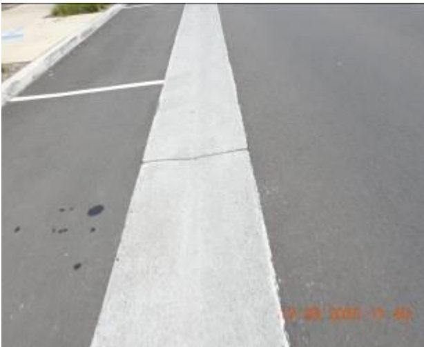
Figure 1367 – Crack propagation and loss of material through gutter
