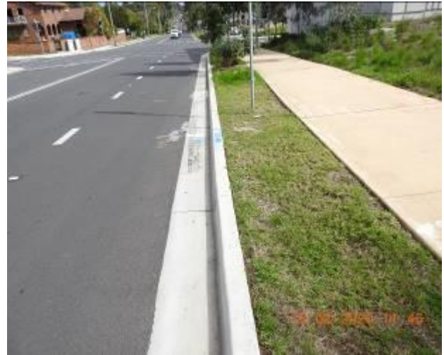
Figure 1674 – General condition of kerb and gutter
