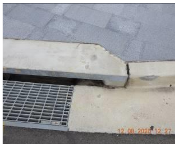
Figure 562 – Loss of material through kerb and gutter
