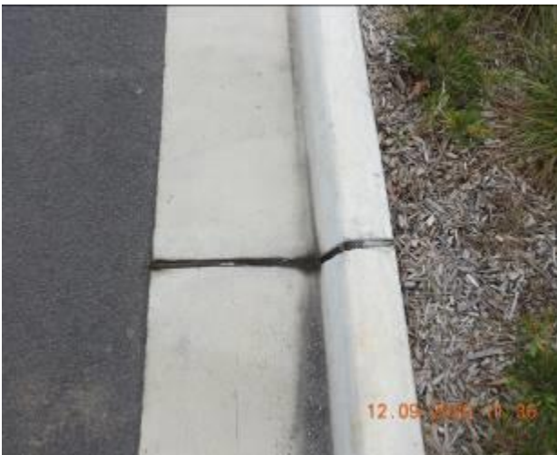
Figure 1223 – Crack propagation and loss of material through kerb and gutter
