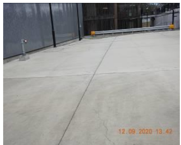
Figure 2431 – Crack propagation through driveway pavement
