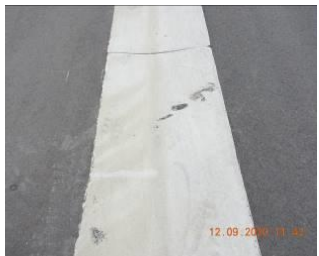
Figure 1328 – Evidence of patchwork, crack propagation and loss of material through gutter
