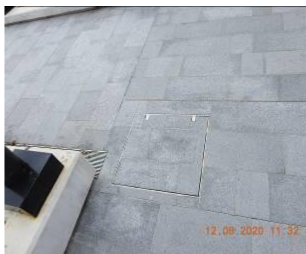
Figure 1606 – Loss of material through service pit pavement/Crack propagation and loss of material through footpath pavement
