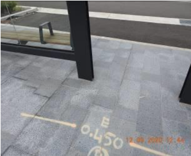
Figure 73 – Hairline cracking and efflorescence through footpath pavement
