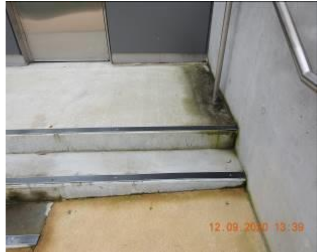
Figure 2403 – Loss of material through steps pavement
