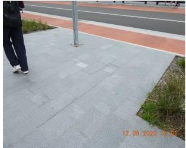
Figure 756 – Loss of material through footpath pavement
