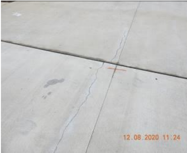
Figure 1541 – Crack propagation and loss of material through driveway pavement
