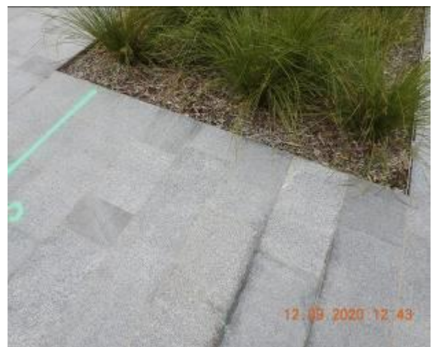
Figure 42 – Hairline cracking and efflorescence through footpath pavement
