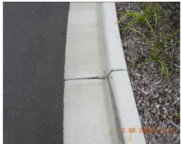
Figure 180 – Crack propagation and loss of material through kerb and gutter
