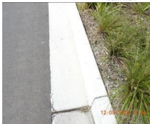
Figure 1372 – Crack propagation and loss of material through kerb and gutter
