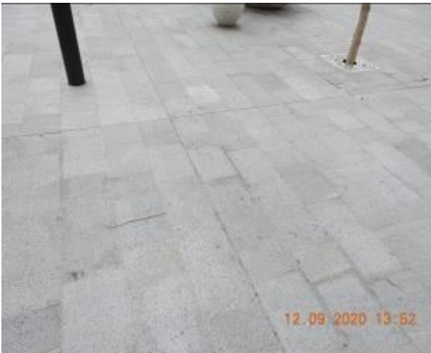
Figure 2452 – Hairline crack propagation through walkway floor
