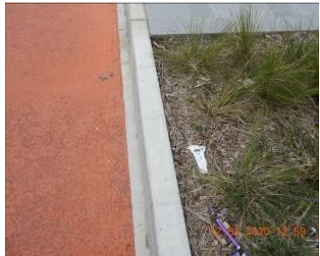
Figure 806 – Hairline crack propagation and evidence of patchwork through kerb
