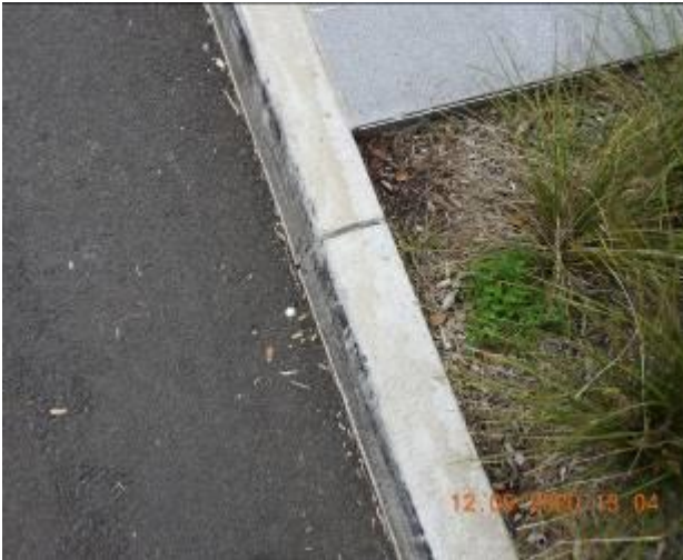
Figure 361 – Crack propagation through kerb
