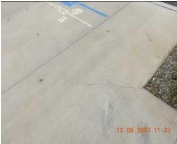
Figure 1073 – Crack propagation through footpath pavement
