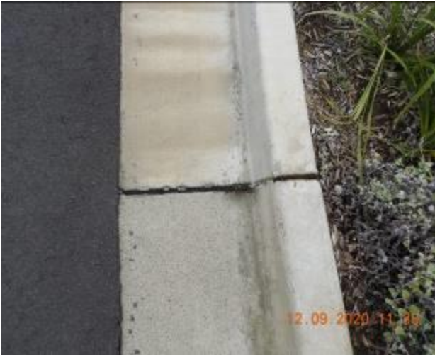
Figure 1209 – Crack propagation and loss of material through kerb and gutter
