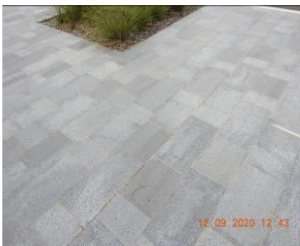
Figure 53 – Hairline cracking and efflorescence through footpath pavement
