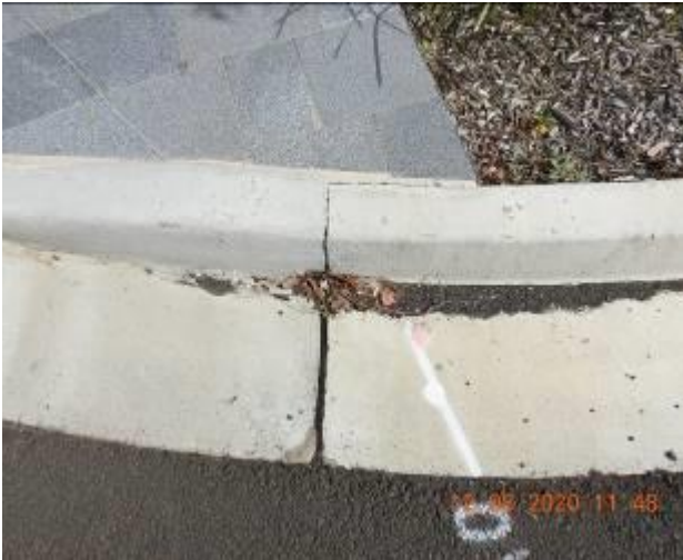
Figure 1691 – Loss of material through kerb and evidence of patchwork through gutter
