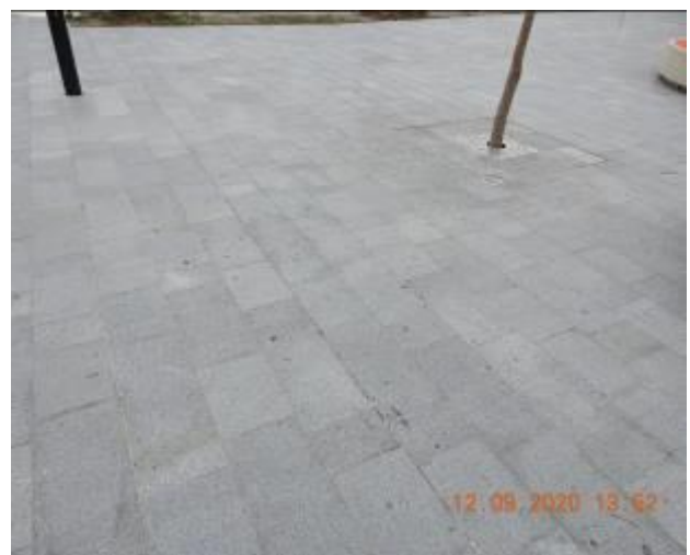
Figure 2455 – Hairline crack propagation through walkway floor
