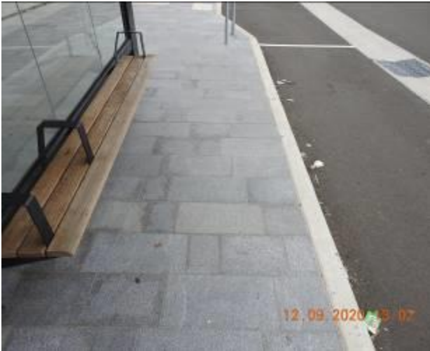
Figure 319 – Hairline cracking and efflorescence through footpath pavement
