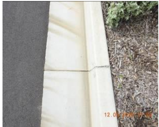
Figure 1278 – Crack propagation and loss of material through kerb and gutter
