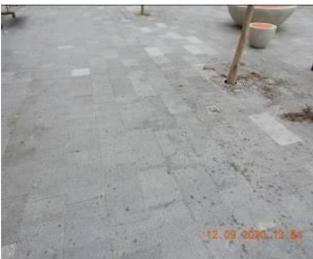
Figure 2496 – Hairline crack propagation through walkway floor
