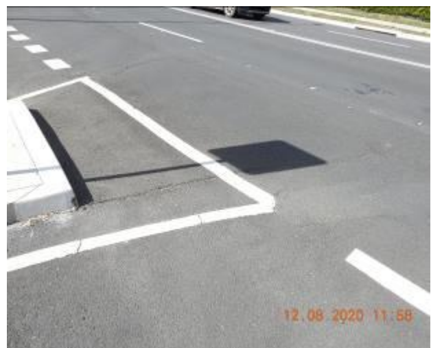
Figure 1804 – Crack propagation and loss of material through road surface
