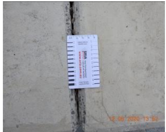
Figure 2114 – Separation through retaining wall Approx. 3mm in width
