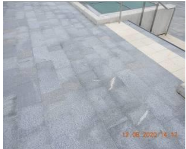
Figure 2294 – Efflorescence and crack propagation through walkway floor
