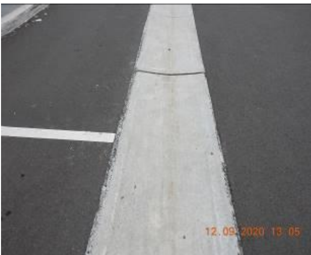
Figure 377 – Crack propagation and loss of material through gutter
