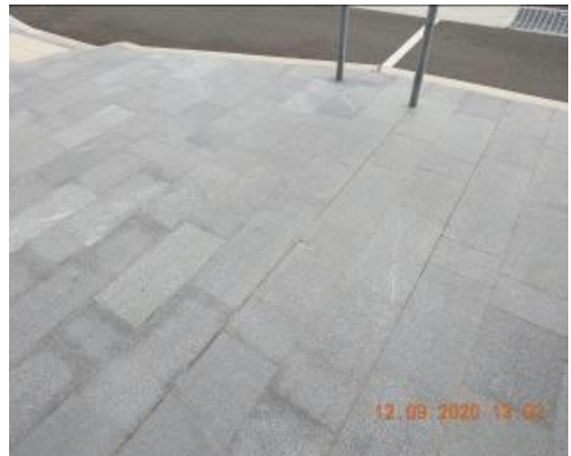
Figure 322 – Hairline cracking and efflorescence through footpath pavement
