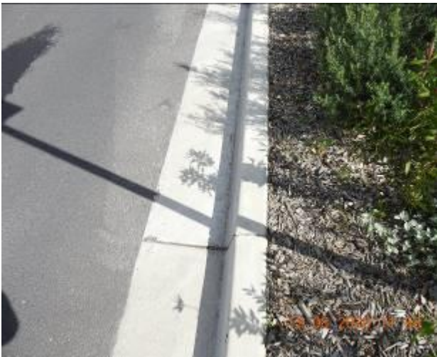
Figure 1783 – Loss of material through kerb and gutter
