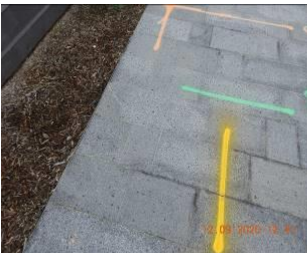
Figure 11 – Hairline cracking and efflorescence through footpath pavement
