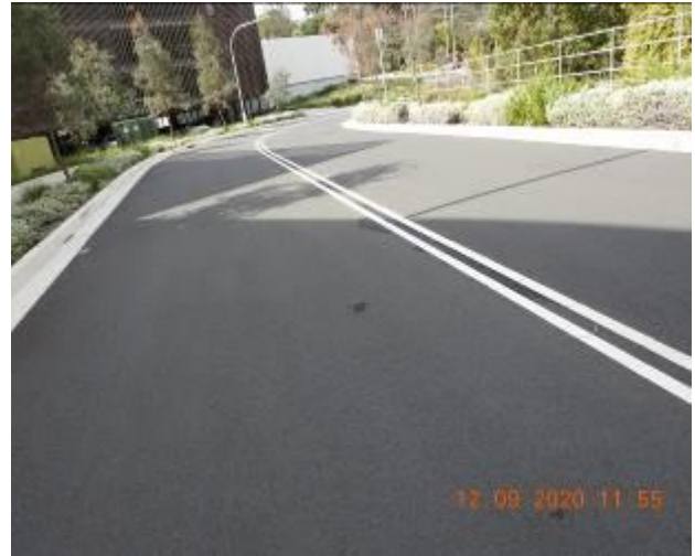
Figure 1456 – Evidence of patchwork through road surface
