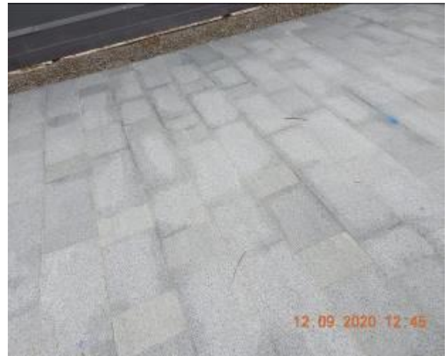
Figure 82 – Hairline cracking and efflorescence through footpath pavement
