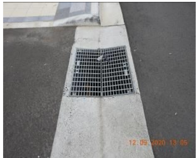
Figure 382 – General condition of stormwater inlet pit
