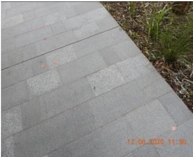
Figure 1591 – Loss of material through footpath pavement
