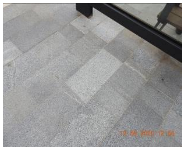
Figure 772 – Hairline crack propagation through footpath pavement
