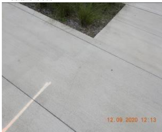
Figure 888 – Crack propagation through footpath pavement
