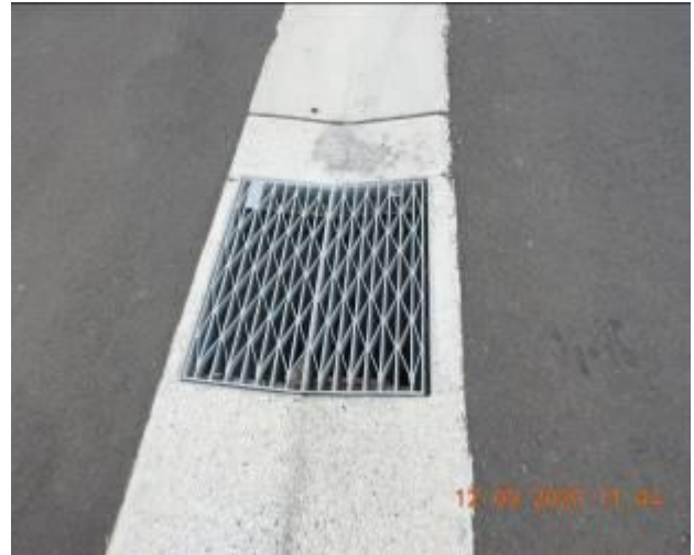
Figure 1348 – Crack propagation and loss of material through gutter/General condition of stormwater inlet pit
