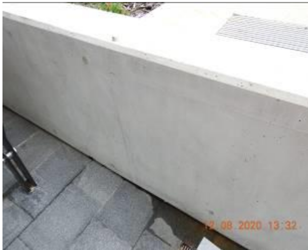
Figure 2016 – Hairline crack propagation through retaining wall
