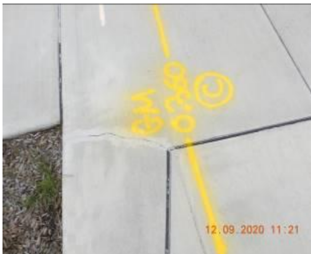
Figure 1055 – Crack propagation and loss of material through footpath pavement
