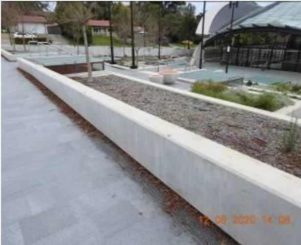
Figure 2249 – General condition of retaining wall
