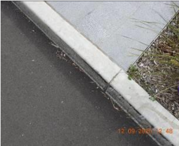
Figure 139 – Crack propagation through kerb
