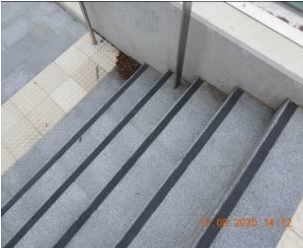
Figure 2285 – Separation through staircase floor
