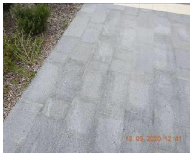
Figure 6 – Hairline cracking and efflorescence through footpath pavement
