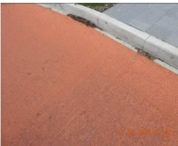
Figure 645 – Crack propagation and loss of material through road surface
