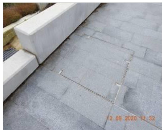
Figure 1600 – Loss of material through service pit pavement
