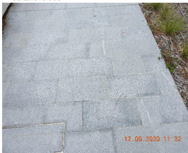
Figure 1601 – Hairline crack propagation and loss of material through footpath pavement
