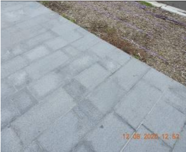
Figure 719 – Loss of material through footpath pavement
