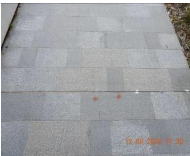
Figure 1593 – Crack propagation and loss of material through footpath pavement
