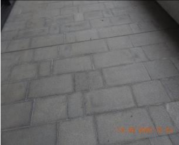
Figure 1966 – Efflorescence through floor tiles
