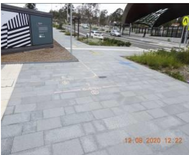
Figure 507 – Hairline crack propagation and loss of material through footpath pavement
