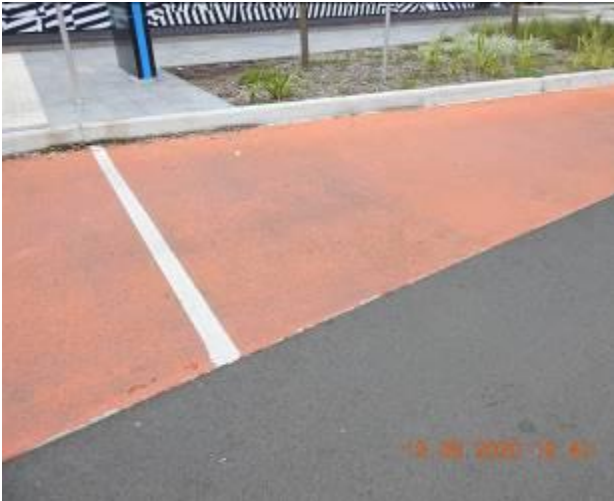
Figure 647 – Paint flaking and loss of material through road surface
