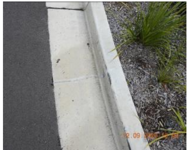
Figure 94 – Evidence of patchwork through kerb and gutter
