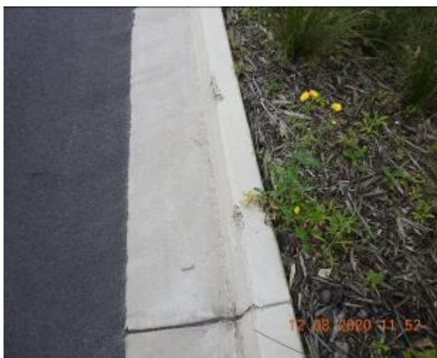
Figure 1735 – Crack propagation and loss of material through kerb
