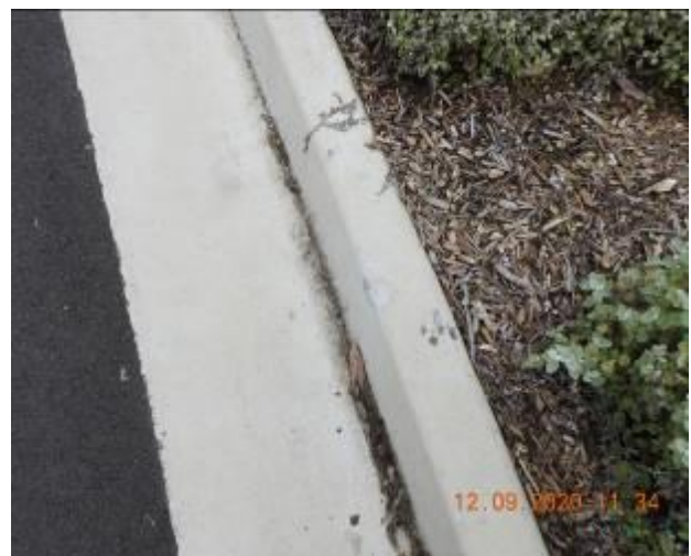
Figure 1190 – Evidence of patchwork through kerb
