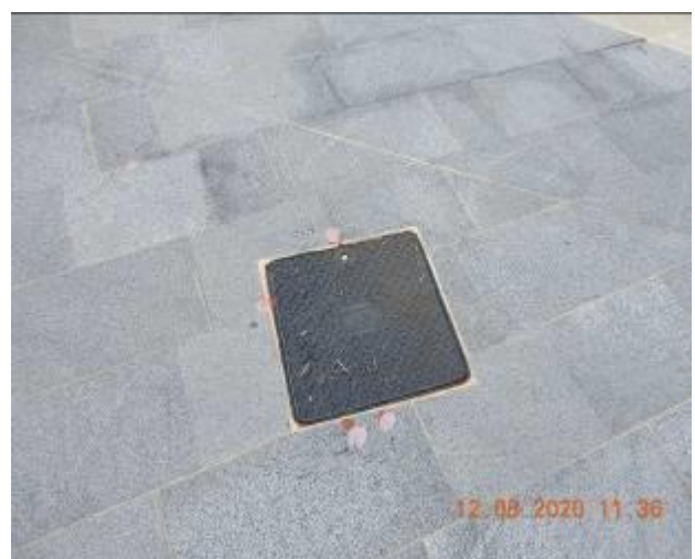
Figure 1636 – General condition of service pit/ Hairline crack propagation through footpath pavement
