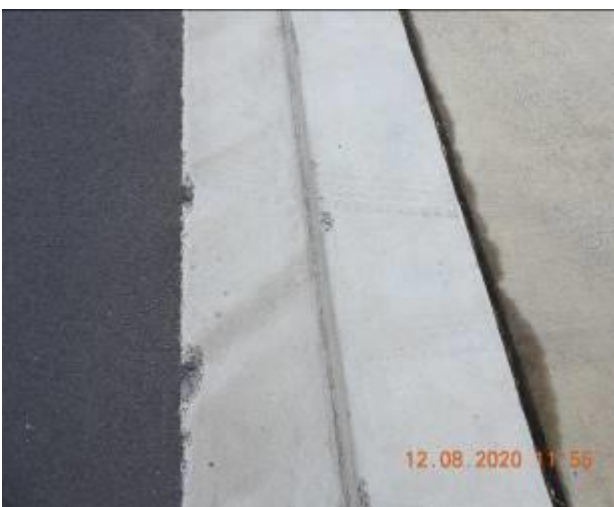
Figure 1773 – Loss of material through layback and gutter
