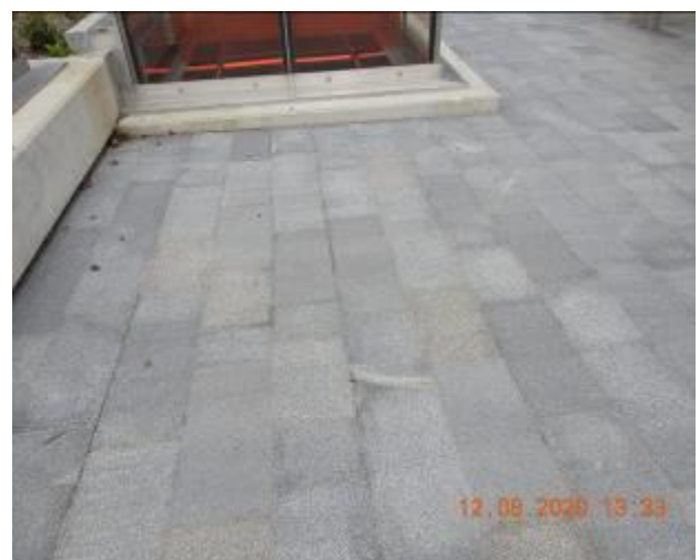
Figure 2037 – Hairline crack propagation through floor tiles
