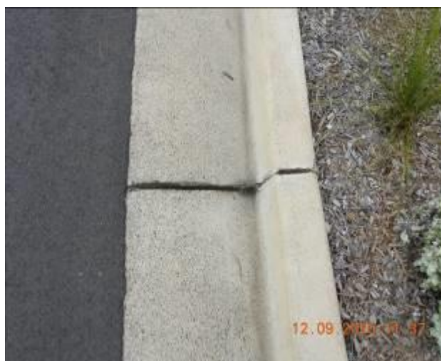
Figure 1237 – Crack propagation and loss of material through kerb and gutter
