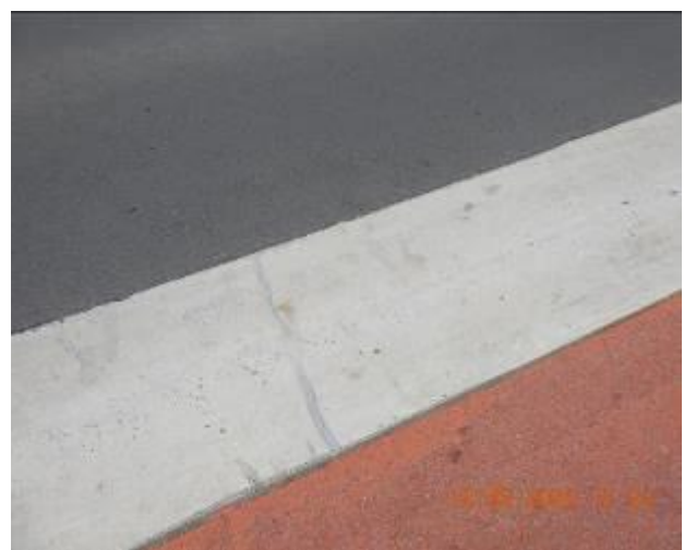
Figure 610 – Hairline crack propagation through and evidence of patchwork through road surface
