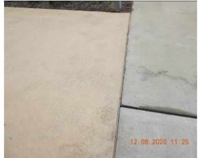
Figure 1548 – Loss of material through footpath pavement
