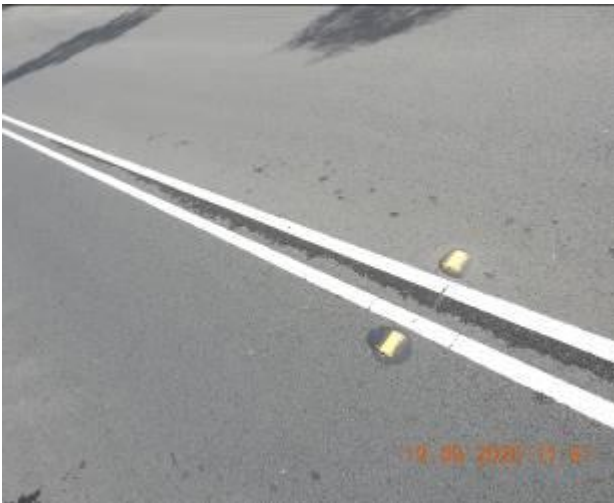
Figure 1415 – Evidence of patchwork, crack propagation and loss of material through road surface
