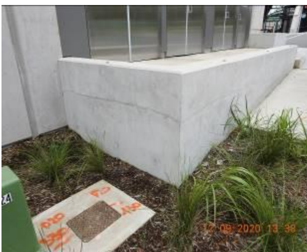
Figure 2394 – Loss of material through retaining wall
