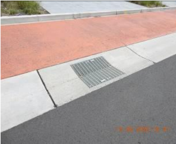
Figure 641 – Crack propagation and loss of material through road surface
