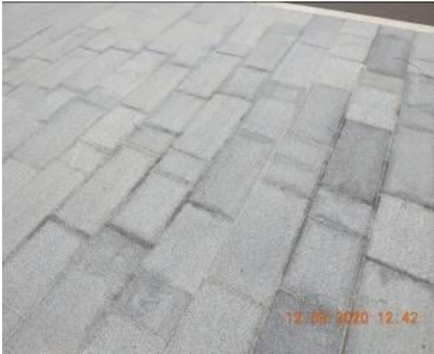
Figure 31 – Hairline cracking and efflorescence through footpath pavement
