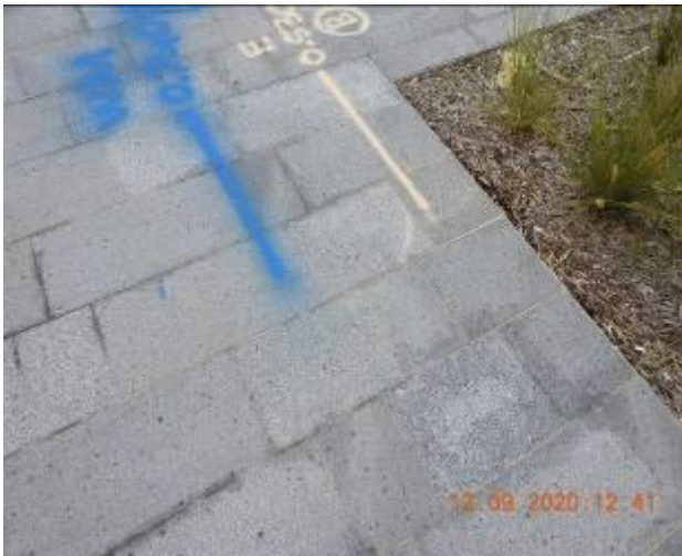
Figure 9 – Hairline cracking and efflorescence through footpath pavement
