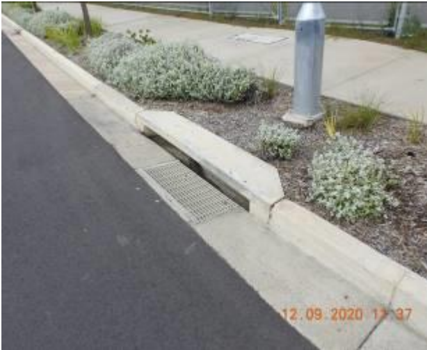
Figure 1239 – General condition of stormwater inlet pit /Loss of material through kerb
