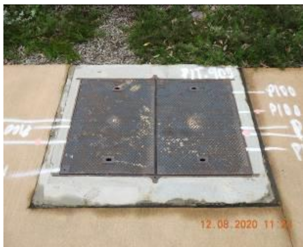
Figure 1531 – Crack propagation and loss of material through service pit pavement
