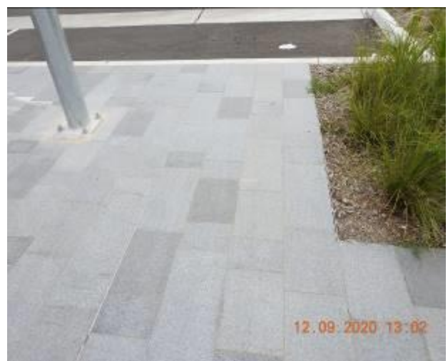
Figure 306 – Hairline cracking and efflorescence through footpath pavement
