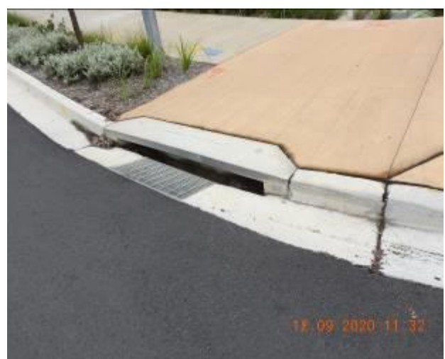
Figure 1166 – General condition of stormwater inlet pit/Evidence of patchwork through kerb
