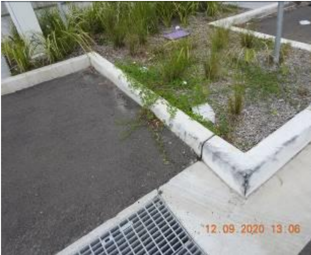
Figure 385 – Loss of material through kerb
