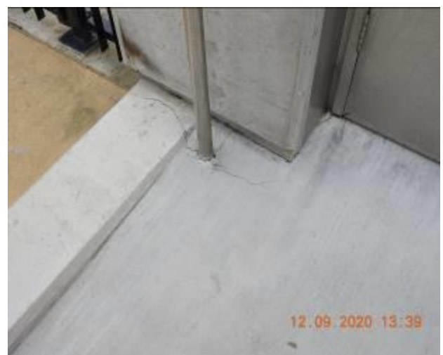
Figure 2407 – Crack propagation and loss of material through steps pavement
