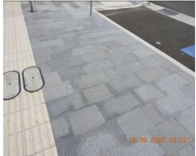
Figure 326 – Hairline cracking and efflorescence through footpath pavement
