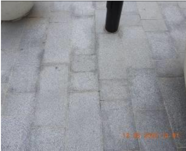
Figure 2165 – Loss of material through walkway floor
