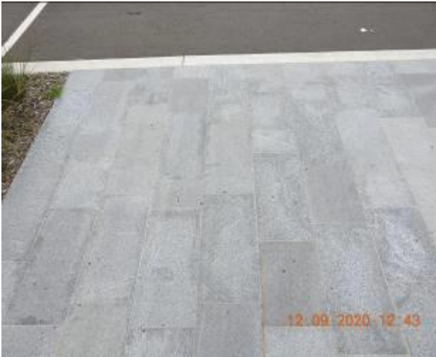
Figure 55 – Hairline cracking and efflorescence through footpath pavement
