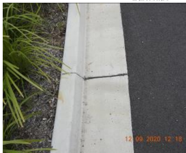
Figure 943 – Crack propagation and loss of material through kerb and gutter
