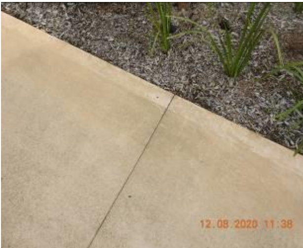
Figure 1657 – Separation through footpath pavement
