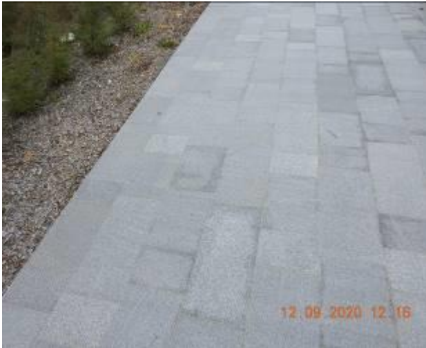
Figure 924 – Hairline crack propagation through footpath pavement
