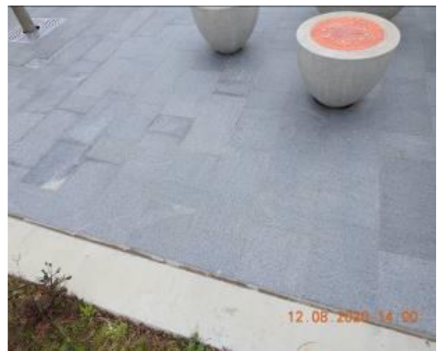
Figure 2156 – Hairline crack propagation and loss of material through walkway floor
