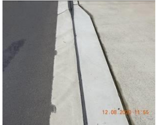
Figure 1776 – Loss of material through layback and gutter
