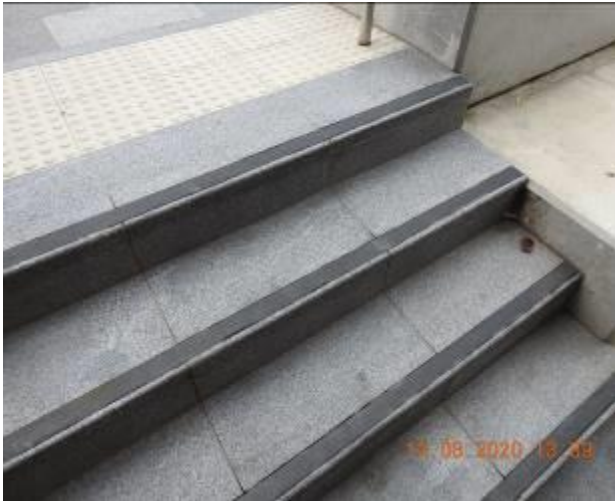
Figure 2086 – Separation through staircase pavement
