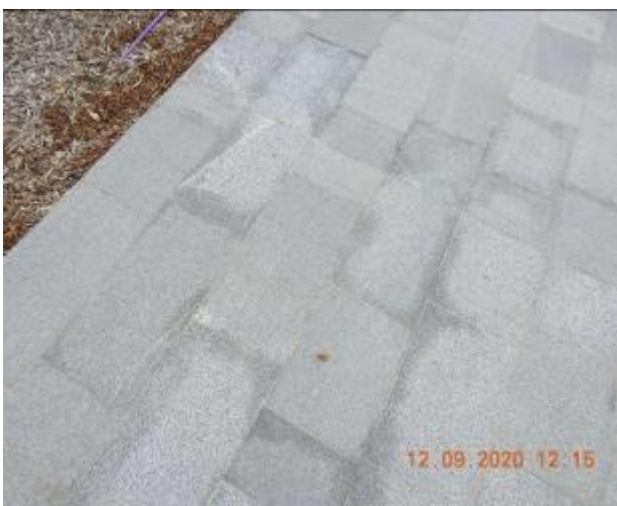
Figure 904 – Loss of material through footpath pavement
