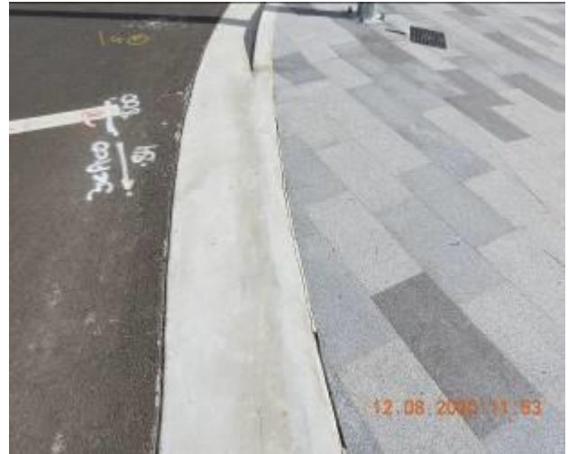
Figure 1748 – Loss of material through layback
