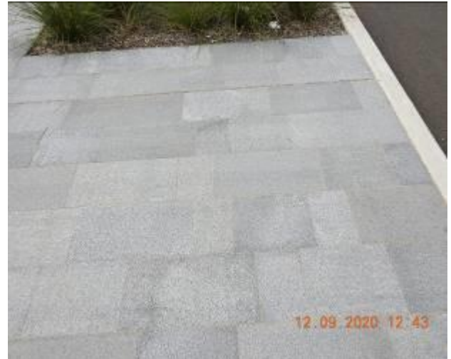
Figure 38 – Hairline cracking and efflorescence through footpath pavement
