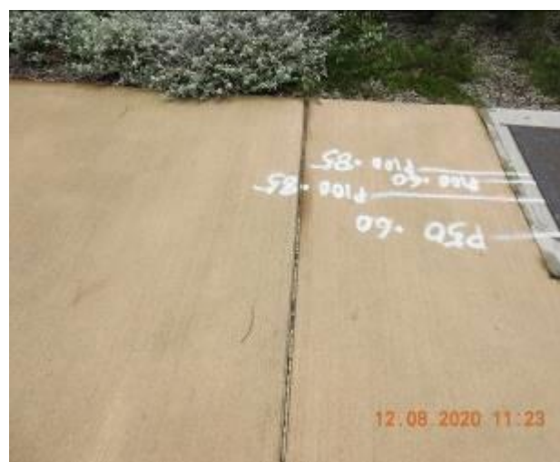
Figure 1534 – Crack propagation and loss of material through footpath pavement
