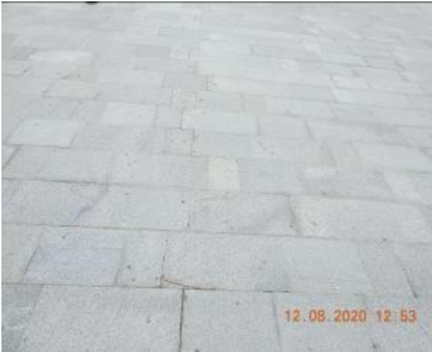
Figure 731 – Efflorescence, hairline crack propagation and loss of material through footpath pavement
