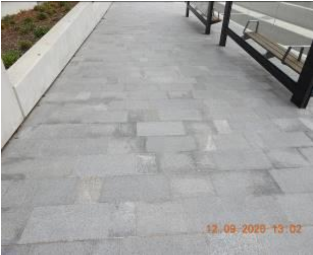
Figure 313 – Hairline cracking and efflorescence through footpath pavement
