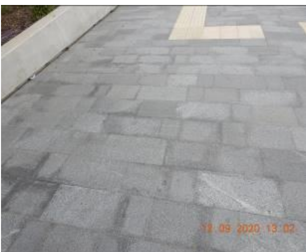
Figure 323 – Hairline cracking and efflorescence through footpath pavement
