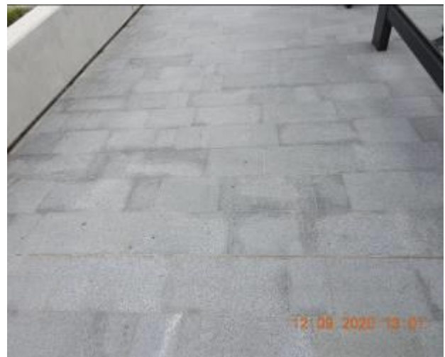
Figure 294 – Hairline cracking and efflorescence through footpath pavement
