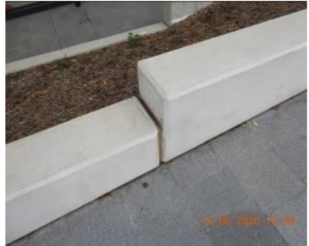
Figure 2093 – Crack propagation and loss of material through retaining wall
