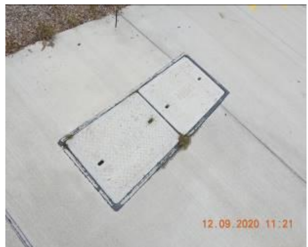
Figure 1058 – Crack propagation and loss of material through service pit pavement
