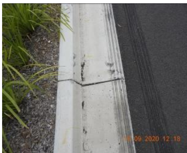
Figure 946 – Crack propagation and loss of material through kerb and gutter
