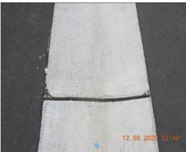
Figure 119 – Crack propagation and loss of material through gutter
