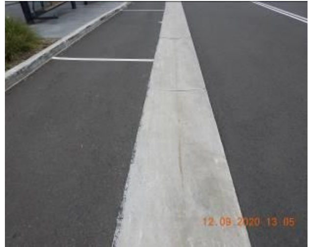
Figure 374 – Crack propagation through gutter
