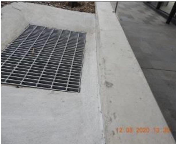
Figure 2058 – Crack propagation through stormwater inlet pit
