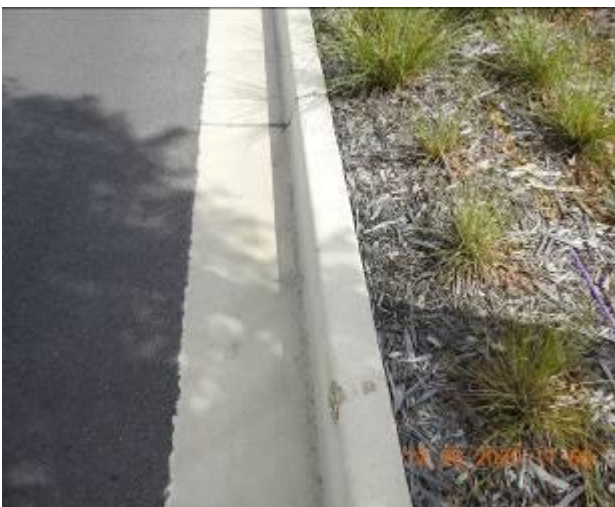
Figure 1713 – Loss of material through gutter
