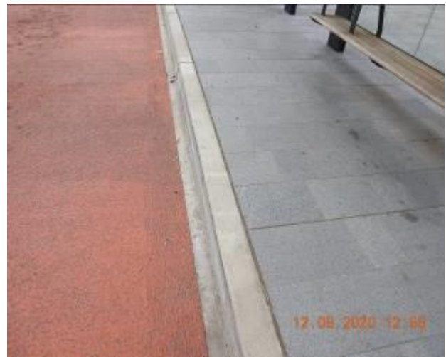
Figure 794 – Hairline crack propagation and evidence of patchwork through kerb
