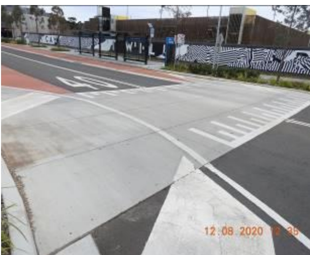
Figure 603 – Paint flaking crack propagation and loss of material through road surface ramp
