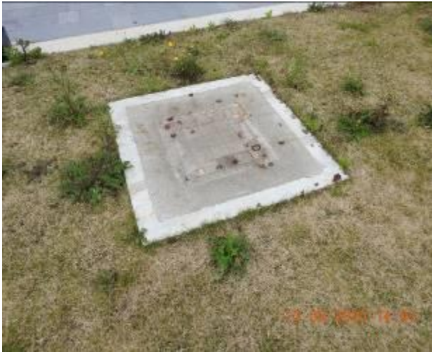
Figure 2189 – Evidence of patchwork through service pit pavement
