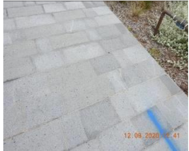
Figure 8 – Hairline cracking and efflorescence through footpath pavement
