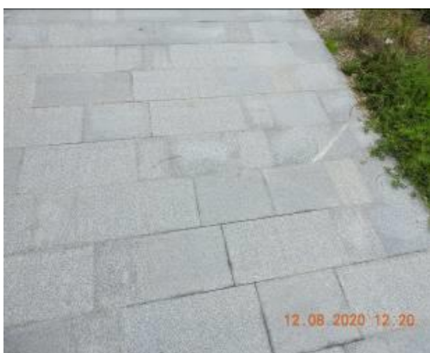
Figure 477 – Efflorescence, crack propagation and loss of material through footpath pavement
