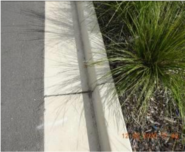
Figure 1703 – Crack propagation and loss of material through kerb and gutter
