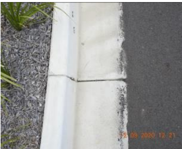
Figure 994 – Crack propagation and loss of material through kerb and gutter
