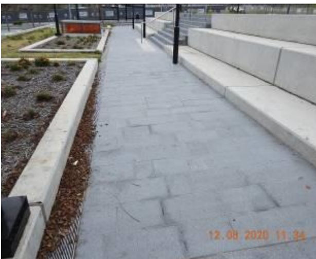
Figure 1617 – Loss of material through showground footpath pavement
