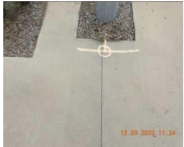
Figure 1080 – Crack propagation and loss of material through footpath pavement
