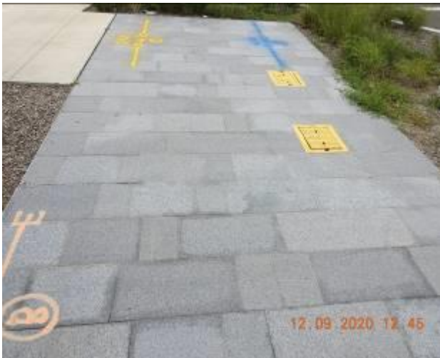
Figure 87 – Hairline cracking and efflorescence through footpath pavement and general condition of service pit
