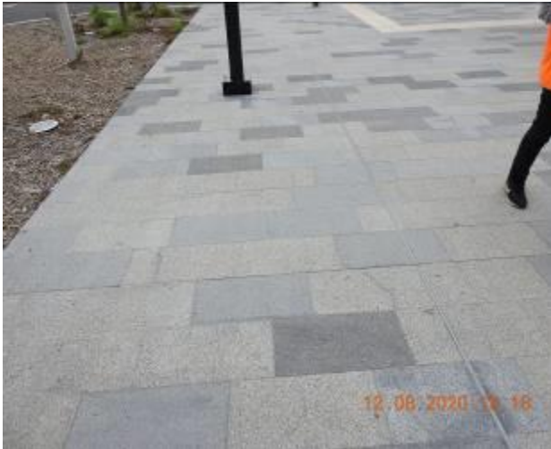
Figure 1936 – Loss of material through floor tiles
