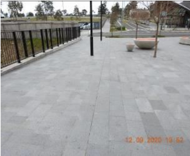
Figure 2450 – Hairline crack propagation through walkway floor
