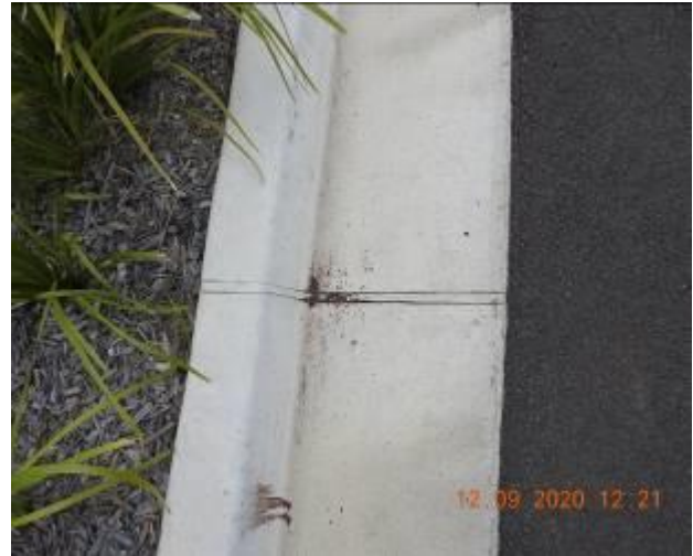
Figure 997 – Crack propagation and loss of material through kerb and gutter
