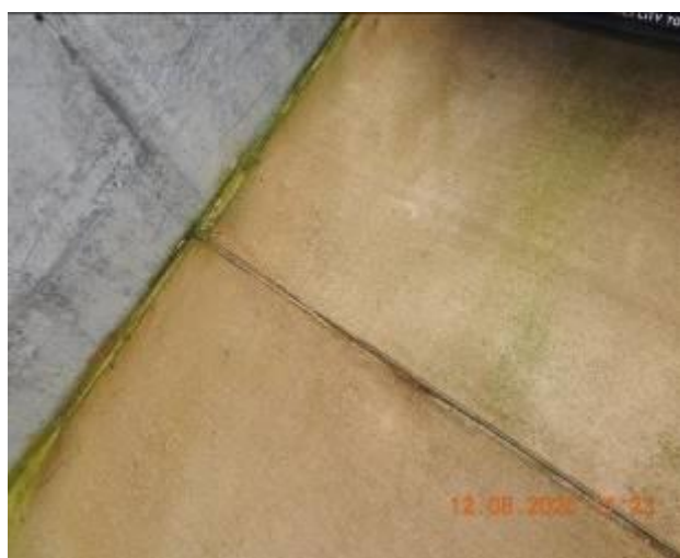
Figure 1533 – Crack propagation and loss of material through footpath pavement
