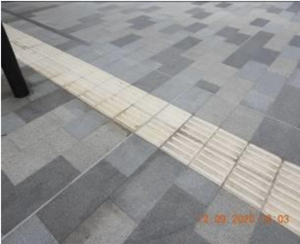
Figure 337 – Hairline cracking and efflorescence through footpath pavement
