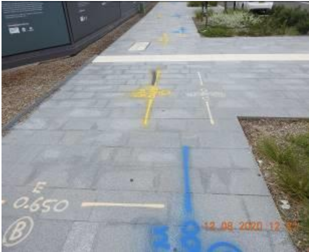
Figure 509 – Loss of material through footpath pavement
