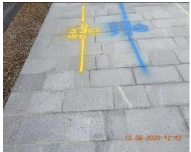
Figure 18 – Hairline cracking and efflorescence through footpath pavement
