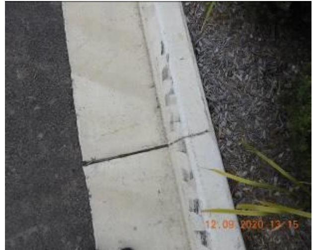
Figure 440 – Crack propagation through kerb
