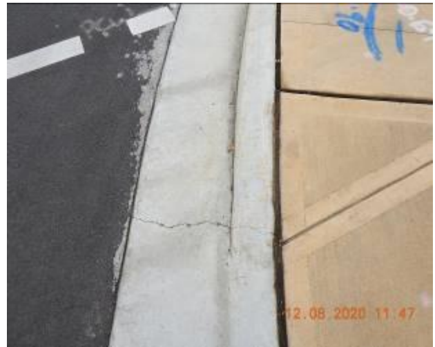
Figure 1688 – Crack propagation and loss of material through layback and gutter
