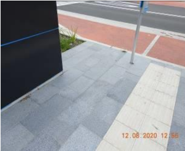
Figure 773 – Hairline crack propagation and loss of material through footpath pavement
