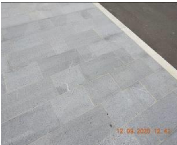
Figure 27 – Hairline cracking and efflorescence through footpath pavement
