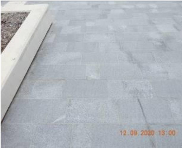
Figure 277 – Hairline cracking and efflorescence through footpath pavement
