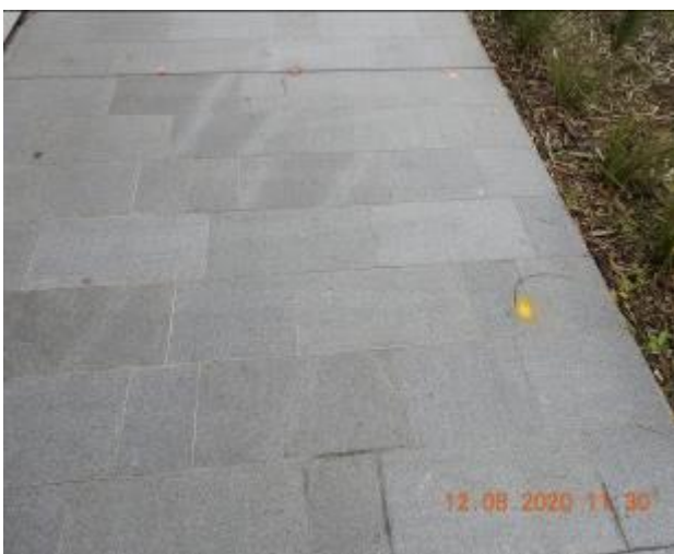
Figure 1587 – Hairline crack propagation through footpath pavement
