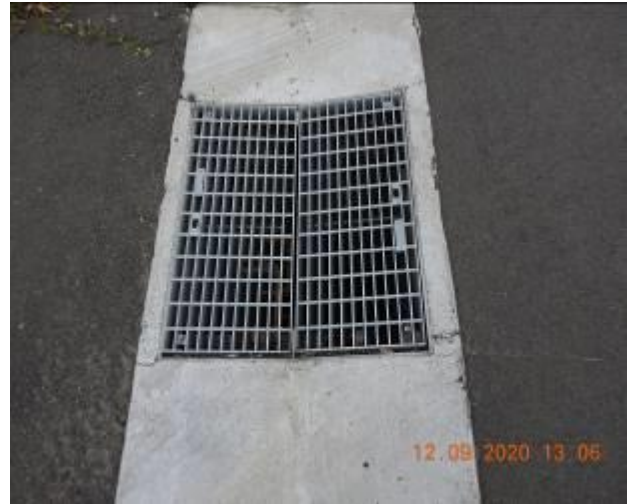
Figure 398 – Crack propagation through gutter and General condition of stormwater inlet pit
