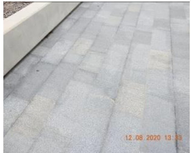
Figure 2029 – Crack propagation and loss of material through floor tiles
