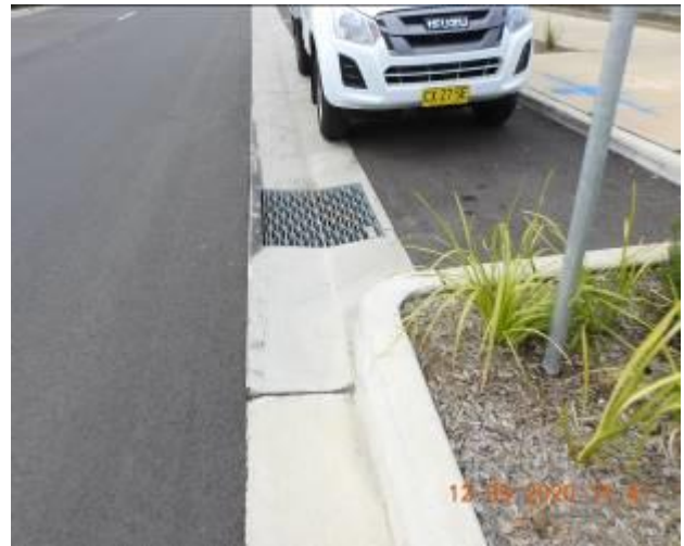
Figure 1314 – Loss of material through gutter
