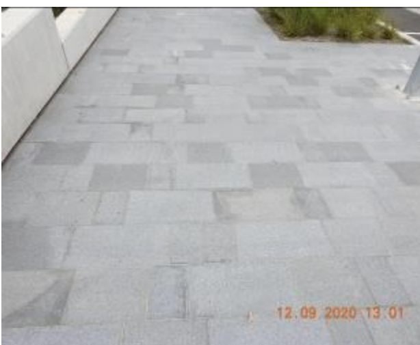
Figure 305 – Hairline cracking and efflorescence through footpath pavement
