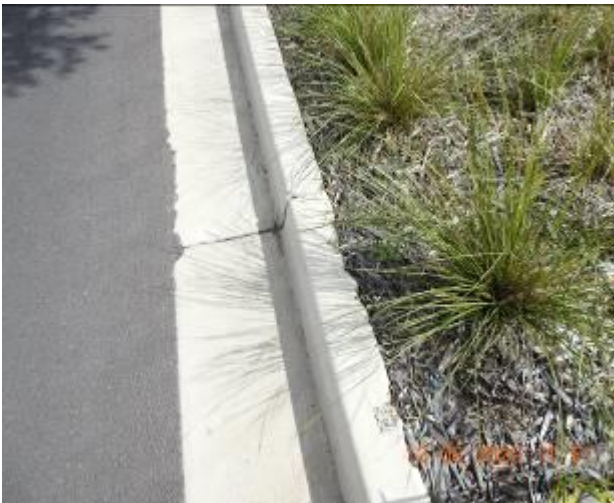
Figure 1723 – Crack propagation and loss of material through kerb and gutter
