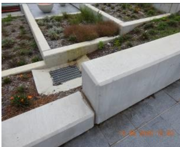
Figure 2103 – Crack propagation through retaining wall
