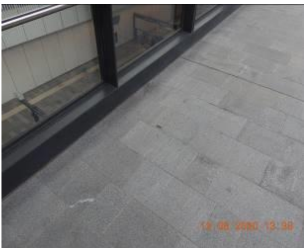
Figure 2072 – Efflorescence and loss of material through floor tiles
