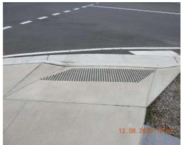
Figure 782 – Crack propagation and loss of material through footpath pavement
