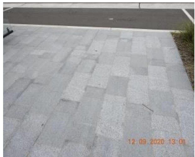
Figure 292 – Hairline cracking and efflorescence through footpath pavement
