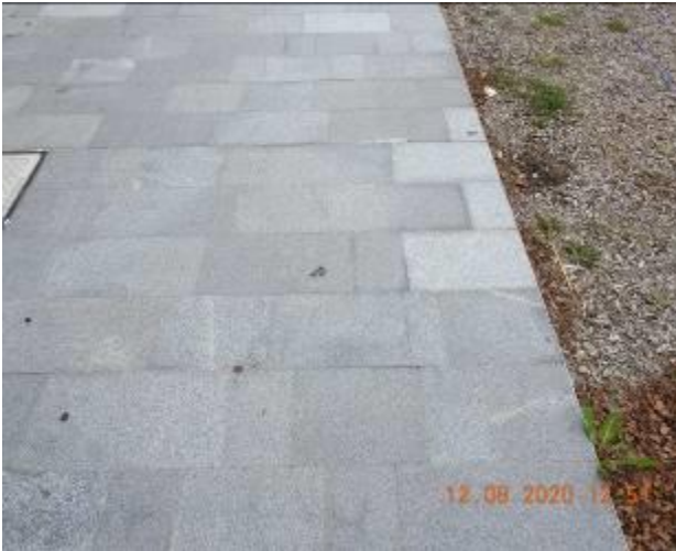
Figure 707 – Efflorescence, crack propagation and loss of material through footpath pavement
