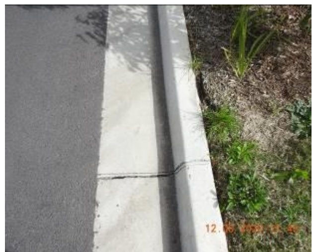
Figure 1678 – Crack propagation and loss of material through kerb and gutter
