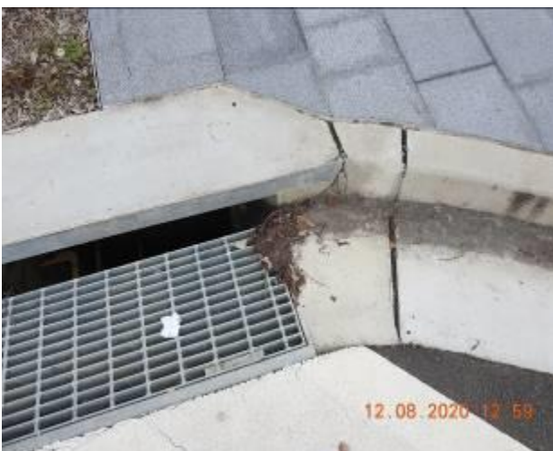
Figure 819 – Crack propagation and loss of material through kerb and gutter
