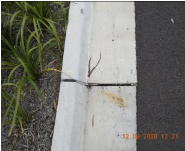
Figure 1004 – Loss of material through kerb and gutter
