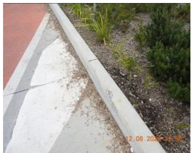
Figure 790 – Crack propagation and loss of material through kerb
