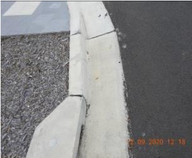
Figure 954 – Crack propagation and loss of material through kerb
