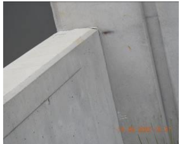
Figure 2393 – Crack propagation and loss of material through retaining wall
