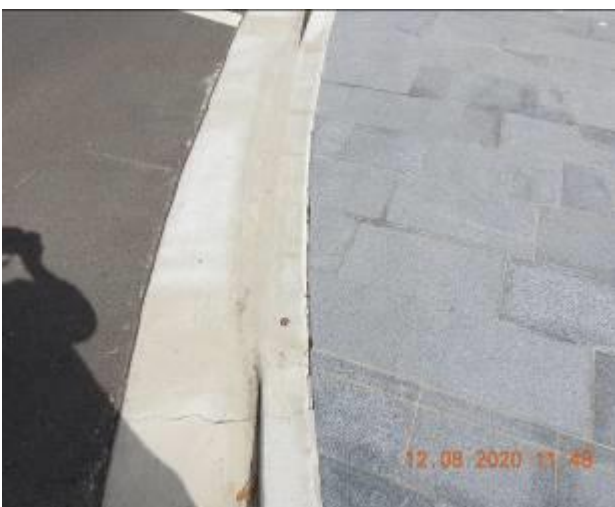
Figure 1695 – Crack propagation and loss of material through layback and gutter
