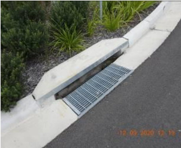
Figure 960 – General condition of stormwater inlet pit/Loss of material through kerb
