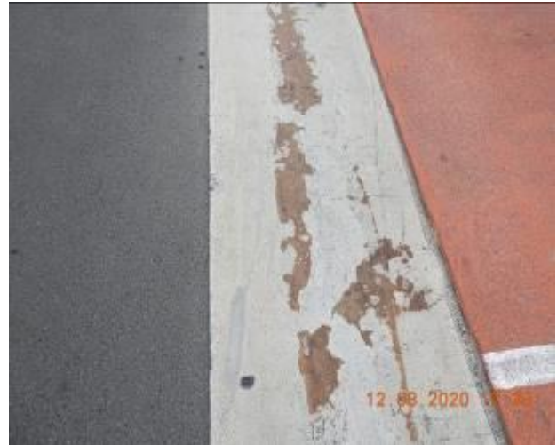
Figure 612 – Hairline crack propagation and evidence of patchwork through road surface
