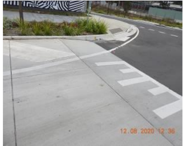
Figure 606 – Loss of material through road surface ramp
