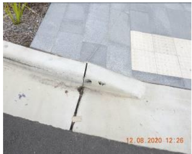
Figure 556 – Separation through kerb and gutter
