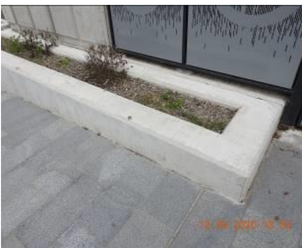
Figure 2364 – Crack propagation and loss of material through retaining wall
