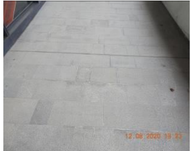
Figure 1961 – Efflorescence through floor tiles
