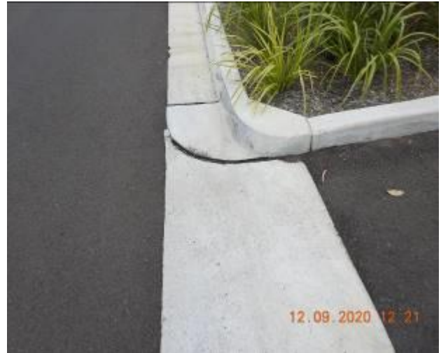
Figure 991 – Loss of material through gutter
