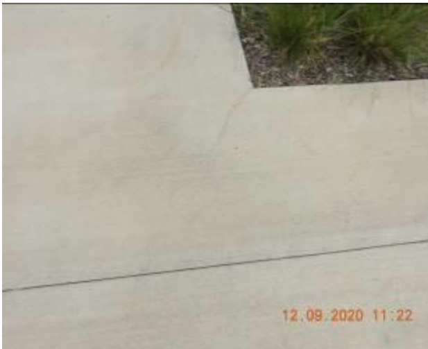
Figure 1067 – Hairline crack propagation through footpath pavement
