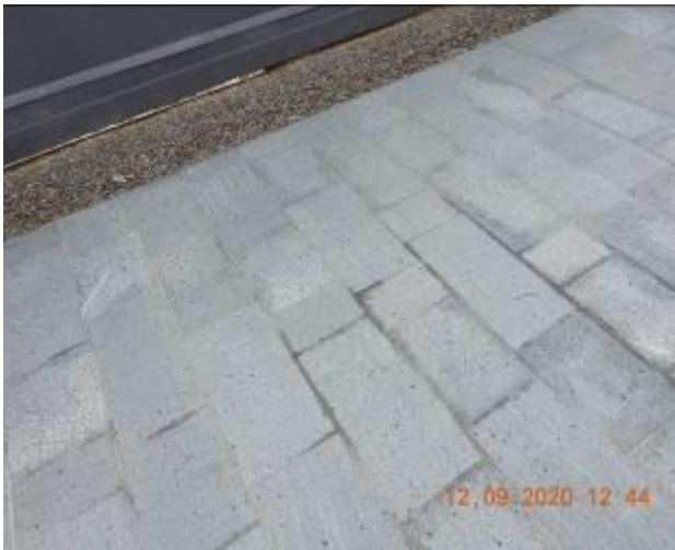
Figure 69 – Hairline cracking and efflorescence through footpath pavement
