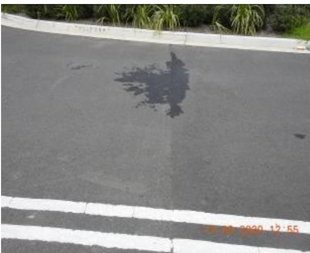
Figure 227 – Loss of material through road surface lines
