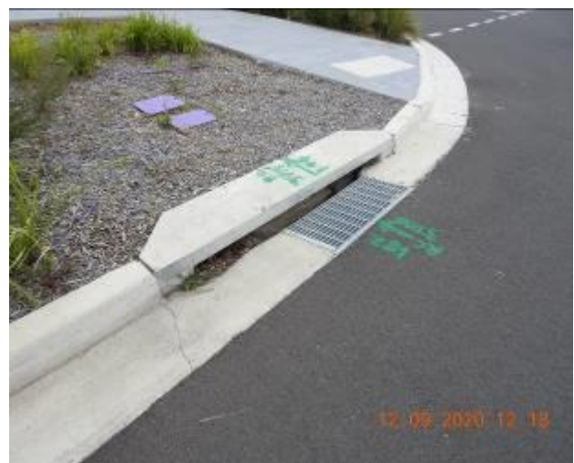
Figure 953 – General condition of stormwater inlet pit/Crack propagation and loss of material through kerb and gutter
