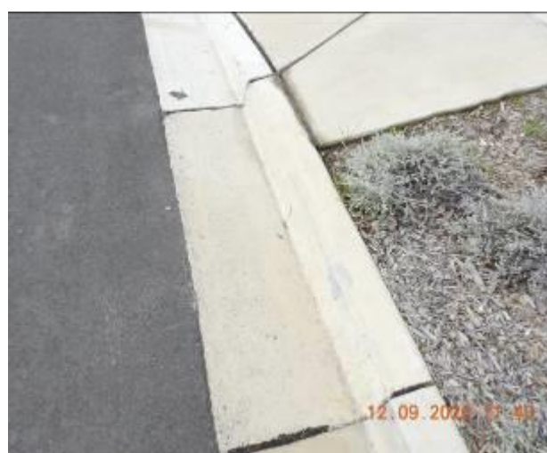
Figure 1292 – Evidence of patchwork and loss of material through kerb and gutter
