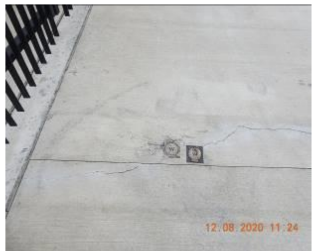
Figure 1540 – General condition of service pits/ Crack propagation and loss of material through driveway pavement
