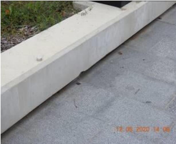
Figure 2255 – Loss of material through retaining wall
