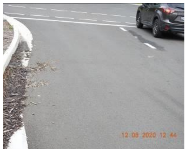
Figure 676 – Loss of material through road surface
