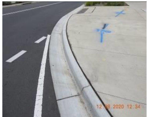
Figure 598 – Crack propagation and loss of material through kerb
