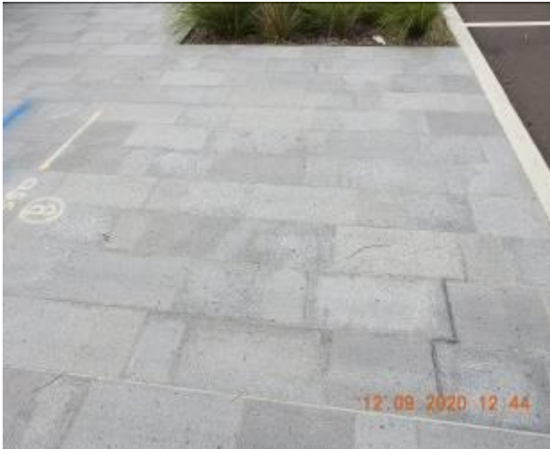
Figure 61 – Hairline cracking and efflorescence through footpath pavement
