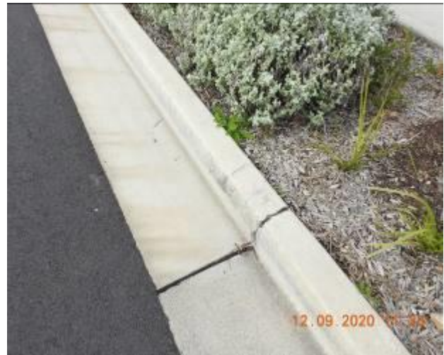
Figure 1260 – Crack propagation and loss of material through curb and gutter
