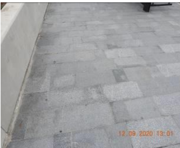
Figure 291 – Hairline cracking and efflorescence through footpath pavement
