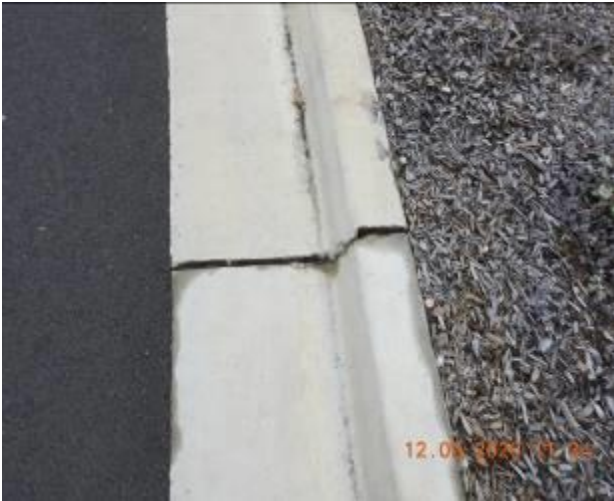
Figure 1185 – Loss of material through kerb and gutter
