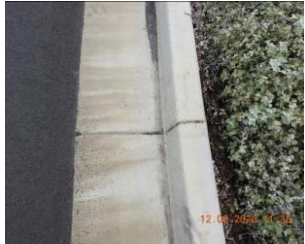
Figure 1210 – Crack propagation and loss of material through kerb
