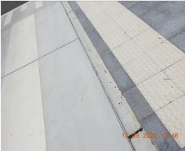
Figure 97 – Crack propagation through layback
