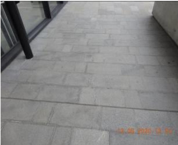
Figure 1968 – Efflorescence through floor tiles
