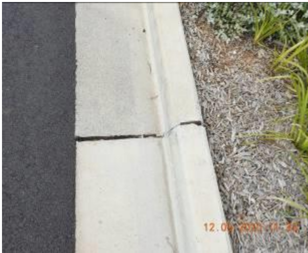
Figure 1257 – Loss of material through curb and gutter
