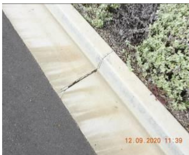
Figure 1285 – Loss of material through kerb and gutter
