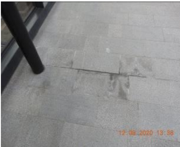
Figure 2070 – Loss of material through floor tiles
