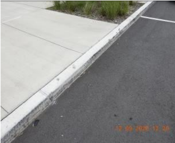
Figure 978 – Loss of material through kerb
