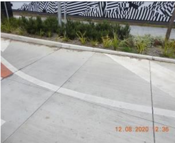
Figure 607 – Loss of material through road surface ramp
