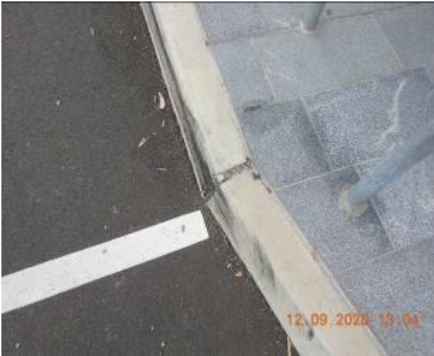
Figure 355 – Crack propagation and loss of material through kerb
