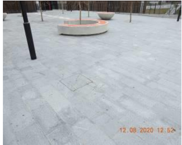
Figure 720 – Efflorescence, hairline crack propagation and loss of material through footpath pavement
