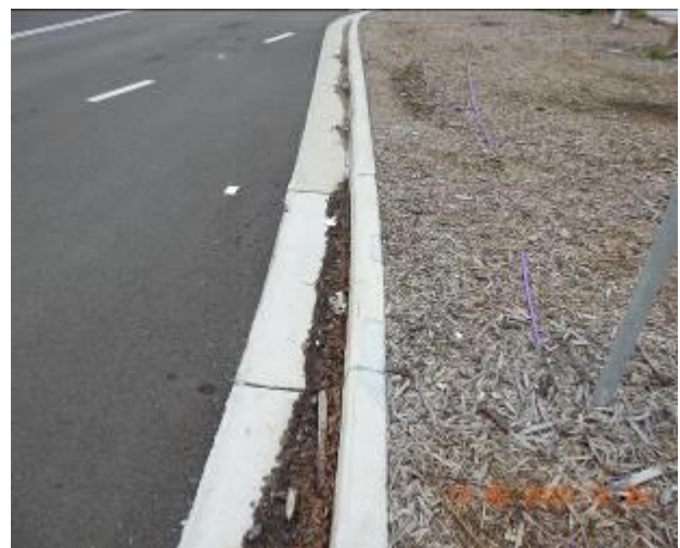
Figure 544 – Loss of material and loss of material through kerb and gutter
