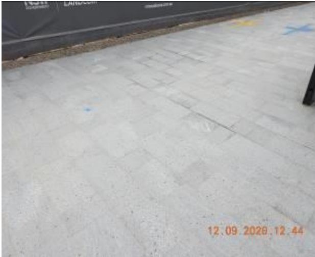
Figure 67 – Hairline cracking and efflorescence through footpath pavement
