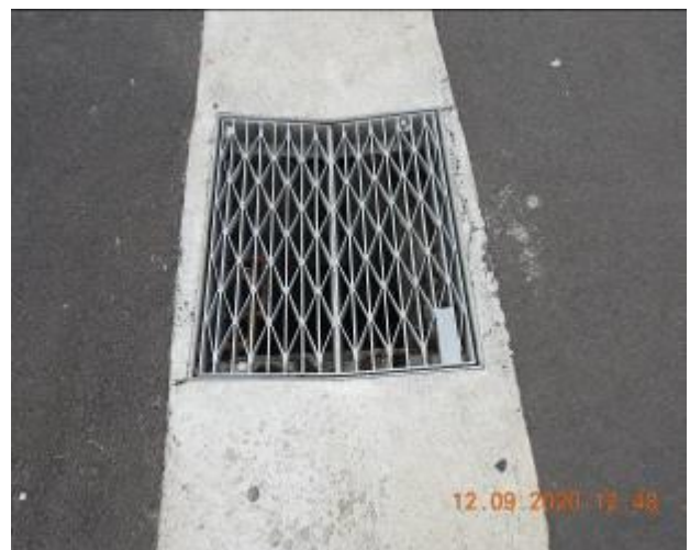
Figure 156 – General condition of stormwater inlet pit and crack propagation through gutter
