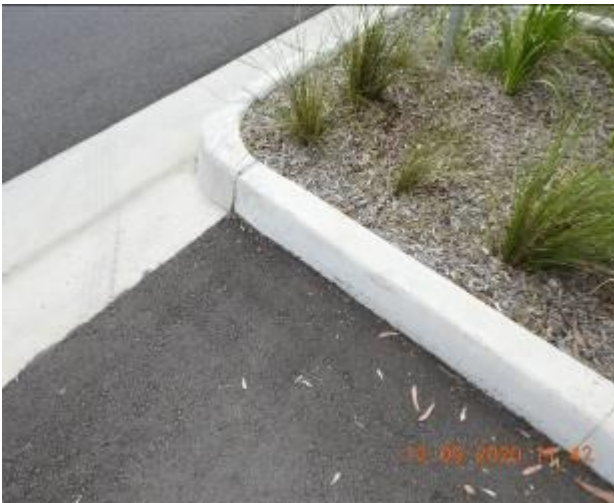
Figure 1325 – Loss of material through kerb
