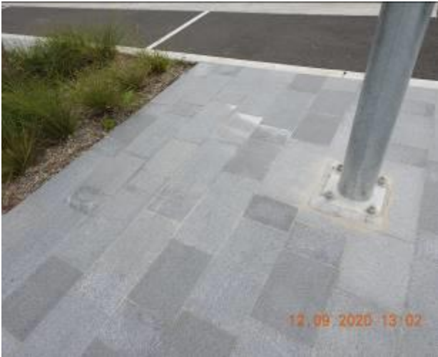
Figure 307 – Hairline cracking and efflorescence through footpath pavement
