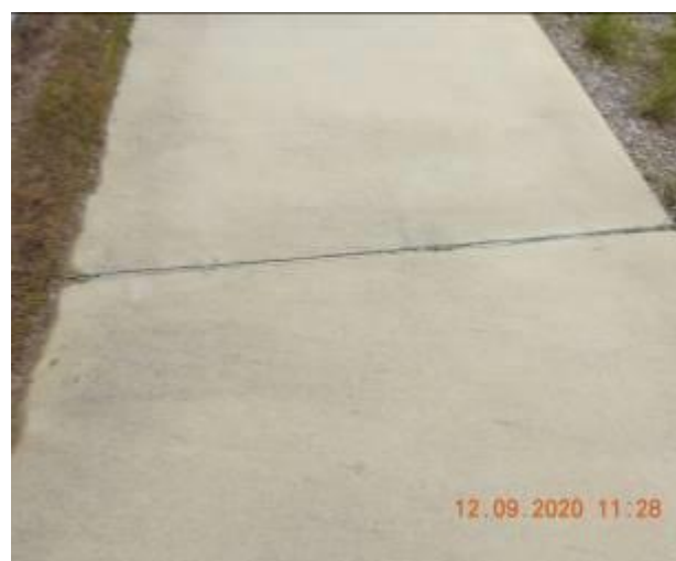
Figure 1124 – Loss of material through footpath pavement
