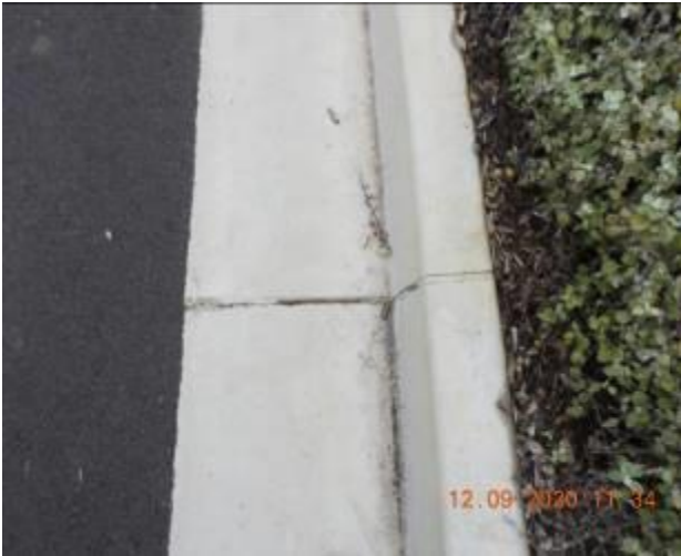
Figure 1191 – Loss of material through kerb and gutter
