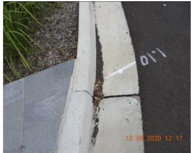
Figure 939 – Evidence of patchwork, crack propagation and loss of material through kerb and gutter
