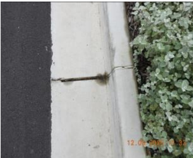
Figure 1181 – Crack propagation and loss of material through kerb and gutter
