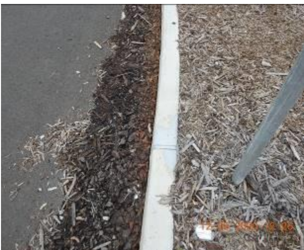
Figure 543 – Loss of material and crack propagation through kerb
