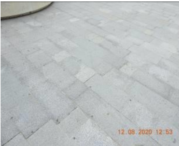
Figure 727 – Efflorescence, hairline crack propagation and loss of material through footpath pavement
