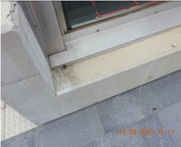
Figure 2273 – Loss of material through retaining wall
