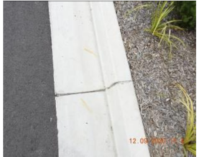
Figure 1312 – Crack propagation and loss of material through kerb and gutter
