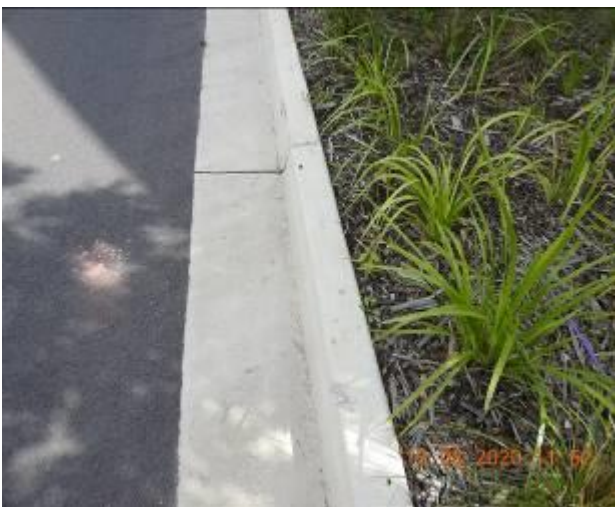
Figure 1731 – Evidence of patchwork through kerb
