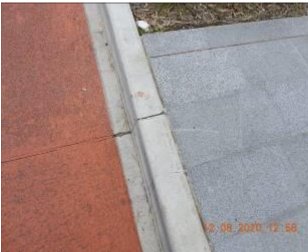
Figure 799 – Evidence of patchwork, crack propagation and loss of material through kerb
