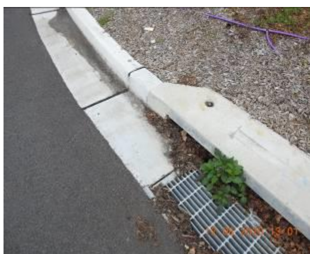
Figure 843 – Loss of material through gutter
