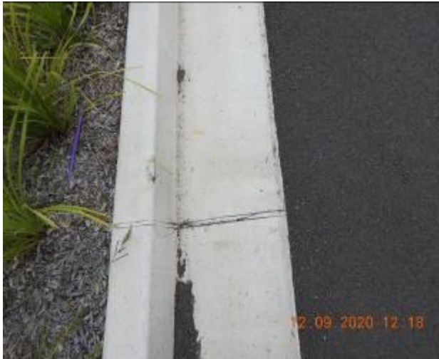
Figure 948 – Crack propagation and loss of material through kerb and gutter
