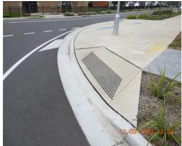
Figure 596 – Loss of material through layback
