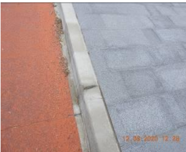
Figure 579 – Evidence of patchwork, hairline crack propagation and loss of material through kerb
