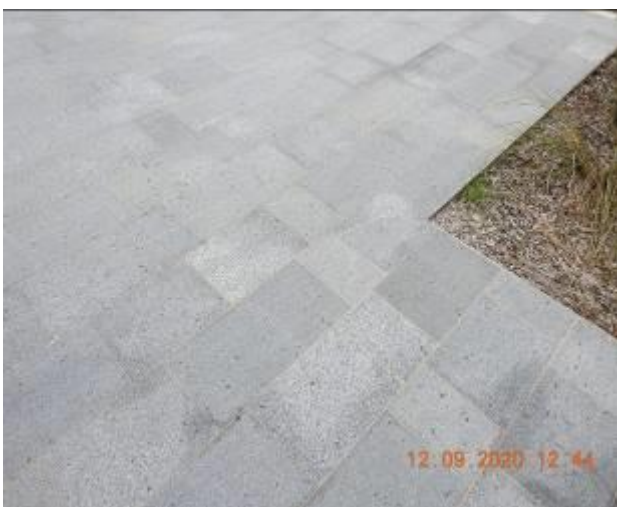
Figure 65 – Hairline cracking and efflorescence through footpath pavement
