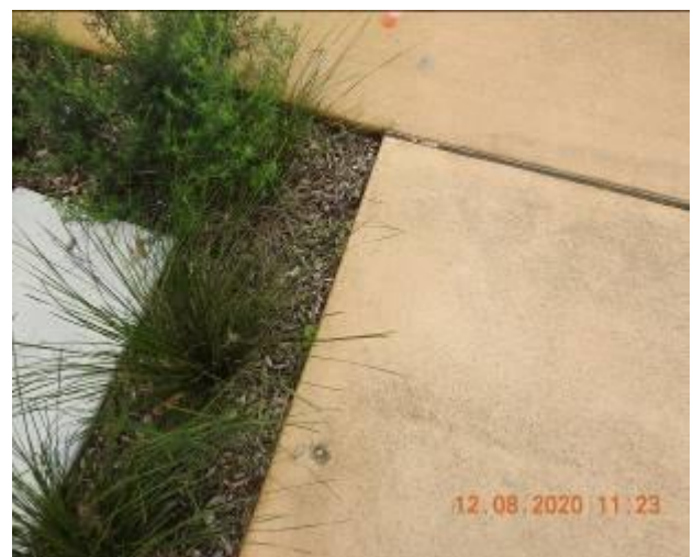
Figure 1528 – Loss of material through footpath pavement
