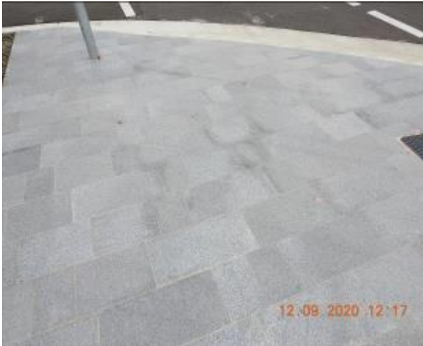
Figure 930 – Hairline crack propagation through footpath pavement
