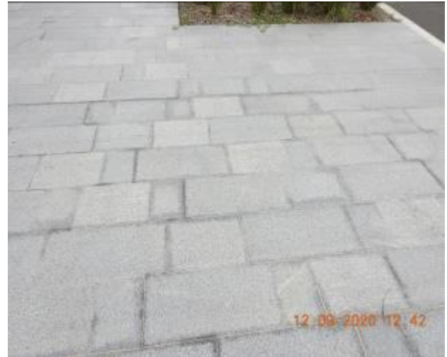
Figure 32 – Hairline cracking and efflorescence through footpath pavement
