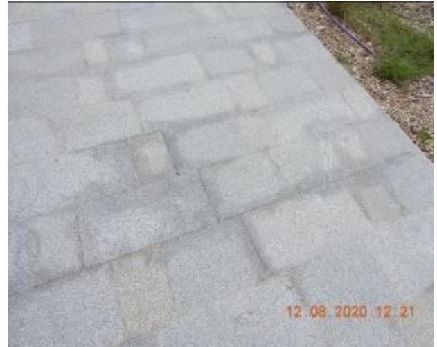
Figure 498 – Loss of material through footpath pavement
