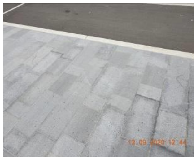
Figure 60 – Hairline cracking and efflorescence through footpath pavement
