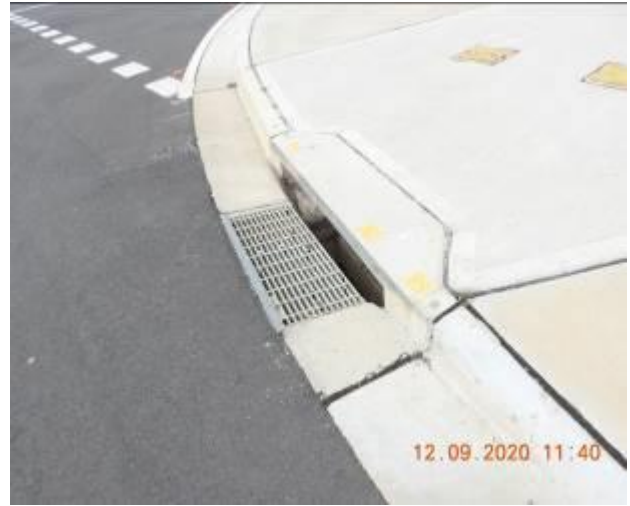
Figure 1294 – General condition of stormwater inlet pit/Crack propagation and loss of material through kerb and gutter
