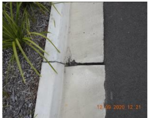
Figure 995 – Loss of material through kerb
