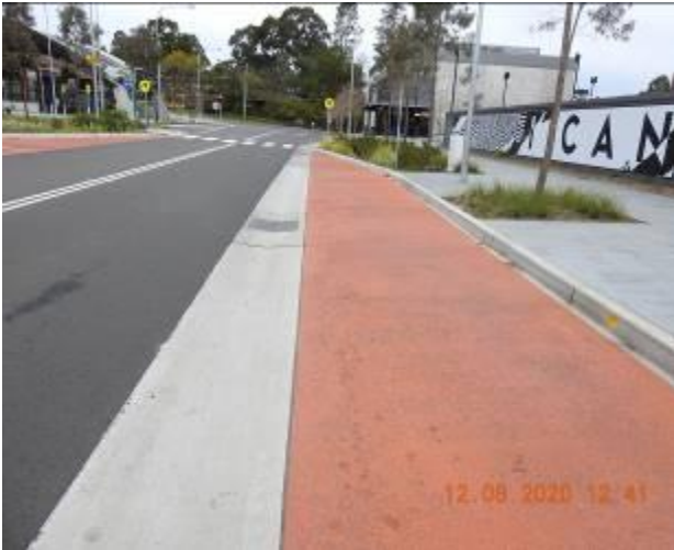
Figure 635 – Evidence of patchwork and loss of material through road surface
