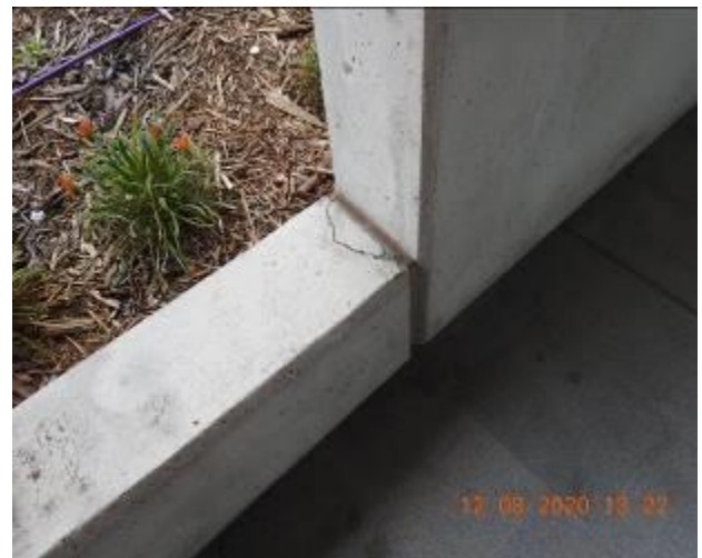
Figure 1947 – Crack propagation and loss of material through retaining wall
