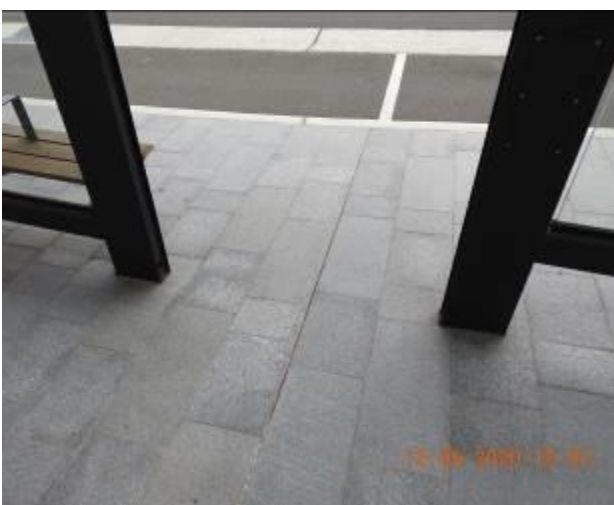
Figure 317 – Hairline cracking and efflorescence through footpath pavement
