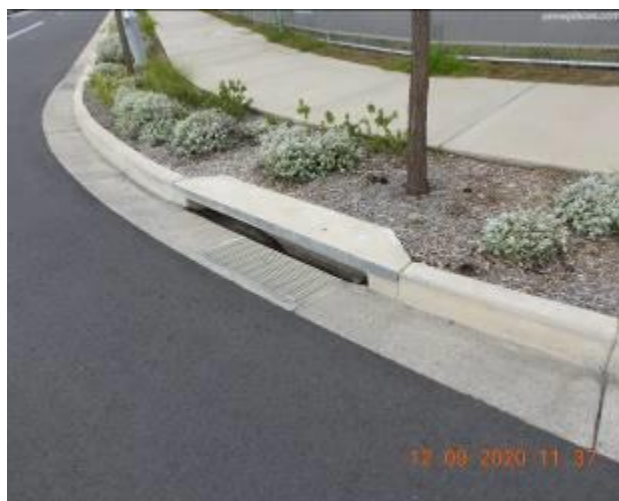
Figure 1235 – Crack propagation and loss of material through kerb and gutter/General condition of stormwater inlet pit
