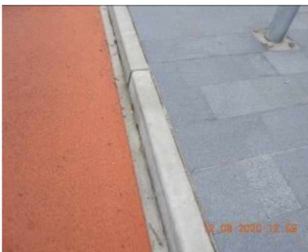
Figure 807 – Hairline crack propagation and evidence of patchwork through kerb
