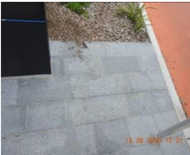
Figure 495 – Crack propagation and loss of material through footpath pavement
