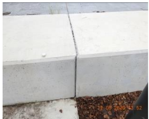
Figure 2116 – Separation through retaining wall
