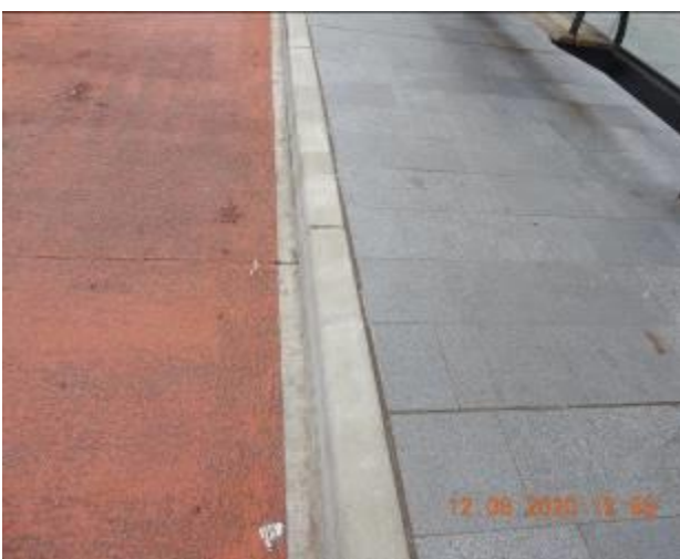
Figure 795 – Hairline crack propagation and evidence of patchwork through kerb
