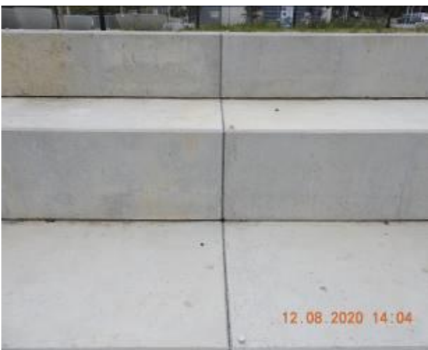
Figure 2205 – Separation through retaining wall
