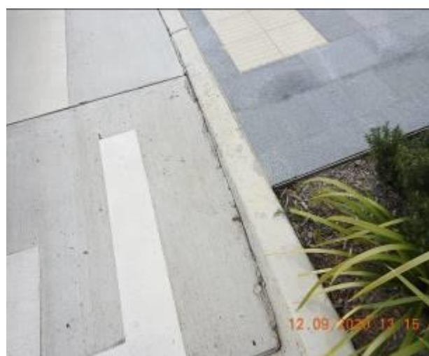
Figure 432 – Crack propagation and loss of material through layback
