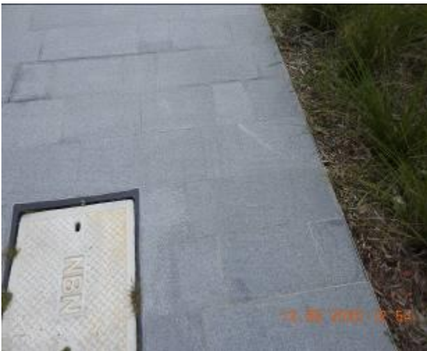
Figure 745 – Crack propagation and loss of material through footpath pavement
