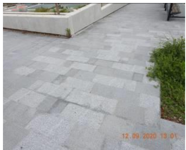
Figure 288 – Hairline cracking and efflorescence through footpath pavement
