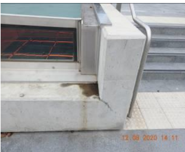
Figure 2277 – Crack propagation through retaining wall
