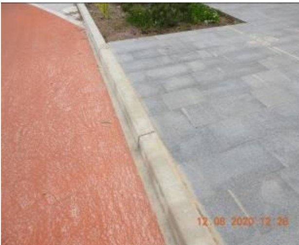
Figure 589 – Evidence of patchwork and hairline cracking through kerb
