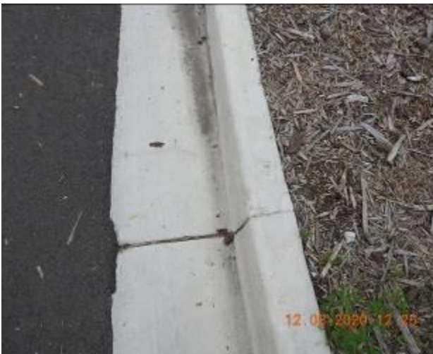
Figure 541 – Evidence of patchwork, crack propagation and loss of material through kerb and gutter
