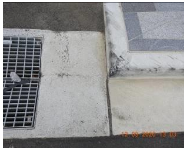
Figure 348 – Crack propagation through kerb
