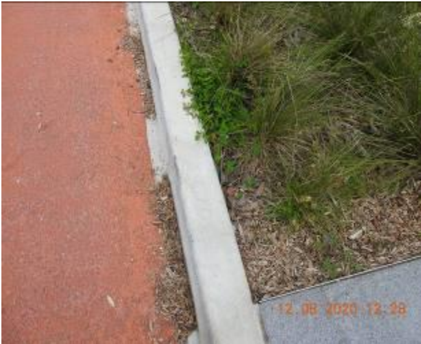
Figure 581 – Evidence of patchwork and hairline crack propagation through kerb
