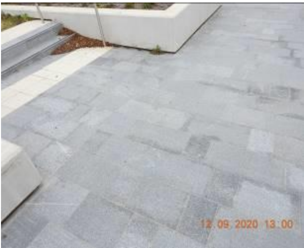
Figure 279 – Hairline cracking and efflorescence through footpath pavement
