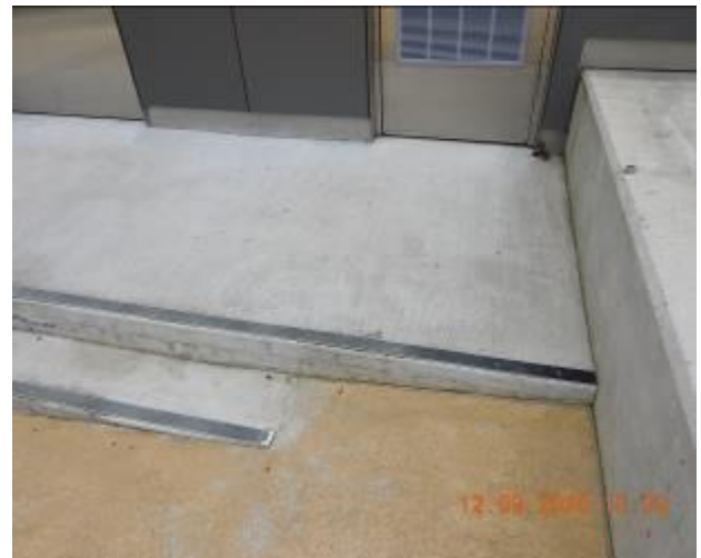
Figure 2405 – Loss of material through steps pavement
