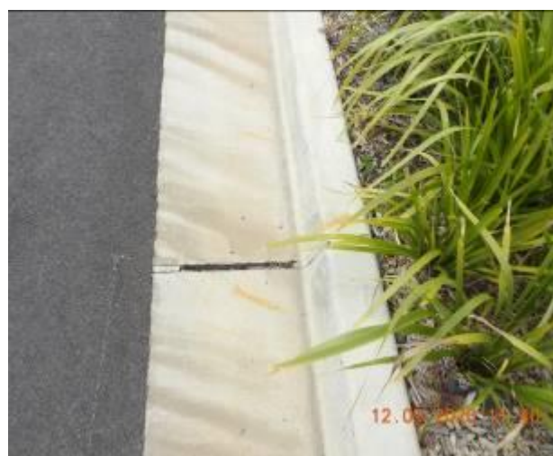
Figure 1290 – Loss of material through kerb and gutter
