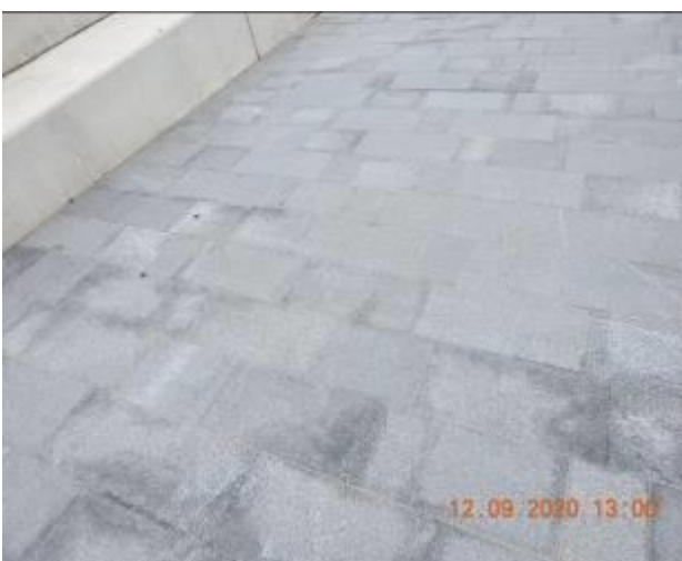
Figure 263 – Hairline cracking and efflorescence through footpath pavement
