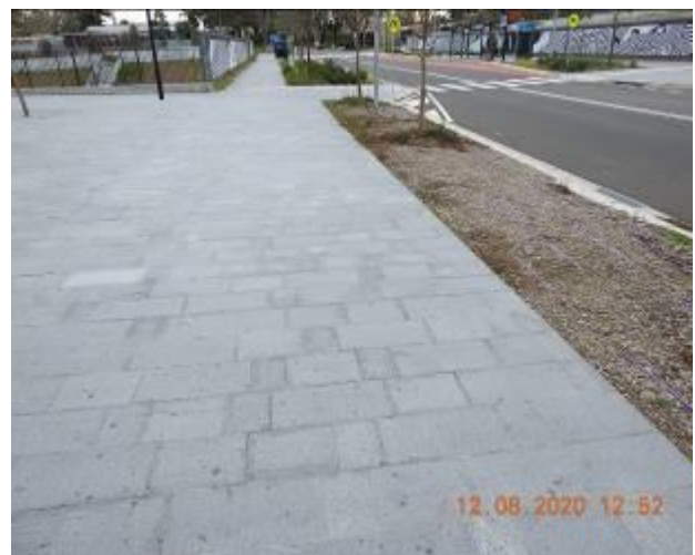
Figure 718 – Efflorescence, hairline crack propagation and loss of material through footpath pavement
