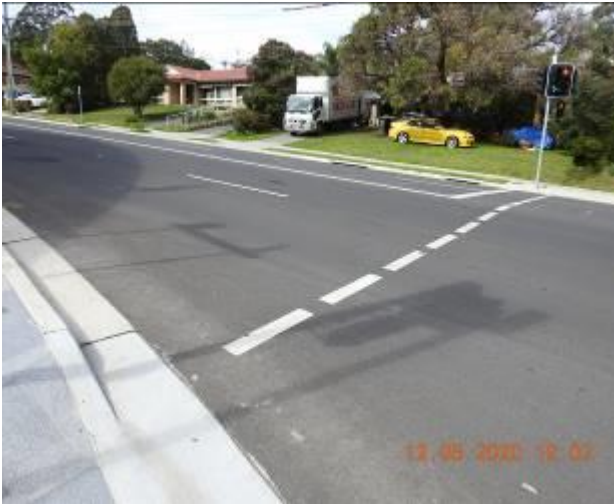
Figure 1835 – Evidence of patchwork through road surface
