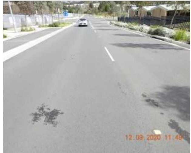
Figure 1396 – Loss of material through road surface
