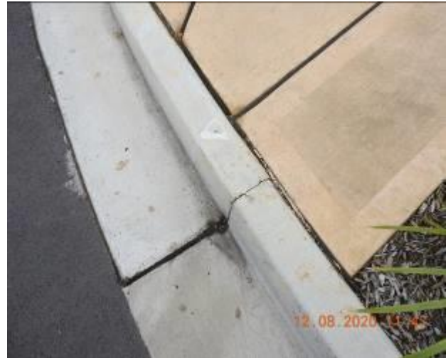
Figure 1686 – Crack propagation and loss of material through kerb and gutter
