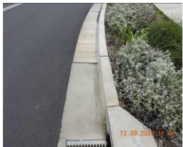
Figure 1208 – Loss of material through kerb
