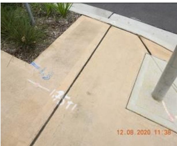
Figure 1653 – Crack propagation and loss of material through footpath pavement
