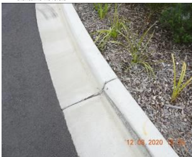
Figure 557 – Crack propagation and loss of material through kerb and gutter
