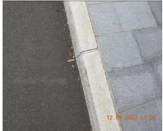
Figure 392 – Crack propagation through kerb
