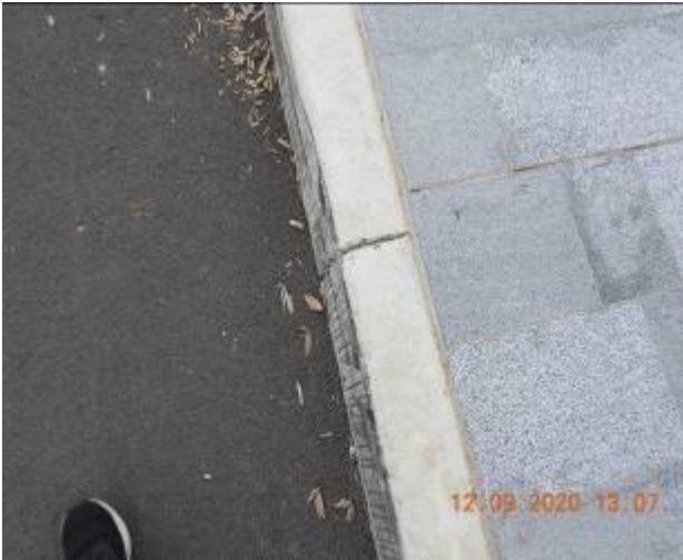
Figure 403 – Crack propagation through kerb
