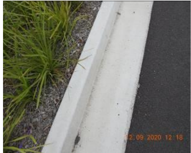
Figure 949 – Hairline Crack propagation through kerb and gutter
