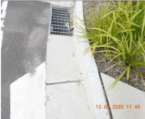
Figure 1299 – Crack propagation through kerb
