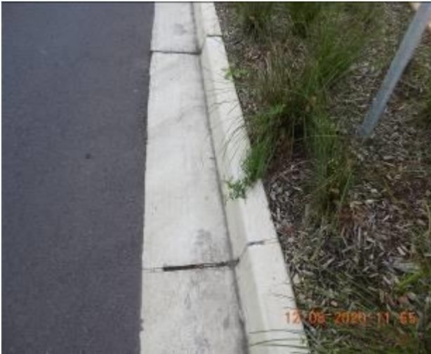
Figure 1763 – Crack propagation and loss of material through kerb and gutter
