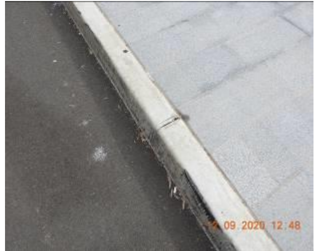
Figure 140 – Crack propagation and loss of material through kerb
