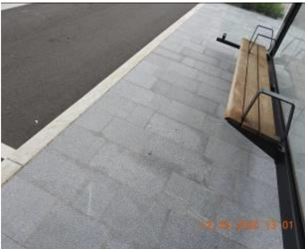
Figure 297 – Hairline cracking and efflorescence through footpath pavement
