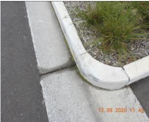
Figure 1355 – Evidence of patchwork, crack propagation and loss of material through kerb and gutter
