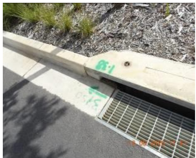
Figure 1720 – Loss of material through kerb
