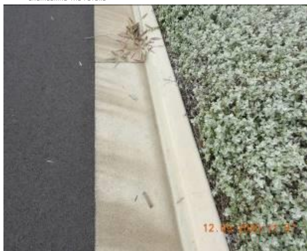
Figure 1245 – Crack propagation through kerb
