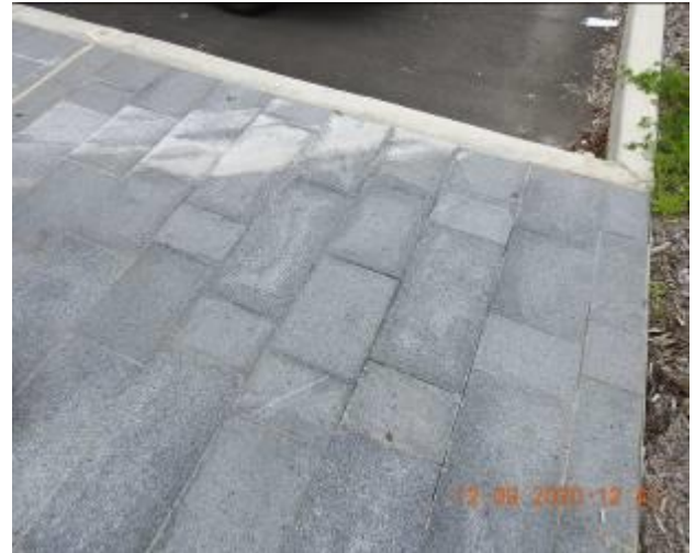
Figure 14 – Hairline cracking and efflorescence through footpath pavement
