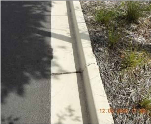
Figure 1709 – Loss of material through kerb and gutter
