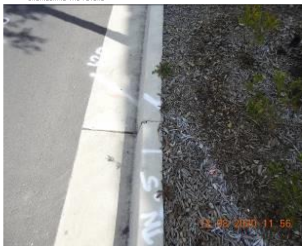
Figure 1787 – Crack propagation and loss of material through kerb and gutter
