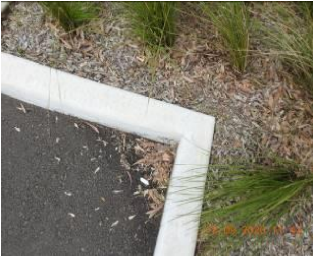
Figure 1335 – Crack propagation through kerb
