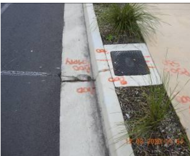
Figure 1761 – Evidence of patchwork through gutter and Loss of material through kerb and gutter
