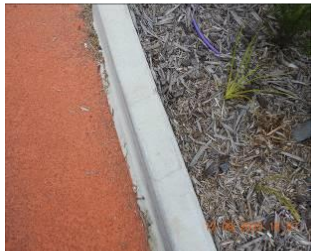
Figure 566 – Evidence of patchwork through kerb
