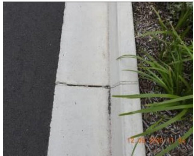
Figure 1194 – Loss of material through kerb and gutter
