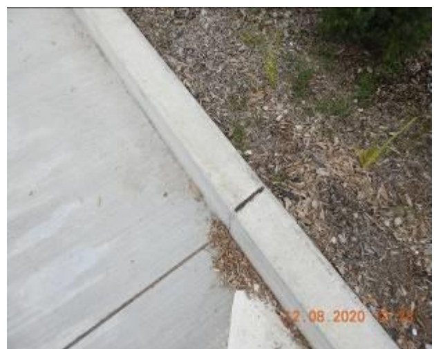
Figure 592 – Crack propagation and loss of material through kerb
