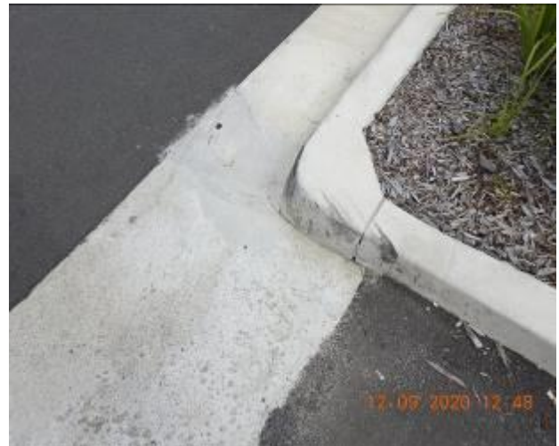
Figure 154 – Evidence of patchwork and crack propagation through gutter
