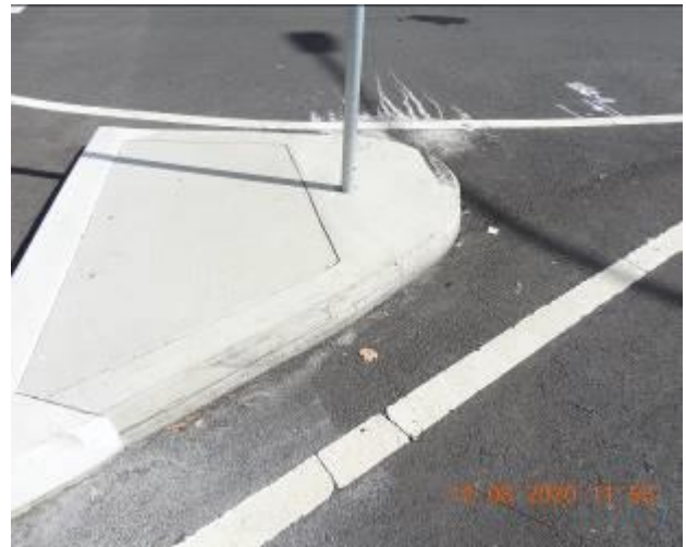
Figure 1808 – Loss of material through traffic island pavement/Crack propagation and loss of material through road surface
