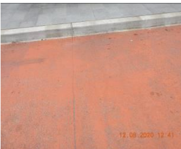
Figure 639 – Crack propagation and loss of material through road surface
