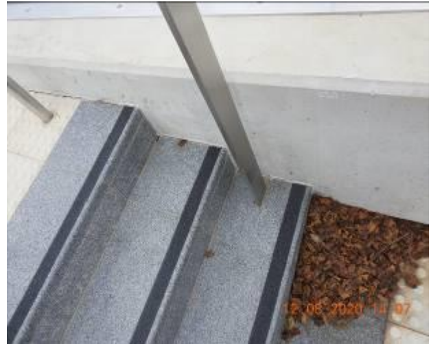
Figure 2232 – Separation through staircase floor
