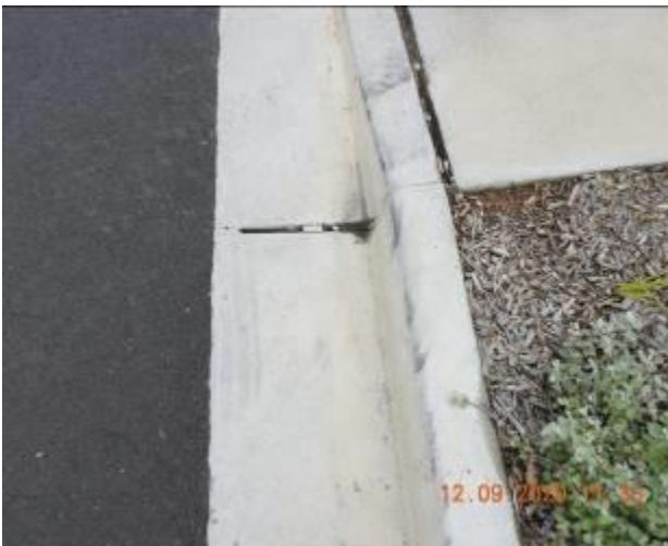
Figure 1175 – Crack propagation and loss of material through kerbs and gutter
