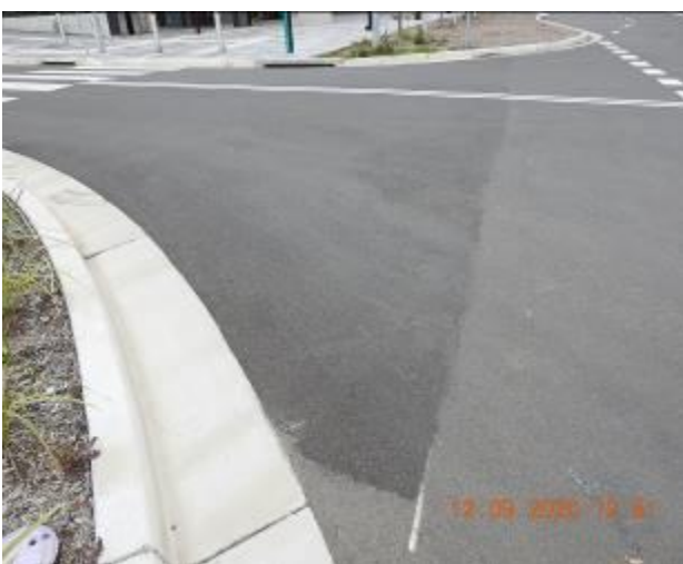
Figure 185 – Loss of material through road surface
