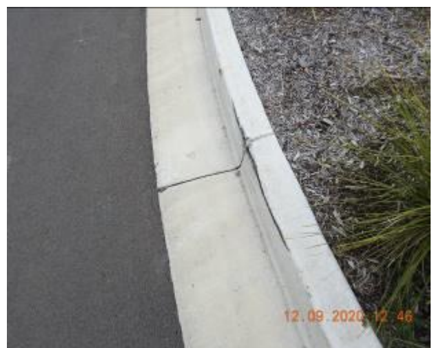
Figure 90 – Loss of material through kerb and gutter
