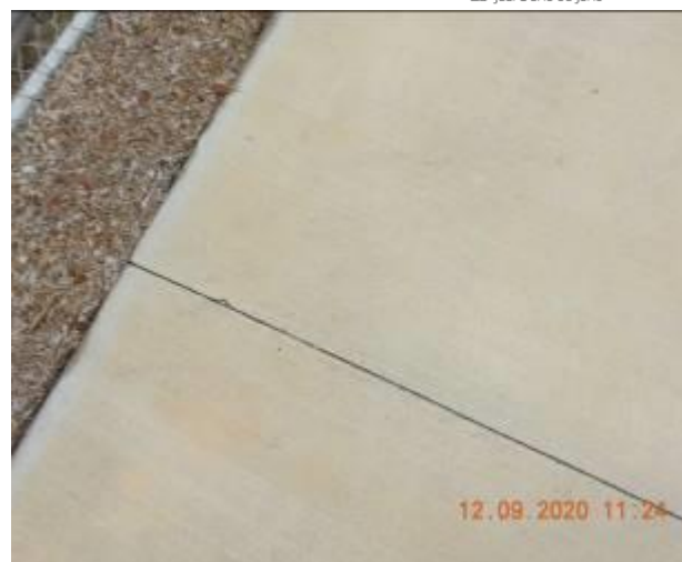
Figure 1084 – Loss of material through footpath pavement
