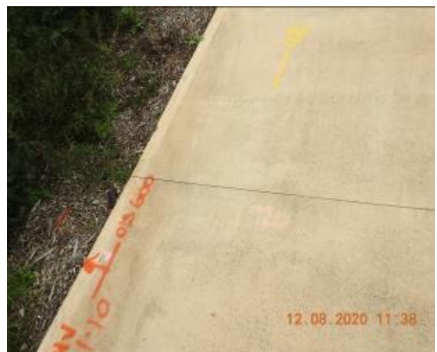
Figure 1654 – Separation through footpath pavement
