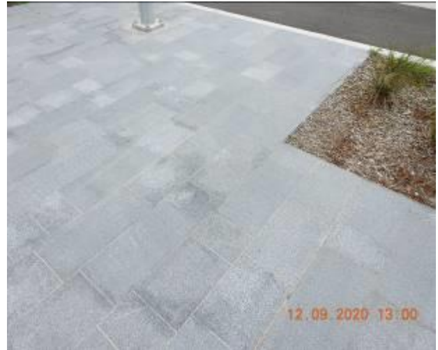
Figure 278 – Hairline cracking and efflorescence through footpath pavement
