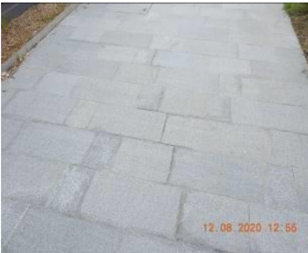
Figure 751 – Crack propagation and loss of material through footpath pavement
