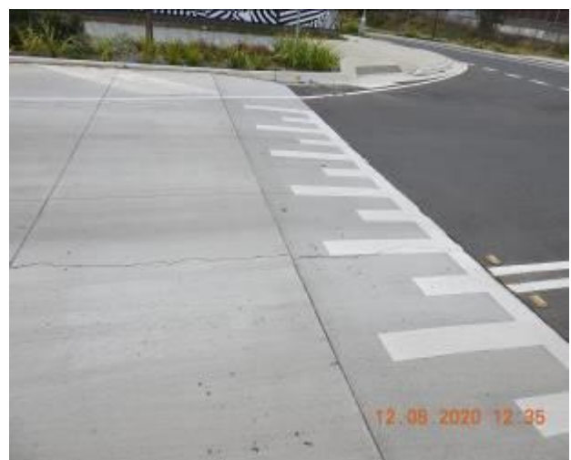
Figure 604 – Crack propagation and loss of material through road surface ramp
