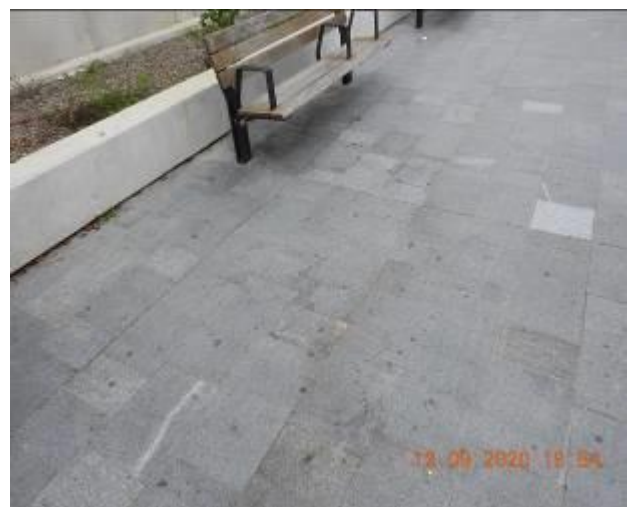
Figure 2497 – Hairline crack propagation through walkway floor
