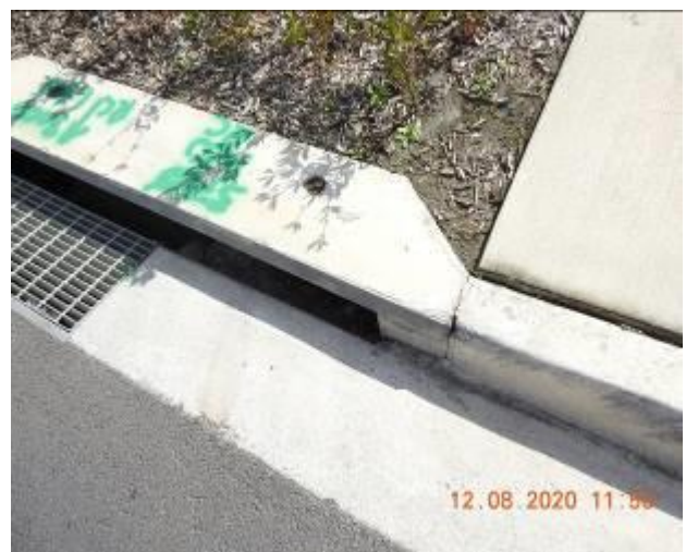
Figure 1780 – Crack propagation and loss of material through curb
