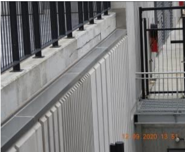
Figure 2440 – Loss of material through external wall
