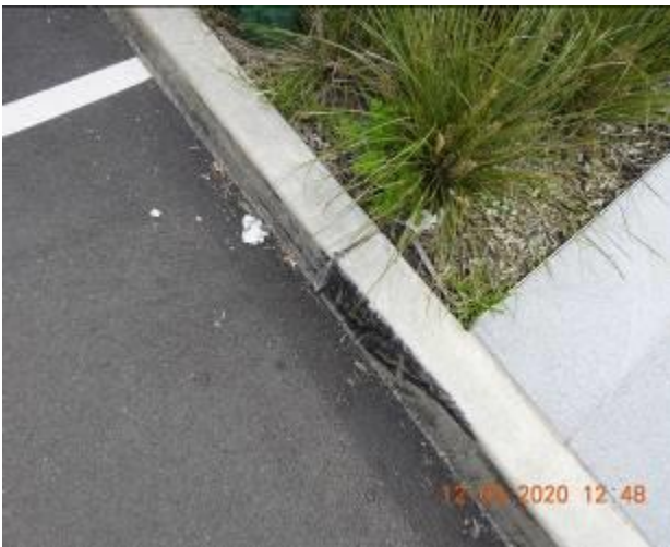
Figure 141 – Crack propagation through kerb
