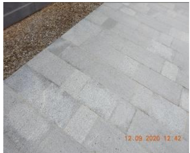
Figure 34 – Hairline cracking and efflorescence through footpath pavement
