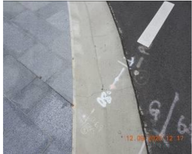
Figure 937 – Crack propagation and loss of material through layback and gutter
