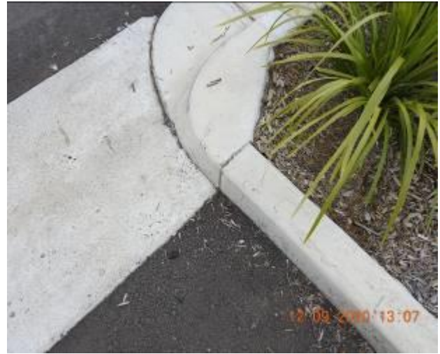
Figure 416 – Crack propagation through kerb
