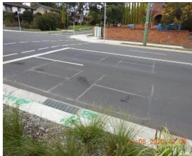
Figure 1848 – Evidence of patchwork and loss of material through road surface
