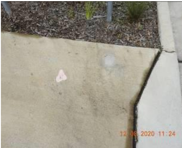
Figure 1543 – Evidence of patchwork through driveway pavement
