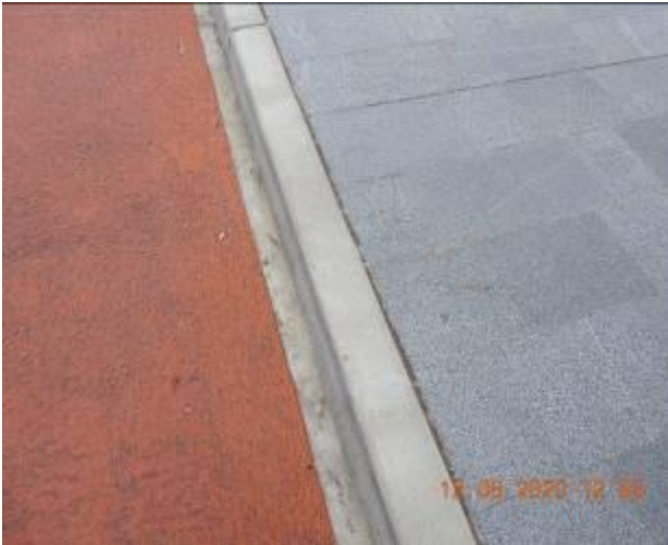
Figure 797 – Hairline crack propagation and evidence of patchwork through kerb
