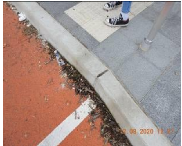
Figure 572 – Evidence of patchwork crack propagation and loss of material through kerb
