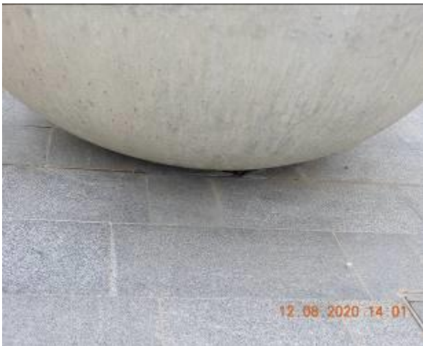
Figure 2161 – Loss of material through walkway floor
