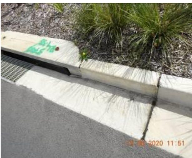
Figure 1719 – Crack propagation and loss of material through kerb and gutter
