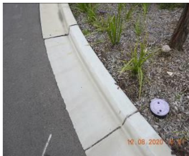
Figure 560 – Crack propagation and loss of material through kerb and gutter
