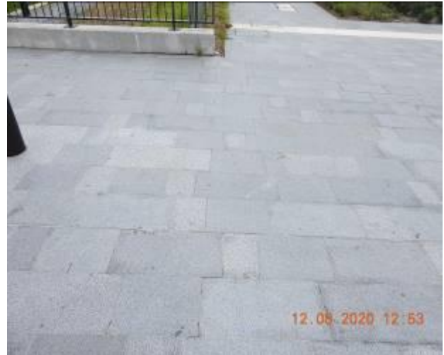
Figure 732 – Efflorescence, hairline crack propagation and loss of material through footpath pavement
