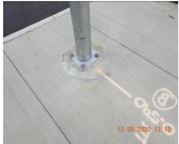
Figure 883 – Crack propagation through footpath pavement
