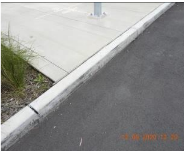
Figure 982 – Loss of material through kerb
