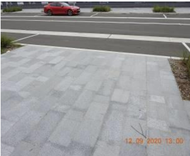
Figure 285 – Hairline cracking and efflorescence through footpath pavement
