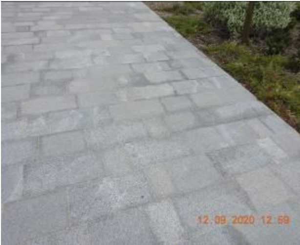
Figure 253 – Hairline cracking and efflorescence through footpath pavement
