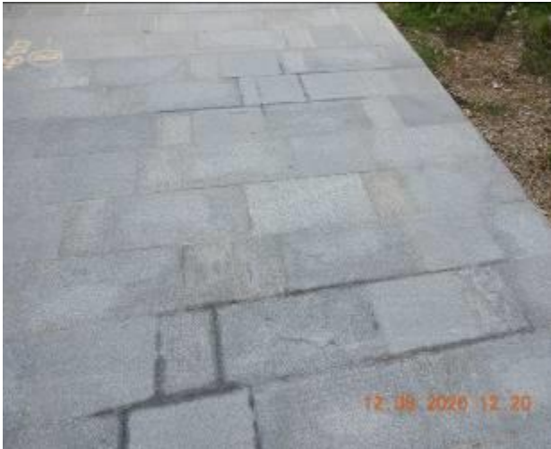
Figure 479 – Loss of material through footpath pavement
