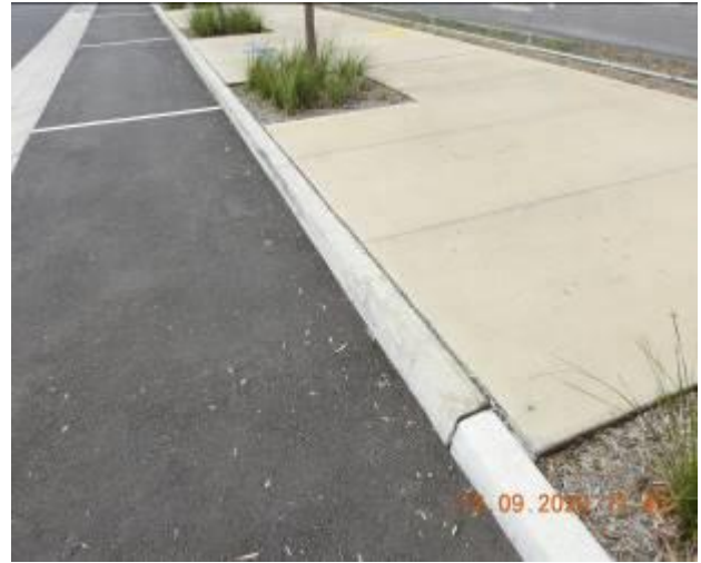
Figure 1336 – Loss of material through kerb
