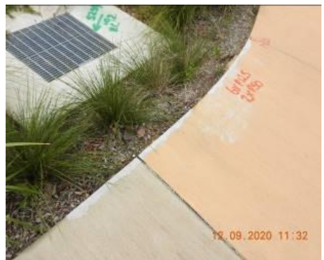
Figure 1160 – Loss of material through footpath pavement
