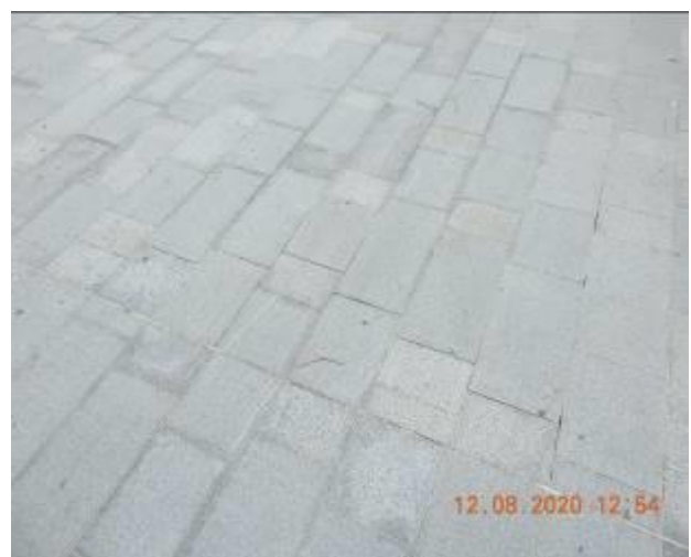
Figure 736 – Efflorescence, hairline crack propagation and loss of material through footpath pavement
