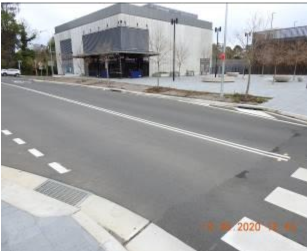
Figure 661 – Evidence of patchwork through road surface
