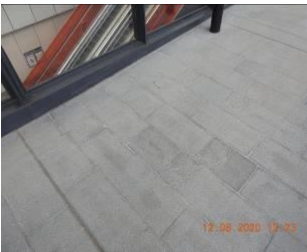
Figure 1962 – Efflorescence through floor tiles
