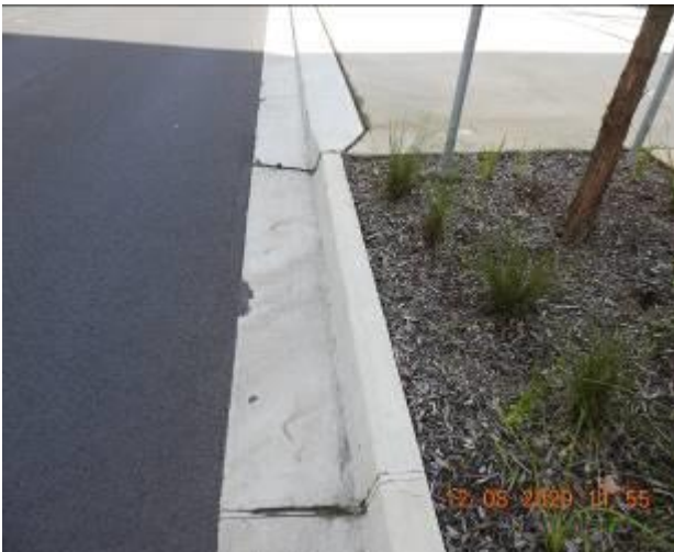
Figure 1771 – Crack propagation and loss of material through kerb and gutter
