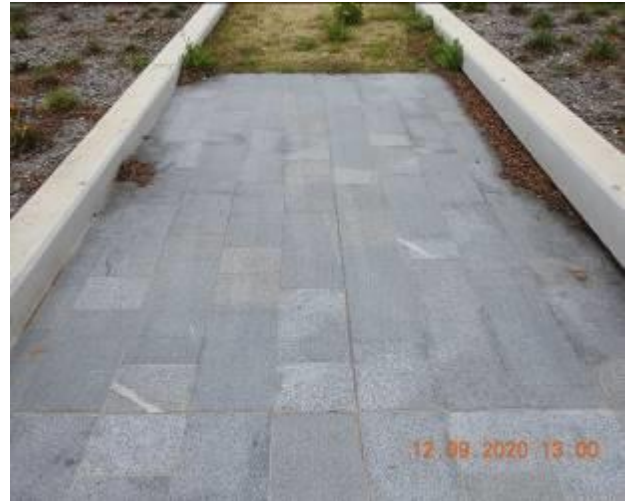
Figure 284 – Hairline cracking and efflorescence through footpath pavement
