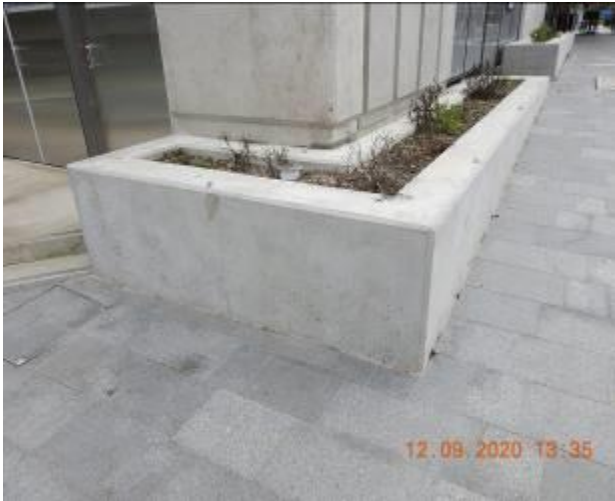
Figure 2366 – Loss of material through external wall
