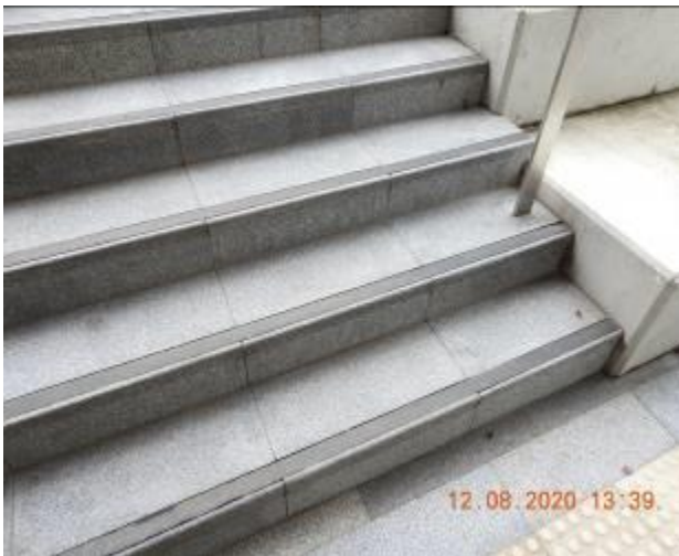
Figure 2082 – Separation through staircase pavement
