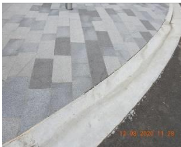
Figure 1573 – Crack propagation and loss of material through footpath pavement
