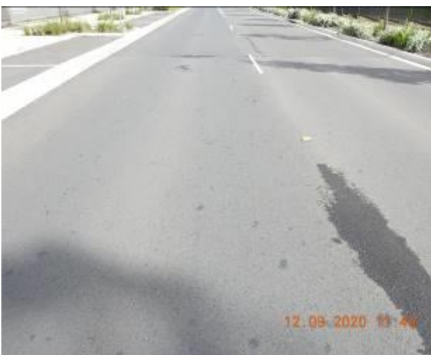
Figure 1393 – Evidence of patchwork through road surface
