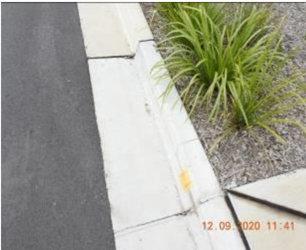
Figure 1307 – Crack propagation and loss of material through kerb and gutter
