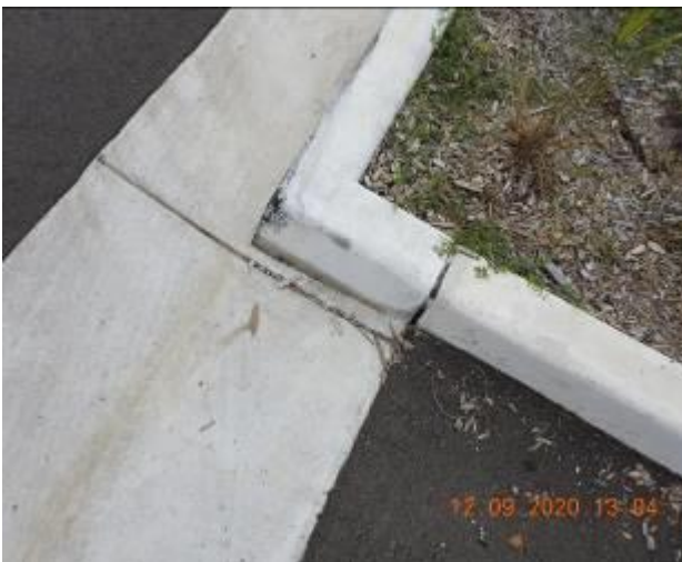
Figure 369 – Loss of material through kerb
