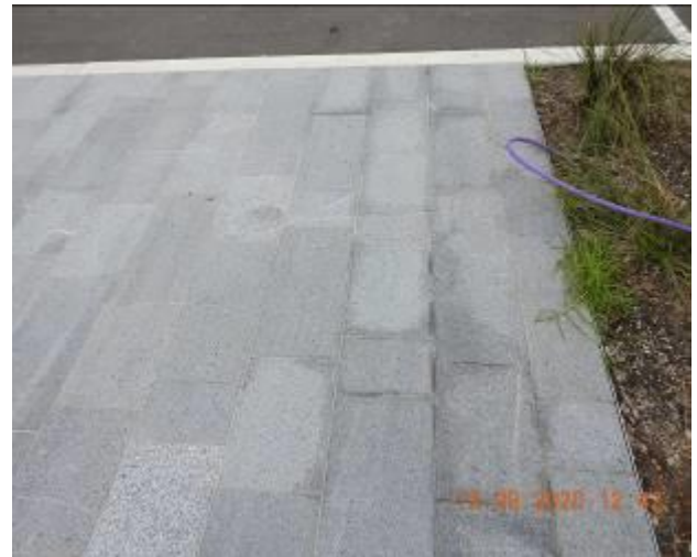
Figure 26 – Hairline cracking and efflorescence through footpath pavement
