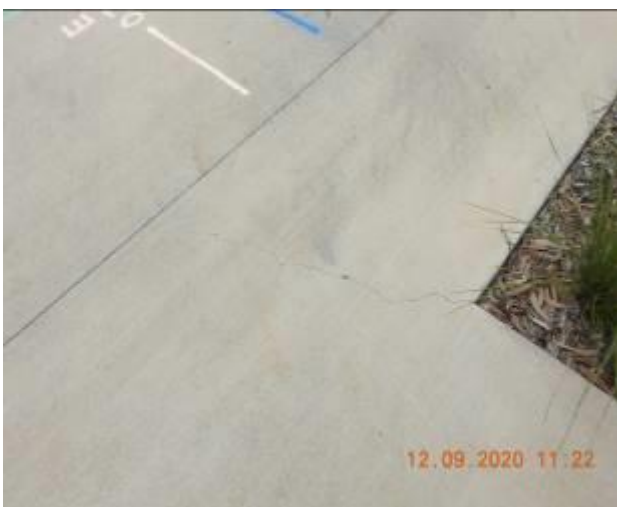
Figure 1069 – Crack propagation through footpath pavement
