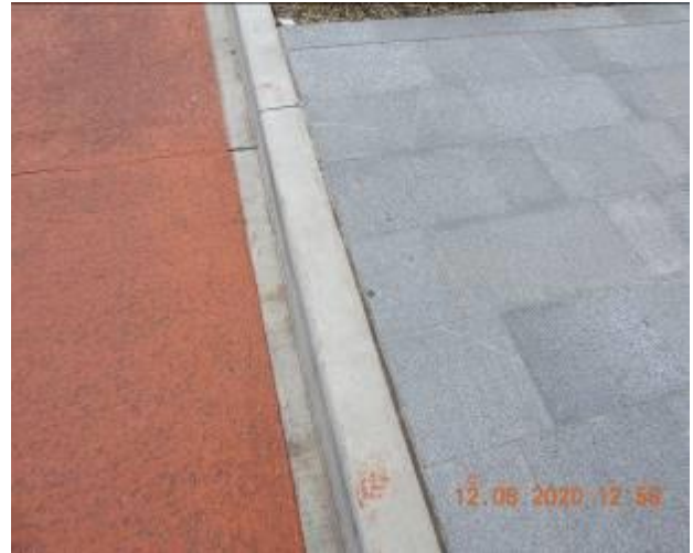
Figure 798 – Hairline crack propagation and evidence of patchwork through kerb
