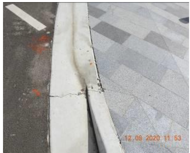
Figure 1750 – Crack propagation and loss of material through layback and gutter
