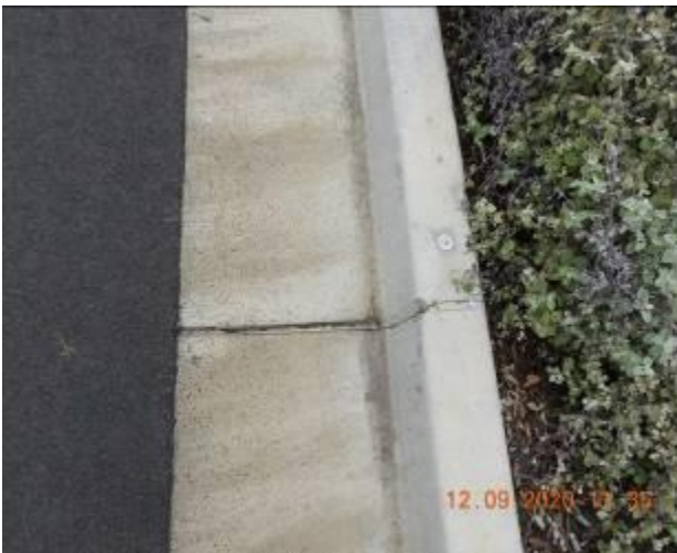
Figure 1205 – Crack propagation and loss of material through kerb and gutter
