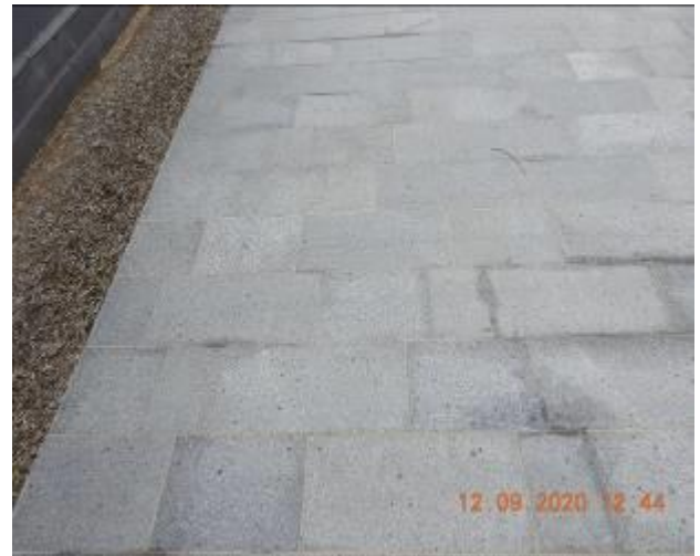
Figure 64 – Hairline cracking and efflorescence through footpath pavement
