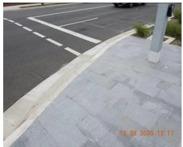
Figure 935 – Hairline crack propagation through footpath pavement
