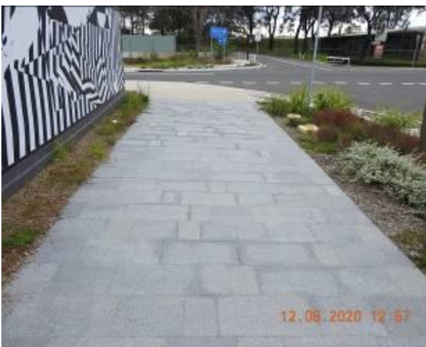
Figure 777 – Loss of material through footpath pavement
