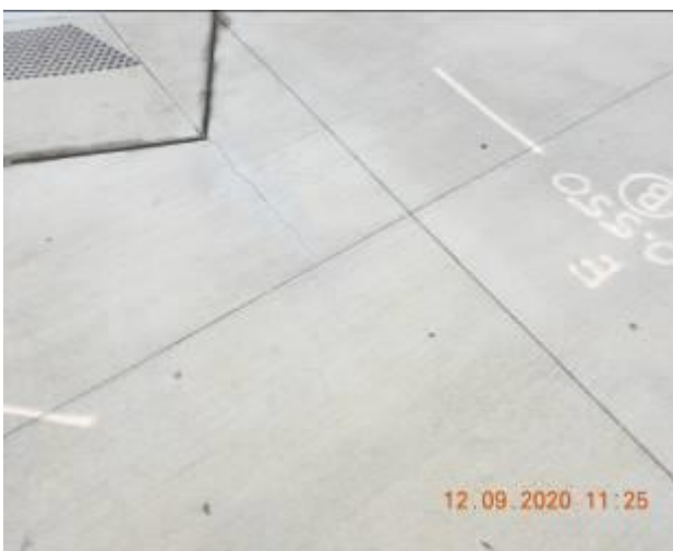
Figure 1093 – Crack propagation and loss of material through footpath pavement
