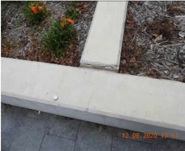
Figure 2111 – Crack propagation and loss of material through retaining wall
