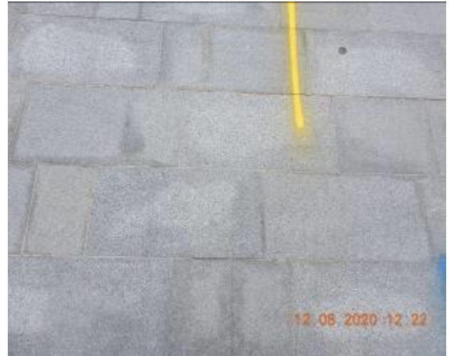
Figure 510 – Loss of material through footpath pavement
