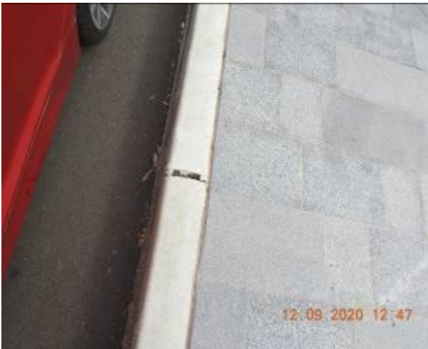
Figure 129 – Crack propagation and loss of material through kerb
