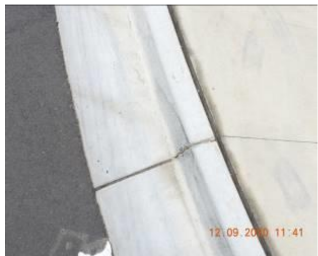
Figure 1304 – Crack propagation and loss of material through kerb
