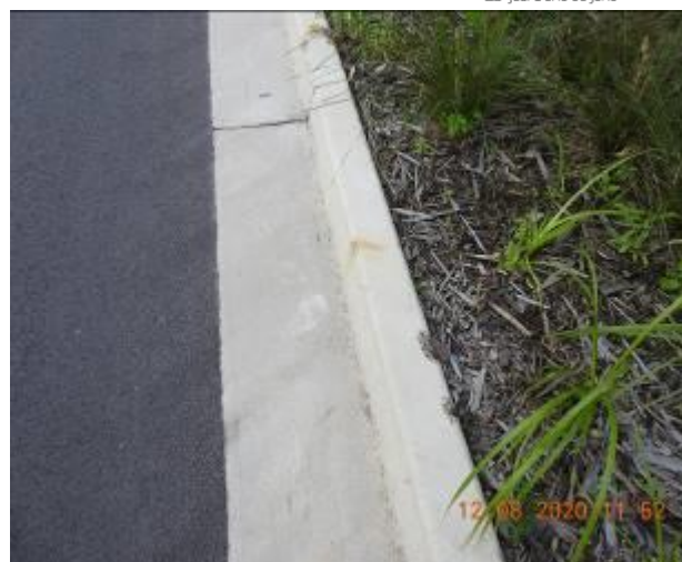
Figure 1734 – Loss of material through kerb
