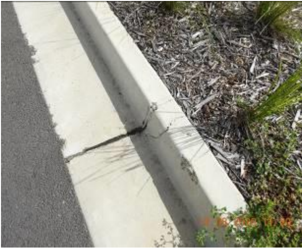
Figure 1715 – Crack propagation and loss of material through gutter
