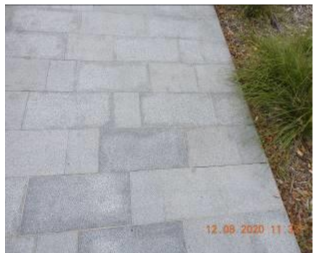
Figure 1612 – Crack propagation and loss of material through footpath pavement
