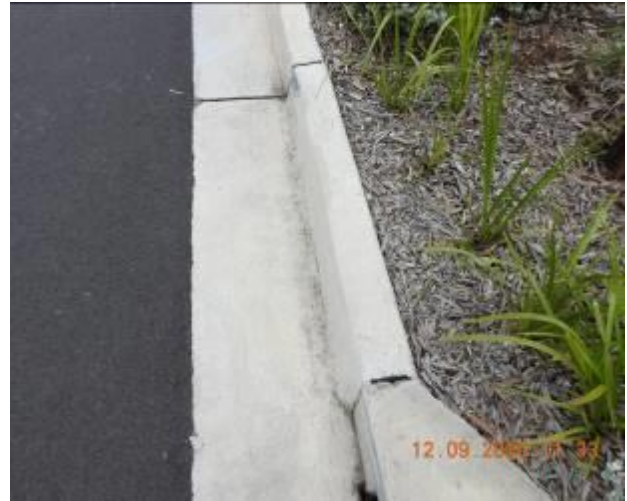
Figure 1174 – Loss of material through kerb
