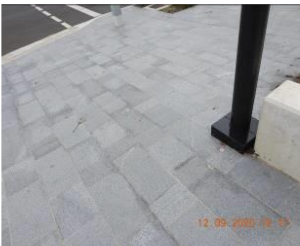
Figure 928 – Hairline crack propagation through footpath pavement
