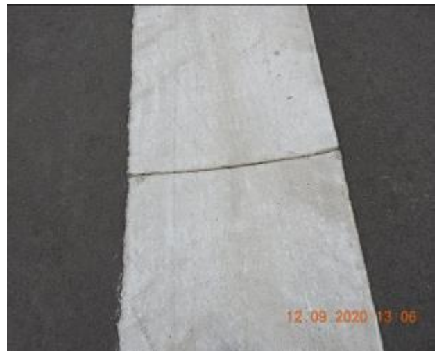
Figure 394 – Crack propagation through gutter
