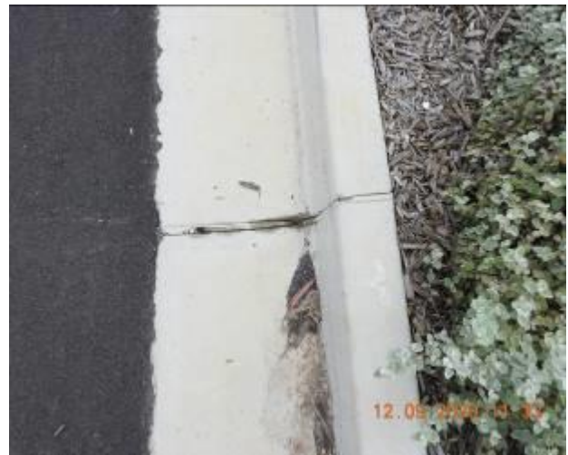
Figure 1170 – Crack propagation and loss of material through kerbs and gutter
