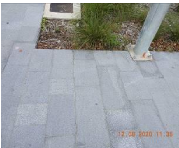
Figure 1629 – Crack propagation and loss of material through footpath pavement
