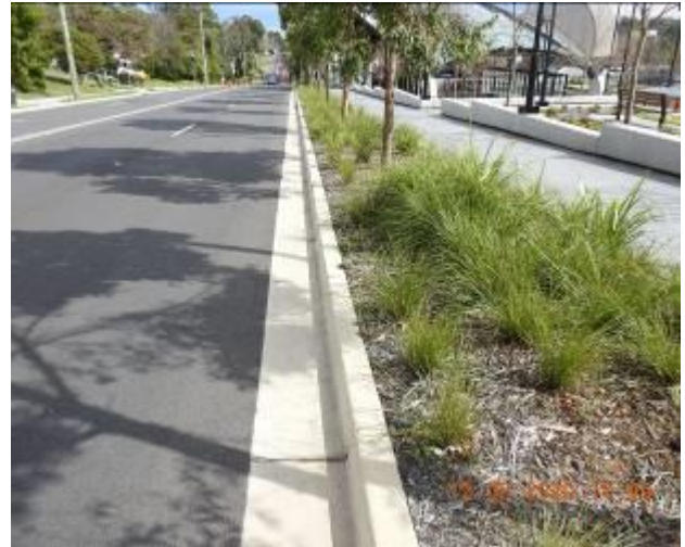
Figure 1706 – Loss of material through kerb and gutter
