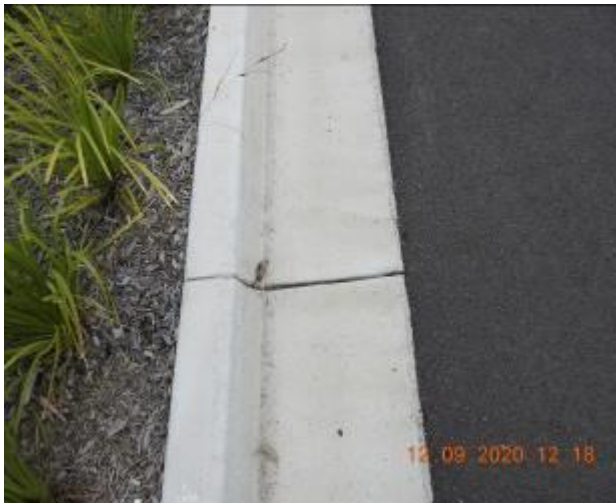
Figure 950 – Crack propagation and loss of material through kerb
