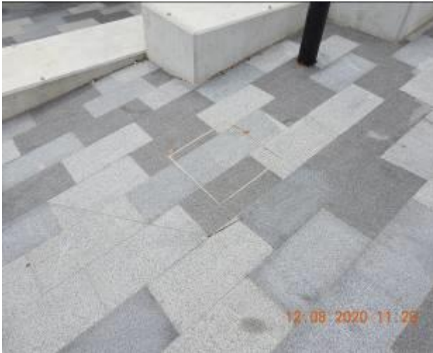
Figure 1577 – General condition of service pit/ Loss of material through footpath pavement
