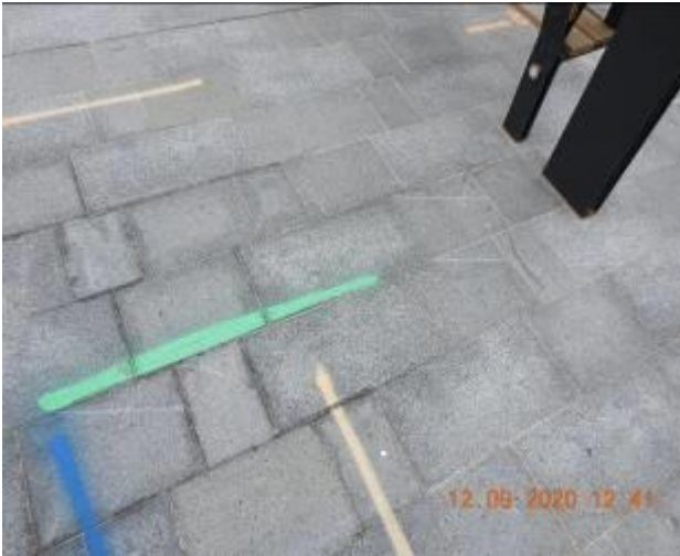
Figure 13 – Hairline cracking and efflorescence through footpath pavement
