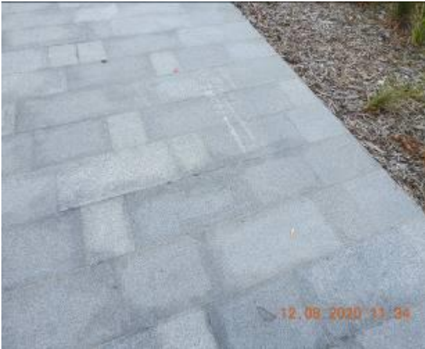
Figure 1625 – Hairline crack propagation through footpath pavement
