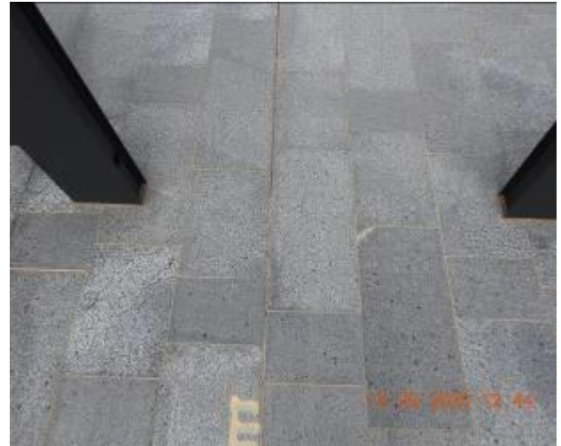
Figure 74 – Hairline cracking and efflorescence through footpath pavement
