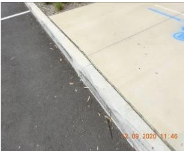
Figure 1361 – Crack propagation and loss of material through kerb
