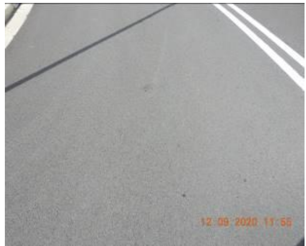
Figure 1452 – Loss of material through road surface
