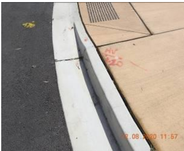
Figure 1801 – Crack propagation through kerb and gutter
