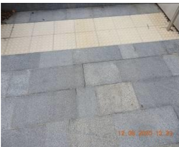
Figure 2036 – Loss of material through floor tiles
