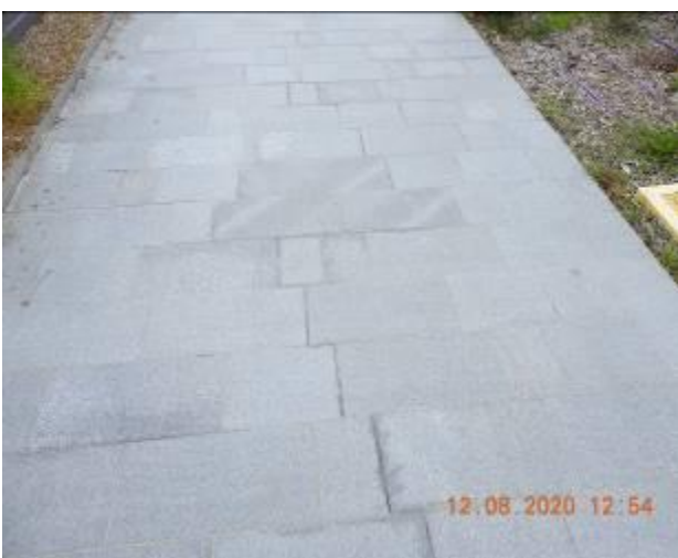
Figure 747 – Loss of material through footpath pavement
