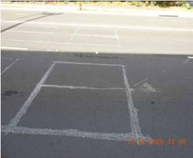
Figure 1823 – Loss of material and evidence of patchwork through road surface
