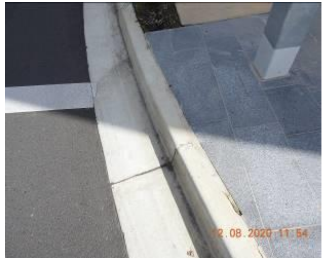
Figure 1760 – Crack propagation and loss of material through kerb
