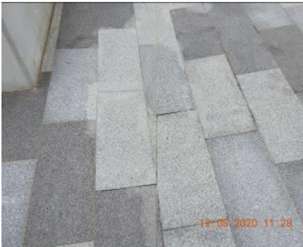
Figure 1579 – Crack propagation and loss of material through footpath pavement
