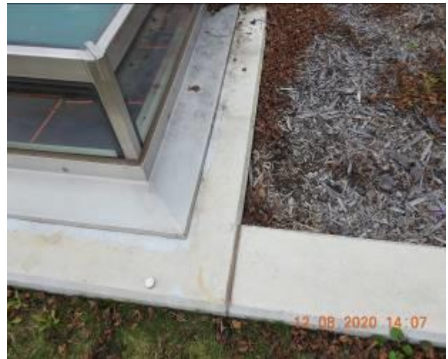
Figure 2234 – Loss of material through retaining wall
