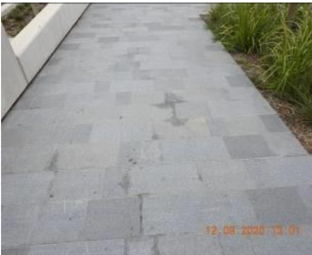
Figure 303 – Hairline cracking and efflorescence through footpath pavement
