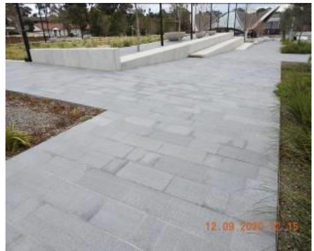
Figure 903 – Efflorescence and crack propagation through footpath pavement
