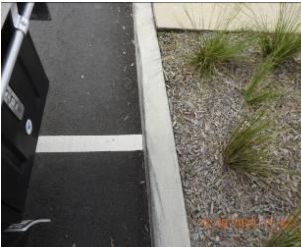
Figure 1319 – Crack propagation through kerb
