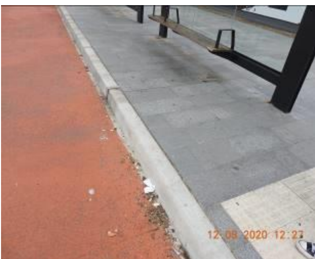
Figure 573 – Evidence of patchwork crack propagation and loss of material through kerb
