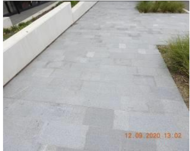
Figure 308 – Hairline cracking and efflorescence through footpath pavement
