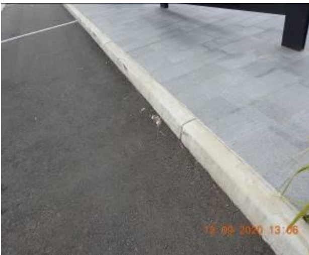
Figure 387 – Crack propagation through kerb
