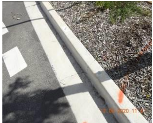
Figure 1796 – Crack propagation and loss of material through kerb and gutter
