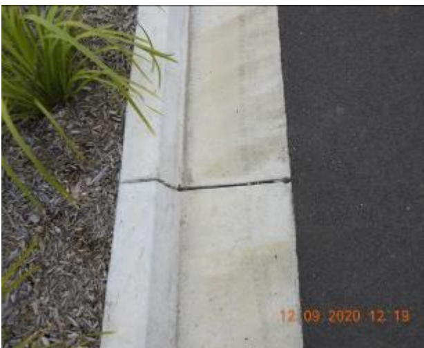
Figure 970 – Crack propagation and loss of material through kerb and gutter
