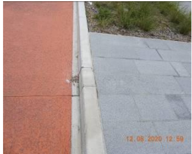
Figure 804 – Crack propagation and loss of material through kerb
