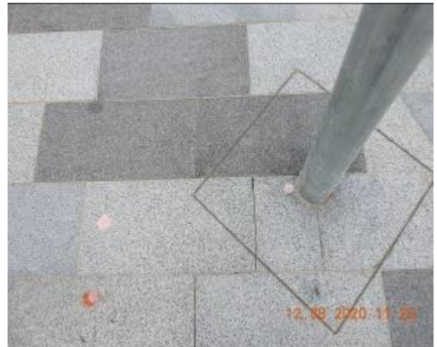
Figure 1580 – Crack propagation and loss of material through footpath pavement
