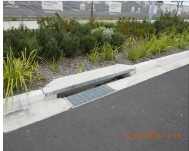
Figure 967 – General condition of stormwater inlet pit
