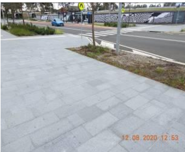
Figure 729 – Efflorescence, hairline crack propagation and loss of material through footpath pavement
