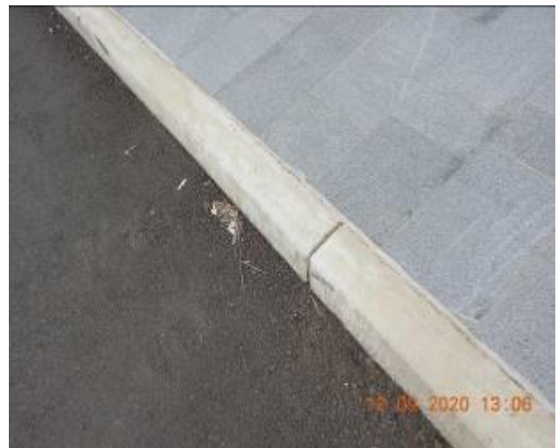
Figure 388 – Crack propagation through kerb
