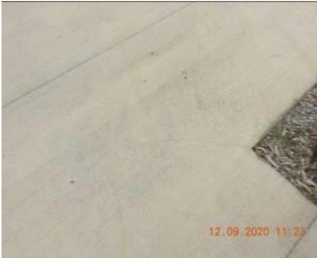
Figure 1071 – Crack propagation through footpath pavement
