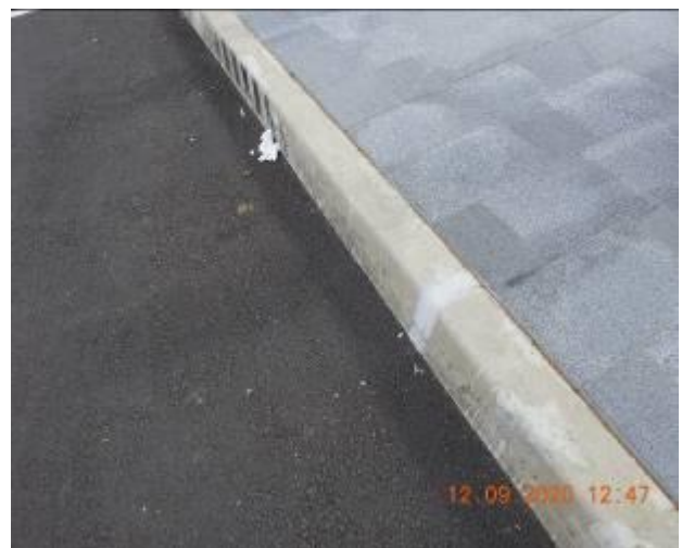
Figure 106 – Evidence of patchwork and crack propagation through kerb
