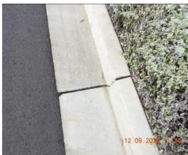
Figure 1271 – Loss of material through kerb and gutter
