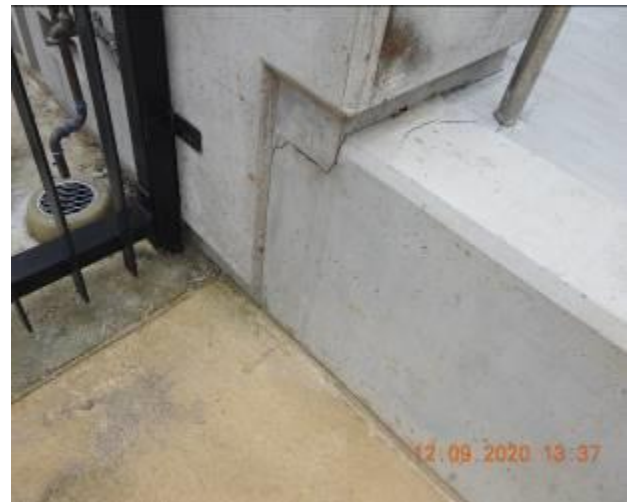
Figure 2387 – Crack propagation and loss of material through staircase pavement
