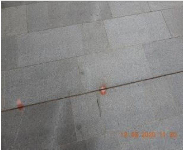
Figure 1589 – Loss of material through footpath pavement
