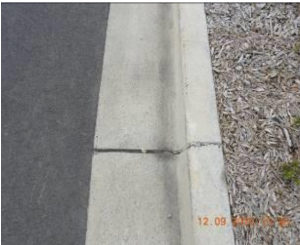
Figure 1229 – Crack propagation and loss of material through kerb and gutter
