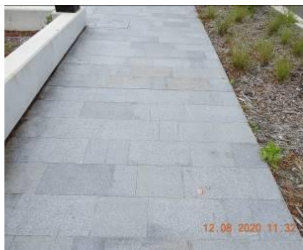
Figure 1604 – Hairline crack propagation through footpath pavement
