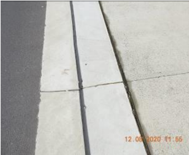
Figure 1775 – Loss of material through layback
