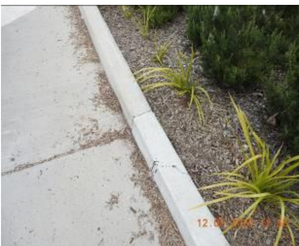
Figure 789 – Loss of material through kerb
