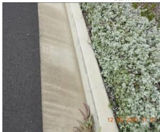
Figure 1246 – Crack propagation through kerb
