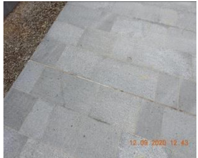
Figure 40 – Hairline cracking and efflorescence through footpath pavement
