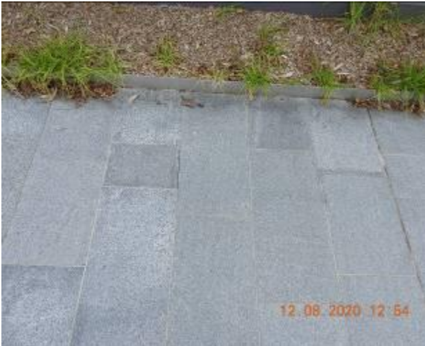
Figure 743 – Loss of material through footpath pavement
