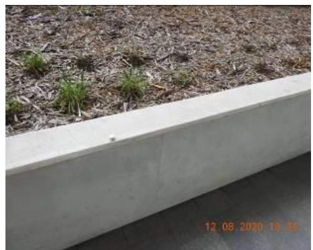
Figure 2049 – Crack propagation through retaining wall
