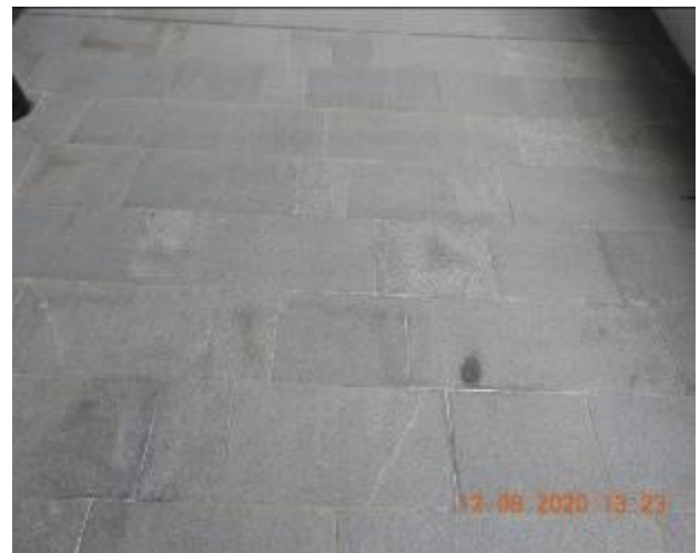
Figure 1959 – Efflorescence and hairline crack propagation through floor tiles
