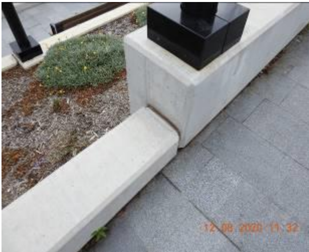
Figure 1597 – Crack propagation and loss of material through show ground retaining wall
