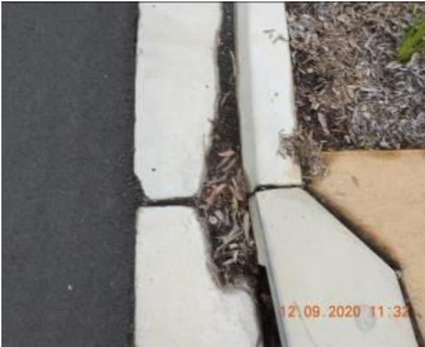
Figure 1167 – Loss of material through kerbs and gutter
