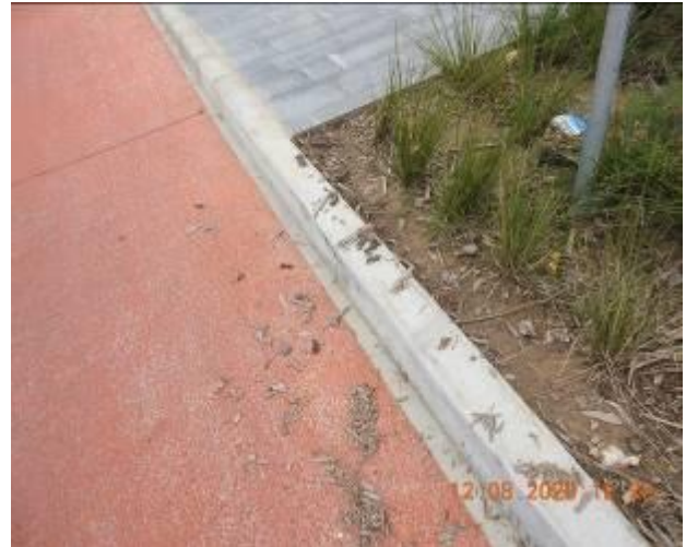
Figure 588 – Evidence of patchwork and hairline cracking through kerb
