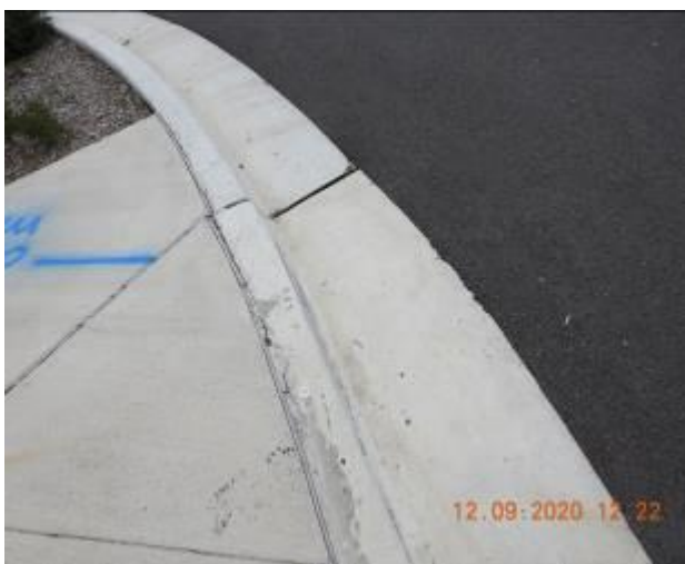
Figure 1006 – Crack propagation and loss of material through kerb and gutter
