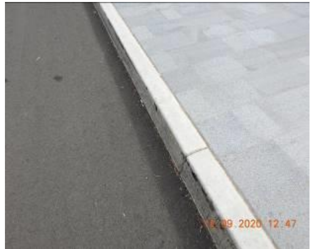
Figure 136 – Crack propagation through kerb
