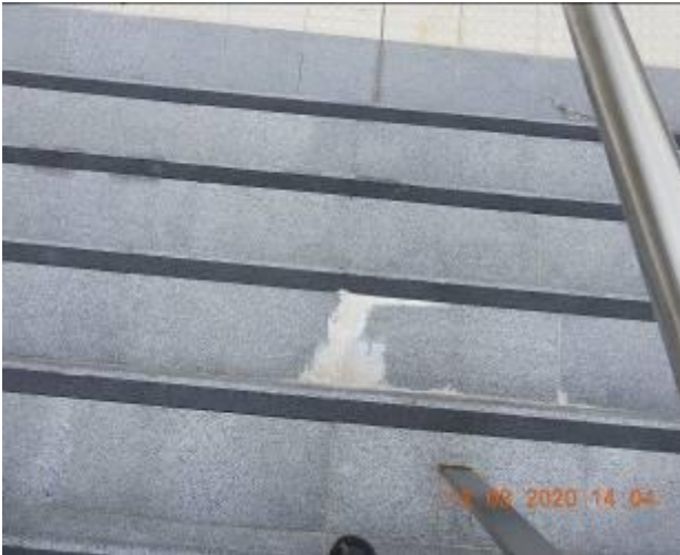
Figure 2201 – Efflorescence through staircase floor
