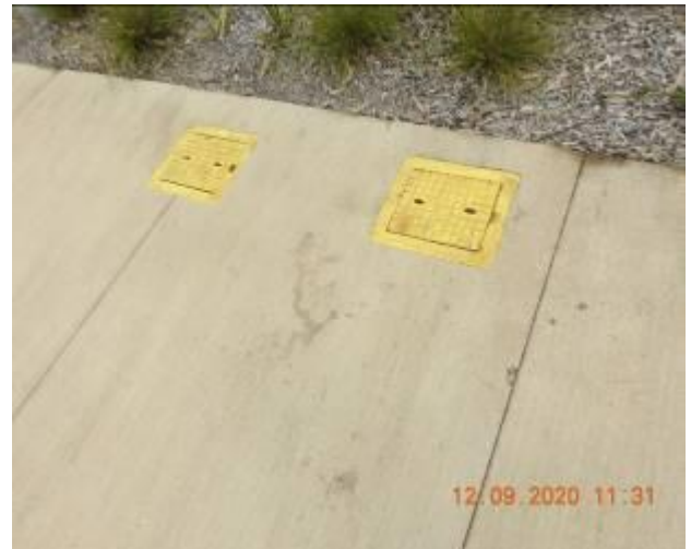
Figure 1158 – General condition of service pit/ Loss of material through footpath pavement
