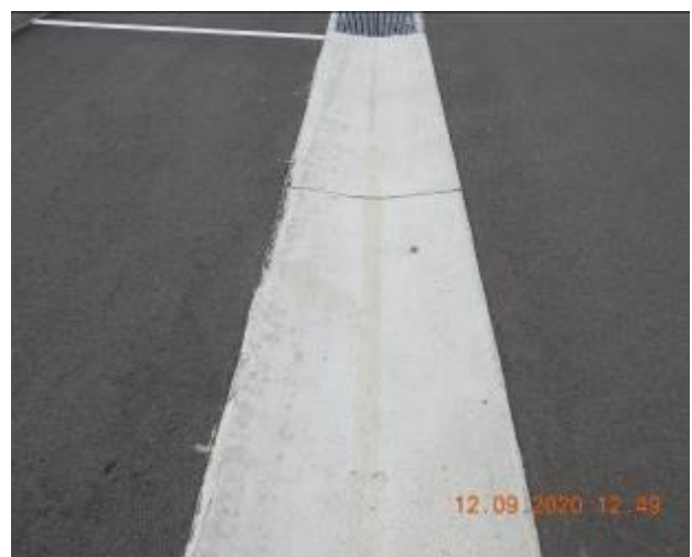
Figure 168 – Crack propagation and loss of material through gutter
