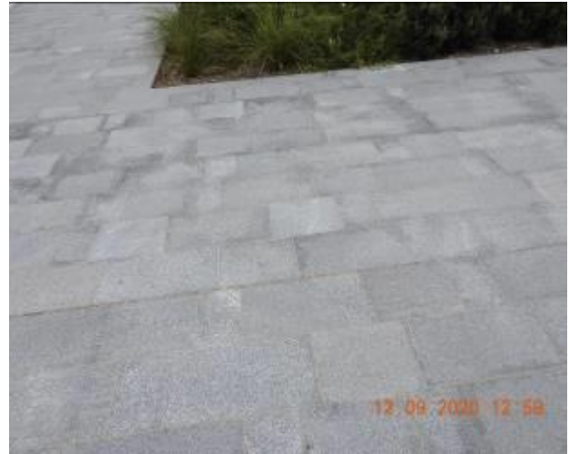
Figure 260 – Hairline cracking and efflorescence through footpath pavement
