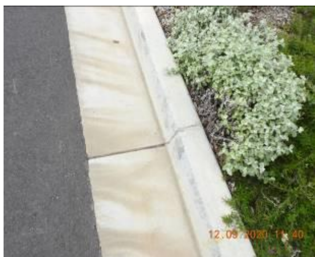
Figure 1289 – Crack propagation and loss of material through kerb and gutter
