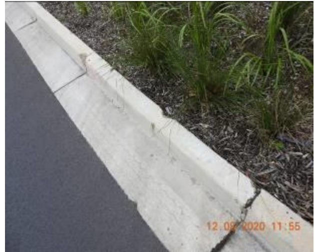
Figure 1770 – Loss of material through kerb and gutter
