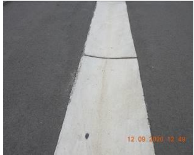
Figure 164 – Crack propagation and loss of material through gutter
