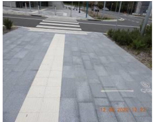
Figure 512 – Efflorescence and hairline crack propagation through footpath pavement
