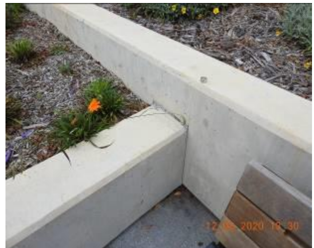
Figure 2001 – Crack propagation and loss of material through retaining wall
