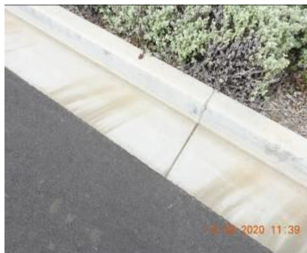
Figure 1284 – Crack propagation and loss of material through kerb and gutter
