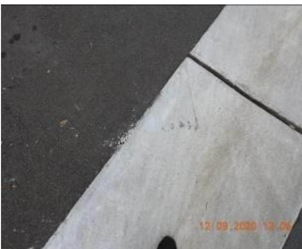
Figure 371 – Crack propagation and loss of material through gutter
