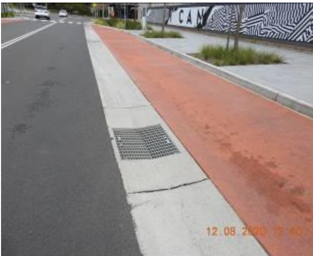
Figure 625 – Crack propagation and loss of material through road surface
