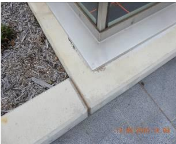
Figure 2259 – Loss of material through retaining wall
