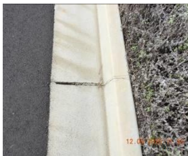
Figure 1266 – Crack propagation and loss of material through kerb and gutter
