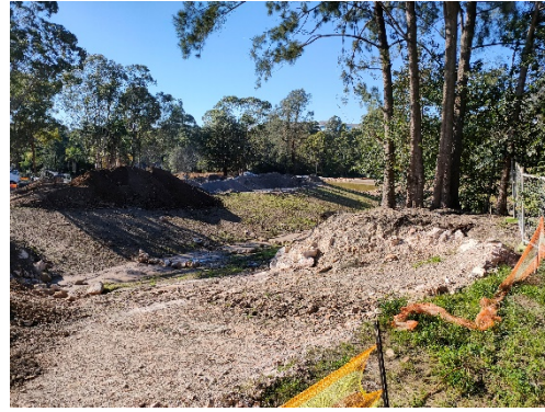
Figure 24 – Temporary drainage channel excavated in eastern portion of SU1. Aspect northeast
