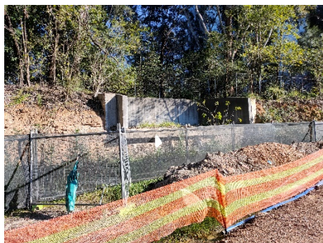
Figure 33 – View south from SU1 at the edge of SU3. Truncation of landform from previous development as well as clear section showing skeletal topsoil onto eroding sandstone bedrock
