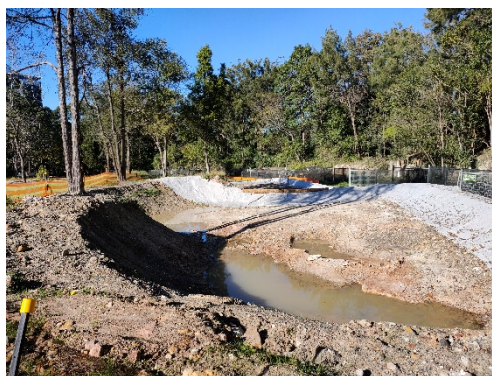
Figure 22 – Temporary drainage channel excavated in eastern portion of SU1. Aspect east
