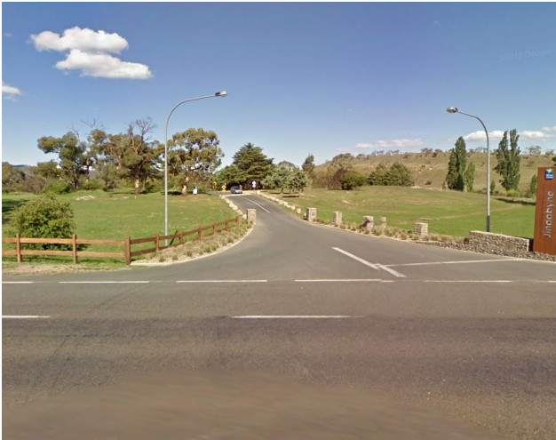
Picture 1 - View of entrance to Jindabyne Sport and Recreation facility from Barry Way
