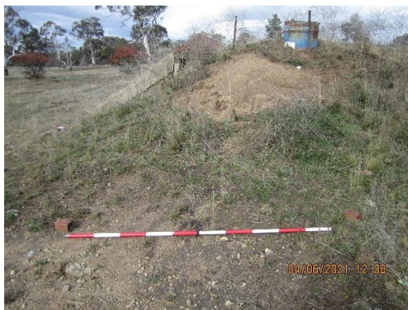
Plate 3-25. Raised ground and associated stairs, georeferenced to the location of a previous accommodation hut from the Snowy Hydro Scheme.
