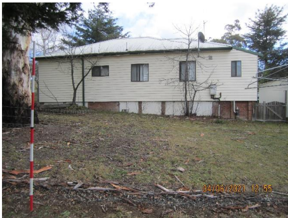
Plate 3-34. Weatherboard locally listed Snowy Hyrdo Scheme accommodation buildings. The building is located on a slight incline and has therefore been constructed on piers.
