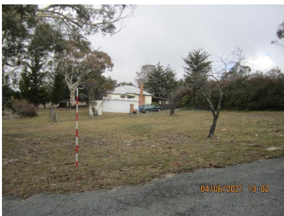
Plate 3-38. View south-west across cottage 17
