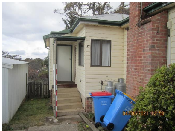
Plate 3-37. Entrance way to the building including raised stairs.
