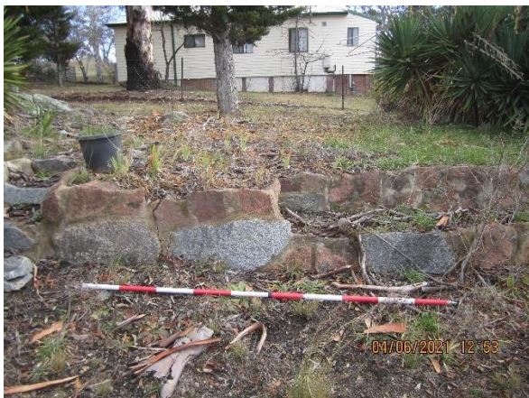
Plate 3-33. Detailed photo of sandstone retaining wall associated with the boundary of one of the accommodation huts.
