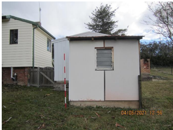
Plate 3-35. Added fibro extension to one of the locally listed Snowy Hydro Scheme accommodation buildings.
