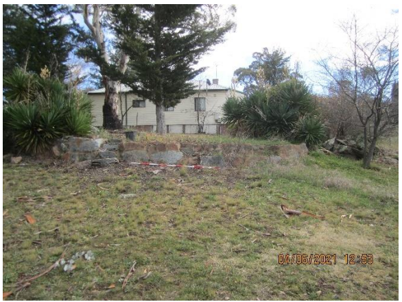
Plate 3-32. Weatherboard accommodation hut and associated sandstone retaining wall.
