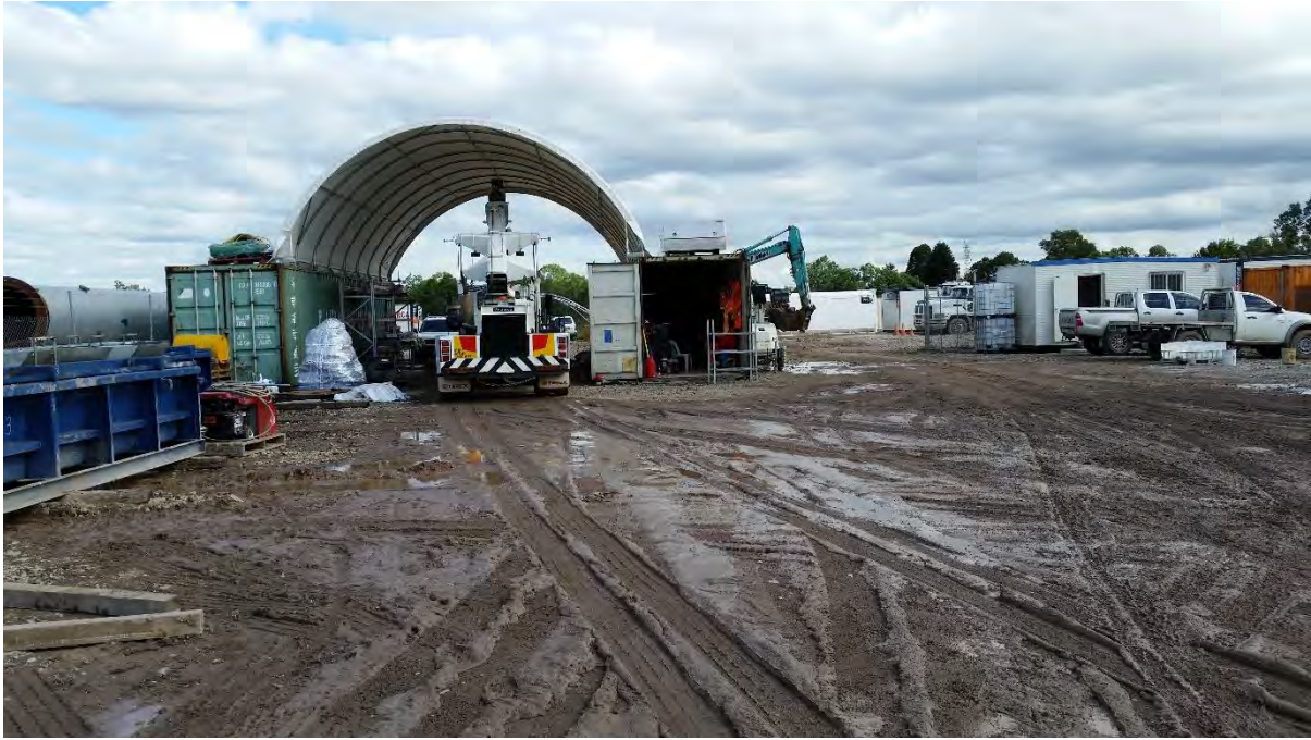
65 Dunheved Circuit, St Marys – Jaybro concrete fabrication yard looking south - 2017
