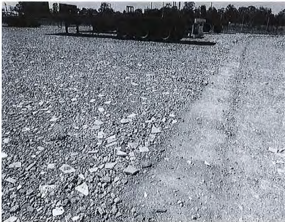
B: Recycled Crushed Concrete & Interface of Recycled Crushed Concrete and Underlying Material.
