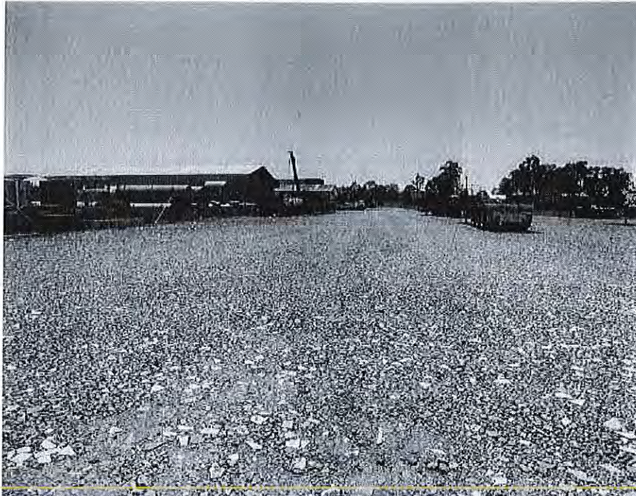
A: Site Condition – taken within south western portion of the site, looking east
