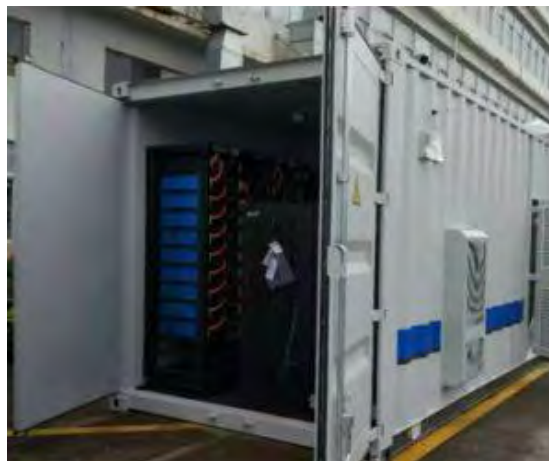
Figure 4: Internally Accessed BESS Units (From OSM marketing)
