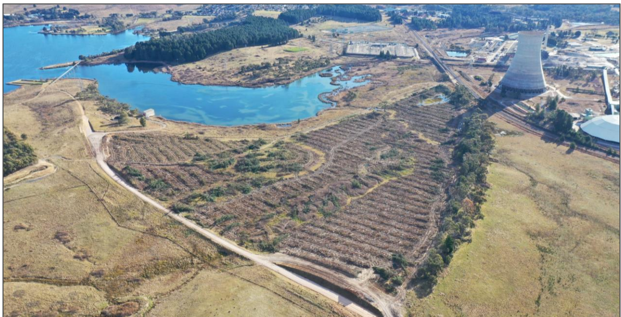
Figure 3 | Project site: aerial view looking west
