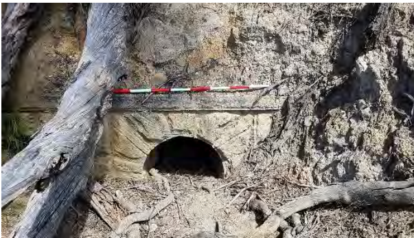
Plate 3-14: Sandstone culvert structure located within the Project Area under passing the railway embankment – eastern side.
