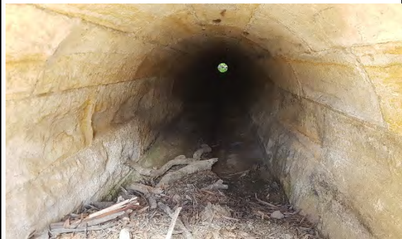
Plate 3-17: View through the sandstone viaduct, noting the rectangular sandstone brick work.
