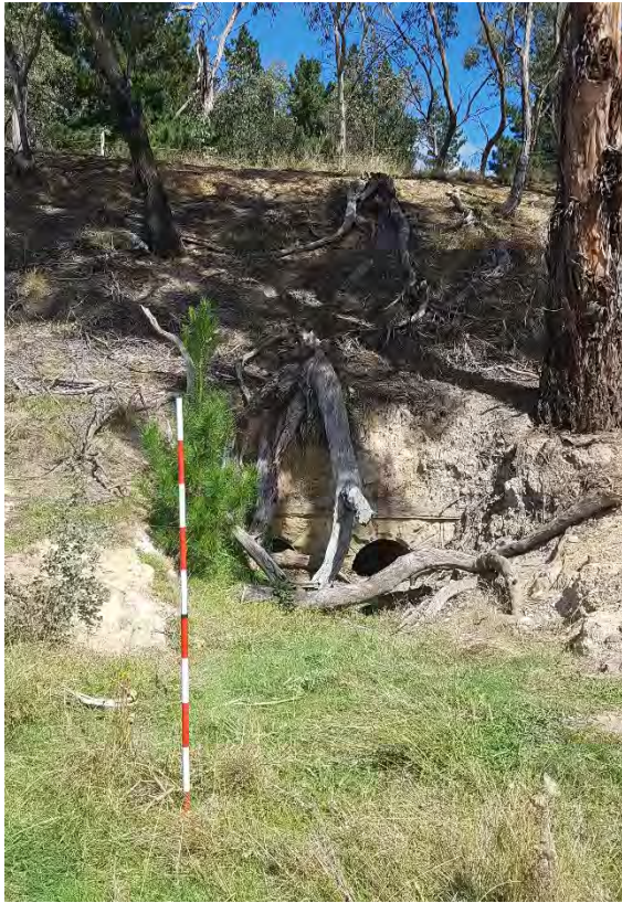
Plate 3-18: Sandstone culvert structure located within the Project Area under passing the railway embankment – western side. Remnant native trees are buried within the built-up railway embankment. Culvert within an ephemeral drainage line
