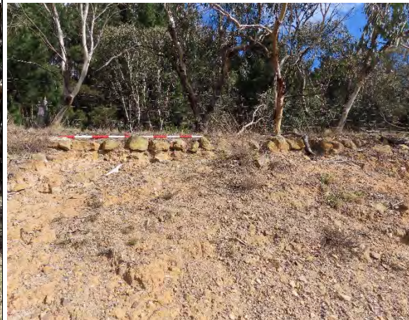
Plate 3-21: Profile view of embankment material with water rolled stones stabilising the edge of the railway line.
