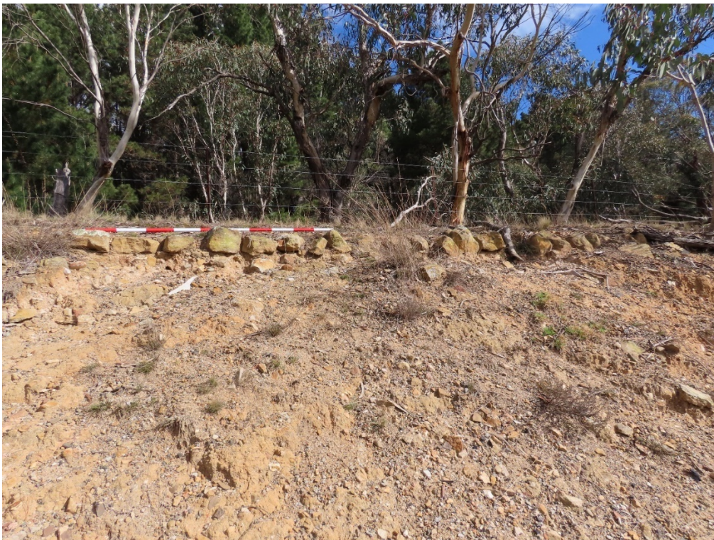
Plate 5-15: View of west of the exposed profile of fill that forms the raised remnant Great Western Railway.
