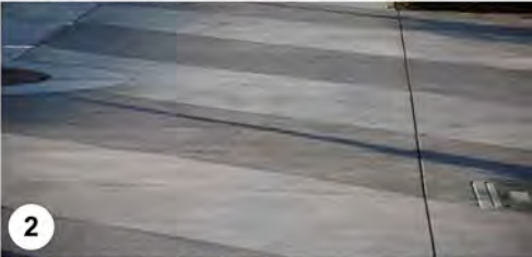
BANDED INSITU CONCRETE PAVING
