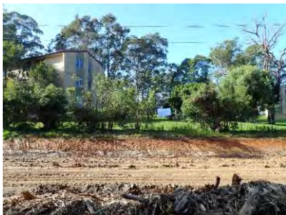
Figure 28 – View north-east across light-rail corridor toward western boundary of subject area. Note the exposed red and grey basal clay layers in the cut.
