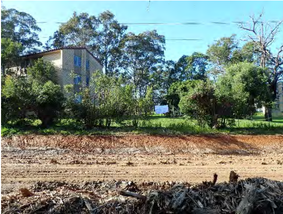
Figure 29 – View north-east across light-rail corridor toward western boundary of subject area. Note the exposed red and grey basal clay layers in the cut.
