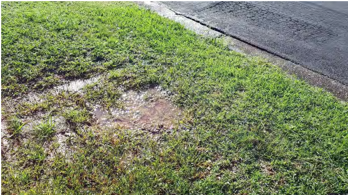
16. Foul odour noted on ground surface of Stage 2A.
