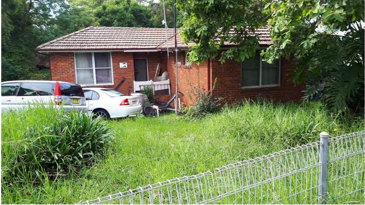
41. Stage3B – Corner of Burke Street and Cunningham Street.
