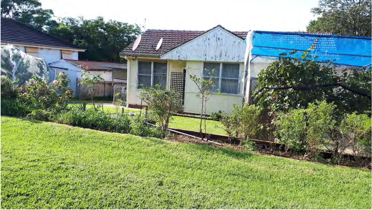
19. North western area of Stage 2A (facing east).
