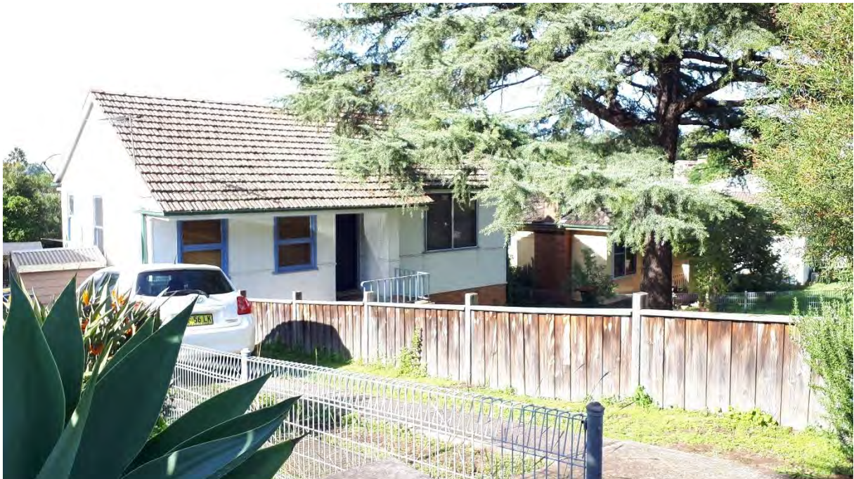
24. Western area of Stage 2B (facing south east).
