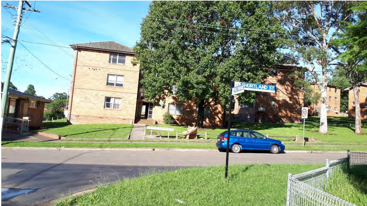
13. Northern area of Stage 1F (facing south).
