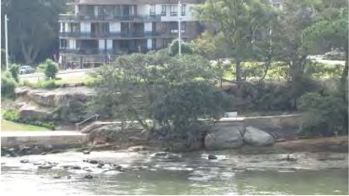
Hawkesbury HGL – Bedrock exposed along Parramatta River, Meadowbank, bordering Glenhaven HGL. Photo taken from Ryde Bridge looking north-east towards Parsonage Street, Meadowbank (Photo: DECCW/Marion Winkler).
