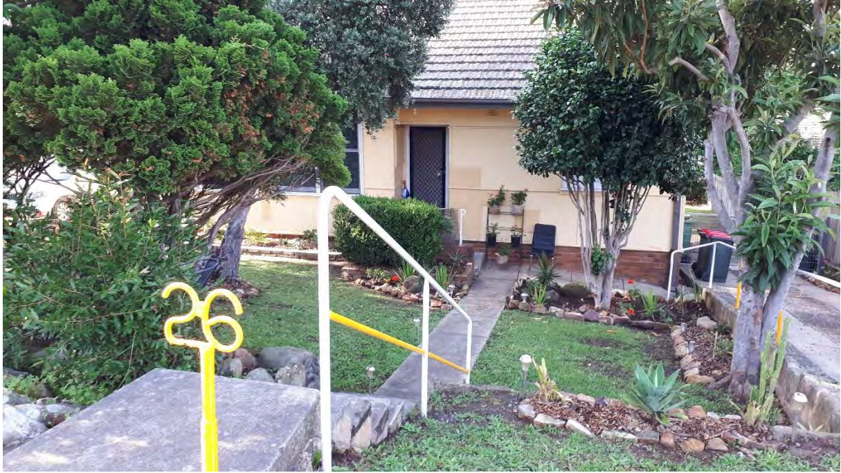
23. Stage 2B – 26 Marshall Road (facing south).
