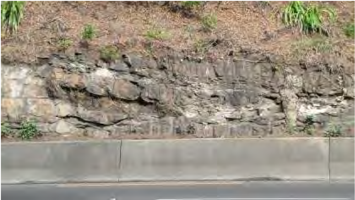
Hawkesbury HGL – Sandstone bedrock cutting boundary with Glenhaven HGL under rail bridge at Victoria Road, West Ryde (Photo: DECCW/Marion Winkler).
