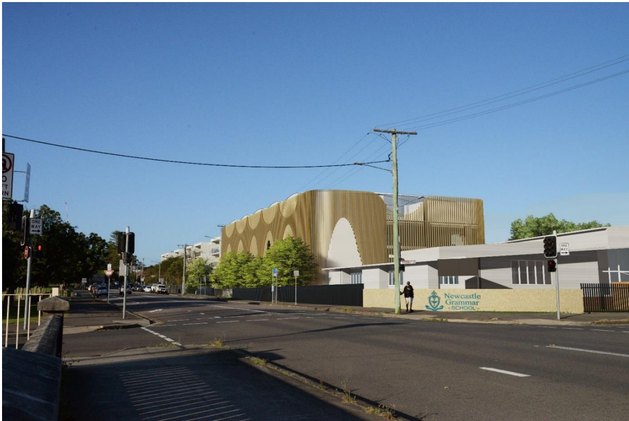
Figure 33 Pedestrian view of site from Union Street
