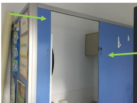
Photo No. 009: Bathroom
