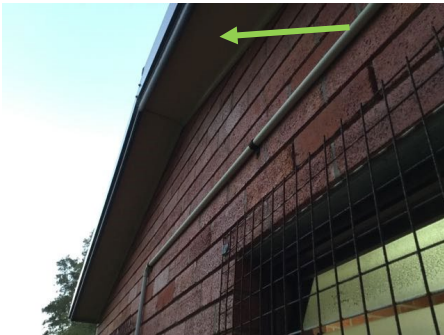
Photo No. 003: Eaves & Soffits
