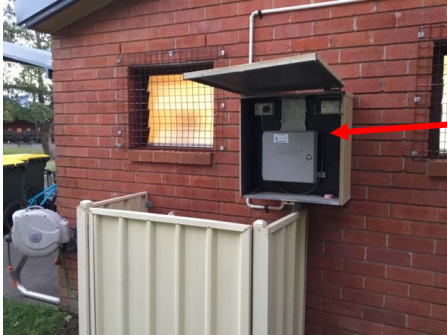
Admin/Library: Photo No. 001: Eastern elevation
