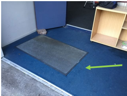
Photo No. 007: External western entry
