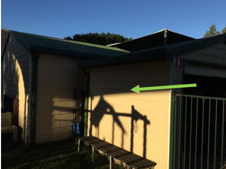
Photo No. 013: Hardiplank® wall cladding
