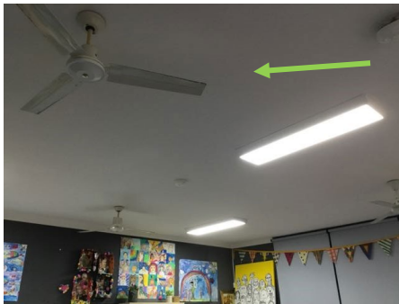
Photo No. 010: Ceiling void
