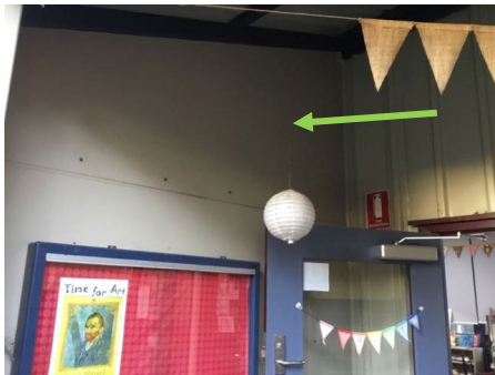
Photo No. 008: Western entry
