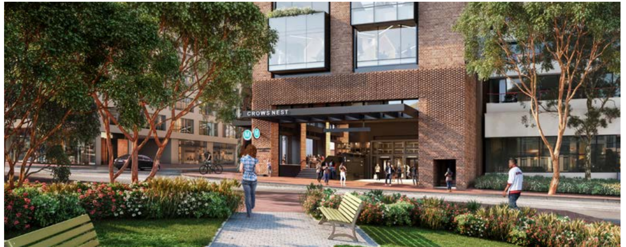
View of Metro Entry from Hume Street Park (indicative future upgrade shown)
