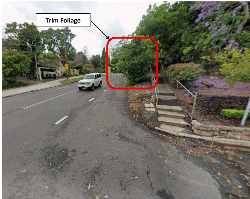
Figure 6: Gate 2 Sight Distance Limitation
