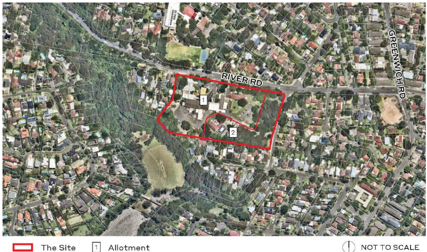
Figure 2 Site aerial and subject lots
