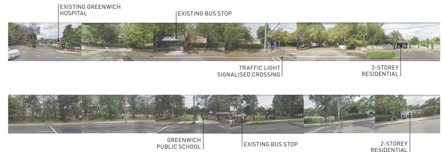
Existing Streetscape - River Road
