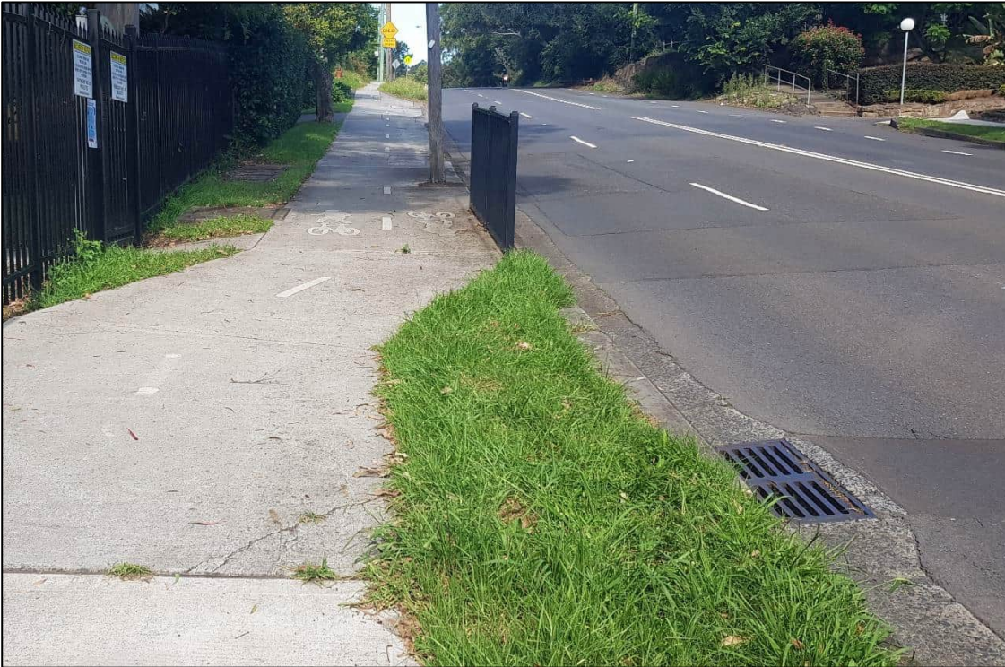
Figure D-3 Stormwater Inlet Pit along River Road
