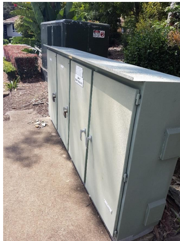
Figure 2.3 – Existing Main Switchboard
