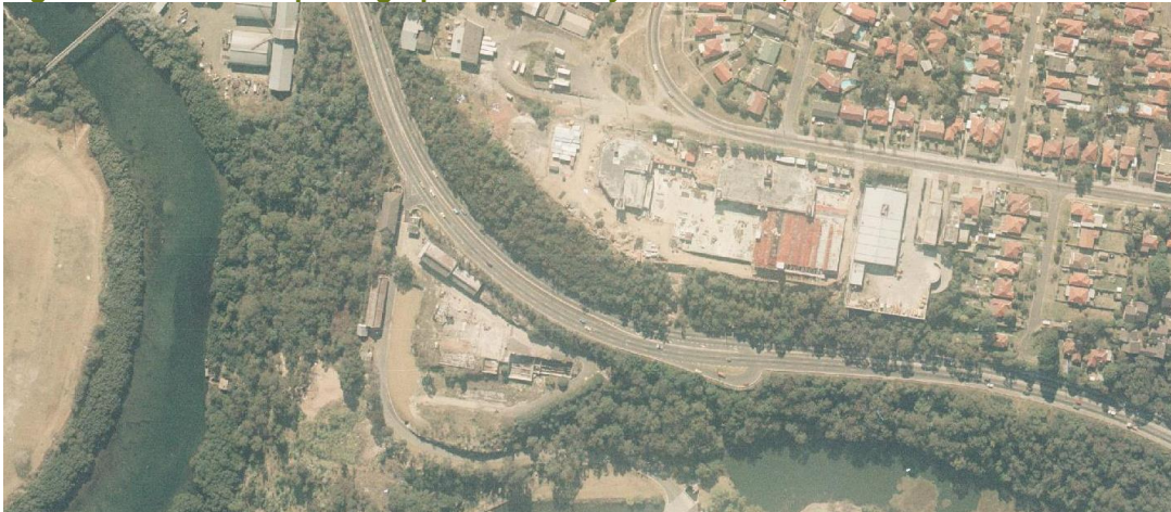
Figure 4: 1986 Aerial photograph of Mowbray Road West, Source NSW Historical Imagery
