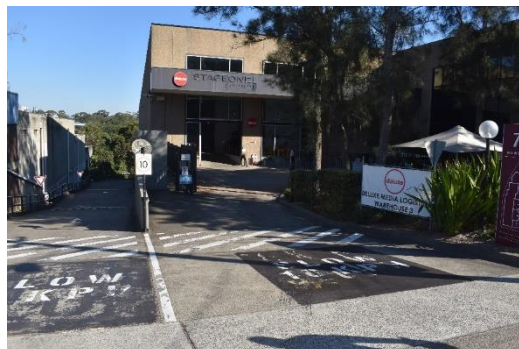
Figure 7: Main driveway to covered parking bays. Modification of landform to enable vehicle movement. Facing south
