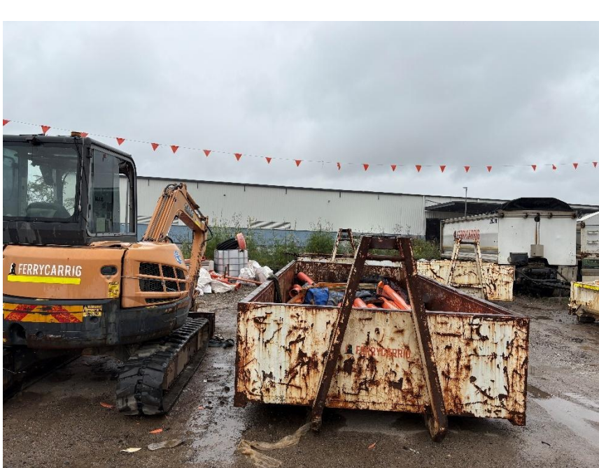
Photo 15: Skip bin and excavator in Ferry Carrig lease area (29/10/2025)
