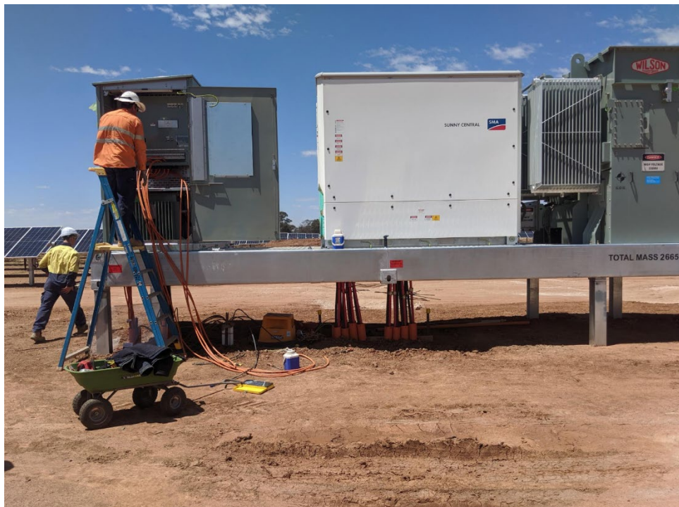
Figure 4-6 PCU installed on pile foundation (Courtesy of Octopus Investments Australia)
