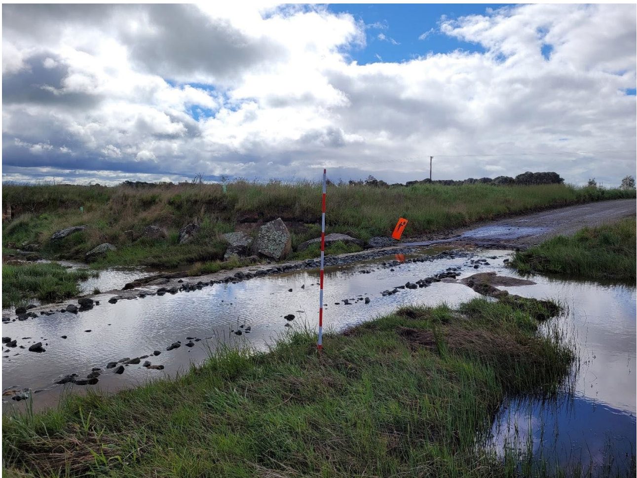
Figure 4-12 Damaged low-level crossing over Blind Creek. This crossing would require repair
