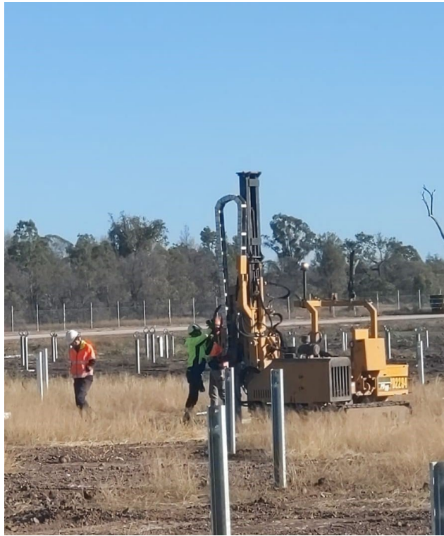
Figure 1-2 Example of typical distances between array support poles (source: NGH stock image).
