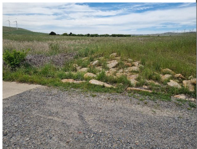
Plate 9-4 Example of the battered side of the creek crossing with loose stones as reinforcement. (Source: Stride Renewables).
