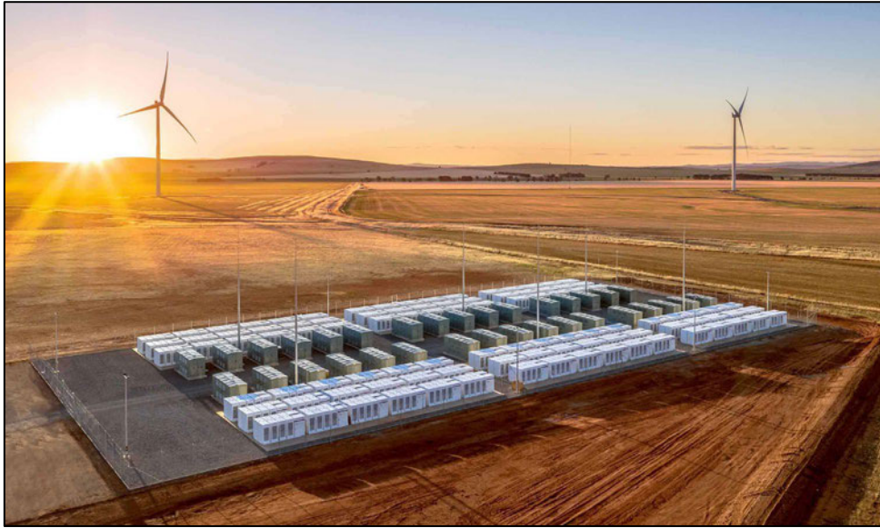
Figure 9-4 Example of an AC-coupled energy storage facility. The Hornsdale Power Reserve is 100MW / 129MWh and has a footprint of less than one hectare (Source Hornsdale Power Reserve)
