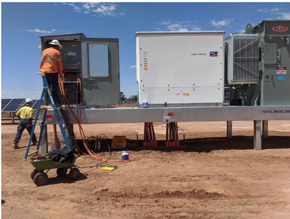
Figure 9-2 PCU installed on pile foundation. Courtesy Octopus Investments Australia
