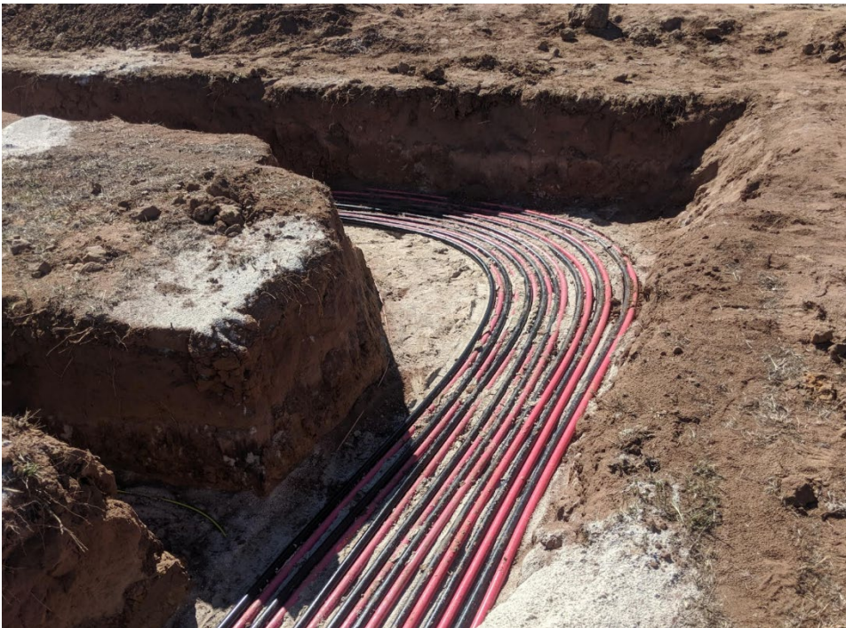
Figure 9-3 Example of AC cabling at a depth of 500mm, a similar style of underground cabling will be adopted for the proposed Blind Creek Solar Farm
