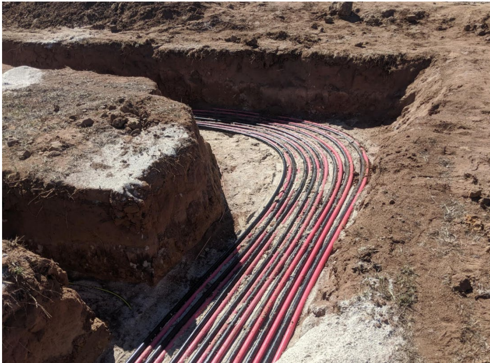
Figure 5-3 Example of AC cabling at a depth of 500mm, a similar style of underground cabling will be adopted for the proposed Blind Creek Solar Farm
