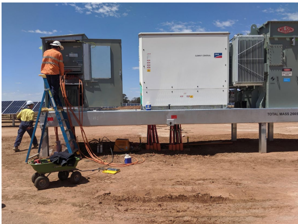
Figure 5-2 PCU installed on pile foundation. Courtesy Octopus Investments Australia
