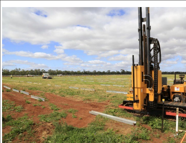
Plate 5-1 Example of machinery typically used to drive poles into the ground for the solar array supports (source: NGH stock image).
