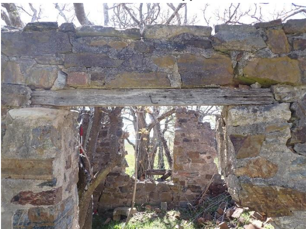
Figure 12 – Stone construction and timber door support
