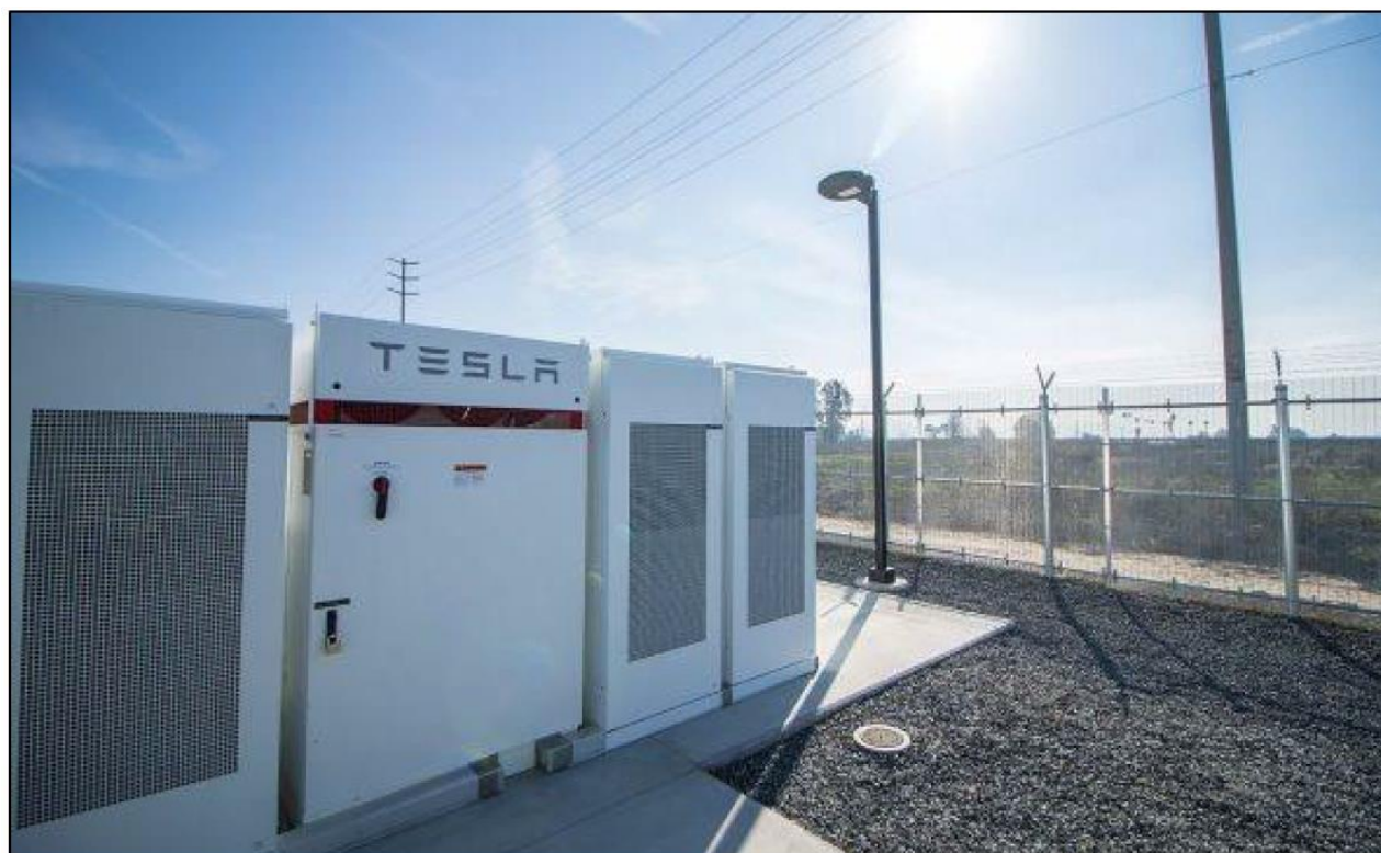
Figure 3-4: Typical BESS
