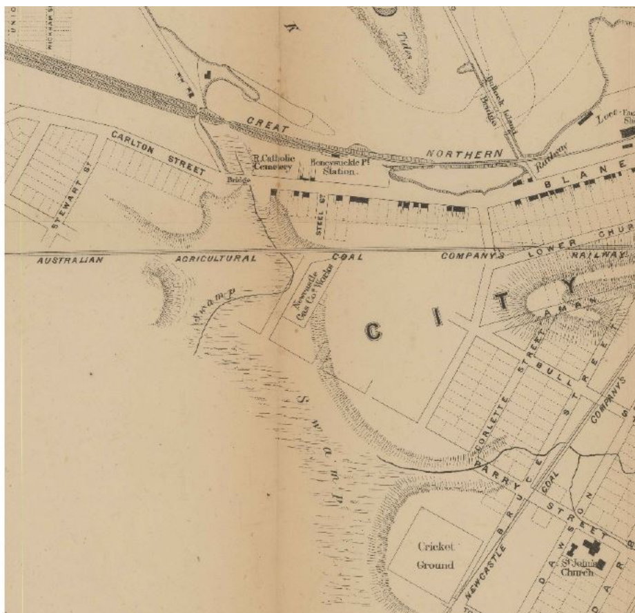
Figure 6. Map 1880 shows swamp edging Parry Street, while the current Project Area is located approximately 2.5 kilometres west of this map, the later 1897 photograph (Figure 5) shows the low-lying swamp area was extensive
