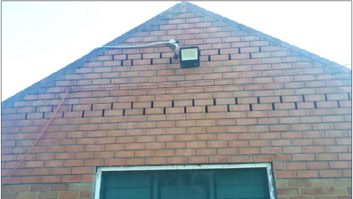
Plate 32: The eastern end of Building 9 to be demolished showing air vents into the brick wall cavity within the study area.
