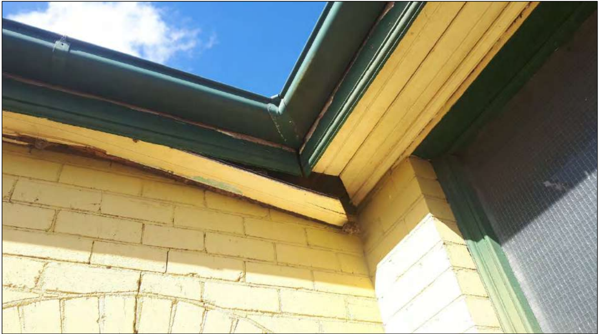
Plate 34: Gaps on the eaves along the northern face of Building 10 to be demolished within the study area.
