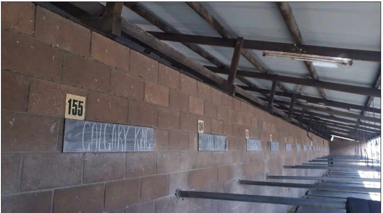
Plate 30: Stables to be demolished within the study area contained Besser block walls which did not extend to the full height of the roof.
