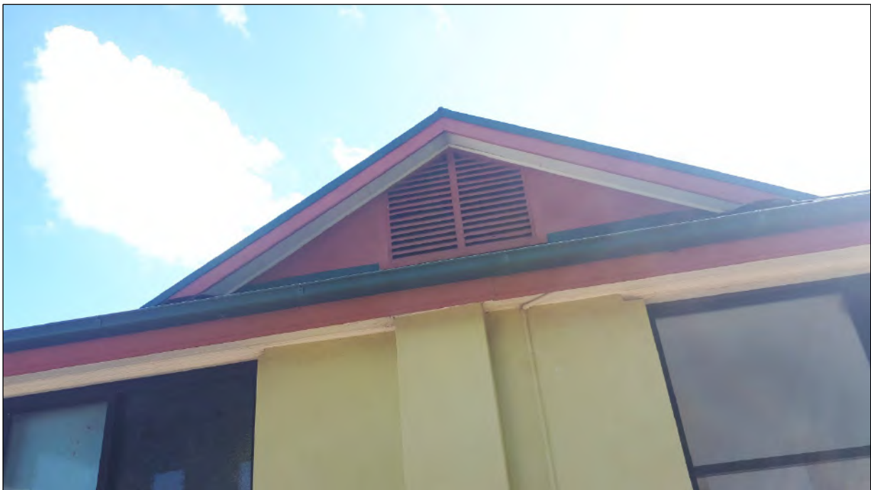
Plate 33: Vents on the eastern and western ends of Building 10 open into the main building space and not into an enclosed cavity within the study area.
