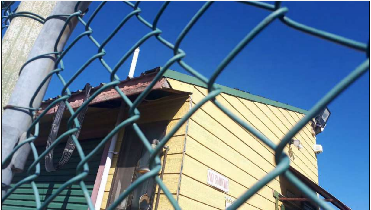
Plate 36: Equine pool shed (Building 11) to be demolished within the study area. Parts of the eave is missing on the northern side of the shed, allowing access into the roof space.
