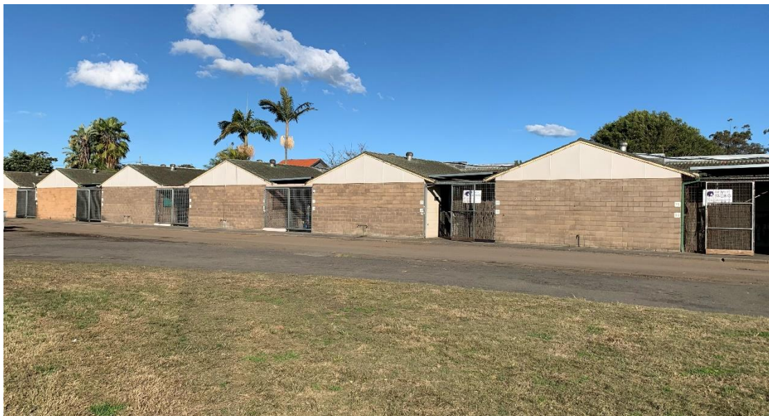
Photo 25: Existing Stables located on the south eastern corner of the NJC site
