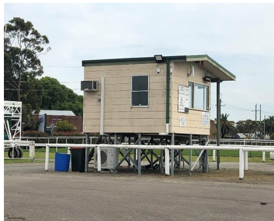
Photo 6: Track supervisor's office
