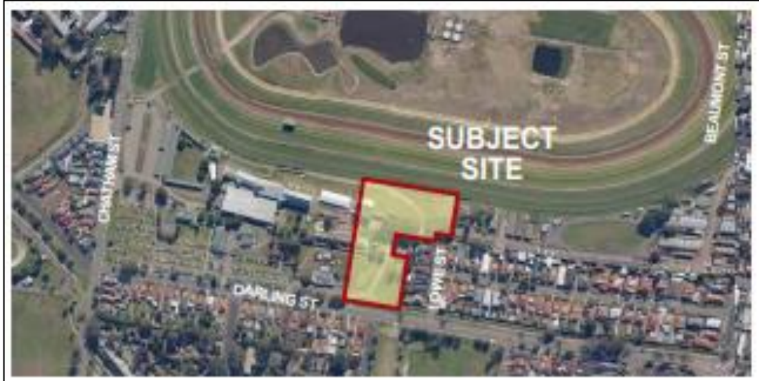
Figure 8: Location of recently completed race day facilities (Source: EJE Architecture)
