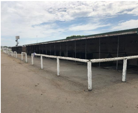
Photo 3: Brick tie up-stalls (west facing)
