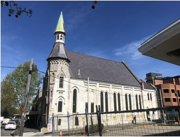
Picture 1 St Luke's Presbyterian Church (opposite the site)
