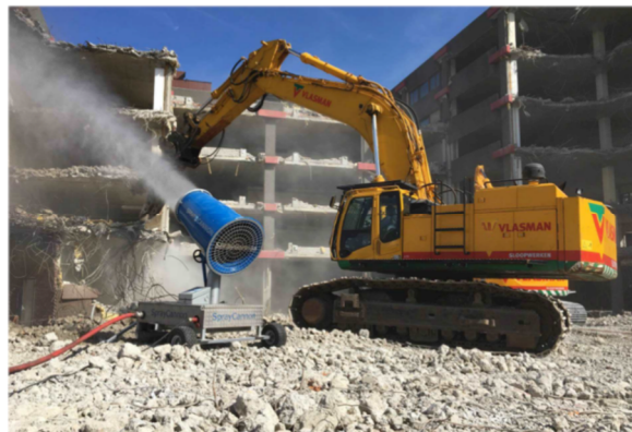
Example of dust control during demolition phase
