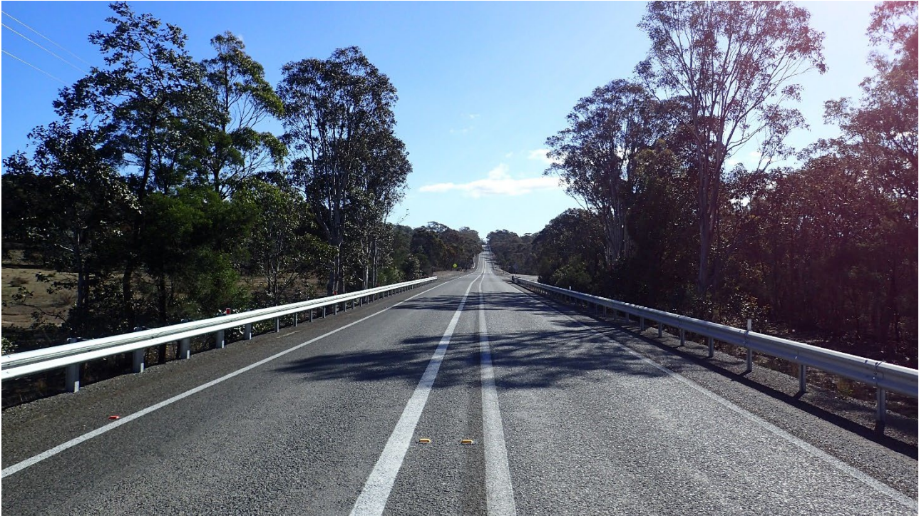
Photograph 2.1 Wide centre line treatment on Brayton Road (July 2018)
