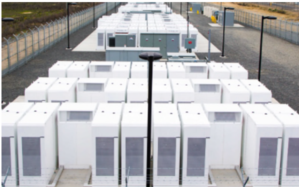
Figure 18-15 Example of typical BESS units (source: https://www.britishgas.co.uk/business/blog/tesla-mega-battery-activated-in-south-australia )
